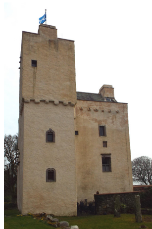
Above: Barholm Castle, Dumfries and Galloway. While originally a simple rectangular towerhouse, characteristic of lowland Scotland, the moulded window detailing to the later stair tower adds to the castle's historical and architectural interest. These features were successfully incorporated into the residential restoration completed in 2006.
