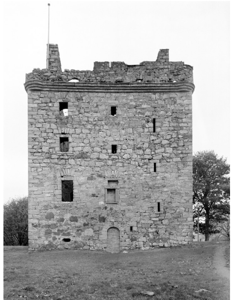
Law Castle, North Ayrshire. Restoration of the 15th Century Law Castle in the 1980s required a series of considered interventions such as the installation of a new roof and partial re-building of the parapet. The existing window openings were re-used, avoiding the need for new openings. A harling was also applied to the restored building. Top: © John Buchanan Smith/Scottish Castles Association. Bottom: © Crown Copyright: Historic Environment Scotland.
