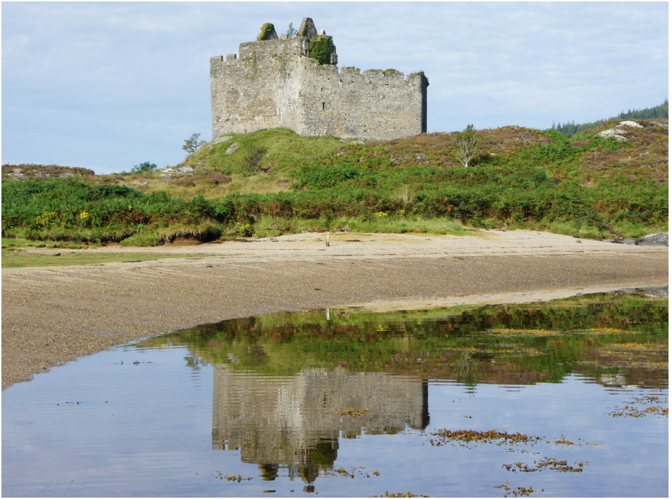
Above: Castle Tioram, Highland. Consideration of the most appropriate method of preserving the cultural significance of a castle for the future will involve a discussion on the merits of consolidation versus restoration. Each case is considered on its own merits. © Peter Drummond.
