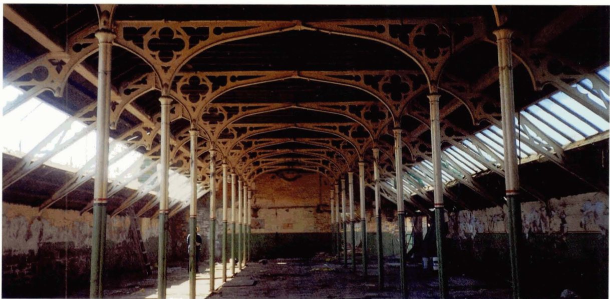
Illustration 55 South Mills, Dundee: New Mill (1851-7, extended 1864 and 1874). A 'Gothic' cast iron framed attic Reeler used structure housed powered reel spinning machinery. Good natural light from above was required so that the reeler could see flaws in the yarn. Large beam spans were not needed for the floors below because the spinning frames were static, though heavy, and unlike the 'mules' used for cotton and wool, did not move backwards and forwards on tracks. About a dozen attics of this type were built in the Dundee area (Picture: Mark Watson, Historic Scotland)
