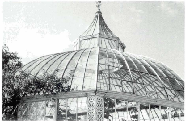
Illustration 267 Kingsknowe Hotel conservatory Decorative cast iron facing panel. The panels conceal the timber and iron posts within the conservatory walls (Picture: T. Swailes)
