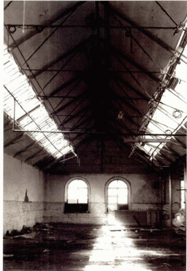
Illustration 56 Seafield Works, Dundee: West Factory (1859) Internal view of weaving shed: The Seafield Works specialised in the manufacture of jute carpet. The High Mill has been converted to housing in 1988-92 but the single storey iron framed weaving sheds demolished. (Picture: Mark Watson, Historic Scotland)
