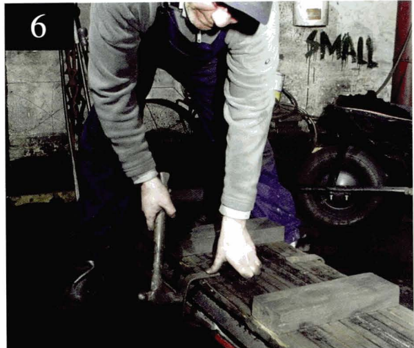
Clamps are fixed, prior to turning over
