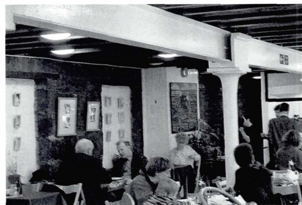
Illustration 68 The 'Edinburgh and Dalkeith ('Innocent') Railway Goods Shed and Terminals (c.1840) Steel beams on cast iron columns, over the cafe at first floor level. The steel beams replace early timber beams and bear the rolling mark LANARKSHIRE STEEL CO LD SCOTLAND 12 x 6 (Picture: T. Swailes)
