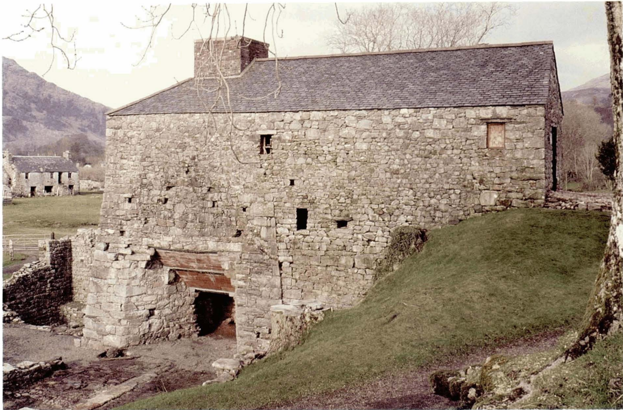
Illustration 23 Bonawe Ironworks Casting house and furnace (Picture: Historic Scotland)
