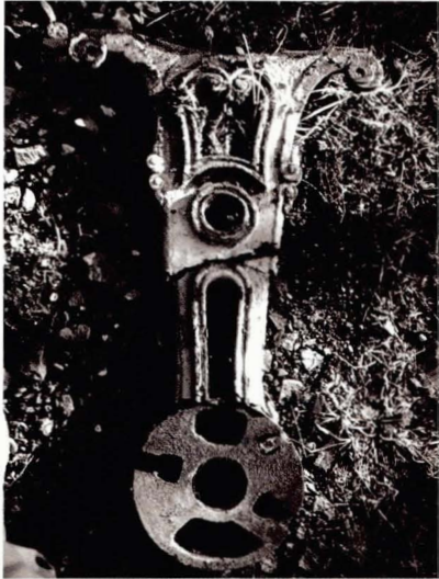
Illustration 71 Haymarket Station Edinburgh (1840). A broken cast iron strut from a roof truss in storage at the Bo'ness Heritage Area where most of the trainshed is now re-erected. The cover plate has been removed, showing anchorage slots for 'upset' iron tie bar ends. (Picture: T. Swailes)
