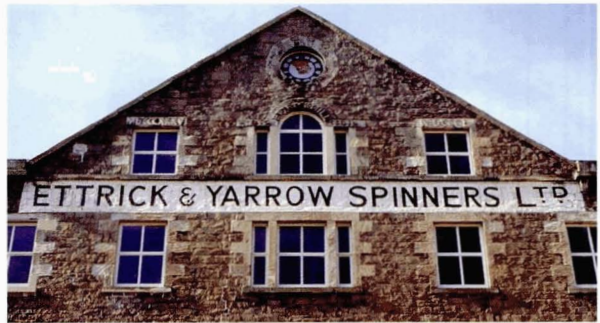
Illustration 41 Ettrick Mills, Selkirk (1835 and 1850) Front gable elevation, with date stones. Built as a mule spinning woollen mill in 1835, with timber floors on cast iron columns, extended in 1850. The fireproof floors in one of the 1850 wings are unusual in being built of local whinstone rather than brickwork (Picture: Shannon Tofts)
