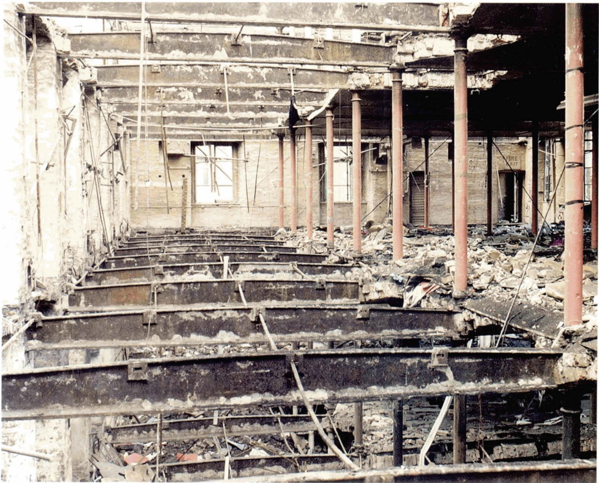
Illustration 199 Havelock Cotton Mill, Manchester (c.1845) Iron framing exposed during demolition in 1995 (Picture: Joe Marsh, UMIST)
