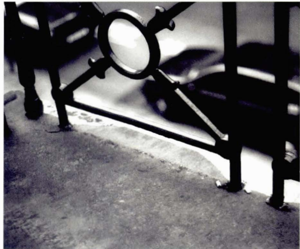
Illustration 247 Spalling and (structural?) repair of stone balcony slab, caused by expansion (thermal or corrosion related?) of inset cast iron railings (Picture: T. Swailes)
