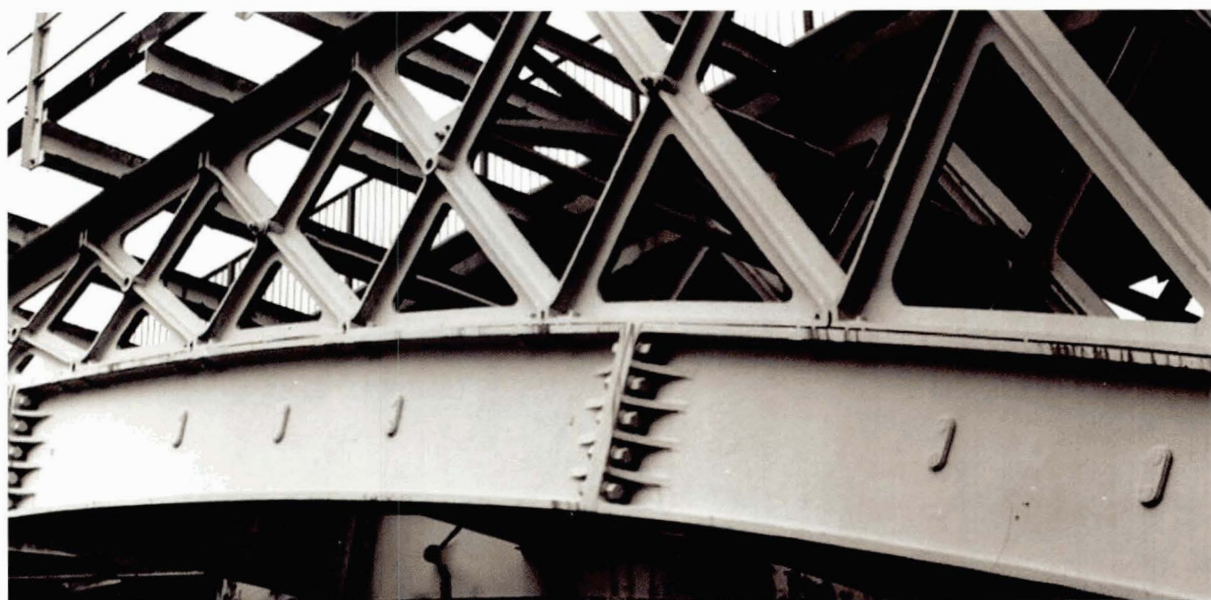
Illustration 116 Carron Bridge (1863) Structural ironwork details. (Picture: Mark Watson, Historic Scotland)
