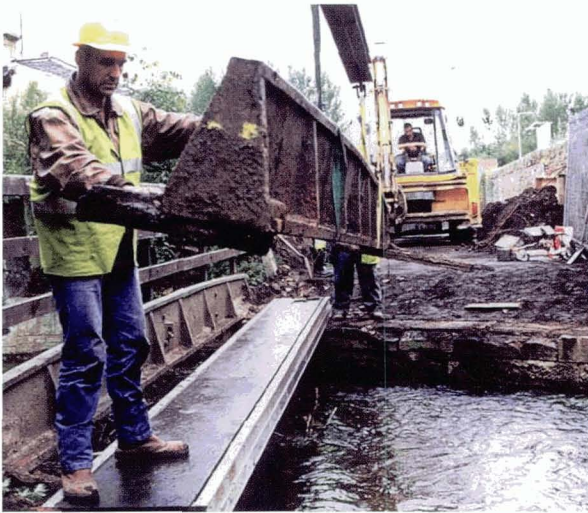
Illustration 127 Edinburgh & Dalkeith Railway, Braid Burn Bridge (1831) General view. Made and erected by Shotts Iron Co. in 1831, the bridge was conserved in 1983 by Lothian Regional Council and raised in level in 2001 (Picture: New Civil Engineer/Roland Paxton)
