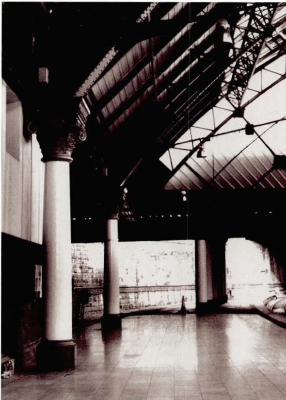
Illustration 78 Queen Street Station, Glasgow: Main train shed roof (1880) Tied wrought iron arches on cast iron columns. Designed by the civil engineer James Carswell, with steel tie bars to the principal wrought iron roof arches. (Picture: T. Swailes)
