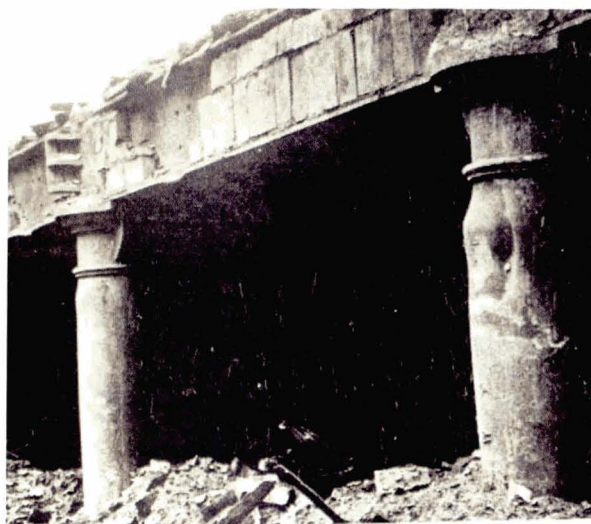
Illustration 243 Local bulging at the tops of cast iron columns as the results of high temperatures reached during a particularly severe fire (Kirby, 1986) (Picture: Mr. C. Ashton, reproduced by permission of Corus (UK) Ltd)
