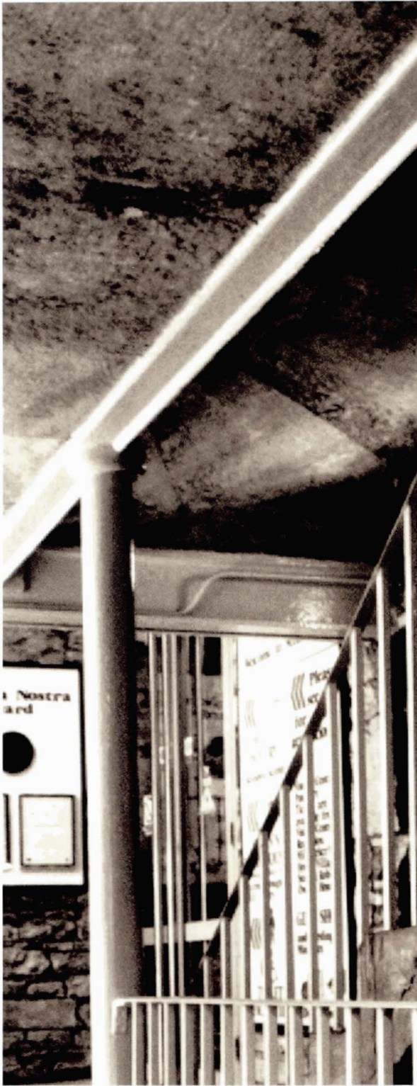
Illustration 35 New Lanark: East End of Mill 3 (c. 1826) Cast iron supports to stone stairs and landing. Mill 3 was built fireproof to replace a timber floored mill destroyed by fire in 1819. The east end of the building formed an iron framed firebreak against Mill 4 also destroyed by fire in 1883 (Picture: T. Swailes)
