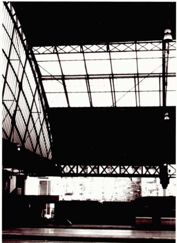
Illustration 79 Queen Street Station, Glasgow: Main train shed roof (1880). The gable screen and the cross-braced roof (Picture: T. Swailes)
