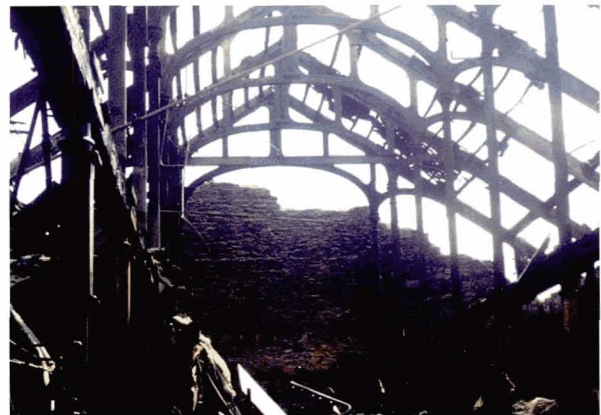
Illustration 139 Larchfield Works, Dundee (1865) The interior, destroyed by fire (Picture: Mark Watson, Historic Scotland)
