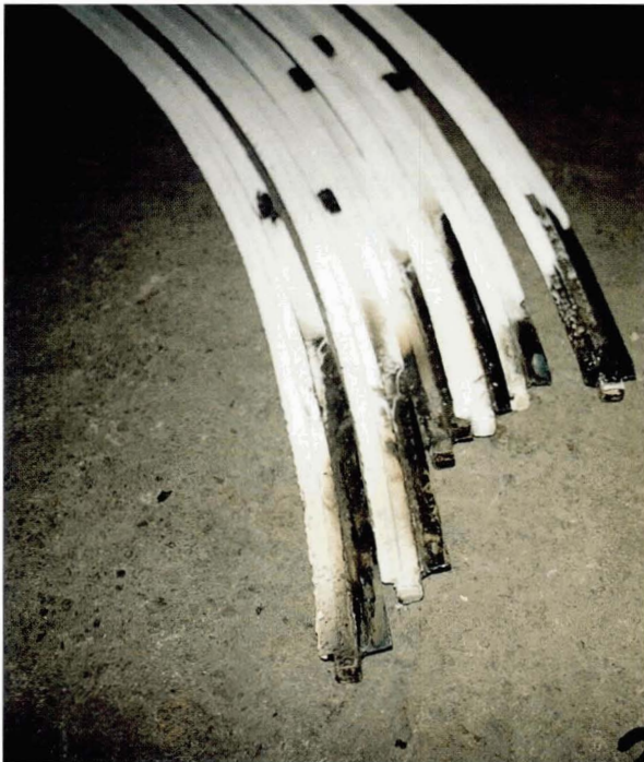
Illustration 263 Welded repairs to wrought iron glazing bar ends (Picture: Heritage Engineering Ltd)
