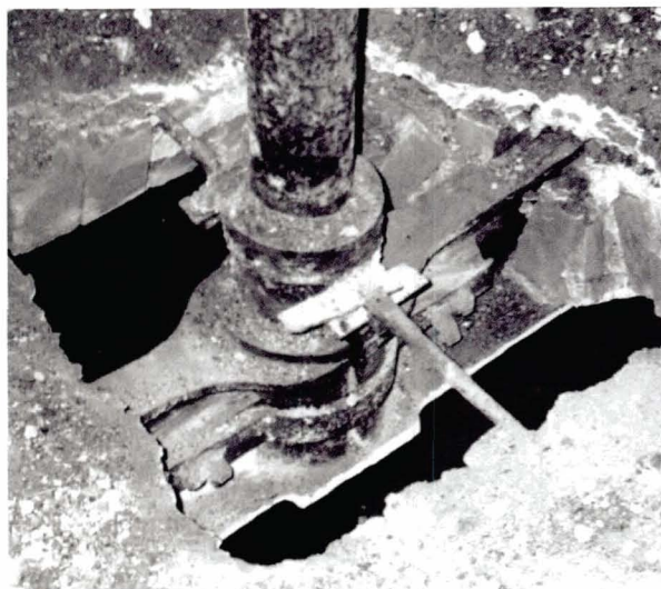
Illustration 142 Clarence Mill, Bollington, England (1854) Opened up beam-column connection (Picture: T. Swailes)
