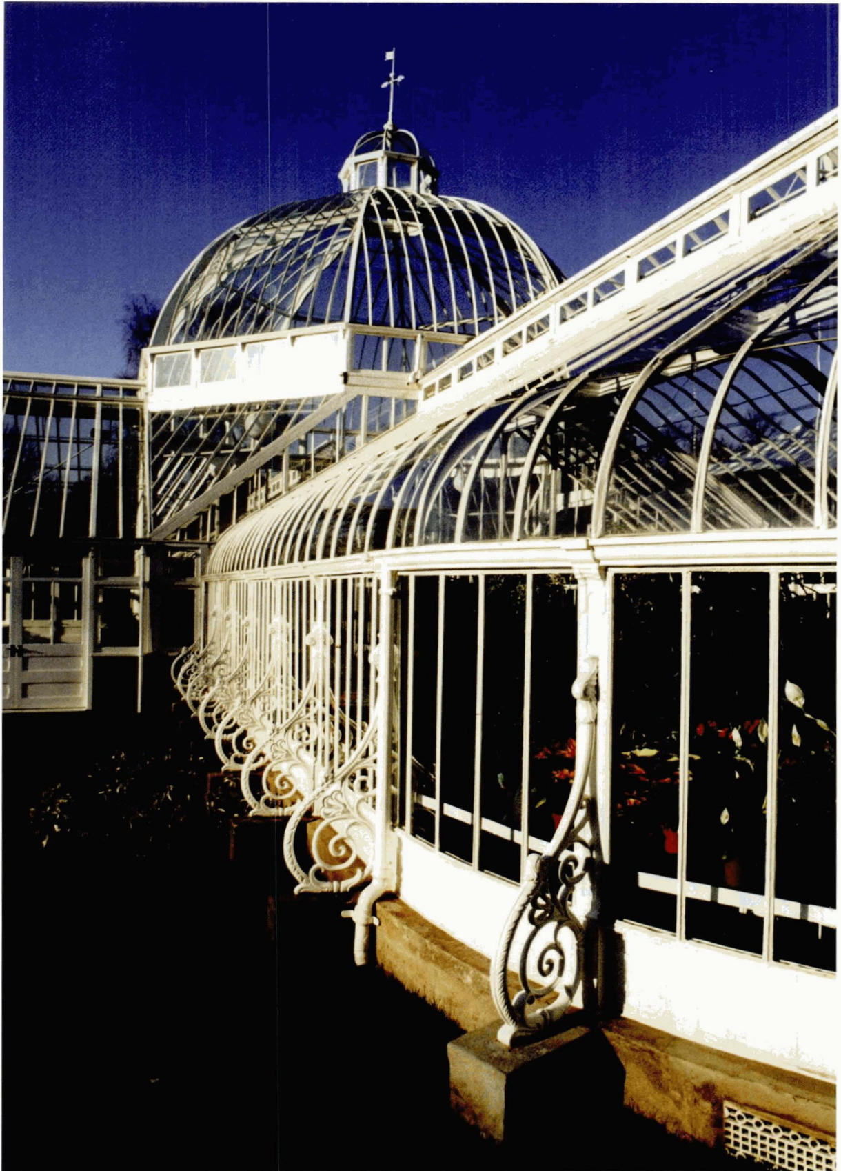
Illustration 101 Tollcross House Conservatory, Tollcross Park, Glasgow (1858) The structure after restoration (Picture: Heritage Engineering, The Industrial Heritage Co, Ltd)
