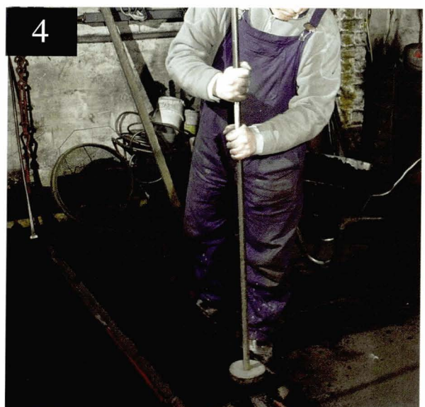
Ramming within the "Peg Rammer", a plain bar, is followed by ramming with the "Dog Rammer" (as shown)
