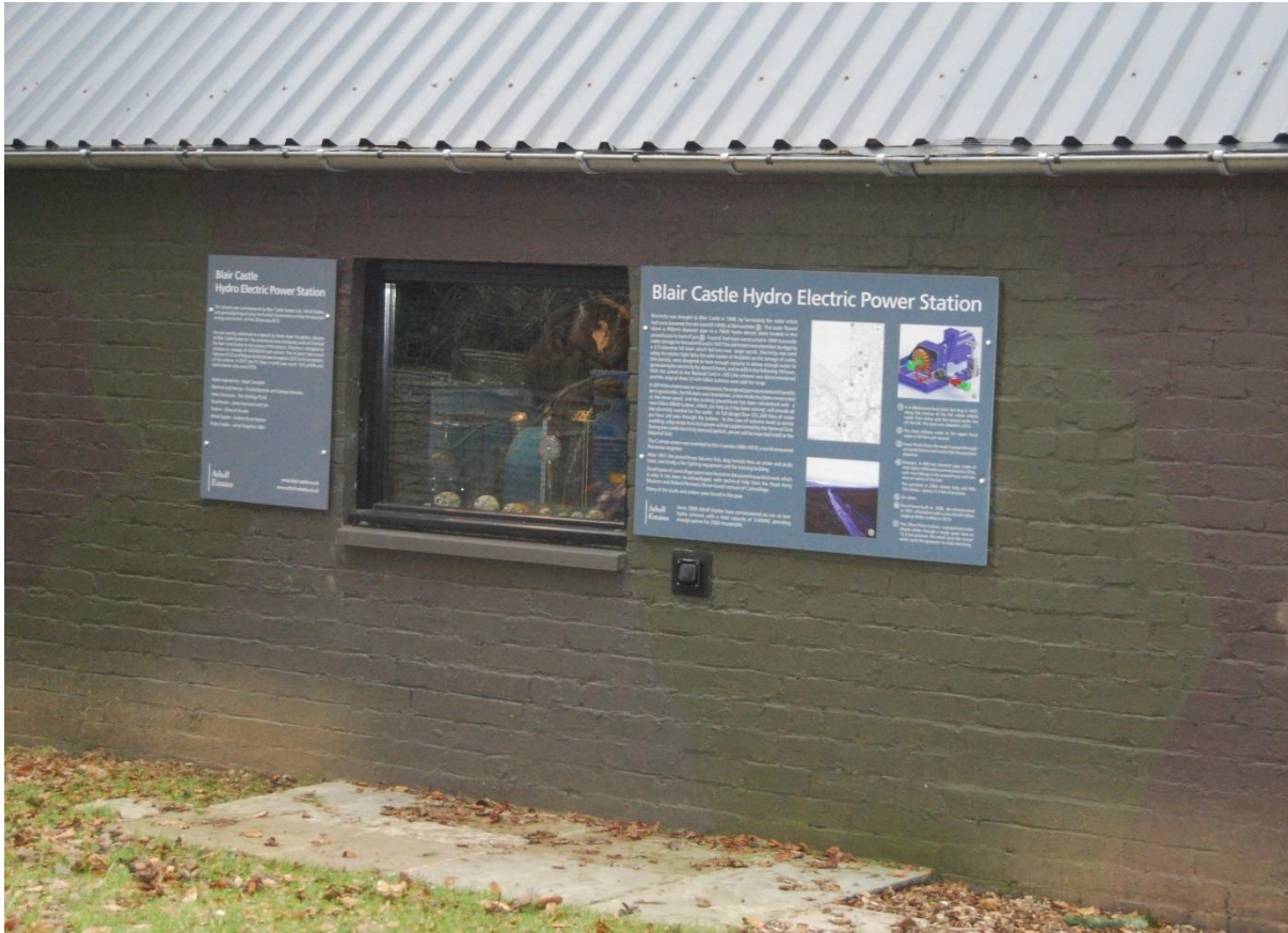
Figure 23: The interpretation board and the viewing window into the power house.
