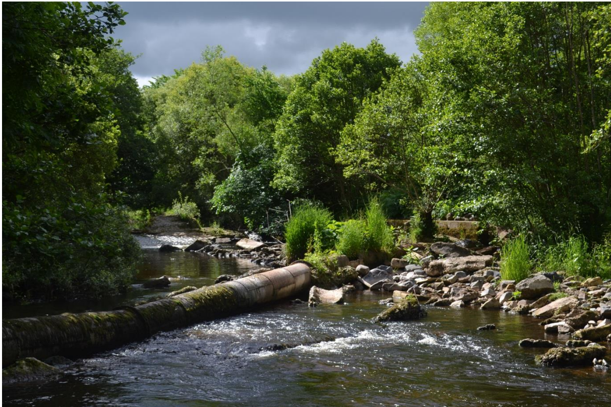
Figure 2: Remains of the steel penstock for the Wells House hydro system of 1905. The remains of the cauld can be seen in the background.
