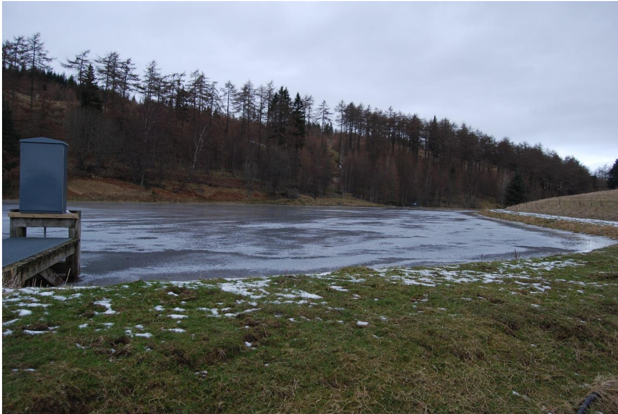
Figure 7: The larger holding pond (called 'Top Pond') for the turbine water supply, excavated in 1908.
