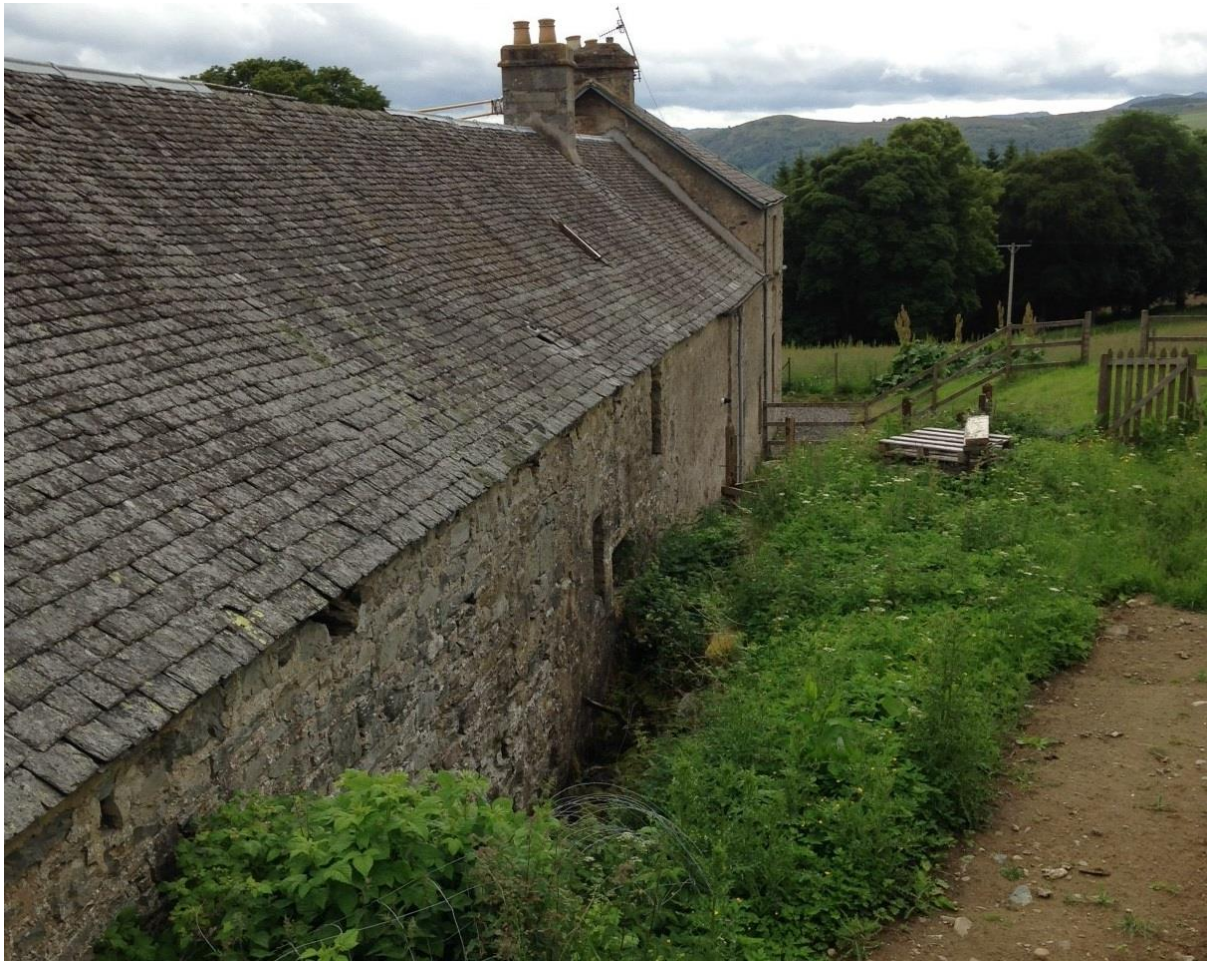
Figure 5: The former Estate sawmill at Blair; this was water powered until 1905. The wheel pit is visible in the middle foreground.
