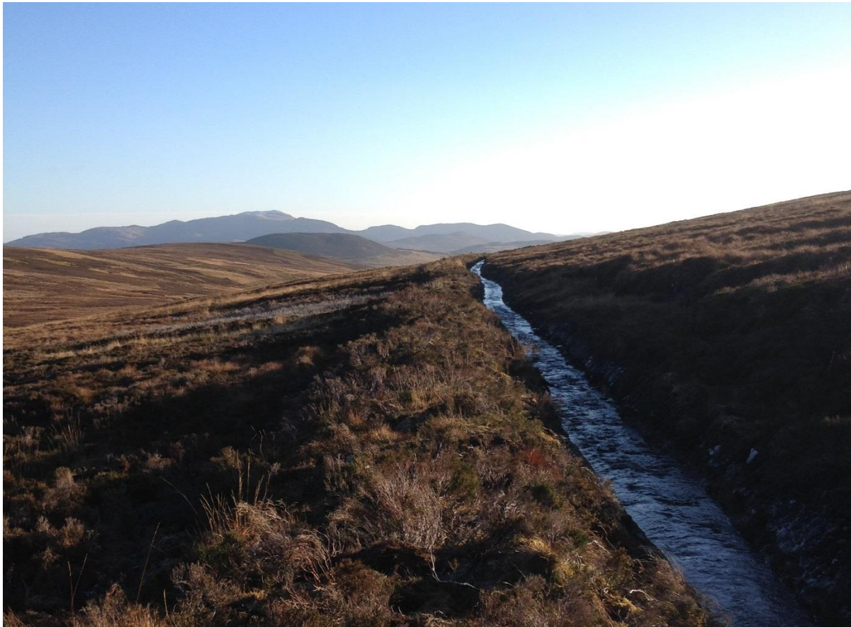
Figure 11: The recently cleared ditch on the hill above the castle, termed ‘the 4 mile ditch’ (image Atholl Estates).
