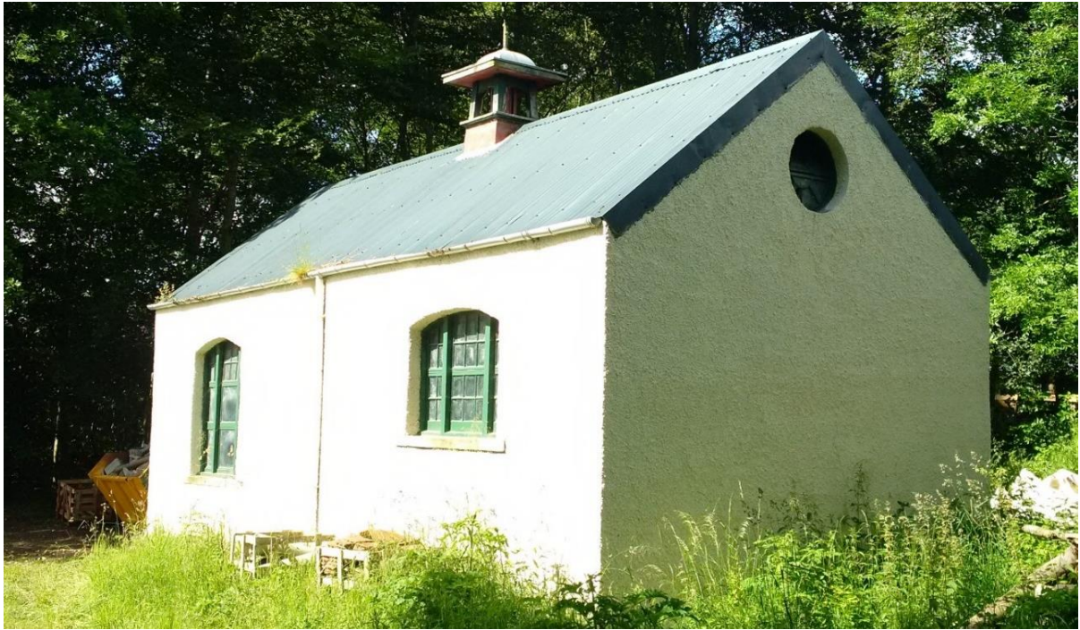
Figure 3: The former battery house at Wells.
