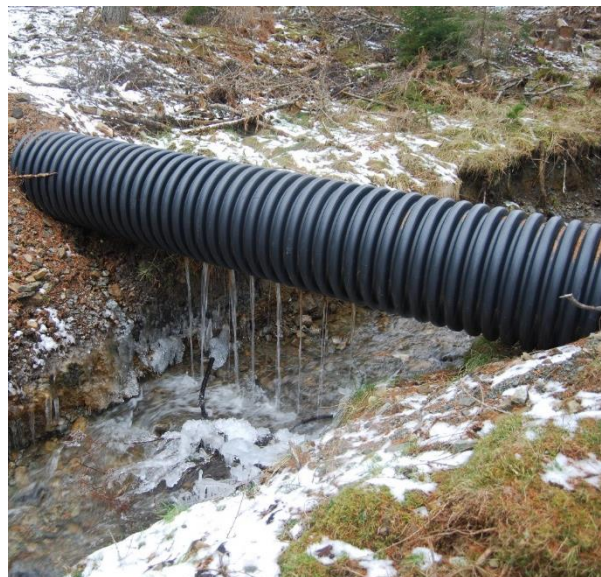
Figure 14: Surplus water management was important at all stages of the pond supply, and lower down the hillside new solutions were needed to route excess water clear of the pond.
