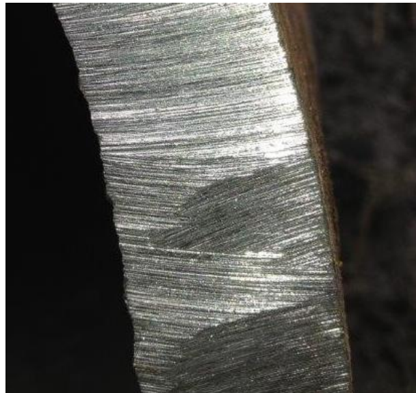
Figure 10: A close view of a cut through the 1908 steel of the penstock; the amount of corrosion was minimal (image Atholl Estates).
