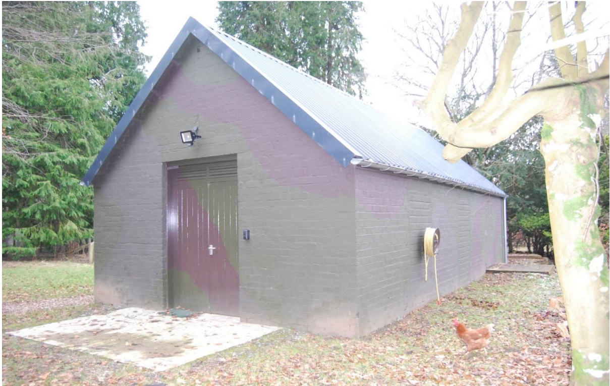
Figure 19: The restored power house in the re-instated disruptive camouflage pattern.
