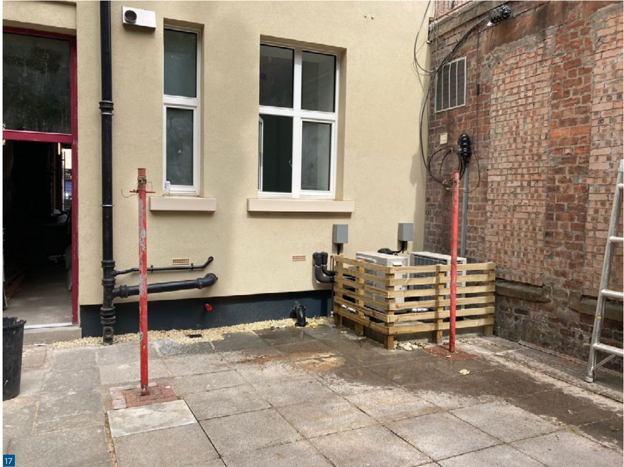
Figure 17. Closer view of the external units with rudimentary timber screening for protection.
