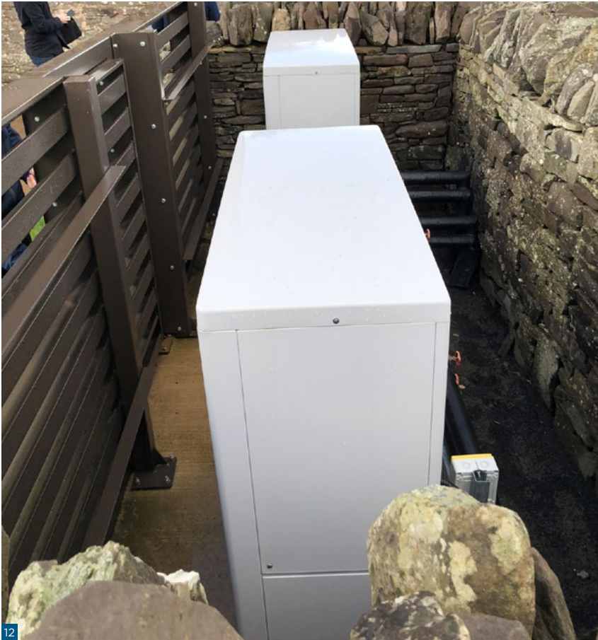
Figure 12. It is important to maintain suitable clearance around the ASHP within the enclosure.
