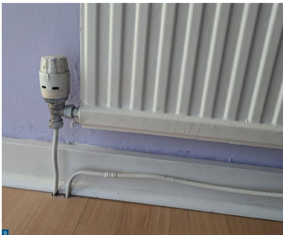
Figure 9. Microbore pipe connecting to radiator.
