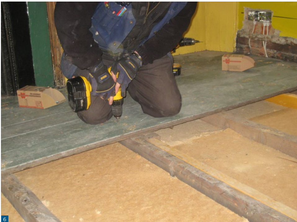
Figure 6. Floor insulation is one of the ways a building can be insulated before installing an ASHP.
