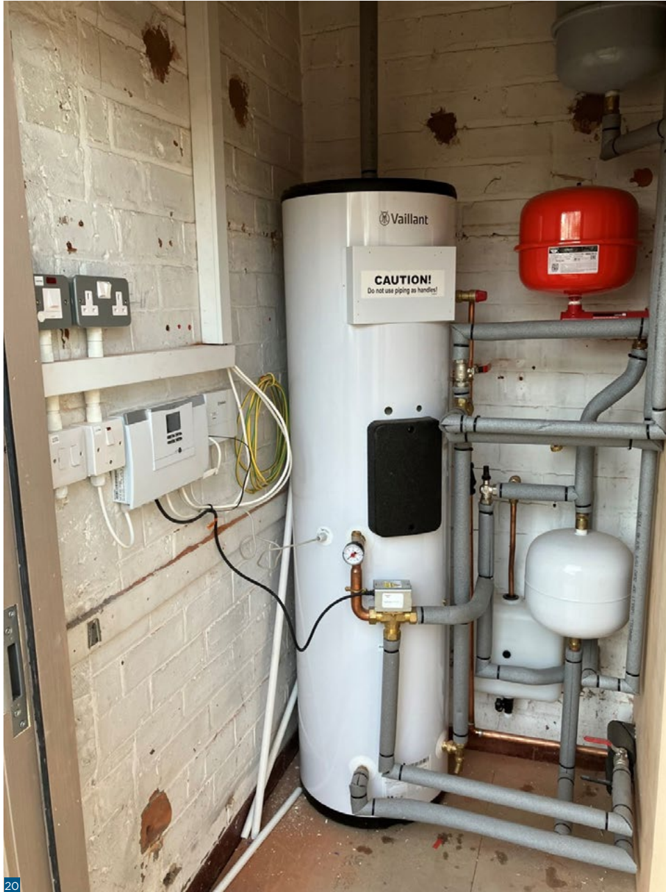
Figure 20. Image showing the internal cylinder and pipework within the shed, which was insulated as part of the works.
