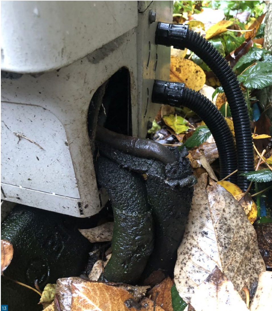
Figure 13. Damaged insulation increases heat losses from the system and should be repaired.
