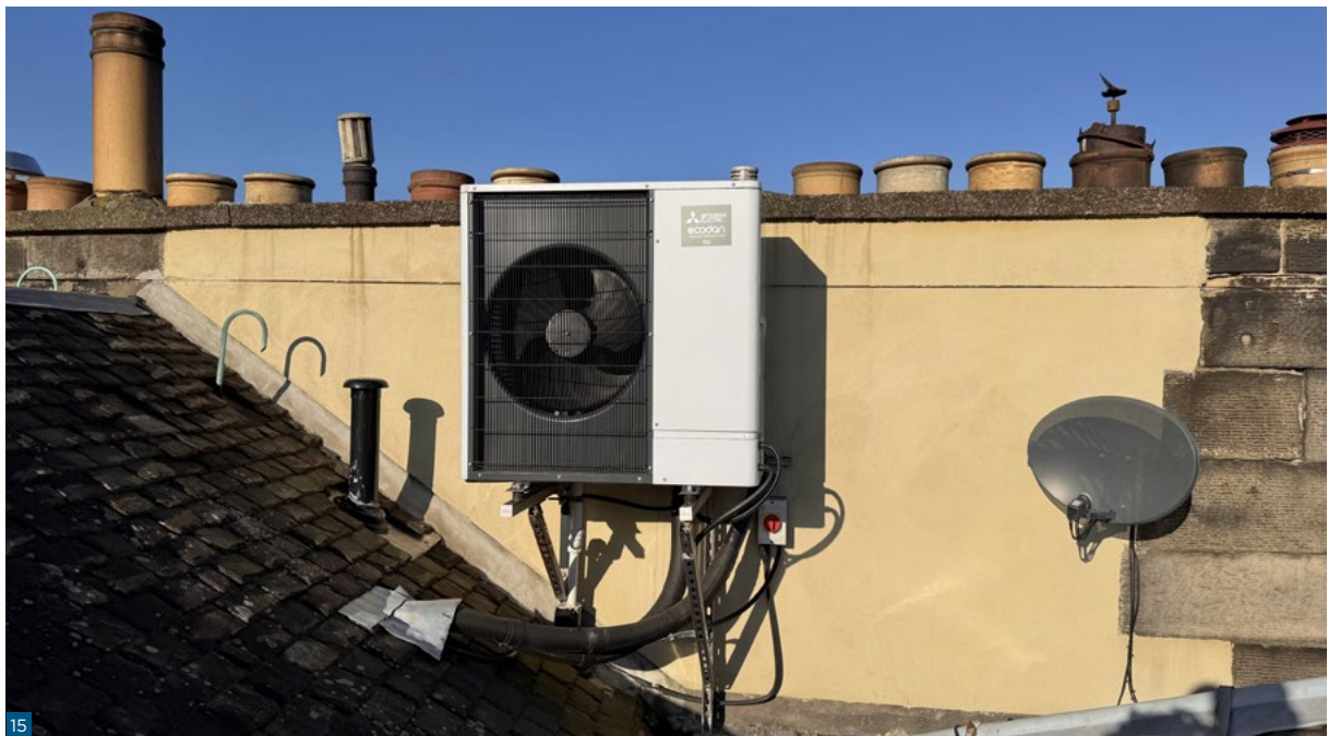
Figure 15. ASHP discreetly sited on roof (© John Jeffery).
