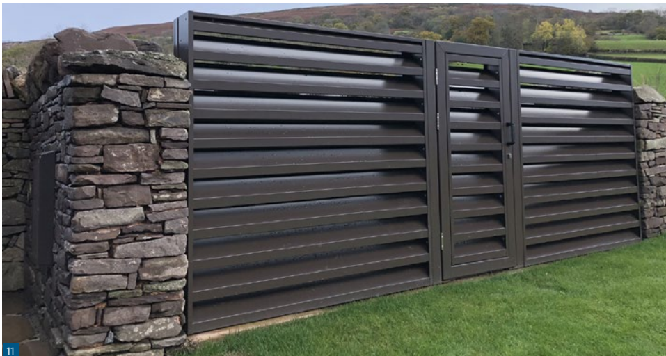
Figure 11. An example acoustic enclosure constructed outside a historic building.
