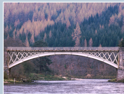
Carron Bridge, Moray, 1863: a railway bridge that is now a road bridge. An application to build a new steel arched bridge, and fix the outer cast-iron ribs to it, was withdrawn after it was found by calculation at a public inquiry to be unnecessary. The cross spandrels read through from side to side, so facadism was not going to work visually.
