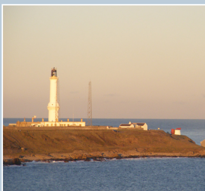
Girdleness lighthouse, Aberdeen, 1833, has typical keepers' houses, flat-roofed to emphasise the height of the tower, a compressor house and foghorn. A radio mast makes it a key part of the UK Global Positioning System (DGPS) and is not out of place.
