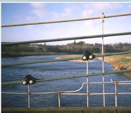
Union Bridge, Scottish Borders, 1821, the oldest suspension bridge still carrying a road, showing a clear distinction between the historic chain links and a 1920s wire cable. The deck is wooden and the parapets do not conform to modern standards. A weight limit and bollards exclude heavy vehicles.
