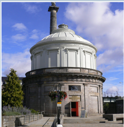
Perth Water Works, now converted for use as the Fergusson Gallery, has a cast-iron cistern made in 1832 that has recently been refurbished.
