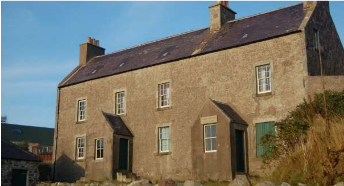
Figure 12: Brae House, Shetland, where the historic lime-based harl survives.
