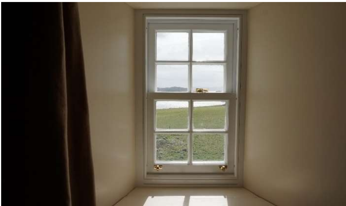
Figure 21: New slim profile double-glazed windows in situ.
