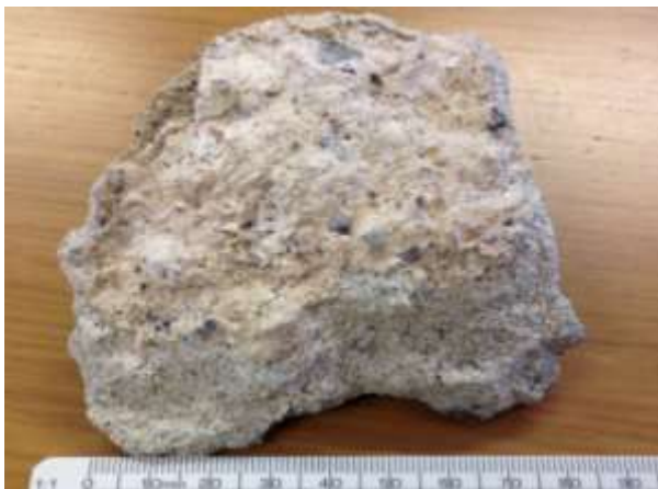
Figure 13: Traces of original lime-mortar finish attached to later roughcast.
