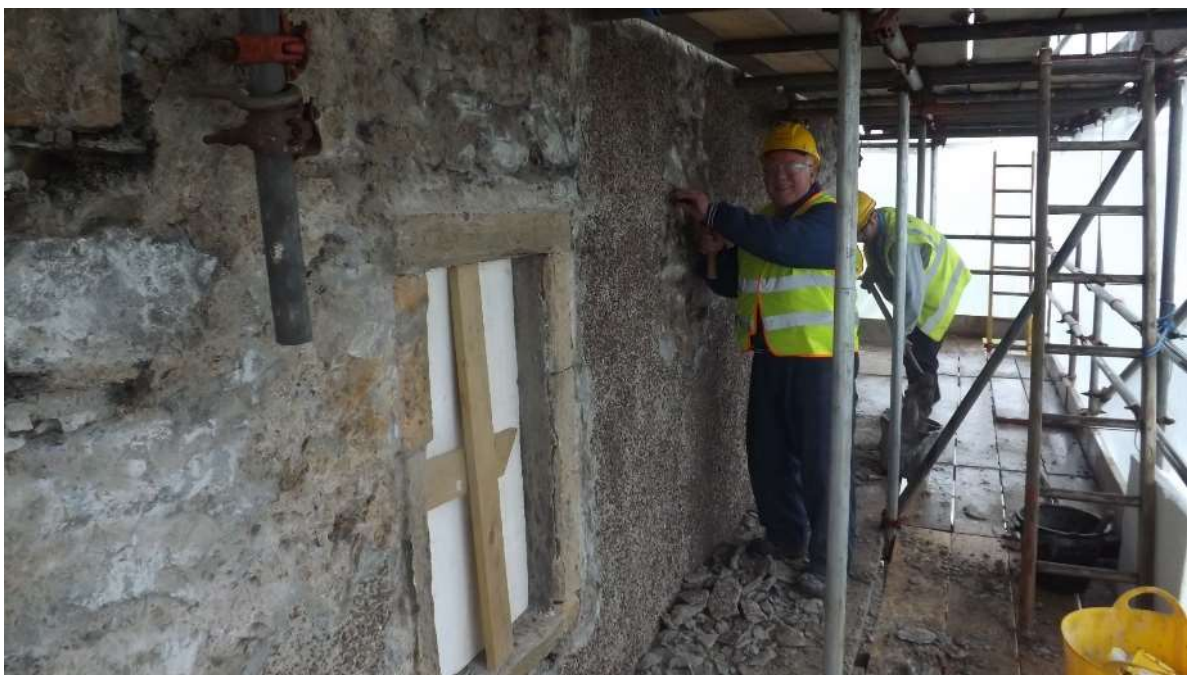
Figure 17: Removing the cement roughcast using hand-tools (Photo: Redman Sutherland Architects).
