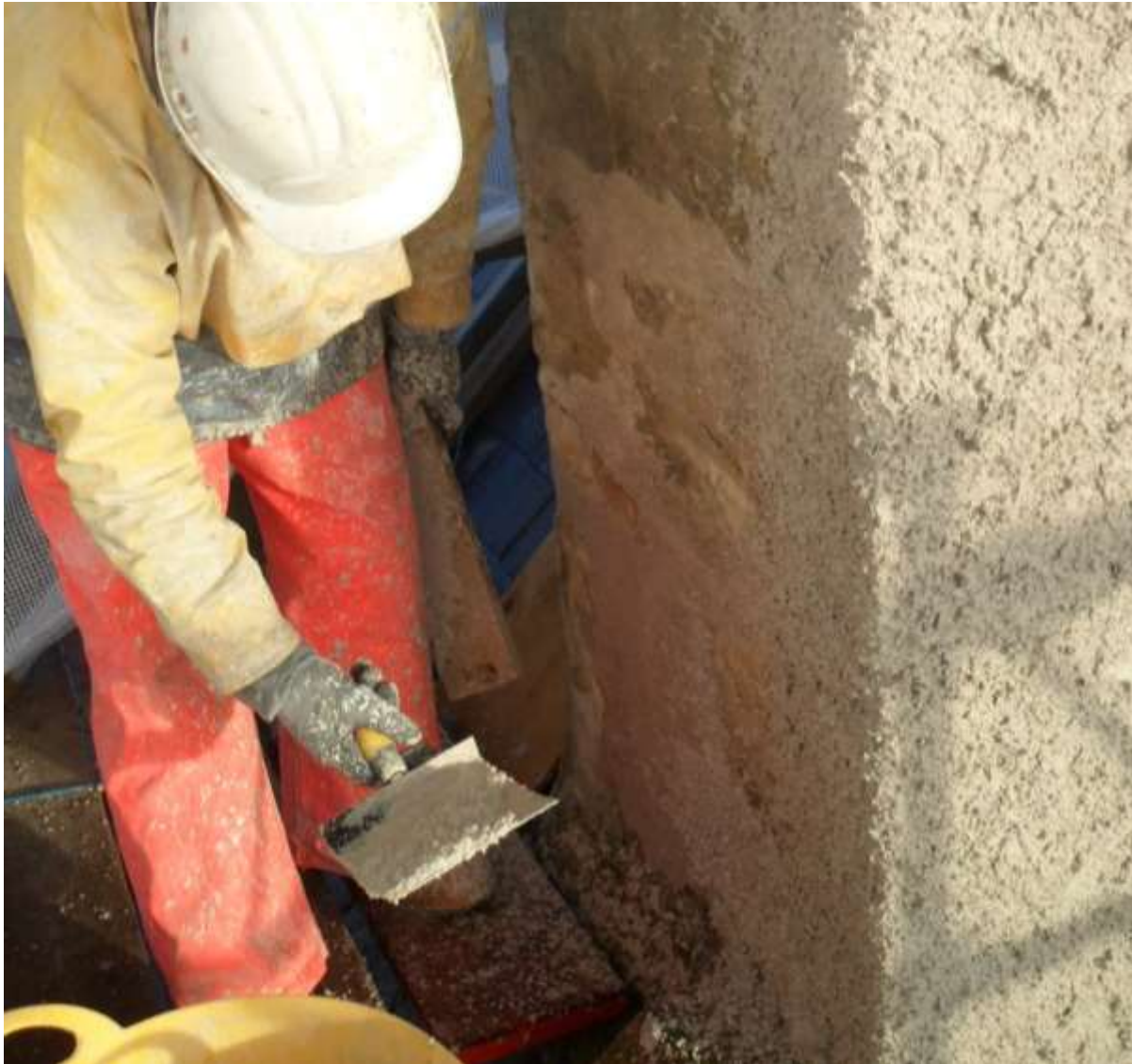
Figure 18. Re-harling the gable and chimney.
