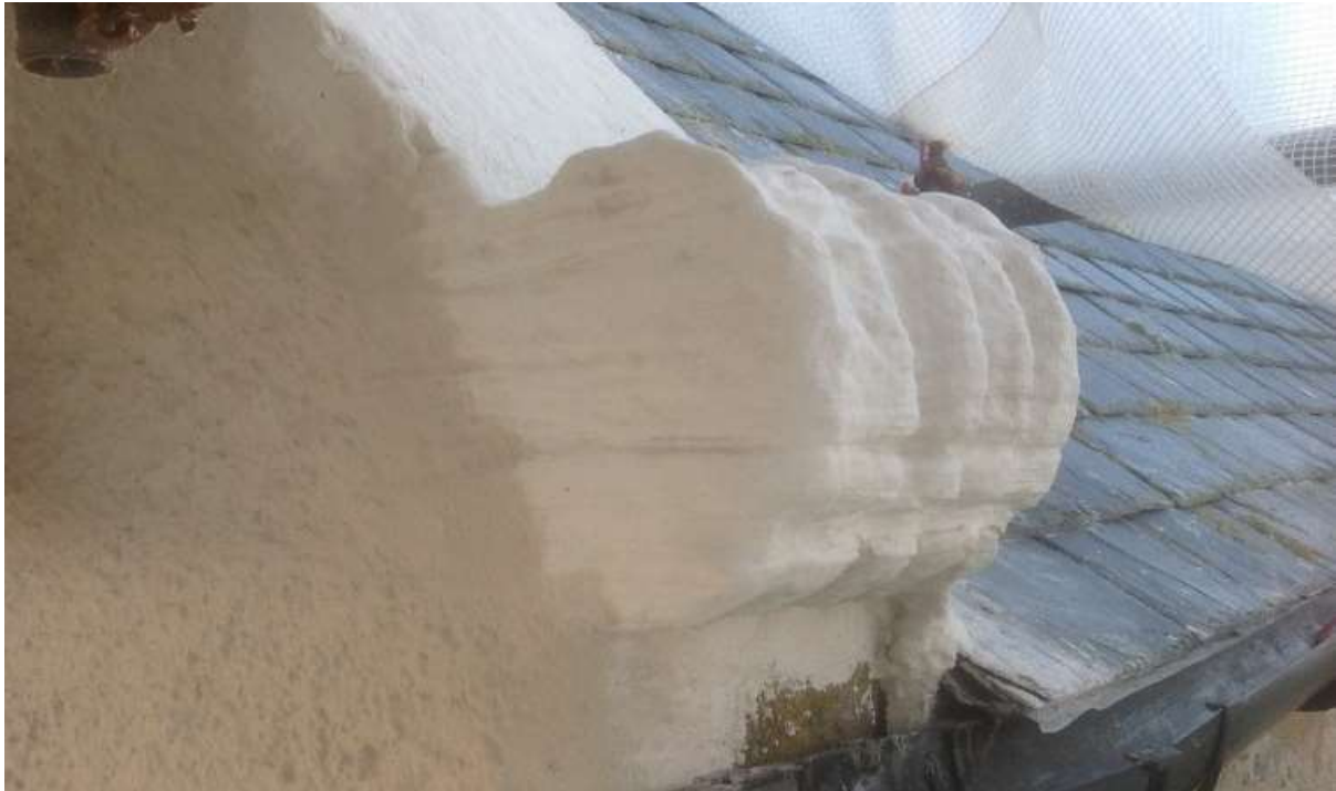
Figure 20: Limewashed decorative skewbutt detail.
