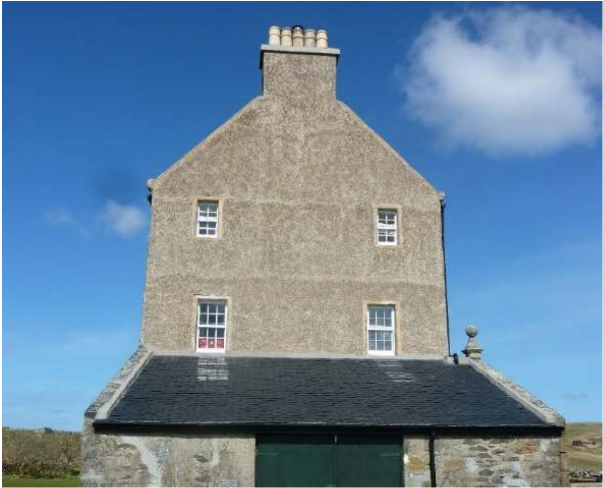
Figure 4: The exposed south east facing gable, prior to works.
