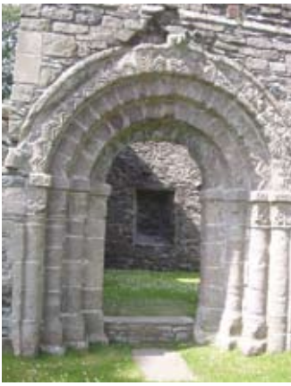
Doorway in the nave
