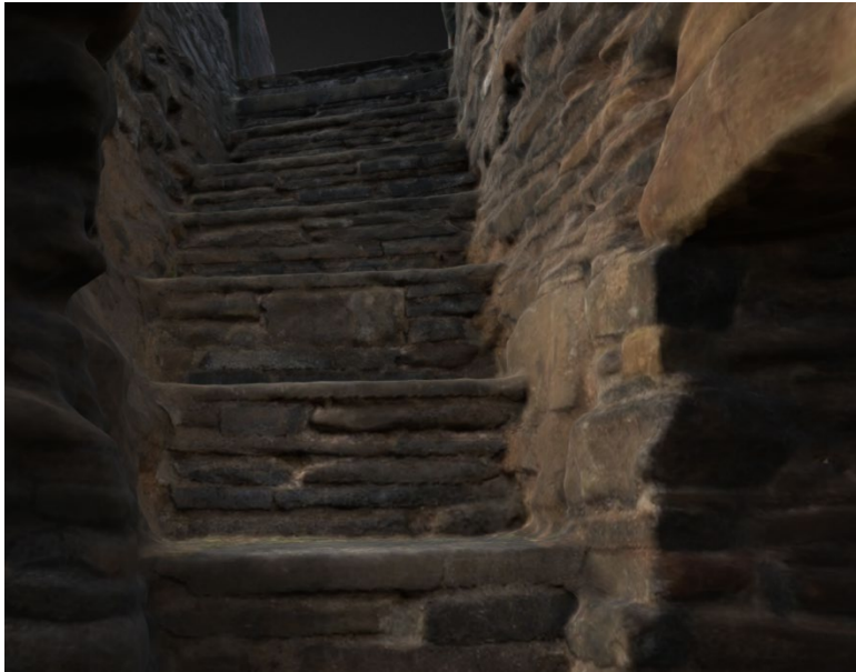
Figure 7 (right): Looking up the stairs towards the modern entrance. Only the lower steps are original (see Figure 2 section). Image is a screenshot from the photogrammetric model of the site, accessible via the HES sketchfab page. © Crown Copyright: HES
