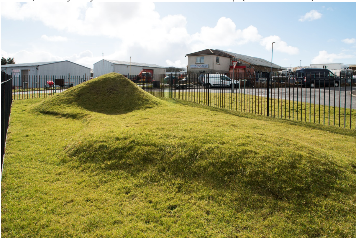
Figure 5: From the exterior, the site is visible as a grassy mound, within a fenced enclosure. The mound is of modern construction and indicates the ground plan of the subterranean structure beneath. The highest point of
