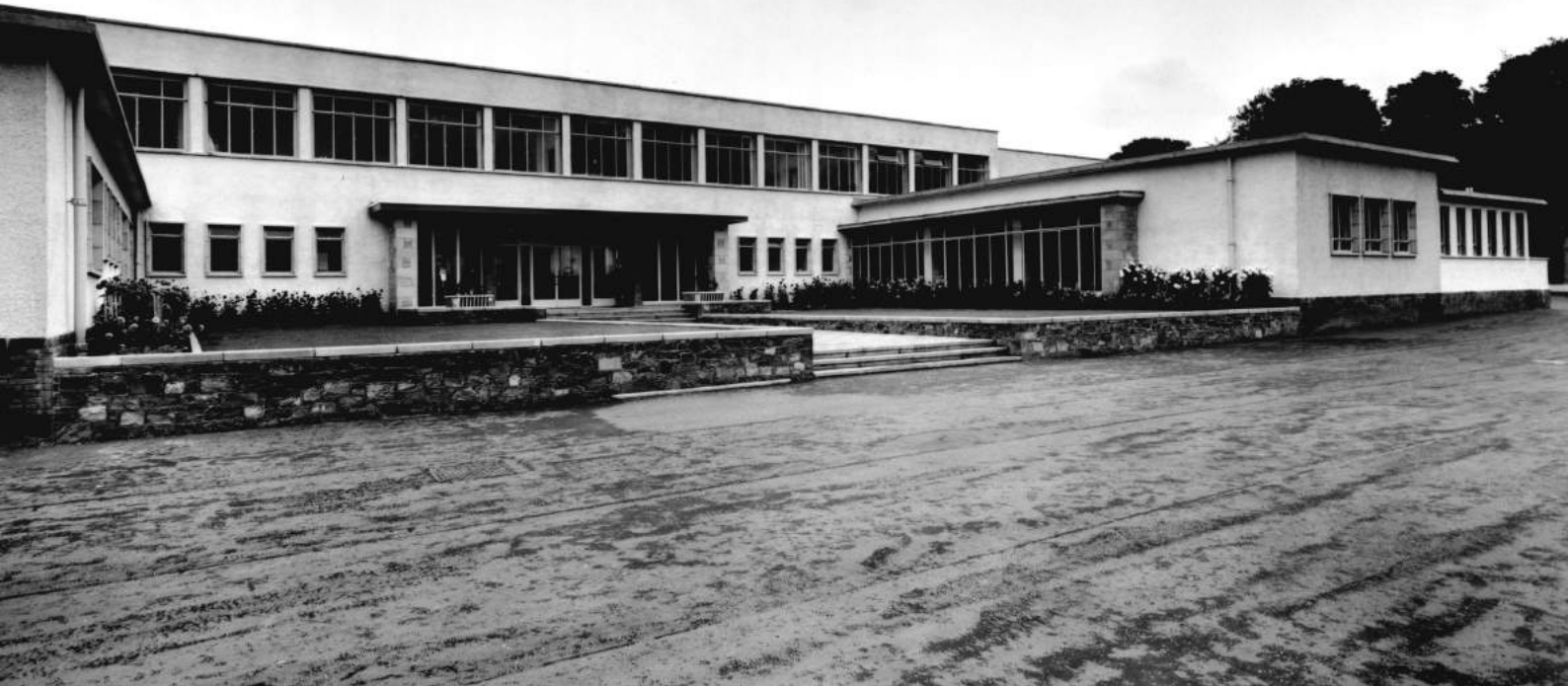
Above: View of the front elevation of the school c. 1955 ©Courtesy of HES (J and F Johnston and Partners)
