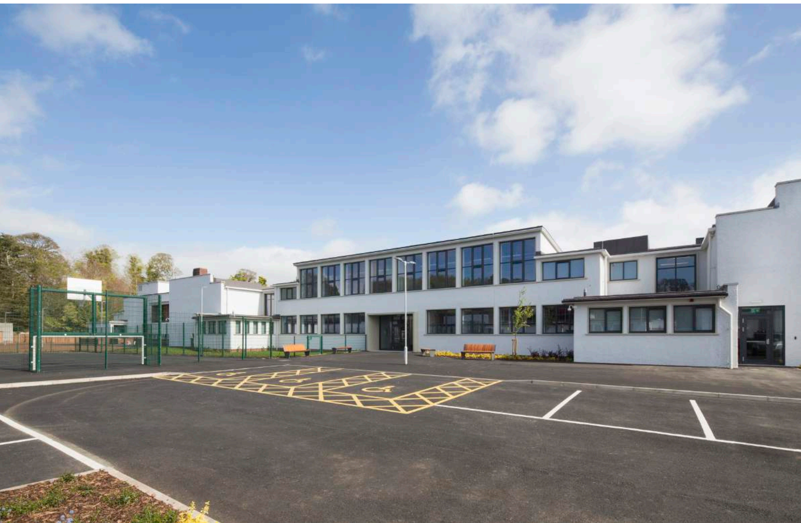
Below: View of the back elevation of the school after the selective demolition ©McAteer
