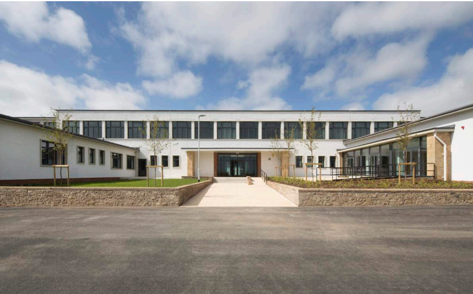
Below: View of the front elevation of the school after the refurbishment ©McAteer
