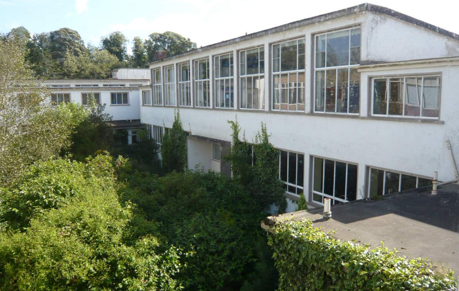
Above: View of the back elevation of the school before the selective demolition ©Courtesy of HES
