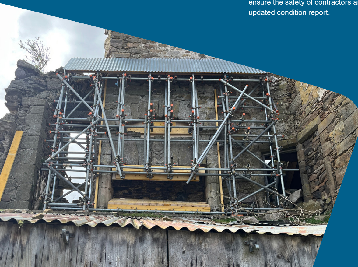
Hall Fireplace at Blervie Castle after stabilisation © Craig Anderson
