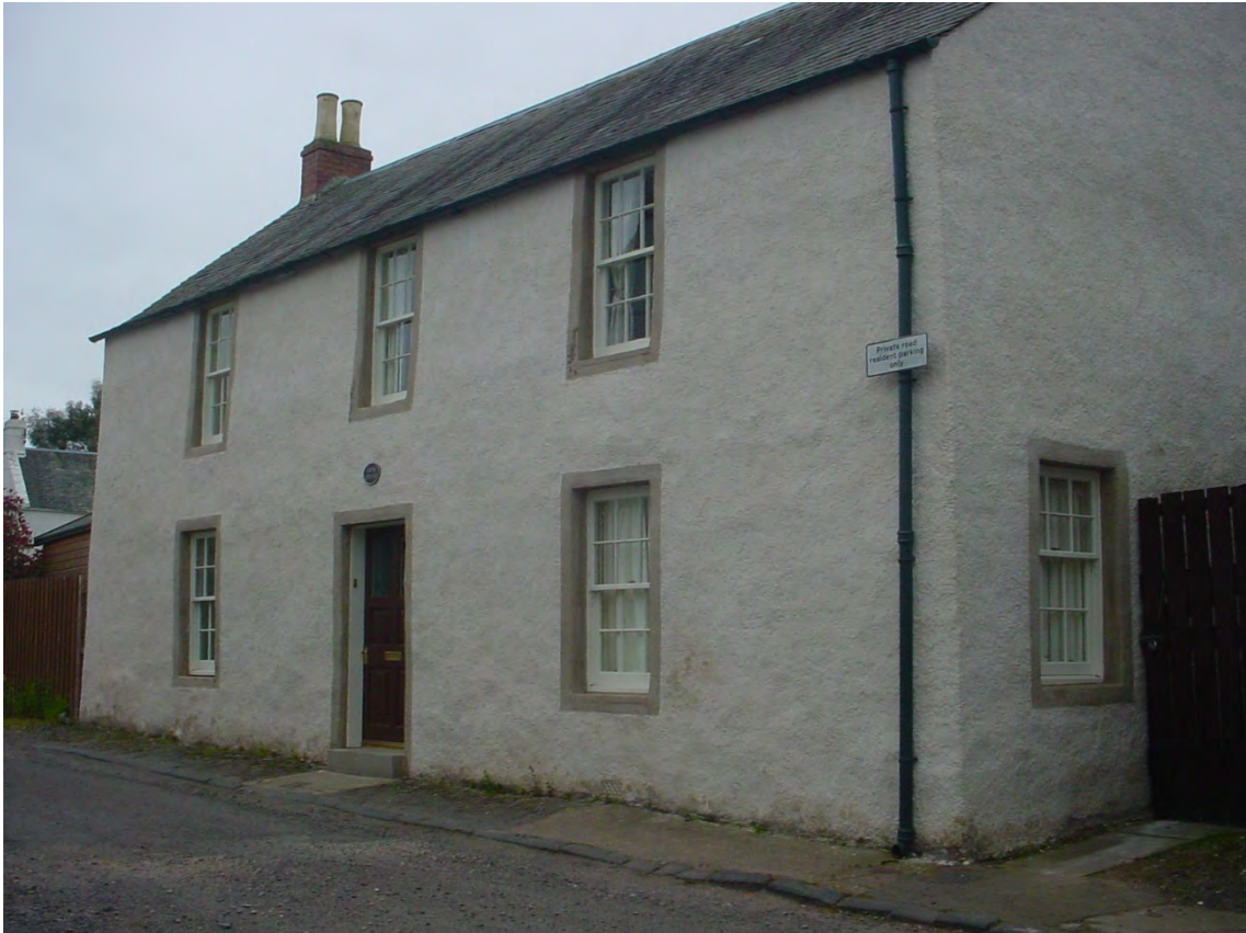
Figure 20: Gray House after the completion of works.
