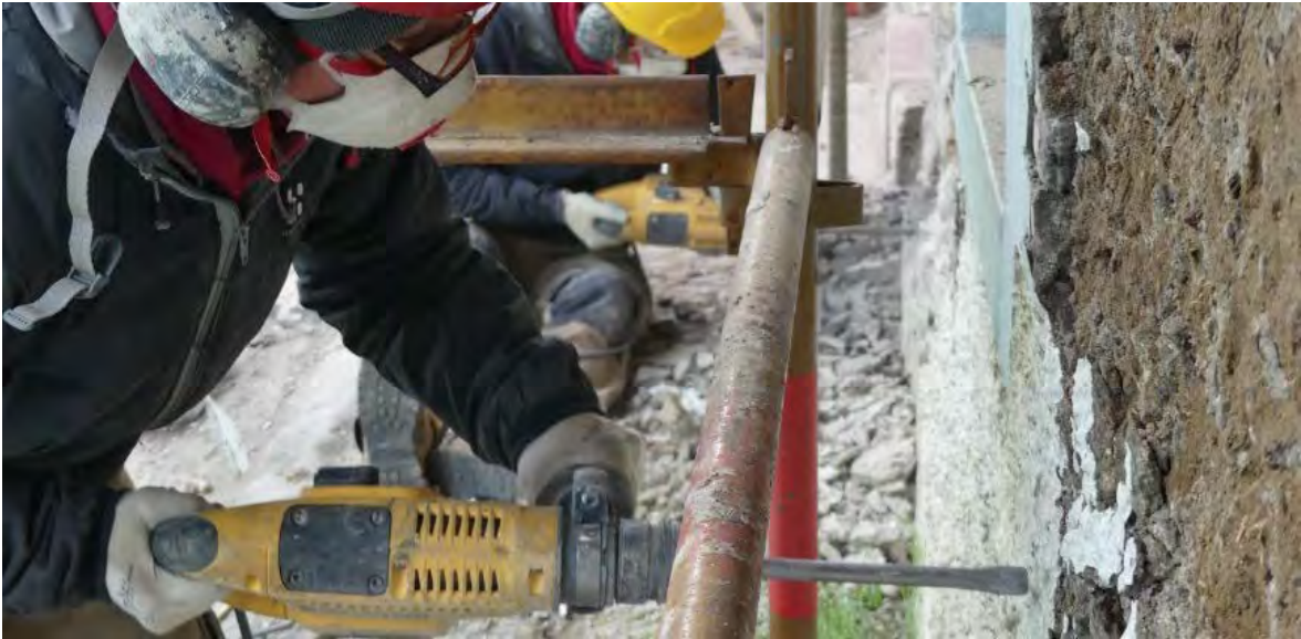
Figure 5: Removing the cement render.
