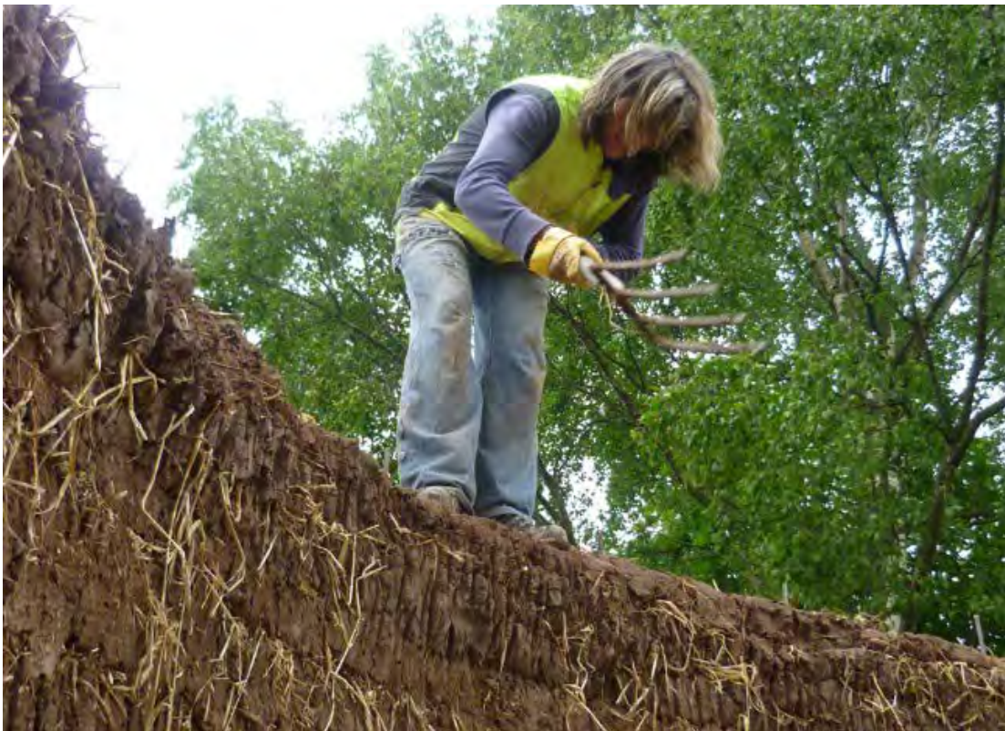
Figure 2: Mudwall being built in the traditional manner.
