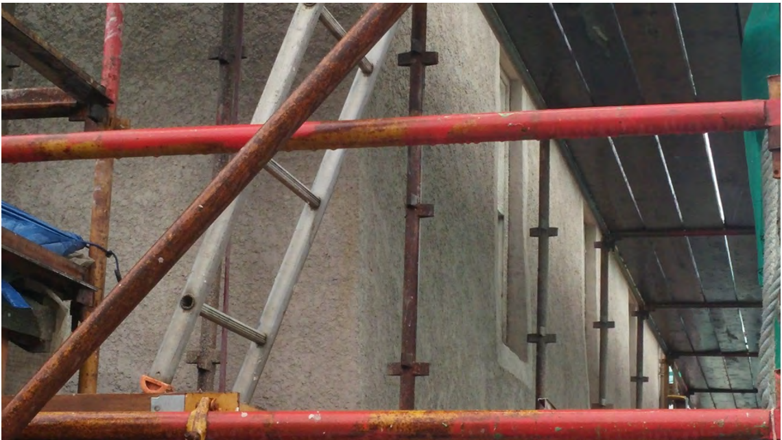
Figure 17: The harling was completed around the scaffold without visible lift lines.
