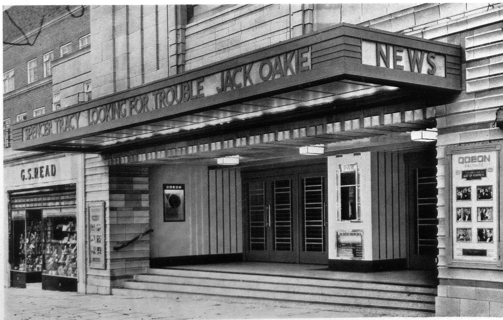
S.G. 920. Canopy in wrought iron and steel with cast light-alloy interchangeable lettering backed with opal glass and illuminated from behind. The combined soffite and roofing are built up in leadcoated sheet steel, and the coved soffite border is hinged in long lengths to give access to strip-lighting
