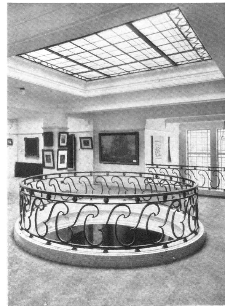
S.G. 320. Circular Well Balustrading in wrought iron with running scroll-work forged swept and welded. Bronze handrail (Section 2, No. 18). Rosettes in fine cast iron
