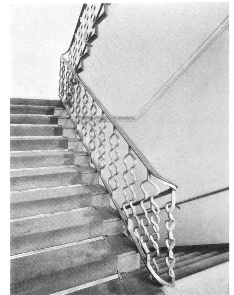
S.G. 321. Narrow Well Balustrading in wrought iron with corkscrew features forged and welded. Bronze handrail (Section 2, No. 16). Cranked fixings to string of stairwell
