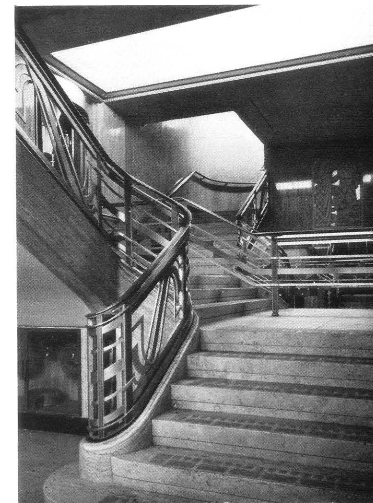
S.G. 322. Staircase Balustrading in wrought iron with heavily forged S scrolls interlaced and running continuously. The main uprights are fitted with machined steel edgings. Bronze handrail (Section 2, No. 17)
