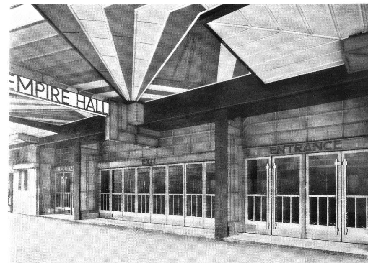
S.G. 419. Batteries of Main Entrance Doors, boxed illuminated Transomes and dividing Pilasters executed in wrought iron and steel, cellulose finished. Tubular handle bars and kicking plates are in mirror polished stainless steel. Double action floor springs fitted to doors throughout
