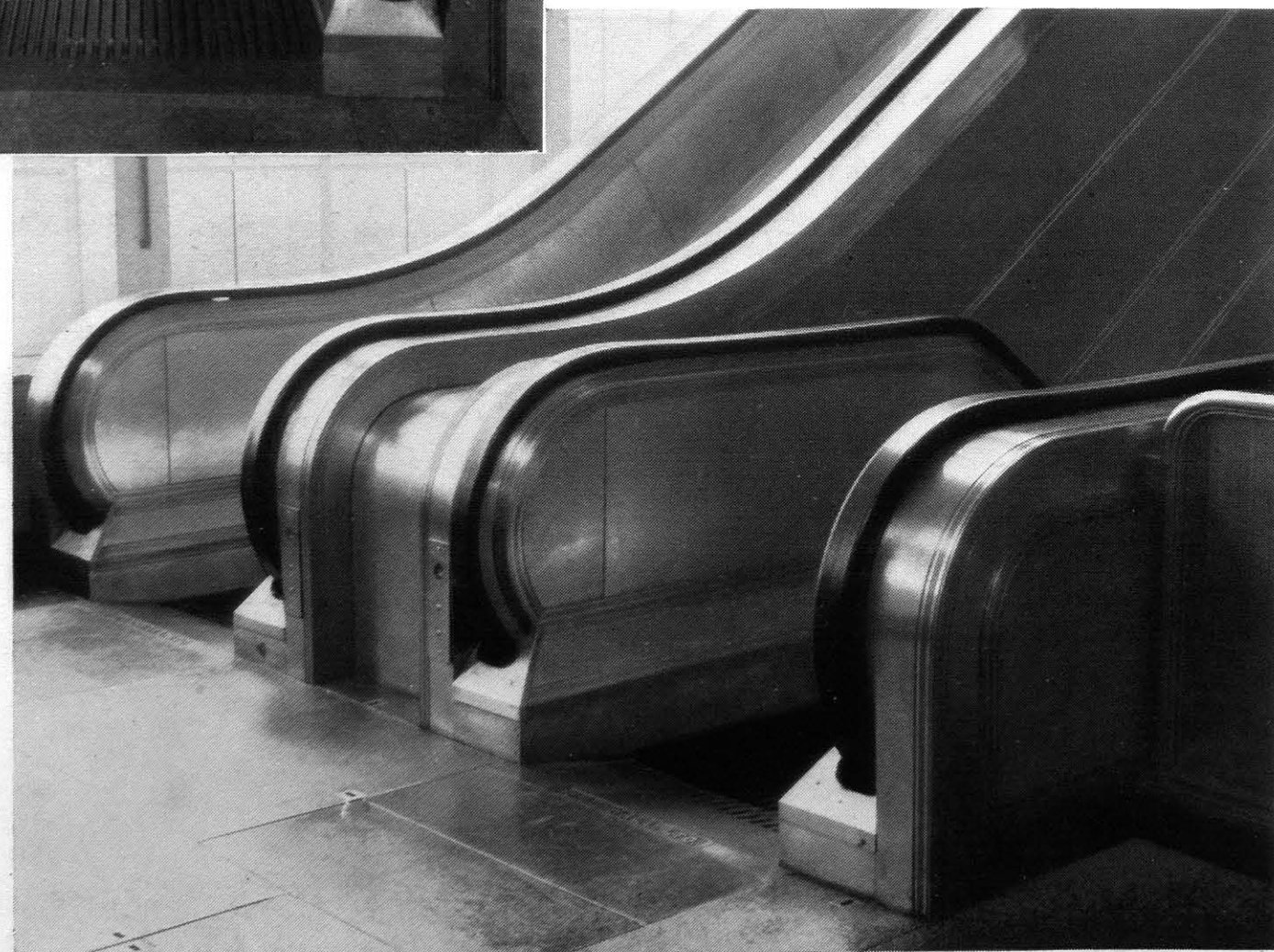
S.G. 9020. View of Escalators arriving and leaving at first floor. The end vertical panels to internal casings, together with the swept panel connecting and fitted between each Escalator, are made removable for access to adjustable wheels operating handrail
