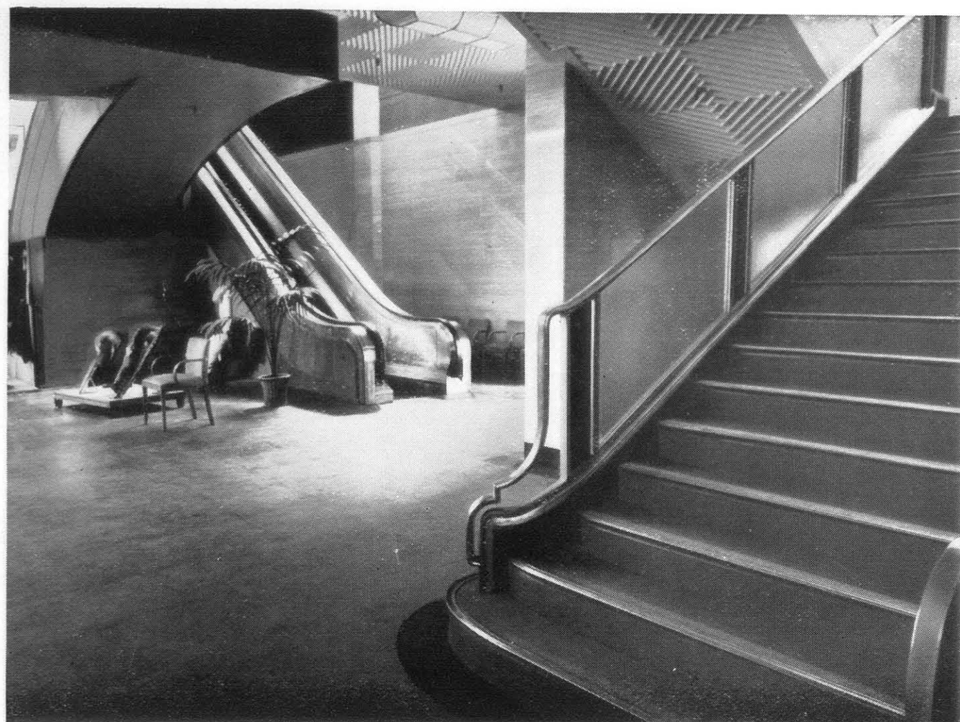
S.G. 332. Glazed Balustrade in cellulosed steel with bronze handrail (Section 2, No. 26) sweeping down to form decorative newel. The concrete curb, also treads and risers, are faced with cork that is fitted flush to bronze edgings and nosings
