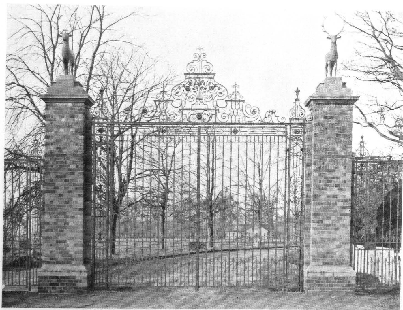
S.G. 835. Private Park Carriage Gates and Railings forged in wrought iron. Single transome rail supporting overthrow built up with channel section on wide shadow rail and forged bent to counteract deflection at centre of span. Stags cast in lead with antlers reinforced in steel
