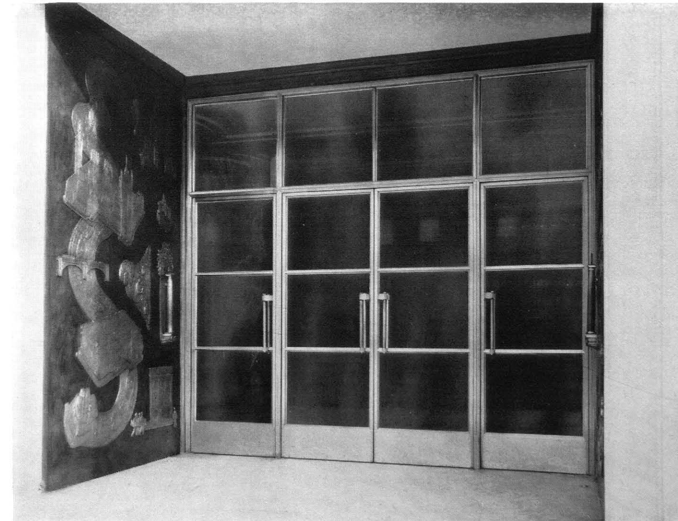
Double Swing Doors to Foyer in extruded and machined silver-bronze. The hanging styles and heels of these exceptionally wide doors are reinforced in steel and braced between kicking plates
