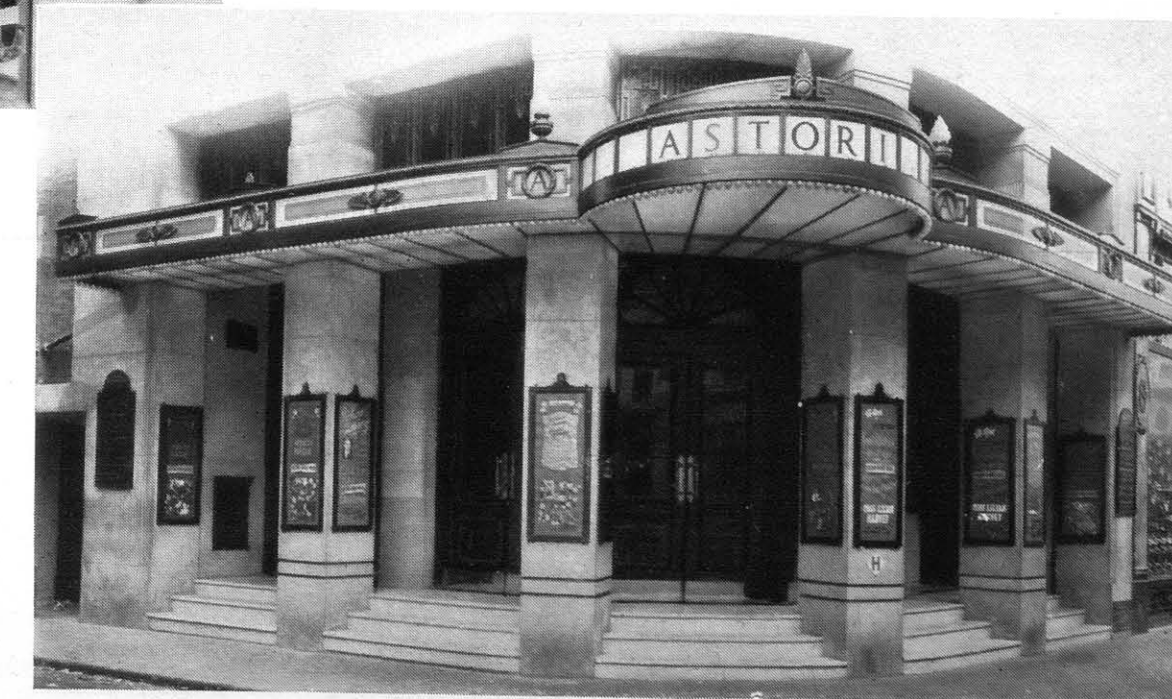
S.G. 910. Horse-shoe shaped Canopy constructed with boxed R.S. channel cantilevers. The lettered fascia is glazed with bent opal glass; the inner curved fascia with obscured amber glass. The border soffite is fitted with continuous bulb lighting and the roof glazed with rough cast Georgian glass
