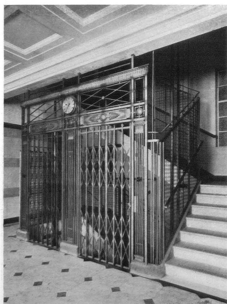
S.G. 211. Double Enclosure in wrought and fine cast iron, and fitted with top-hung steel collapsible gates
