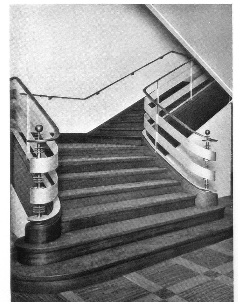
S.G. 323. Balustrading in wrought iron with 4 \text{ in.} \times \frac{3}{8} \text{ in.} flat steel intermediate rails passing through upright standards. The circular newels are in bronze with rails winding round centre shaft. Bronze handrail (Section 2, No. 21)
