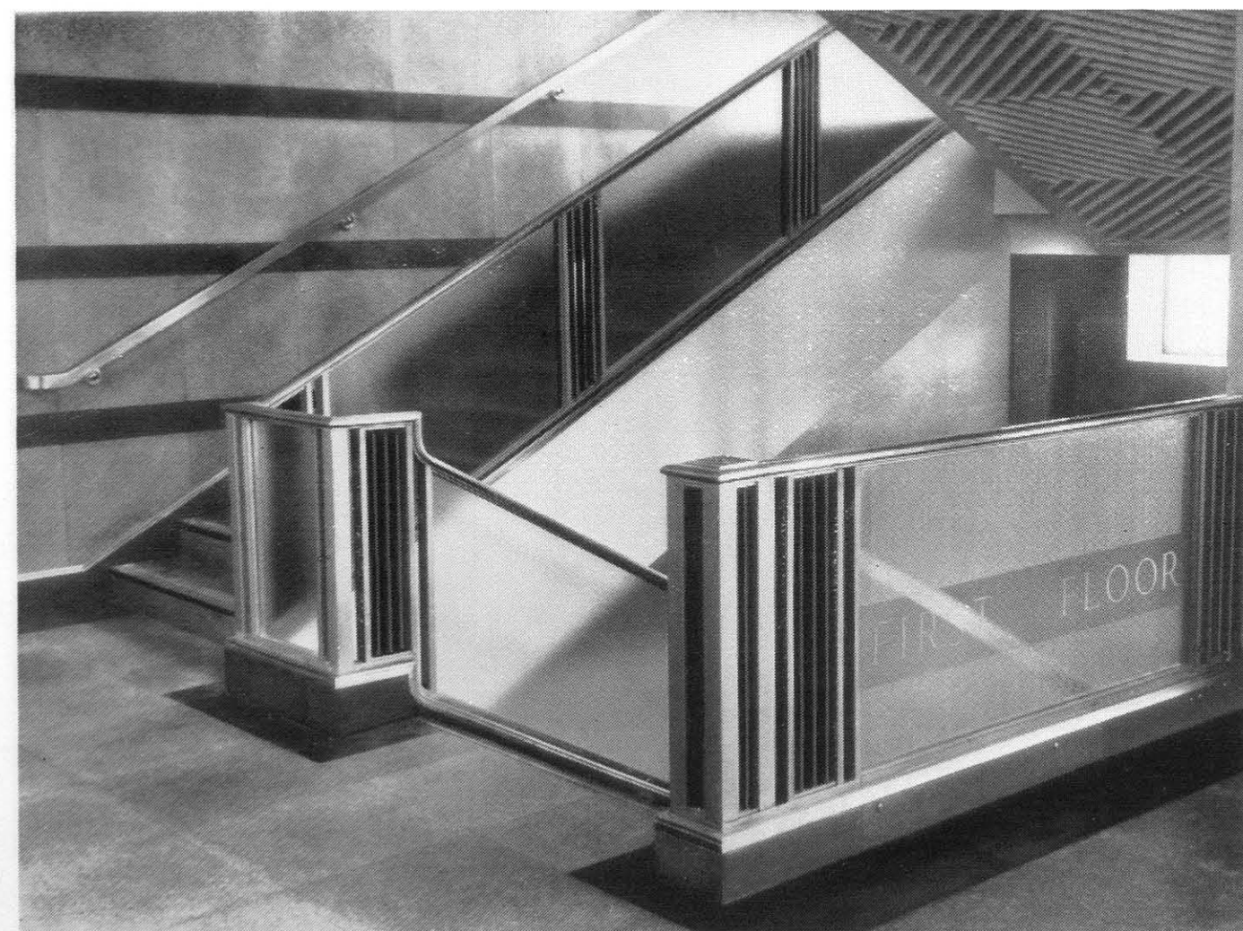
S.G. 333. Balustrade showing lettered Landing Panel illuminated through lower edge of sandblasted rough cast glass by strip lights fitted immediately behind access plate in curb. The walls and floors are adhered in two shades of cork and the string is edged with bronze to match finish under balustrade
