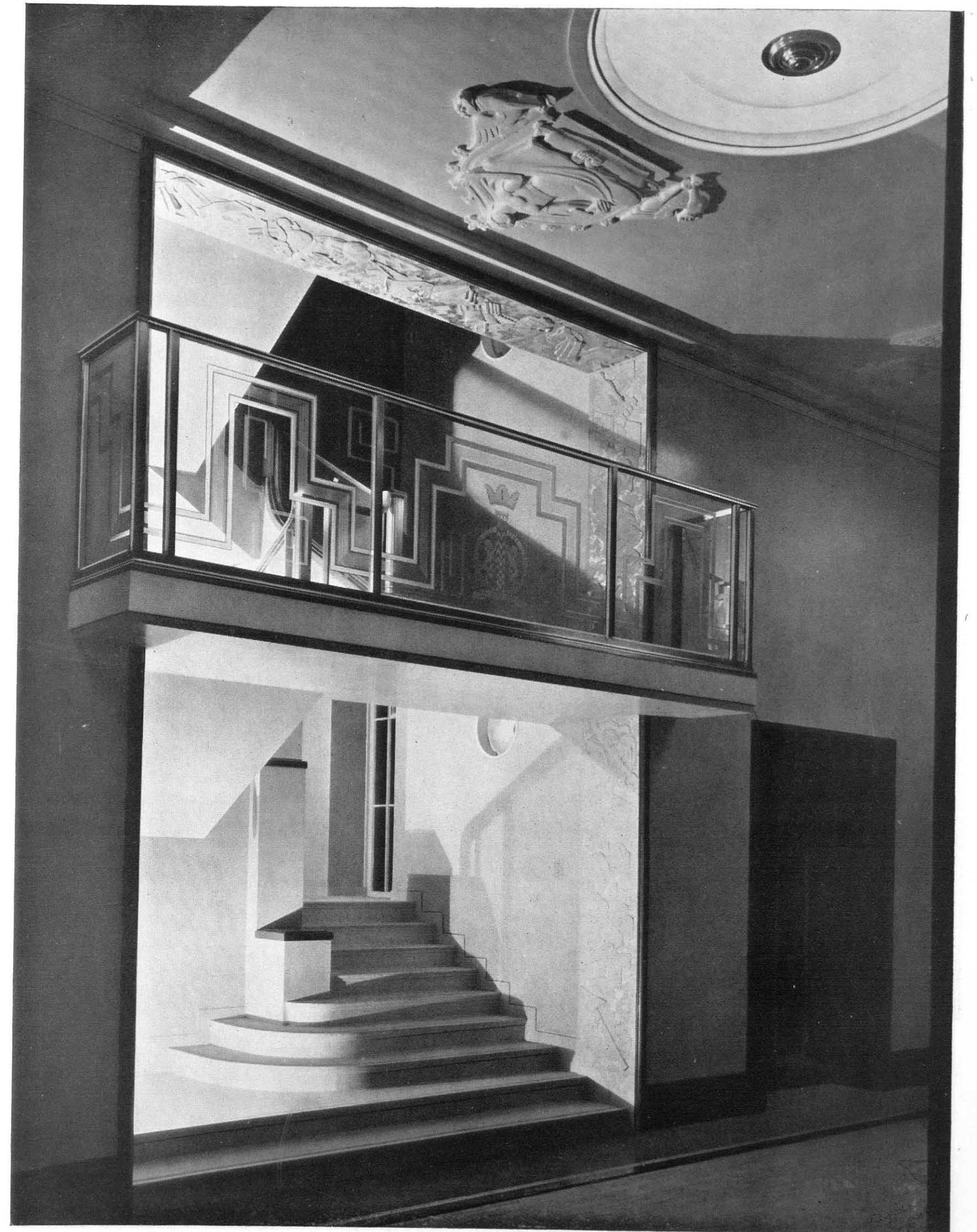
Overhanging Balcony Balustrading in light sectioned silver-bronze with copper-bronze handrail capping. The intermediate uprights are reinforced in steel for rigidity over long span
