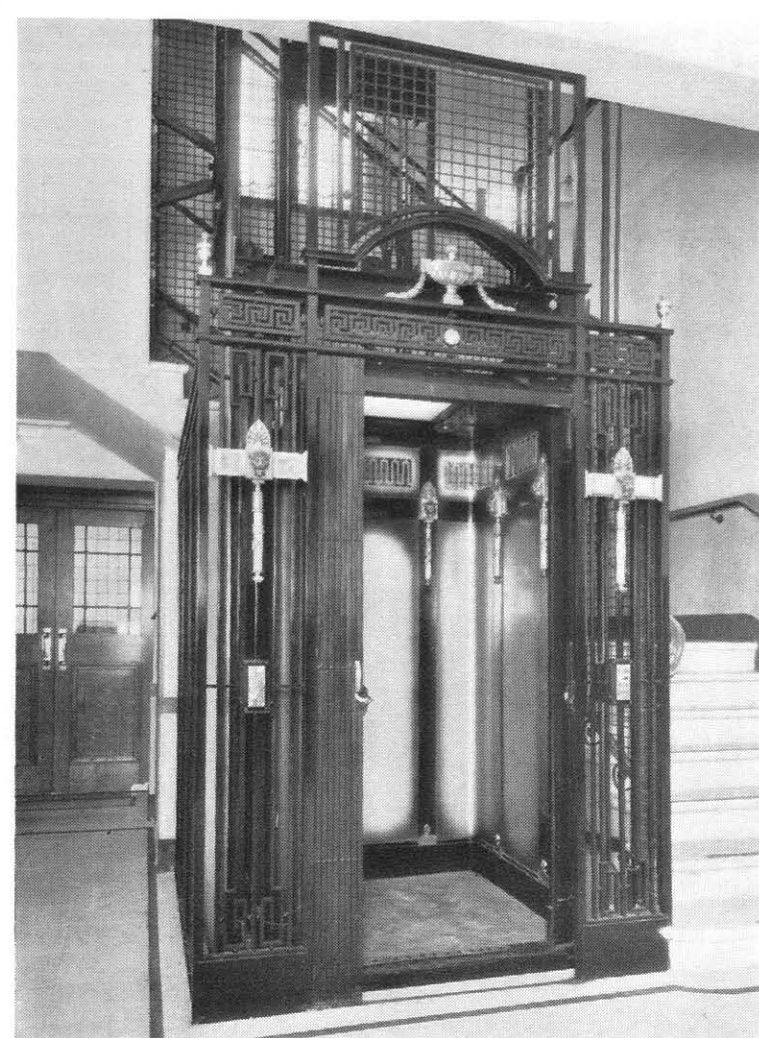
S.G. 210. In wrought iron with fine cast iron enrichments. The Lift Car is built up with planished steel plates on skeleton flat steel strap-ping. Cellulosed decorated to high gloss finish
