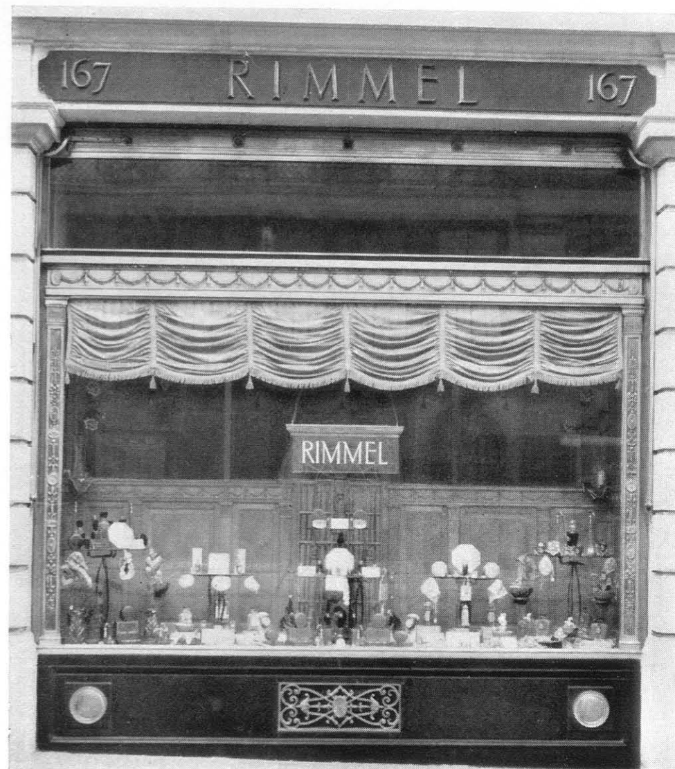
S.G. 5007. Shopfront executed in fine cast and extruded silver bronze mounted on black marble stall-riser, with the carved wood interior window-screens in silver sycamore
