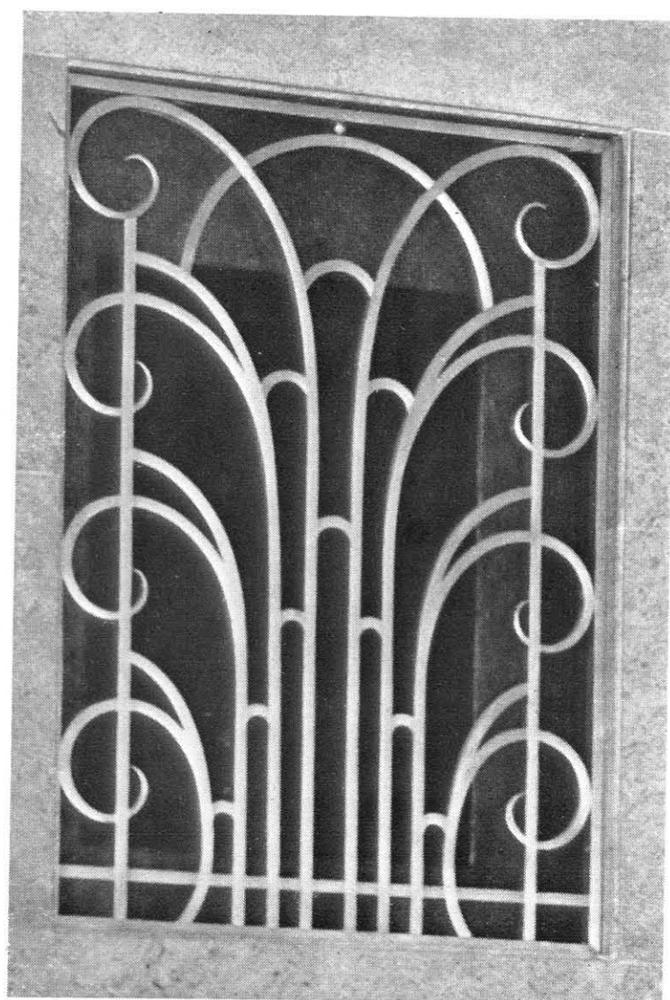
S.G. 605. Grille in forged and machine-halved silver-bronze; backed with bronze mesh
