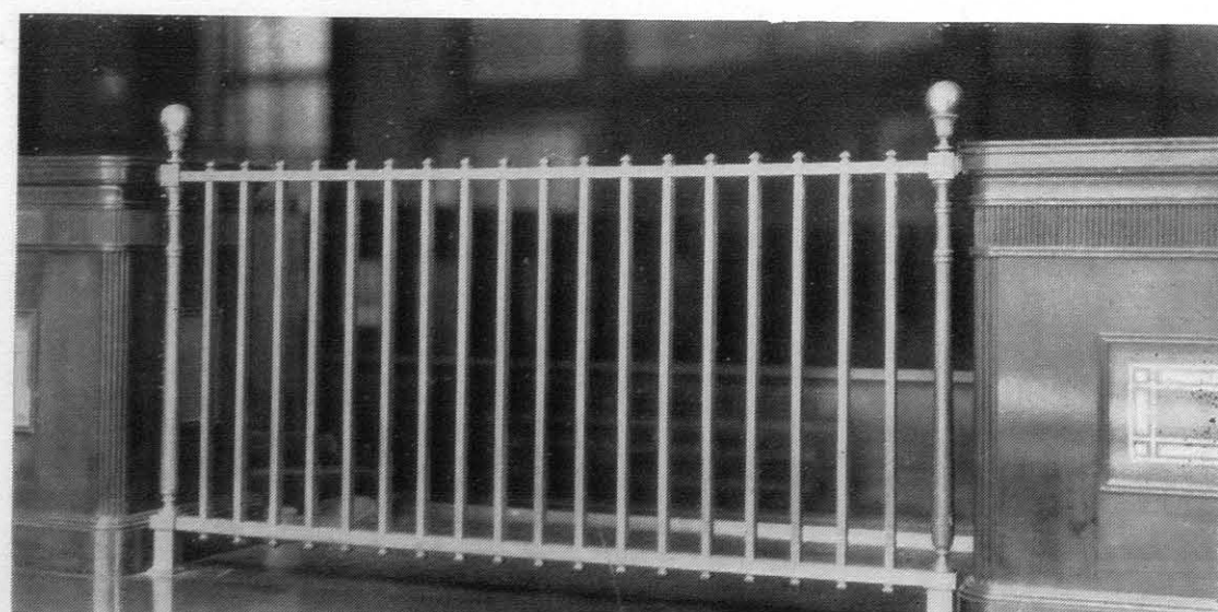
S.G. 606. Counter Grille in extruded bronze, with fine cast vase terminals and turned bronze spindles
