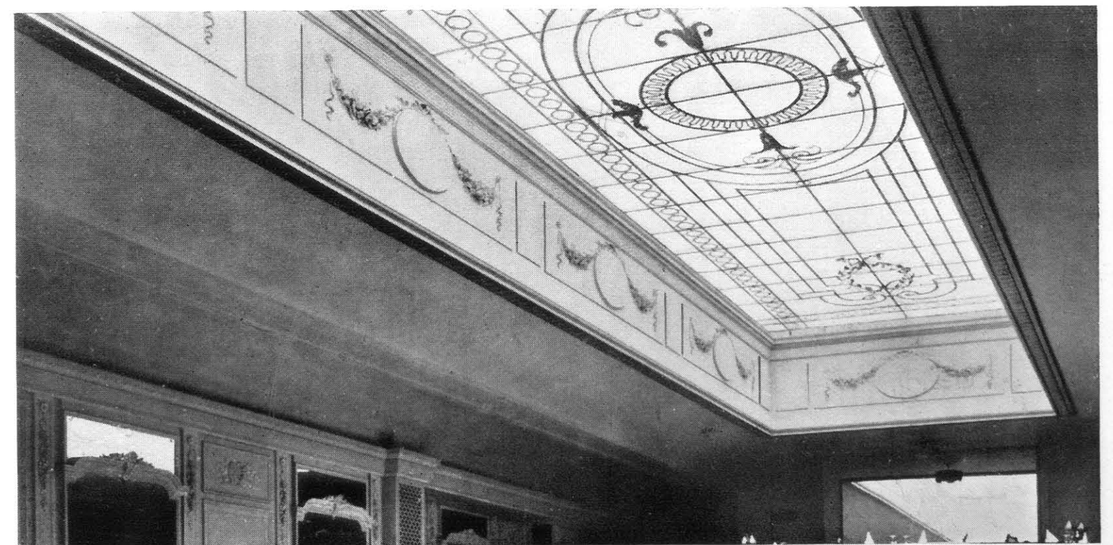
S.G. 1025. Laylight constructed in wrought steel with applied forged and hammered iron enrichments. Glazed with rough cast sand-blasted glass and flood lighted
