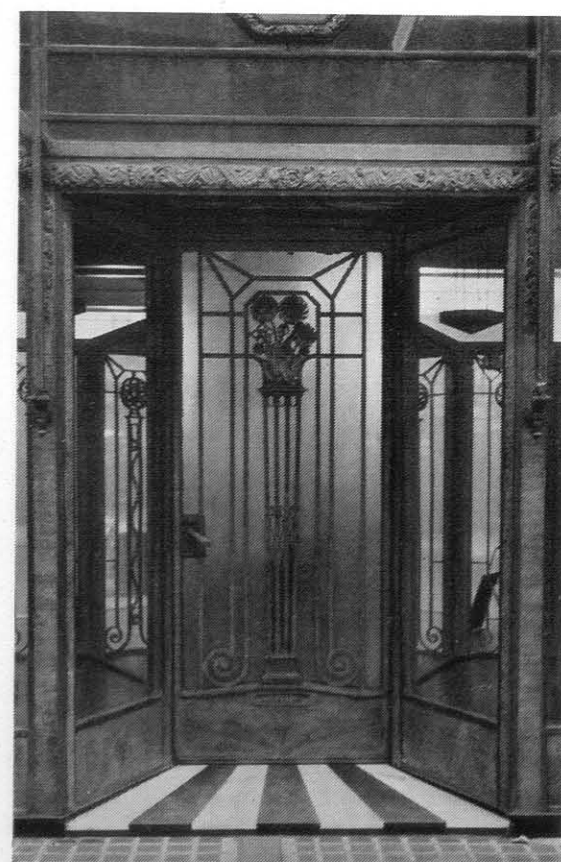
S.G. 5009. Shop Entrance Doorway in wrought and hammered steel with foliage patterned enrichments in fine cast iron. Cellulosed vert-antique
