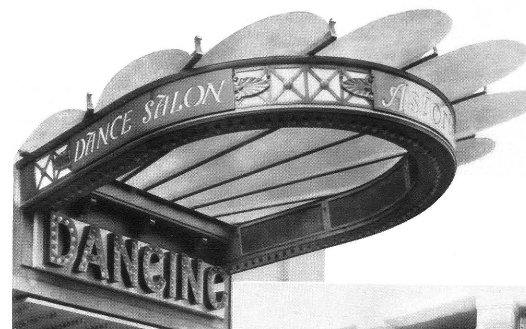
S.G. 908. Canopy executed in extruded bronze with glazed apron, soffite and roof. The soffite is fitted with hinged access panels
