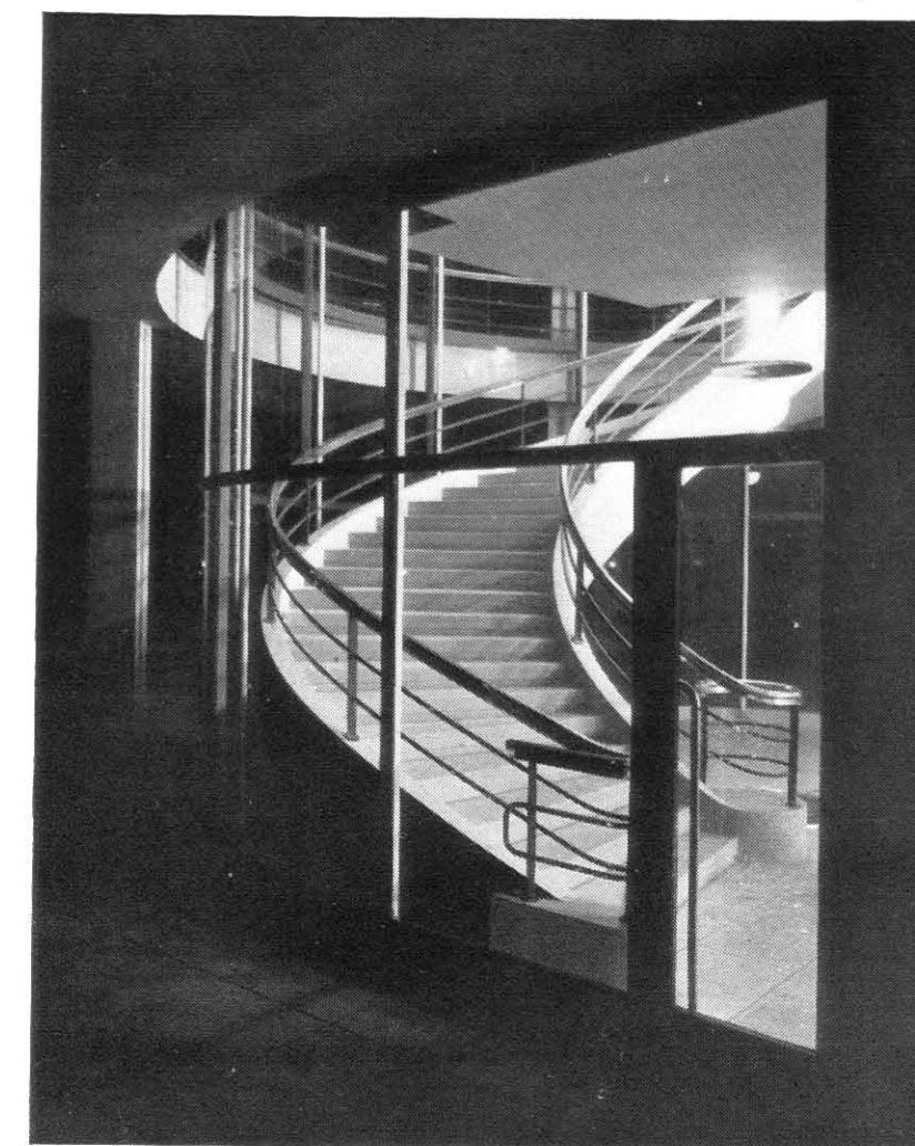
S.G. 328. Balustrade to Winding Staircase terminating with swept newels on either side
