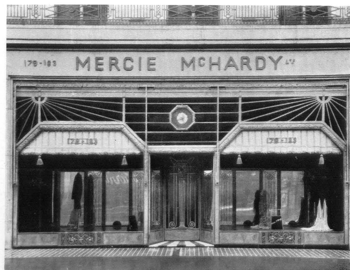
S.G. 5010. Shopfront and Mirrored Window-screens in wrought steel enriched with fine cast iron foliage and hammered-patterned ornament. The blind lath is in reinforced aluminium
