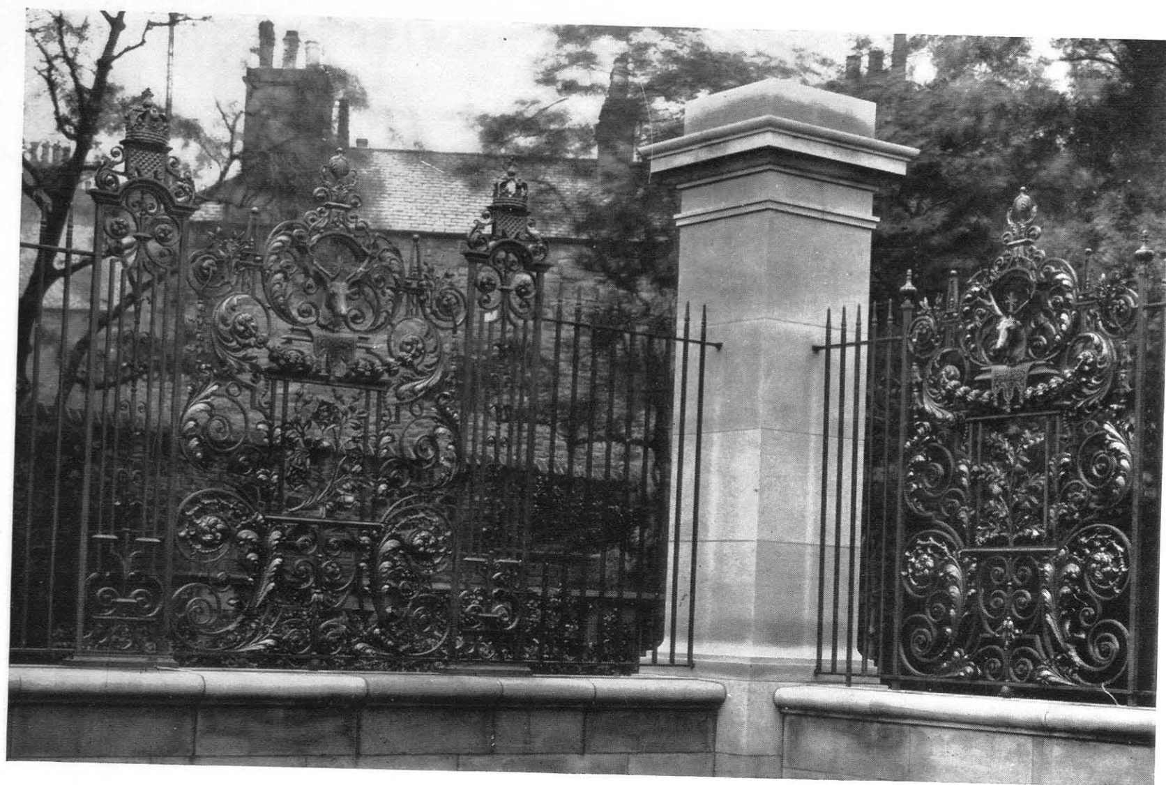
S.G. 834. Palace Screens executed in wrought iron with hammered steel leafwork, rosettes, husks, aprons and foliage; crowns, vases and stagheads in modelled and fine cast bronze; enrichments double-sided throughout
