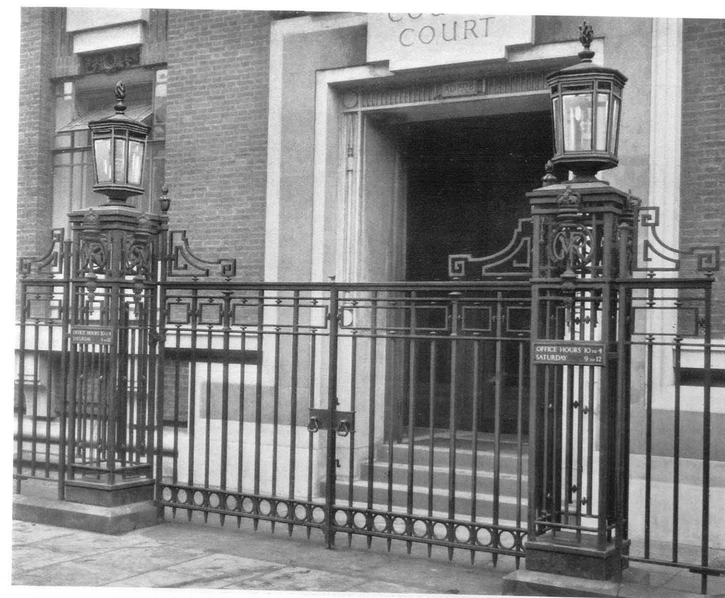
S.G. 829. County Court Gates and Railings executed in wrought iron with bronze lamps; Royal Crests in cast and sanded bronze with lettering forged and interlaced. Gates hung on gunmetal bushed journals, fitted to the inner back styles of square pilasters
