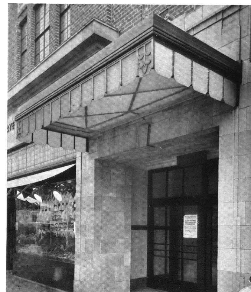
S.G. 908. Canopy executed in extruded bronze with glazed apron, soffite and roof. The soffite is fitted with hinged access panels
