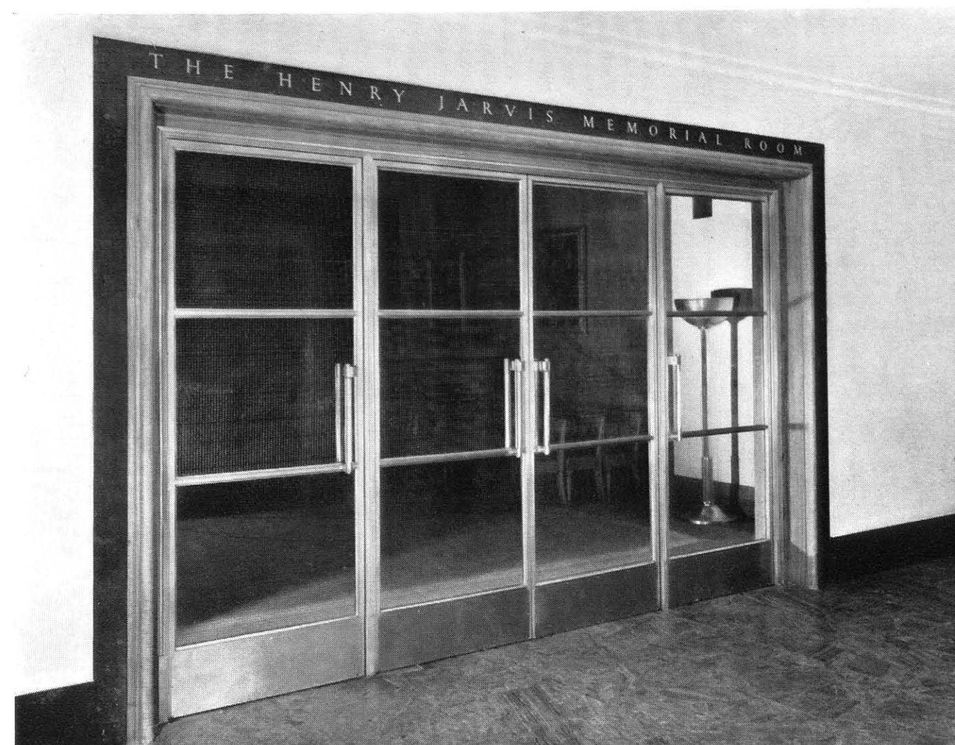
Double Swing Doors to Foyer in extruded and machined silver-bronze. The hanging styles and heels of these exceptionally wide doors are reinforced in steel and braced between kicking plates
