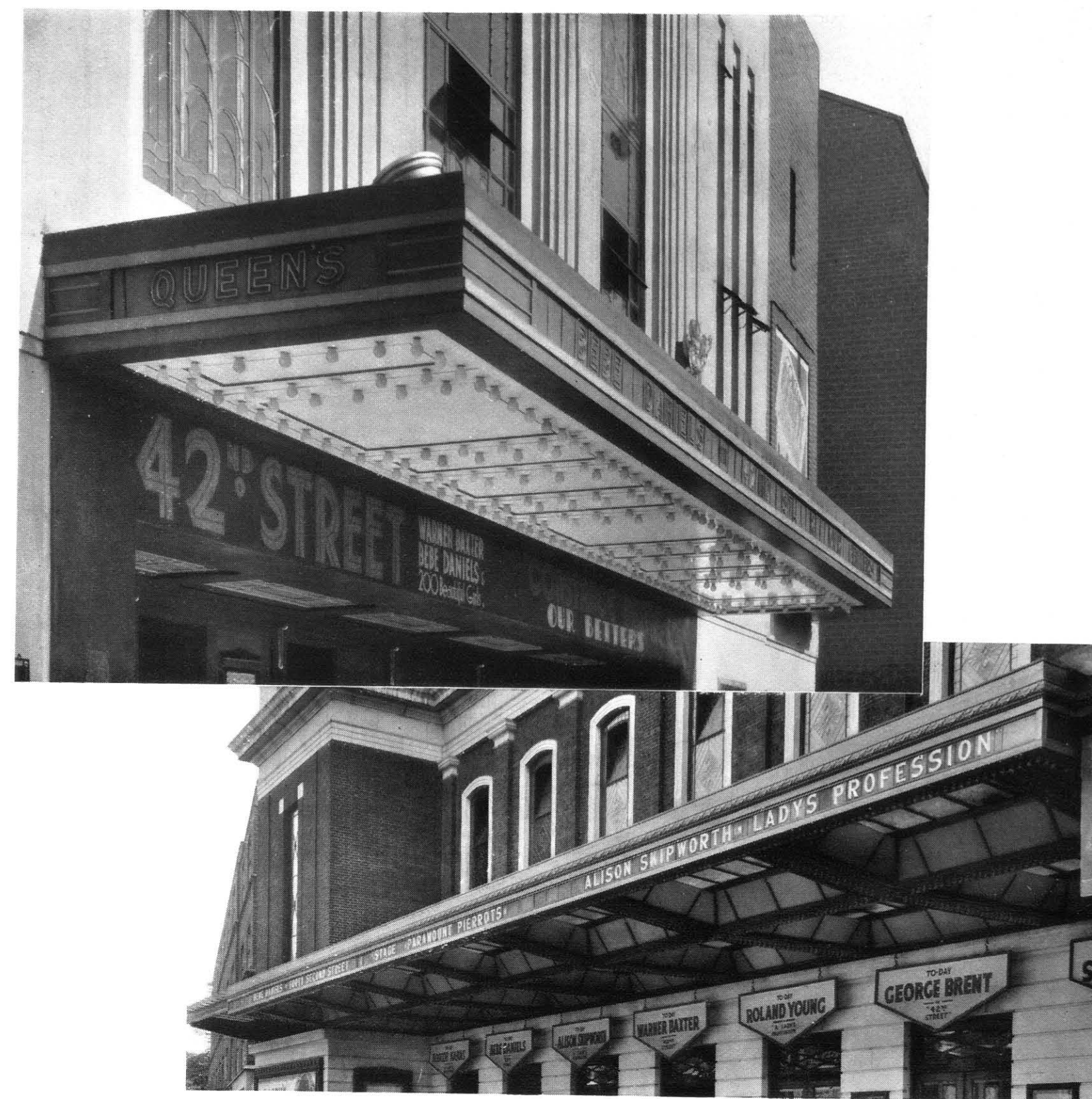
S.G. 921. Canopy in wrought iron with built-up sheet steel soffite. The fascia is fitted with interchangeable lettering illuminated from behind. The borders to soffite panelling are outlined with bulb lighting. Exposed metalwork is cellulosed to three-colour scheme
