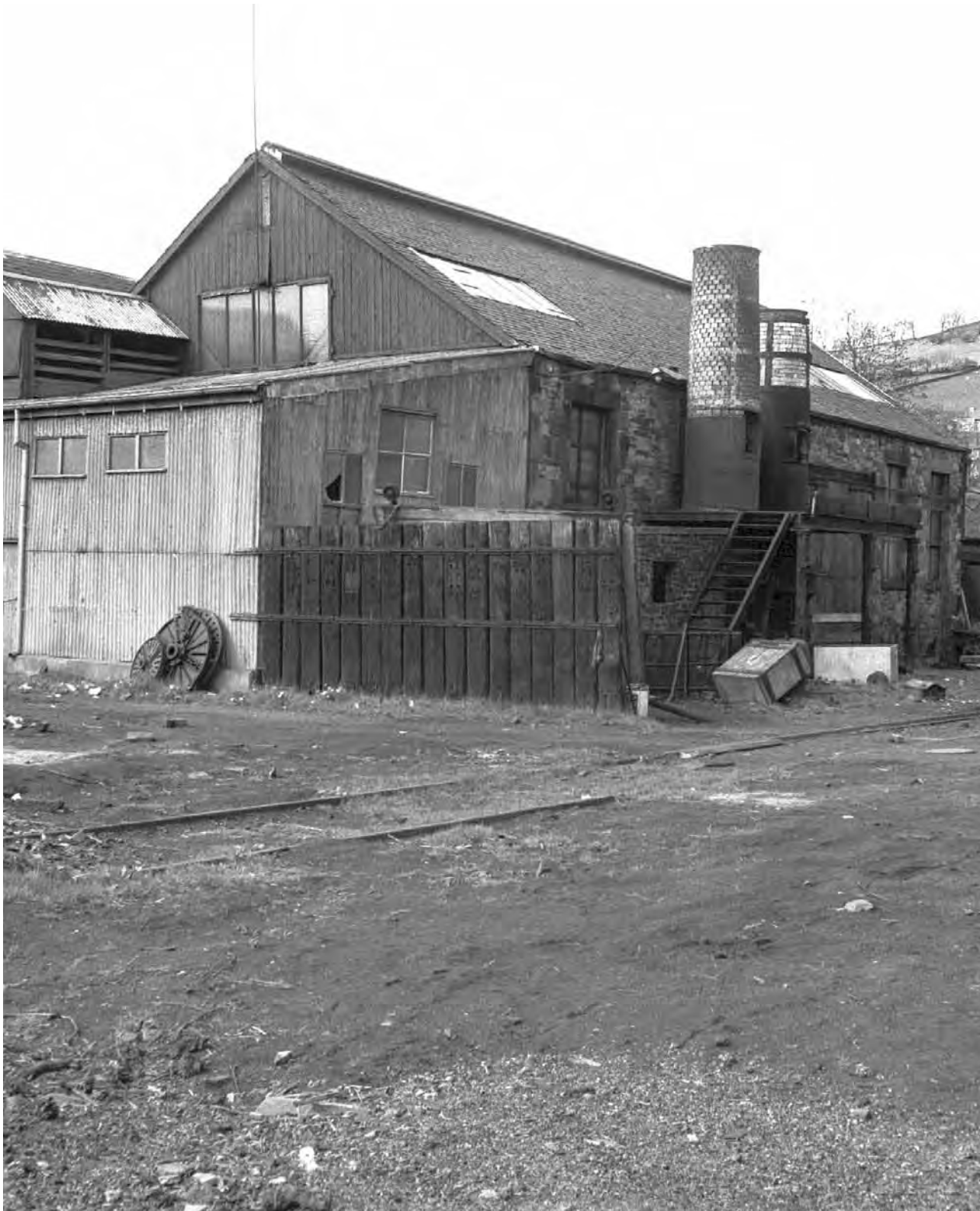
Fig. 8 View of Waverley Iron Works, Huddersfield Street, Galashiels Image courtesy of The Royal Commission on the Ancient and Historic Monuments of Scotland
