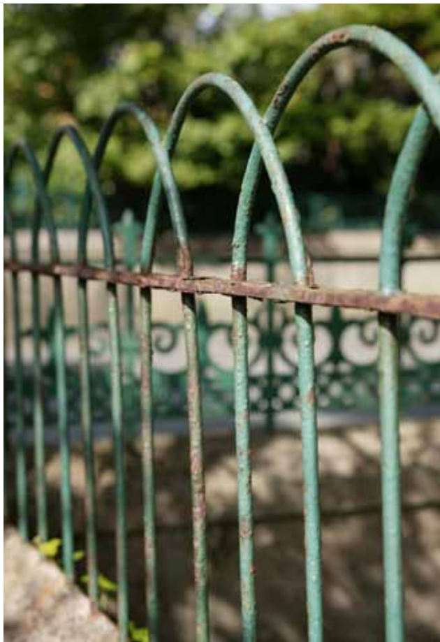
Figs. 414 - 416 Severe corrosion occurring to wrought iron gates and railings around the town
