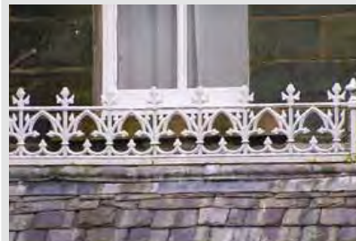
Fig. 329, Taybridge Road, Aberlady, Made by Walter MacFarlane & Co, pattern number 40 Image courtesy of The Scottish Ironwork Foundation
