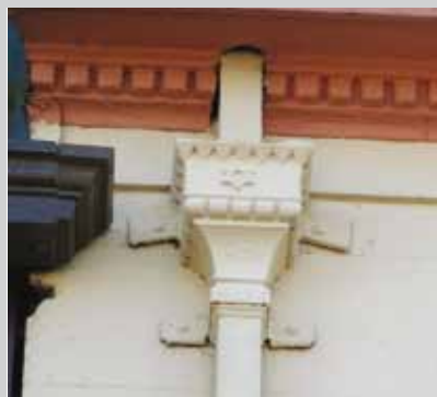
Fig. 214, Hopper 6 Made by Walter MacFarlane & Co, pattern 35
