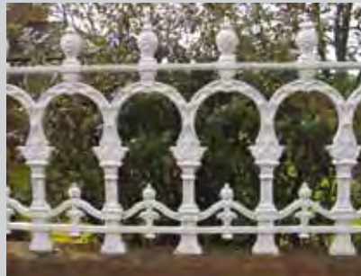
Fig. 290, Railing 16 , Stornoway Unmarked but probably made by Walter MacFarlane & Co, pattern number 1125
