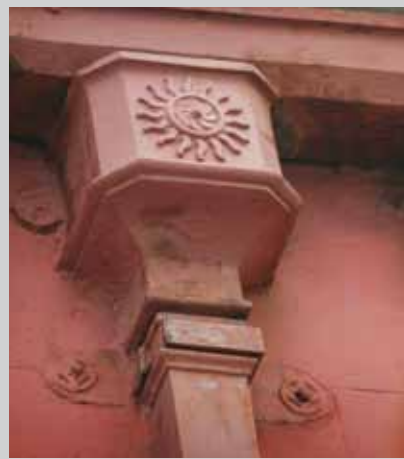
Fig. 239, Hopper 17 Made by Walter MacFarlane & Co, pattern number 92
