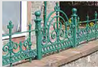
Figs. 280 & 281, Tongland Road, Kirkcudbright Made by Walter MacFarlane & Co, pattern number 145 This example includes a two- leafed gate and an unusual railing panel detail with newel posts. Image courtesy of The Scottish Ironwork Foundation
