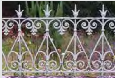
Figs. 306 & 307, Proby Street, Maryburgh, Highland, Made by Walter MacFarlane & Co, pattern number 213 Image courtesy of The Scottish Ironwork Foundation
