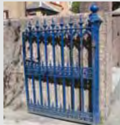
Gate 25a Walter MacFarlane & Co., pattern number unidentified but matching Railing 25, pattern number 830
