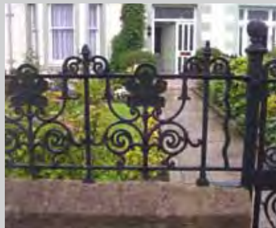
Fig. 292, Railing 8 , Stornoway Made by Walter MacFarlane & Co (as marked on the matching gate), pattern number unidentified
