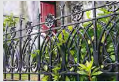
Fig. 273, Vinicombe Street, Glasgow Made by Walter MacFarlane & Co The finials between the flower detail are very different from the variations made by Lion Foundry, Alpine Ironworks and Mitchell & Carlaw Image courtesy of The Scottish Ironwork Foundation
