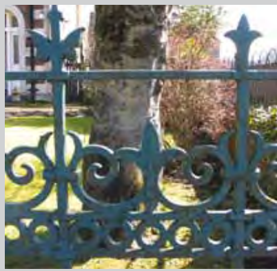
Fig. 186, Railing 12 Unmarked, but probably made by Lion Foundry, pattern number 247
