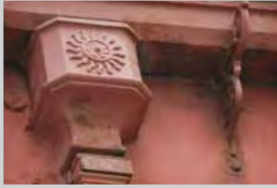
Fig. 353, Hopper number 17 , Stornoway Made by Walter MacFarlane & Co, pattern number 92
