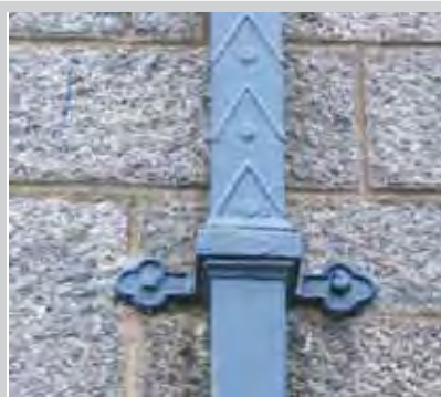
Fig. 217, Downpipe no. 2, Made by Walter MacFarlane & Co., pattern number 17
