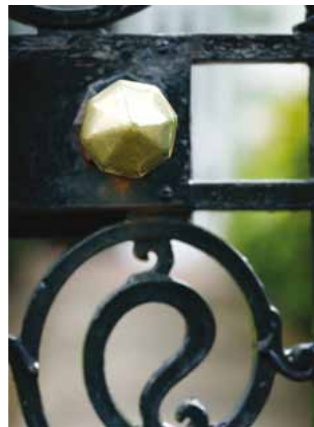
Fig. 174 Detail of the brass handle on Gate 8 (made by Walter MacFarlane & Co), Matheson Road, pattern number 830
