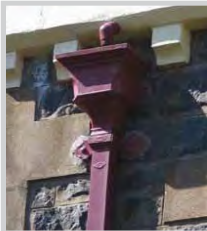
Fig. 232, Hopper 13 Made by Walter MacFarlane & Co, pattern number 44
