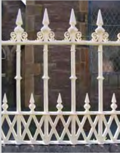
Fig. 301, Railing 23 , Stornoway Made by George Smith & Co, pattern number 949
