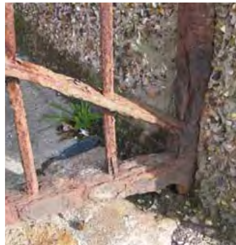
Figs. 414 - 416 Severe corrosion occurring to wrought iron gates and railings around the town
