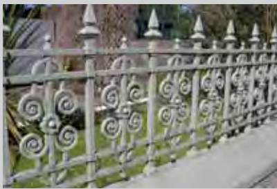
Fig. 283, Railing 10 , Stornoway Made by Walter MacFarlane & Co, pattern number 1031
