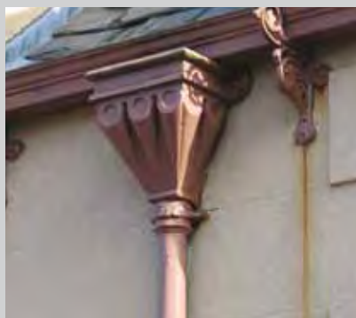
Fig. 229, Hopper 11 Manufacturer unidentified, but probably either Walter MacFarlane & Co. or George Smith & Co.
