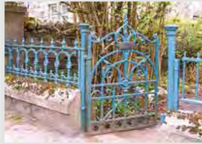
Fig. 334, Taybridge Road, Aberfeldy Made by Walter MacFarlane & Co, pattern number 946 (with adjoining railings R16 also by Walter MacFarlane & Co, pattern number 1125) Image courtesy of The Scottish Ironwork Foundation
