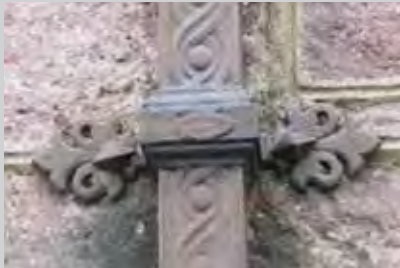
Fig. 362, Downpipe 1 , Stornoway Made by Walter MacFarlane & Co, pattern number 18
