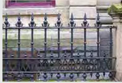
Fig. 301, Railing 23 , Stornoway Made by George Smith & Co, pattern number 949
