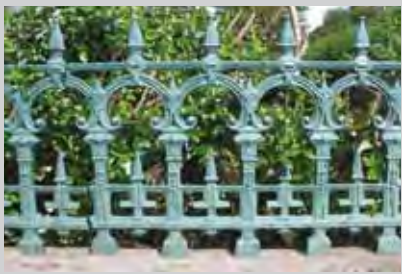
Fig. 159, Railing 6 Unmarked, but probably made by Walter MacFarlane & Co, pattern number 1126
