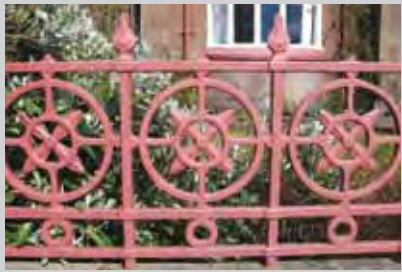
Fig. 201, Railing 21 Made by Carron, pattern number 111
