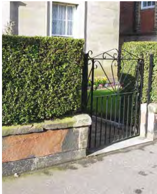
Fig. 34 Mild steel railings and hedges have now replaced many of the railings that were removed
