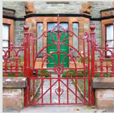
Fig. 336, St Mary Street, Kircudbright Made by Walter MacFarlane & Co, pattern number 946. This variation does not have the additional detailing along the base Image courtesy of The Scottish Ironwork Foundation
