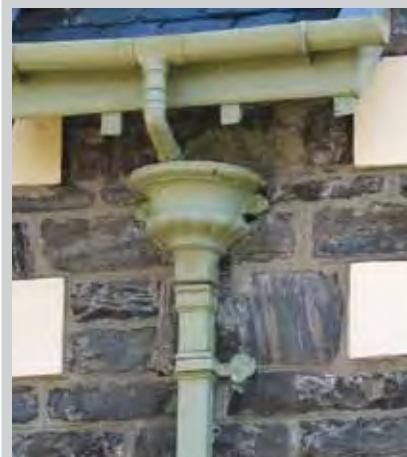
Fig. 236, Hopper 14 Made by Walter MacFarlane & Co, pattern number 12
