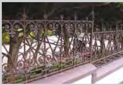
Fig. 308, Railing 1a , Stornoway) Unmarked but probably made by Walter MacFarlane & Co, pattern number 213
