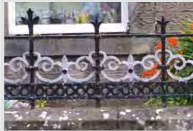
Figs. 275 & 276, High Street, Aberlour, Moray. Made by Walter MacFarlane & Co, pattern number 145 Walter MacFarlane & Co Ltd produced a variation of this design which is almost identical but can be distinguished by the circle detail on the leaf – the MacFarlane version has only one circle, whereas the Stornoway version has four in a vertical line which increase in diameter from top to bottom. The finial detail is also slightly different. Image courtesy of The Scottish Ironwork Foundation
