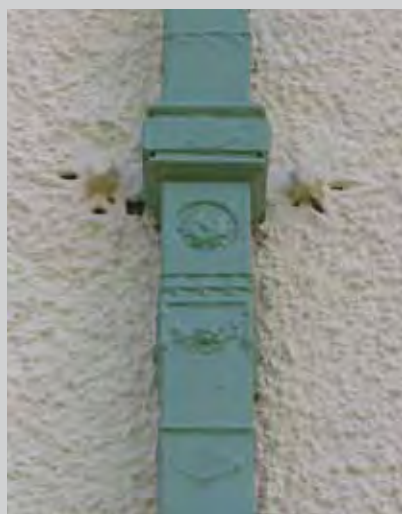
Fig. 219, Downpipe 3 Made by Walter MacFarlane & Co, pattern 24
