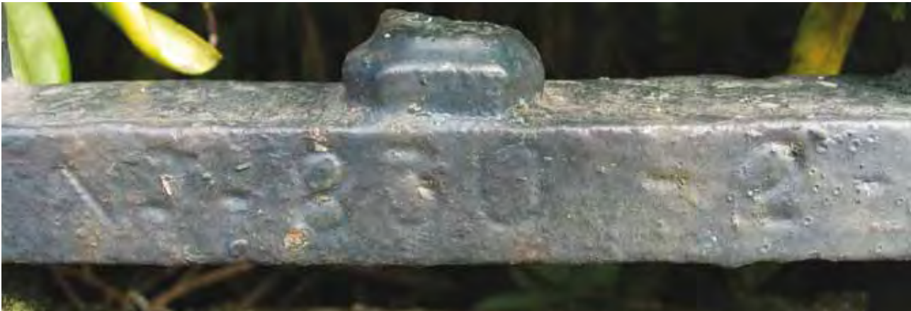
Fig. 98 Railing 25, showing the pattern number of the casting
