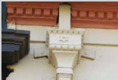
Fig. 357, Hopper number 6 , Stornoway Made by Walter MacFarlane & Co pattern number 35
