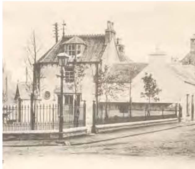
Fig. 52 Post Office, Cromwell Street Image courtesy of Western Isles Libraries
