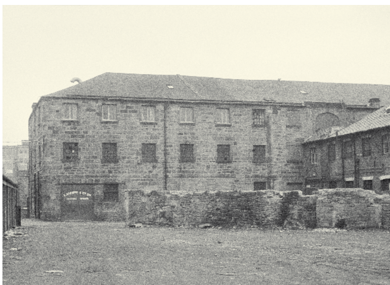
Fig. 12 View of Milton Iron Works, No 142 North Woodside Road, Glasgow Image courtesy of The Royal Commission on the Ancient and Historic Monuments of Scotland
