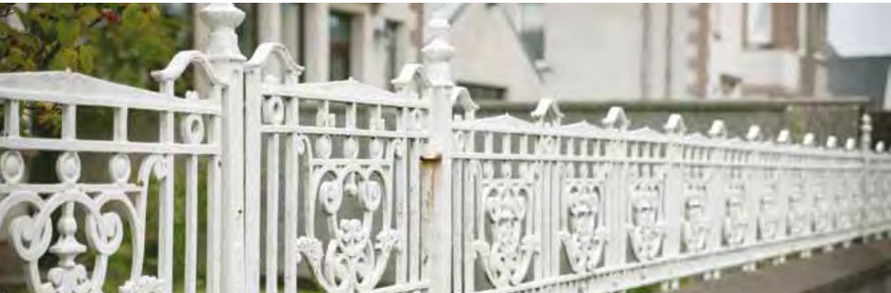
Fig. 101 Railing 30 and Gate no. 30 made by Aimers McLean Ltd
