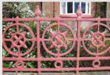
Railing 21 Height: 540mm (21¼ inches) Carron Iron Foundry Works pattern number 111
