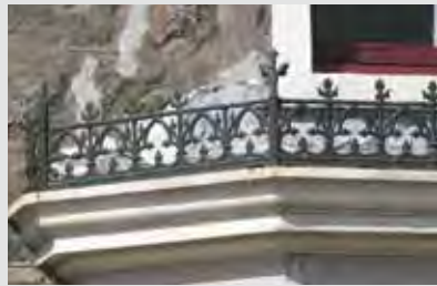
Cresting 2 Maker unidentified. Variations of this design were made by all the major Scottish foundries
