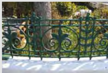
Railing 50 Height: 596mm (23½ inches) McDowall Steven & Co. pattern number 2107
