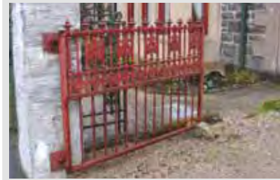
Gate 27a Falkirk Iron Company
