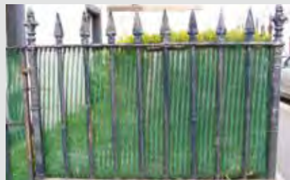
Railing 48 Manufacturer unidentified but possibly Carron Foundry Company pattern number 100 or George Smith & Co. pattern number 1485
