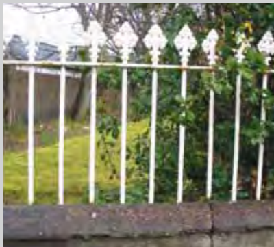
Fig. 296, Railing 3 , Stornoway Unmarked but possibly made by George Smith & Co, pattern number 783 (although catalogue illustration has a fluted bar)
