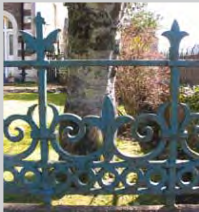
Fig. 153, Railing 12 Unmarked but probably Lion Foundry, pattern number 247
