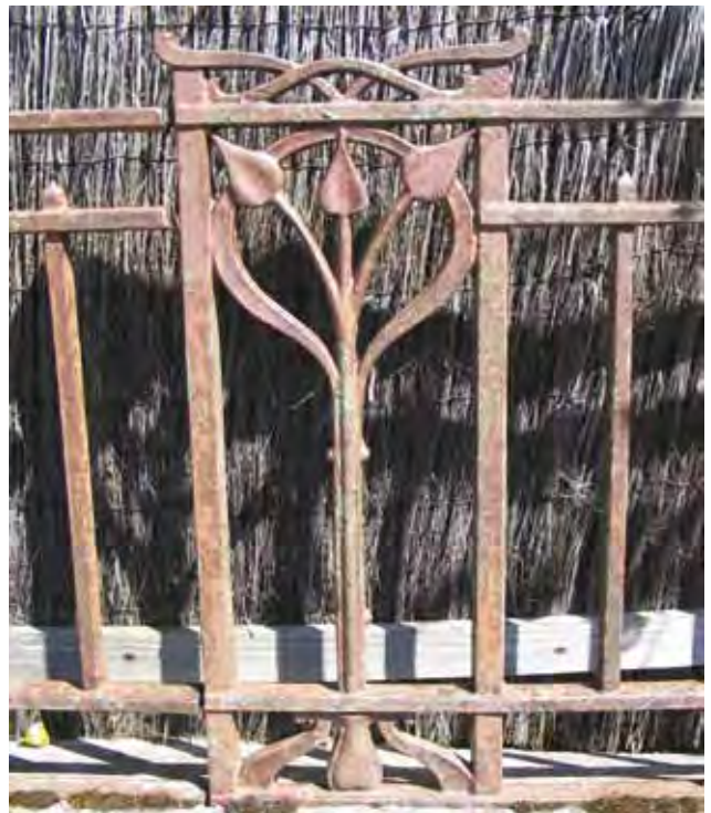
Fig. 122 Railing 31, maker unidentified
