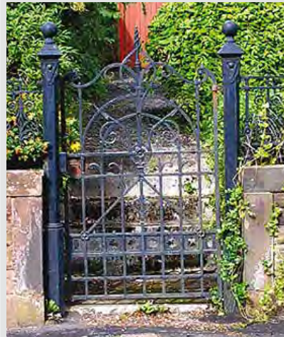
Fig. 335, Glasgow Road, Sanquhar Made by Walter MacFarlane & Co, pattern number 946 This variation has an extra section added to the base of the gate Image courtesy of The Scottish Ironwork Foundation
