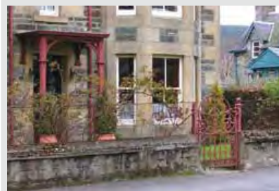
Fig. 341, Kenmore Road, Aberfeldy Made by Walter MacFarlane & Co, pattern number 189 Image courtesy of The Scottish Ironwork Foundation
