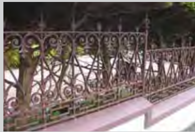
Fig. 125, Railing 1a Made by Walter MacFarlane & Co, pattern number 213
