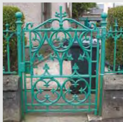
Fig. 177, Railing 25 Made by Walter MacFarlane & Co, pattern number 830
