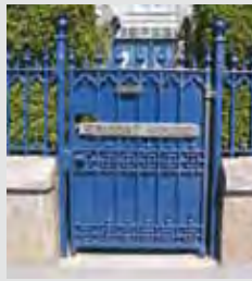
Gate 25 Walter MacFarlane & Co., pattern number unidentified but matching Railing 25, pattern number 830
