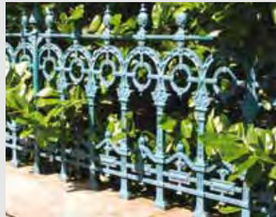
Fig. 291, Ernspie Road, Castle Douglas Made by Walter MacFarlane & Co, pattern number 1125 This example is a slight variation of the Stornoway version Image courtesy of The Scottish Ironwork Foundation
