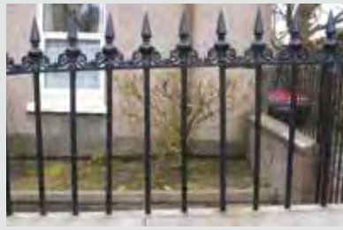
Railing 5 Height: 850mm (33½ inches) Manufacturer unidentified but possibly George Smith & Co.
