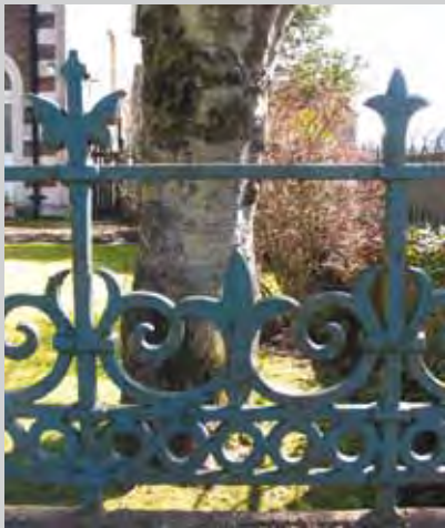
Fig. 274, Railing 12 , Matheson Road, Stornoway, Unmarked but believed to be Lion Foundry pattern 247
