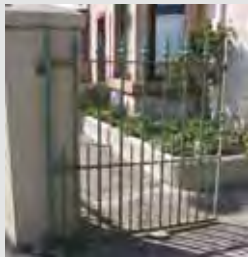
Gate 2 Matching Railing 2, George Smith & Co pattern number 789 or Carron Iron Works pattern number 119
