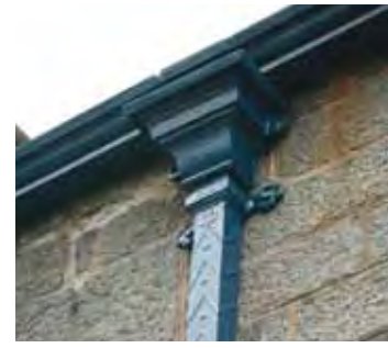
Fig. 385 Downpipe 2 and hopper 7
