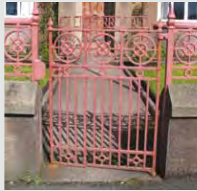
Fig. 202, Gate 21 Made by Carron Foundry Works, pattern number 111
