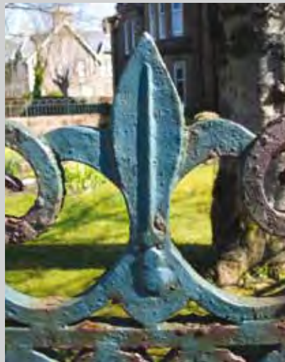
Fig. 154, The Lion Foundry version is recognisable by the row of dots increasing in size from top to bottom on the leaf detail
