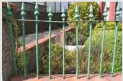
Railing 2 Height: 647mm (25½ inches) George Smith & Co pattern number 789 or Carron Iron Works pattern number 119
