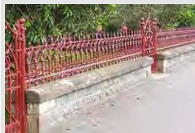
Fig. 288, St Mary Street, Kirkcudbright Unmarked but probably made by Walter MacFarlane & Co, pattern number 1126 Image courtesy of The Scottish Ironwork Foundation
