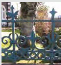
Railing 12 Height: 635mm (25 inches) Lion Foundry Company pattern number 247
