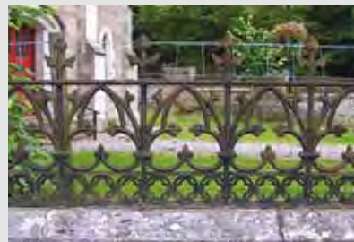
Fig. 320, Cresting number 2 , Stornoway Maker unidentified, but possibly made by: Carron, pattern number 57 or Alloa Iron company, pattern number 1233 or Bo'Ness Foundry, pattern number 500 or Walter MacFarlane & Co, pattern number 40 or George Smith & Co, pattern number 1185 or Lion Foundry, pattern number 286
