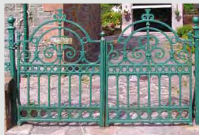
Figs. 280 & 281, Tongland Road, Kirkcudbright Made by Walter MacFarlane & Co, pattern number 145 This example includes a two- leafed gate and an unusual railing panel detail with newel posts. Image courtesy of The Scottish Ironwork Foundation
