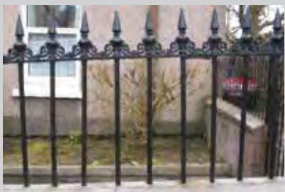
Fig. 130, Railing 5 Unmarked but possibly made by George Smith & Co
