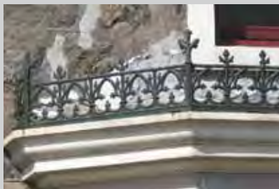
Fig. 320, Cresting number 2 , Stornoway Maker unidentified, but possibly made by: Carron, pattern number 57 or Alloa Iron company, pattern number 1233 or Bo'Ness Foundry, pattern number 500 or Walter MacFarlane & Co, pattern number 40 or George Smith & Co, pattern number 1185 or Lion Foundry, pattern number 286
