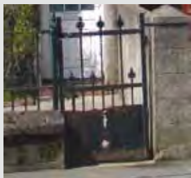
Gate 4 Manufacturer unidentified
