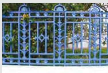
Railing 22 Height: 762mm (30 inches) Lion Foundry Company, pattern number 461
