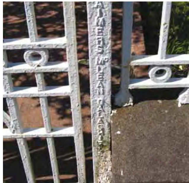
Fig. 100 Railing 30 and Gate 30, made by Aimers McLean, Galashiels
