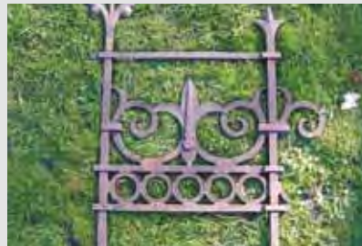
Fig. 154, The Lion Foundry version is recognisable by the row of dots increasing in size from top to bottom on the leaf detail
