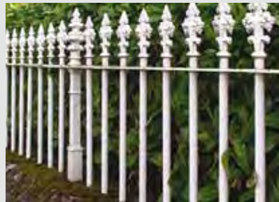
Fig. 296, Railing 3 , Stornoway Unmarked but possibly made by George Smith & Co, pattern number 783 (although catalogue illustration has a fluted bar)
