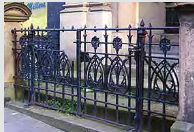
Fig. 272, St John's Church, Dunoon Made by Alpine Ironworks This variation has slightly different finials between the flower details Image courtesy of The Scottish Ironwork Foundation
