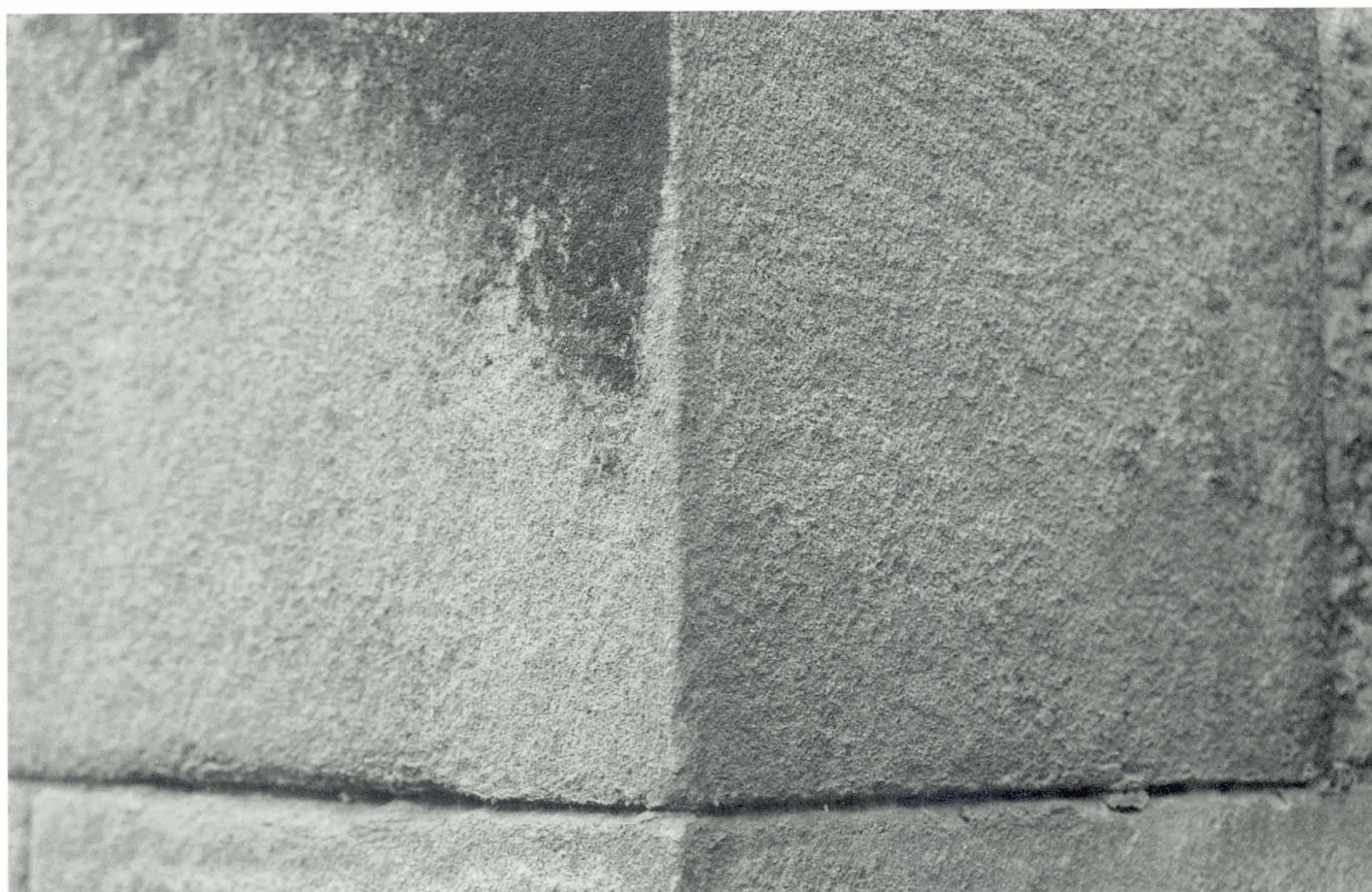
Plate 4.18 Sandstone partially cleaned using low pressure grit blasting. Right side of corner cleaned, left side uncleaned. The left side shows soiling at the top and a naturally unsoiled area to lower left. The cleaned area to the right was originally black with soiling. Its appearance now resembles the natural weathered patina. Tool marks are retained.
