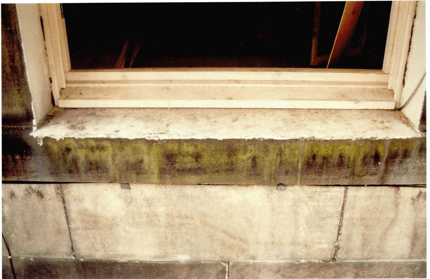
Plate 4.25 Before wet grit blast cleaning. Algal growth below window ledge.
