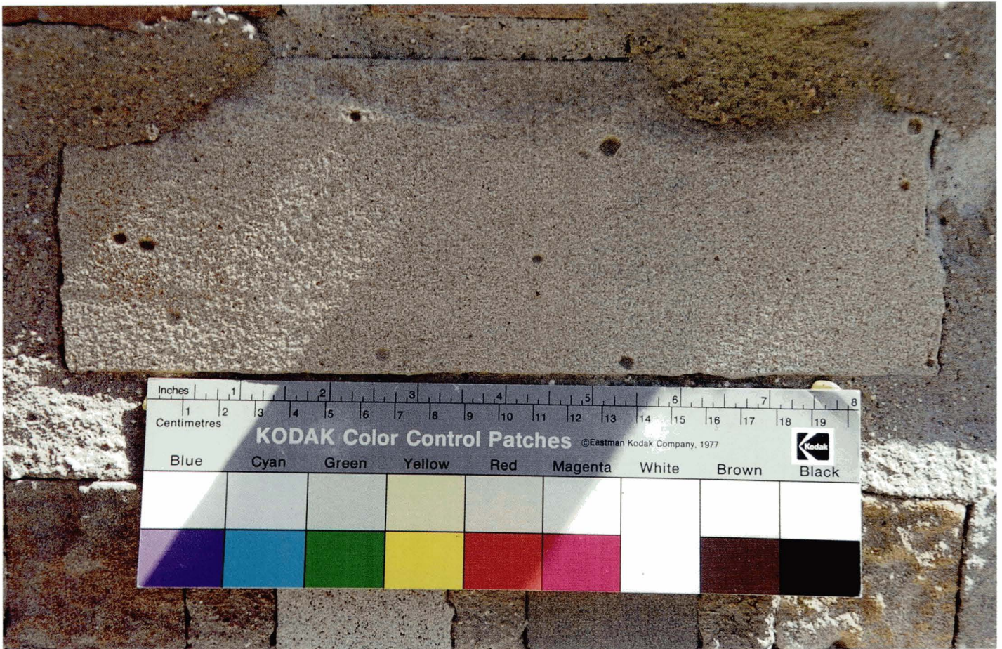
Plate 4.5 Pitting of sandstone following dry grit blasting, due to erosion of calcite cemented areas.
