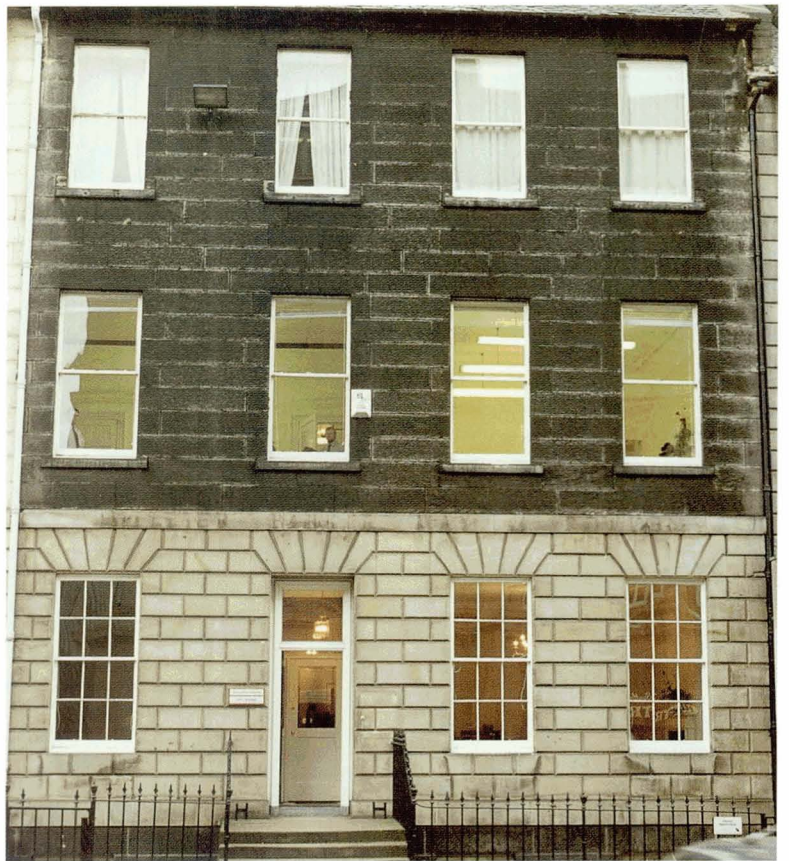
Plate 3.21 The detrimental aesthetic effects caused by the partial cleaning of a building.
