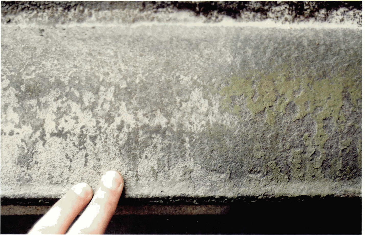
Plate 4.21 This thickly encrusted organic growth has not been removed by low pressure grit blasting.
