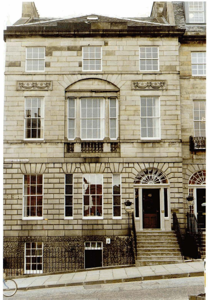
Plate 3.18 Cleaned sandstone facade.
