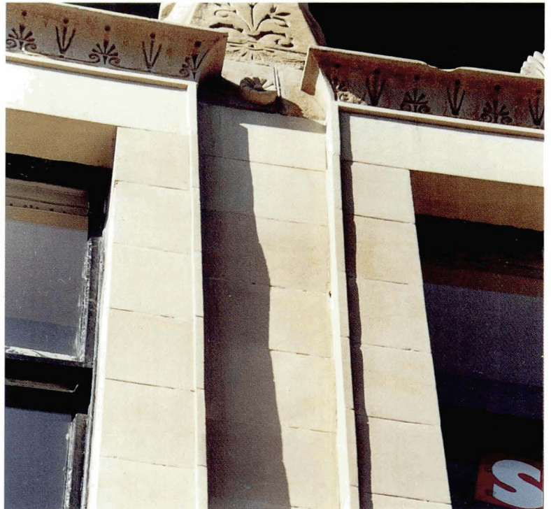
Plate 4.24 Following cleaning this arris is no longer straight, as the shadow shows.
