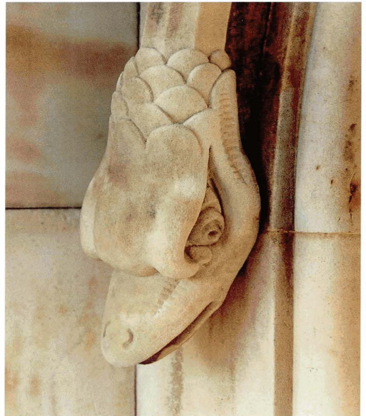
Plate 3.8 After cleaning. Much improved contrast after cleaning helps reveal sculptured details.
