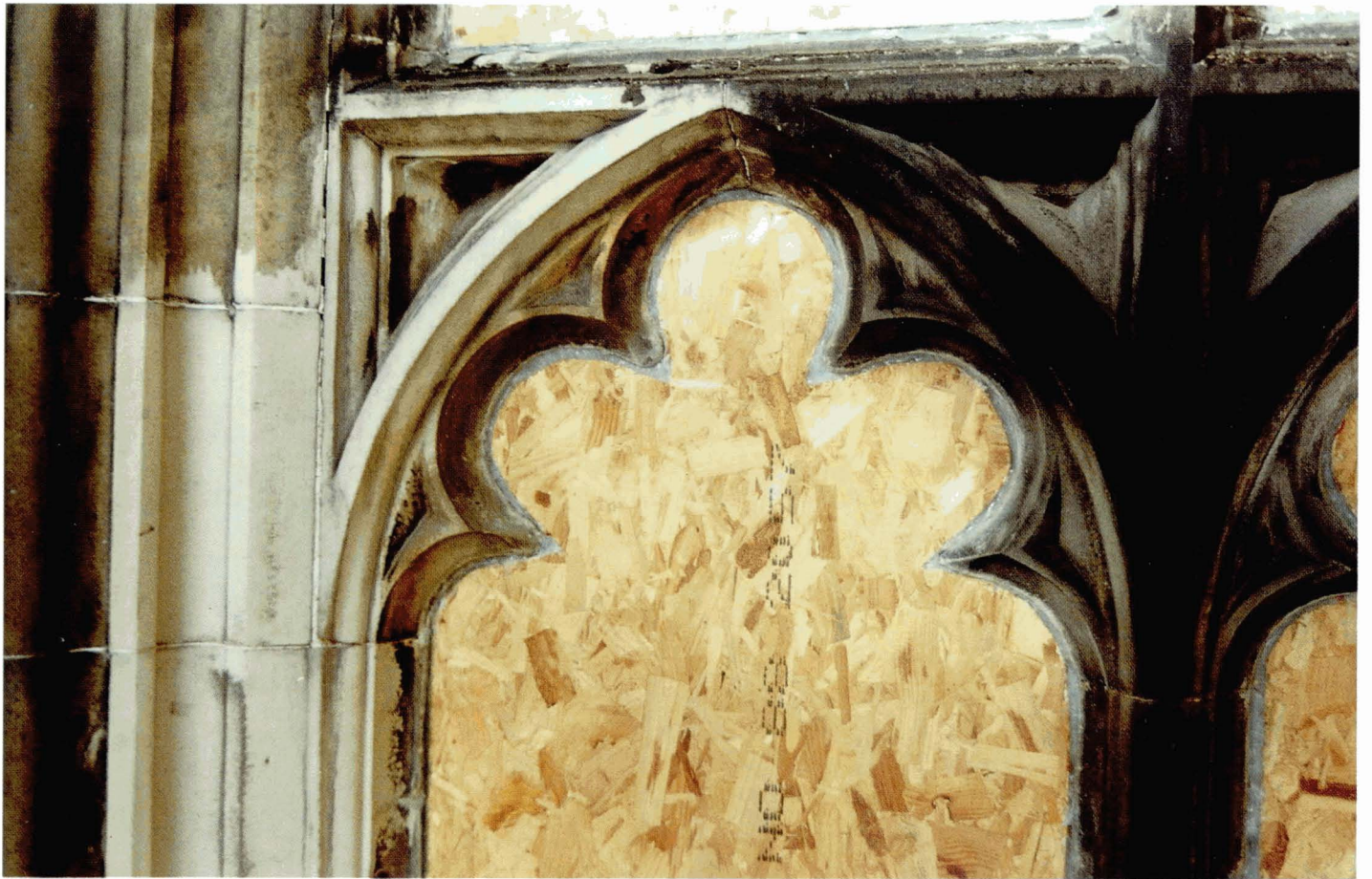
Plate 5.13 Proper protection of areas from which chemicals are to be excluded is essential.
