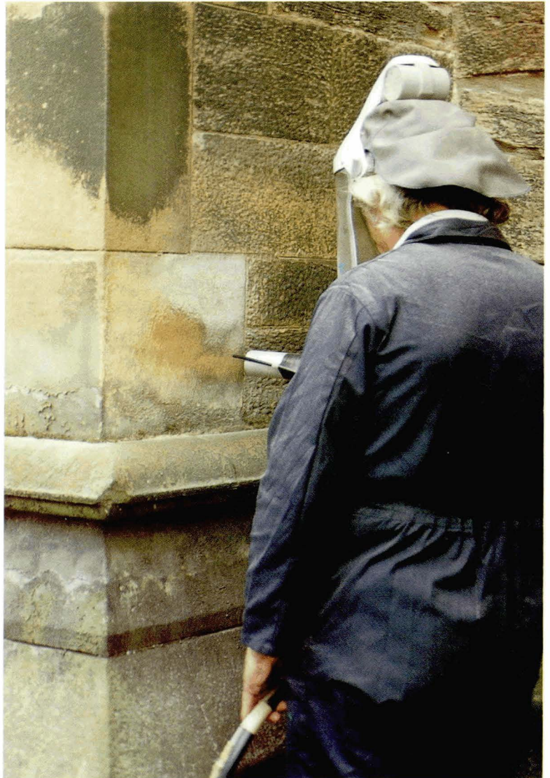
Plate 4.16 Low pressure grit blasting in operation.
