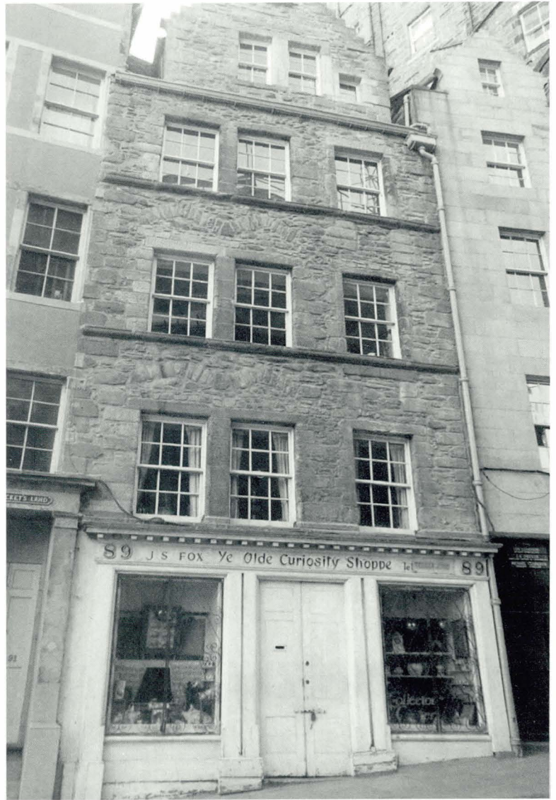
Plate 4.23 A rubble constructed building cleaned by dry brushing.
