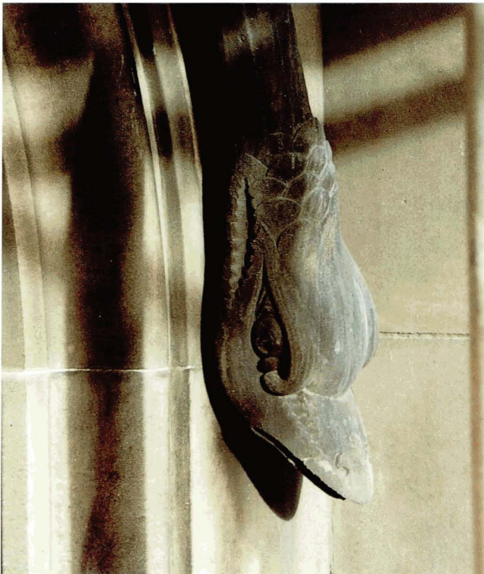
Plate 3.7 Before cleaning. Area of soiled detail showing obscuration of features.
