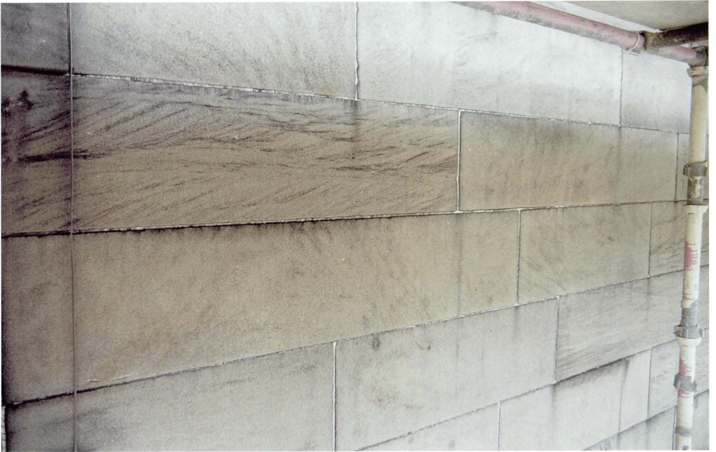
Plate 4.1 Sandstone building before grit blasting. Note how soiling on smooth faced stones tends to follow particular horizons.
