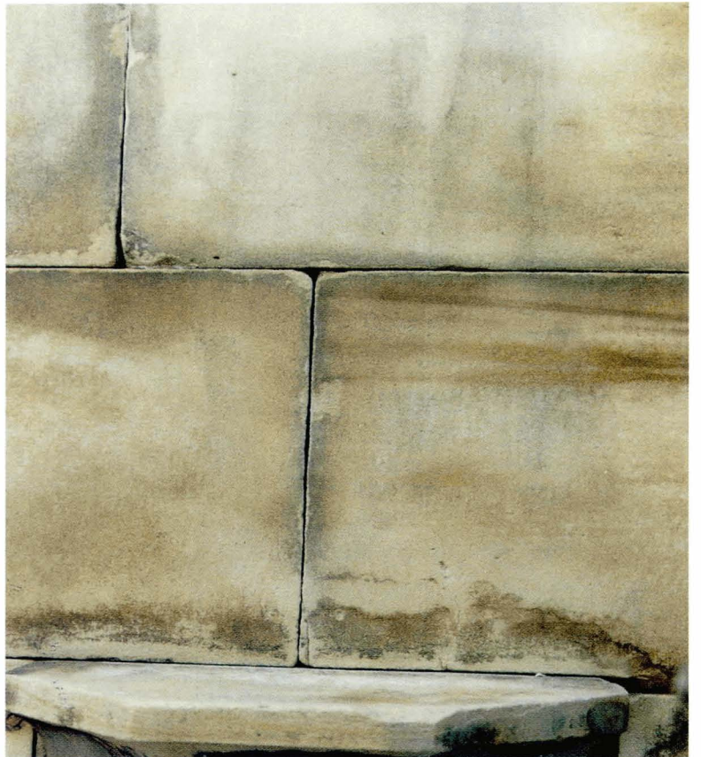
Plate 5.7 Same area as above one month after cleaning, showing temporary disappearance of efflorescences. Efflorescences are ephemeral and come and go as temperature, humidity and moisture levels change in the stone.
