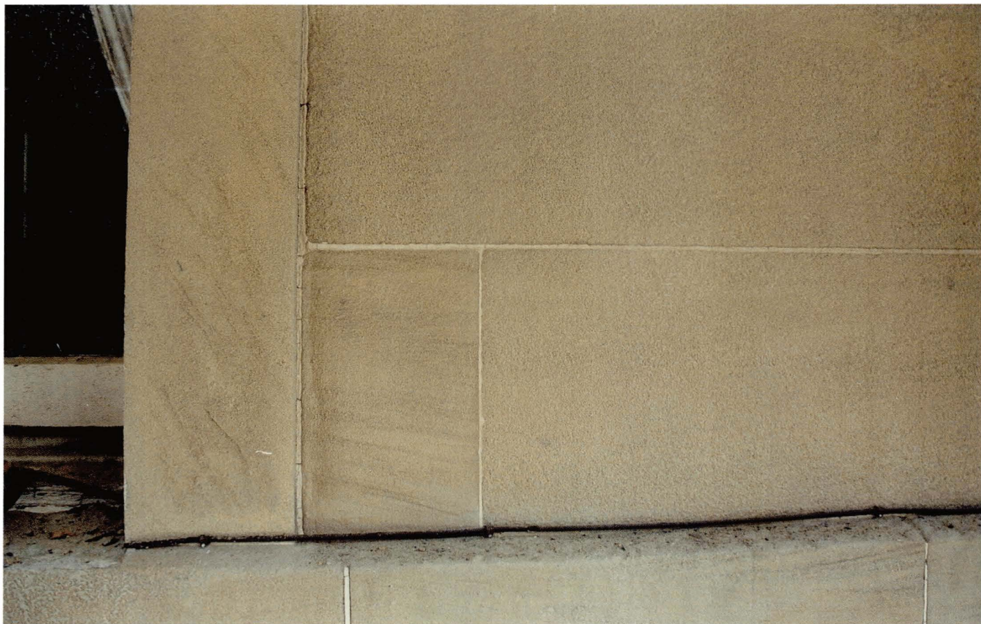
Plate 3.25 Soiling in these bedding planes is aesthetically acceptable and may enhance the appearance of the stone.
