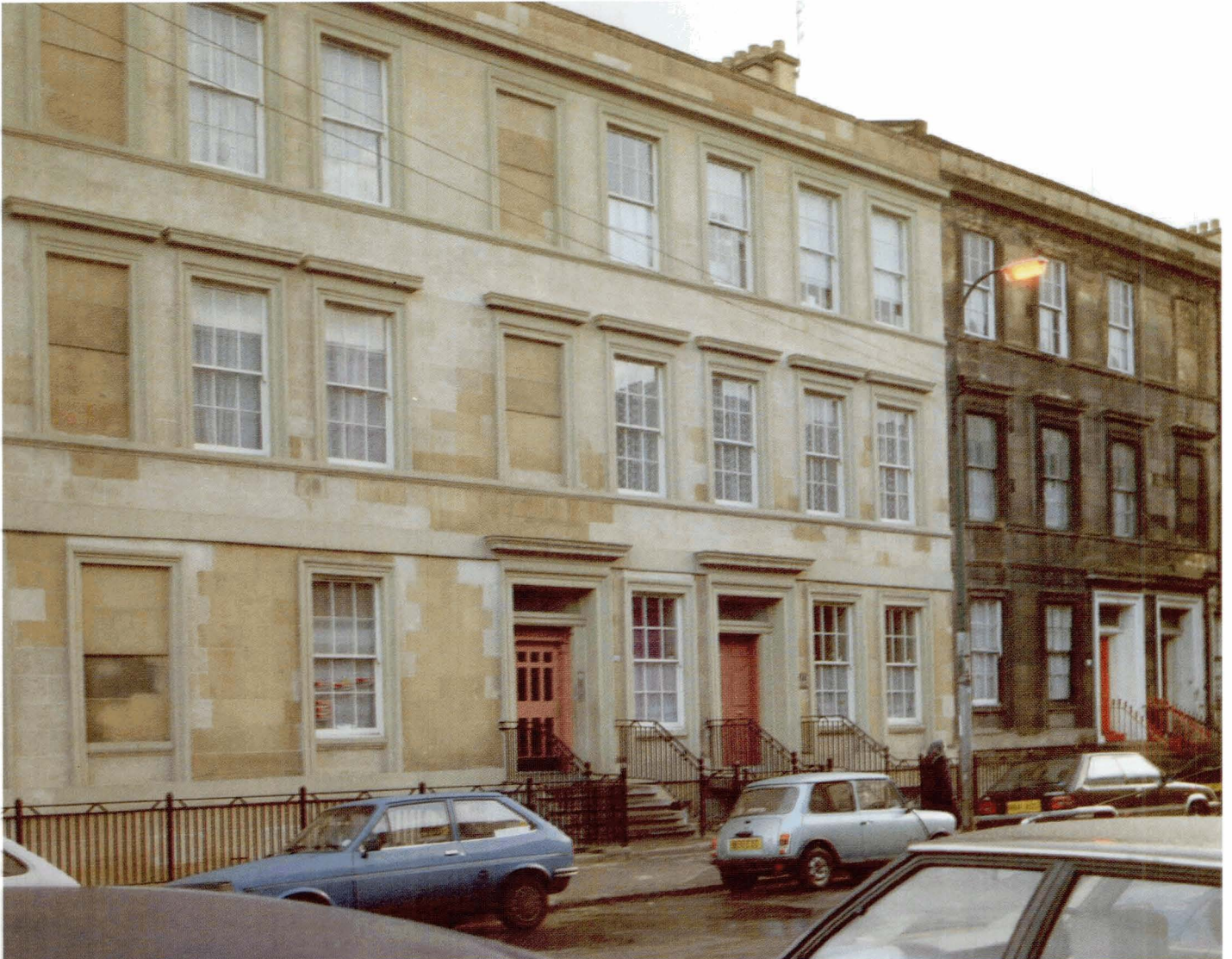
Plate 3.19 Stonecleaning in a residential street.
