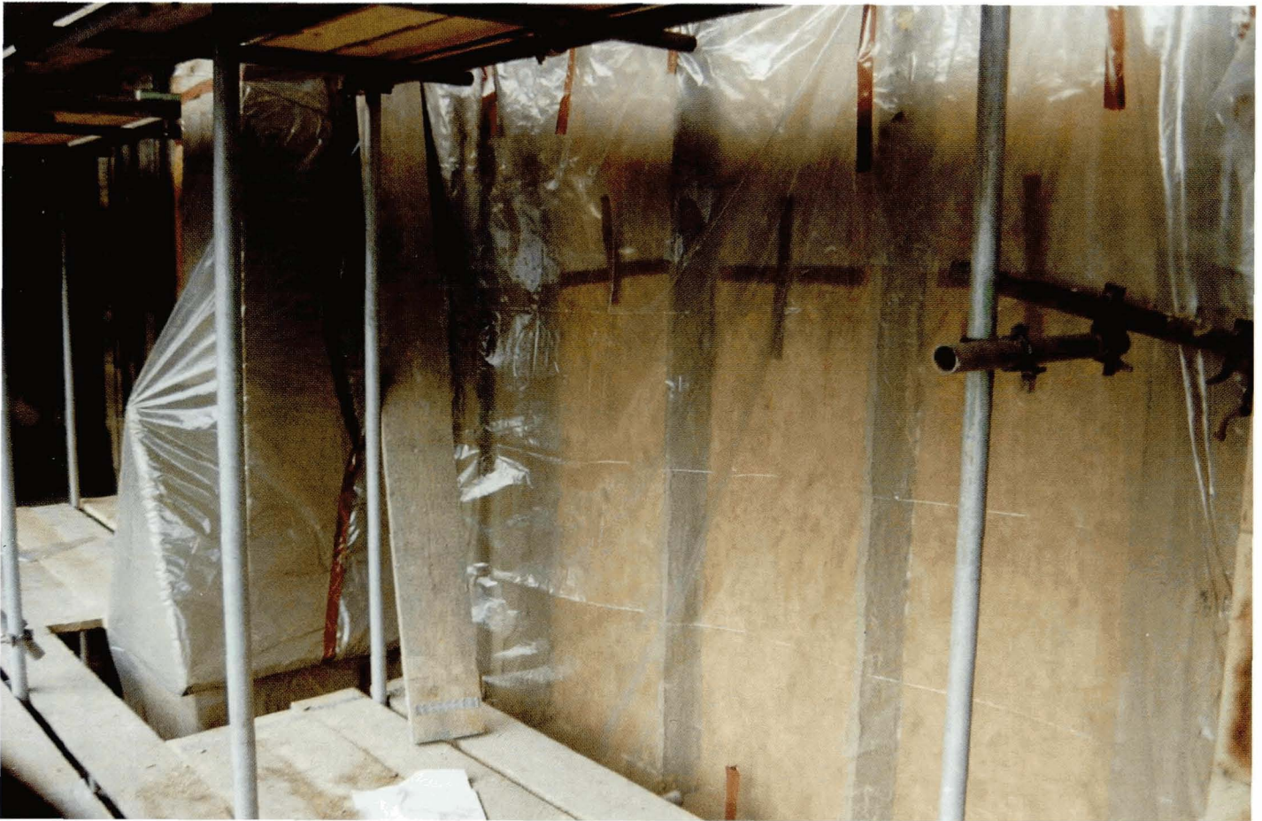
Plate 5.14 Poultice cleaning. Plastic film in place to prevent poultice drying out.
