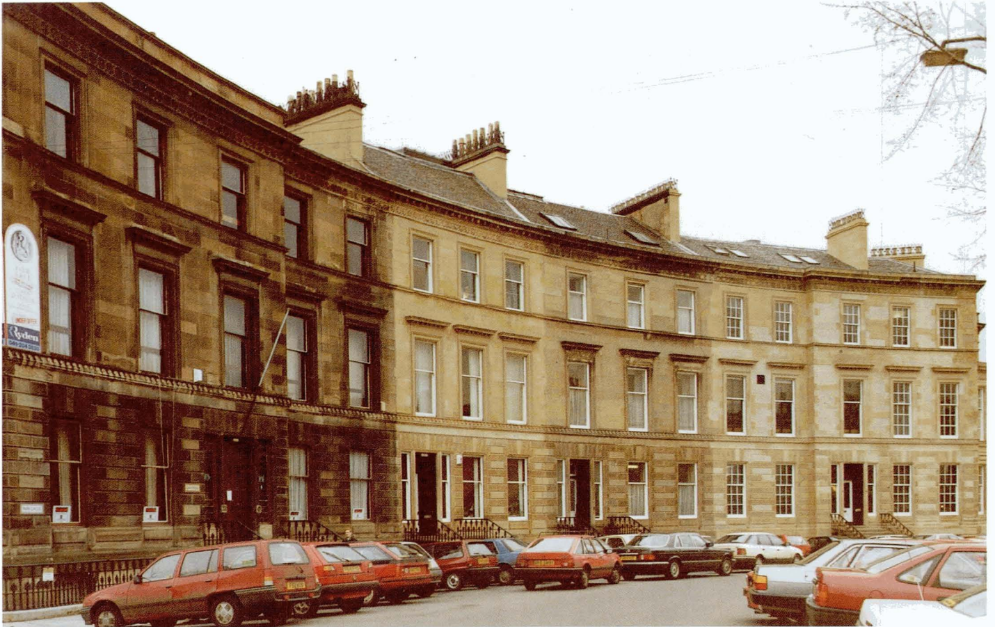
Plate 3.4 15-21 Park Circus, Glasgow. The properties in this crescent have been cleaned on an individual basis. The result is not as pleasing as 22-29 Park Circus which was cleaned as a single unit (Plate 3.5).
