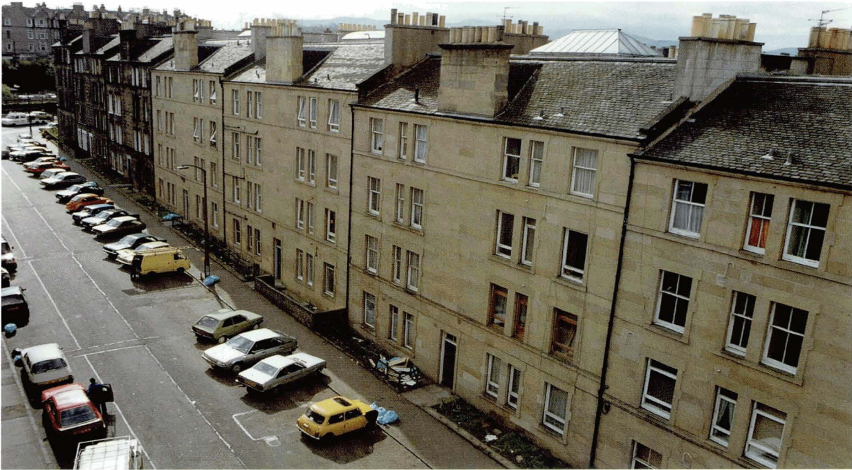
Plate 3.6 The cleaning of these tenements has resulted in a marked increase in reflected light at street level.
