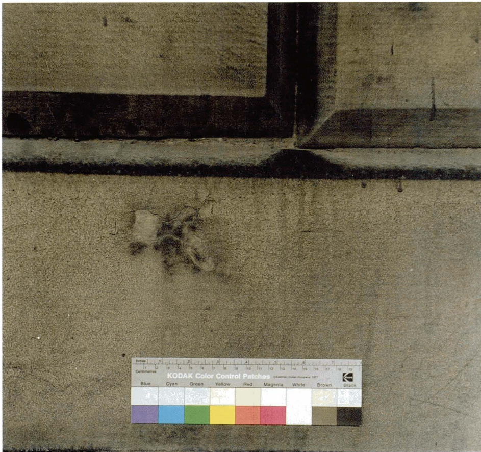
Plate 3.12 Soiled ashlar sandstone before cleaning. Note how soiling tends to obscure stains and small blemishes on the masonry surface.
