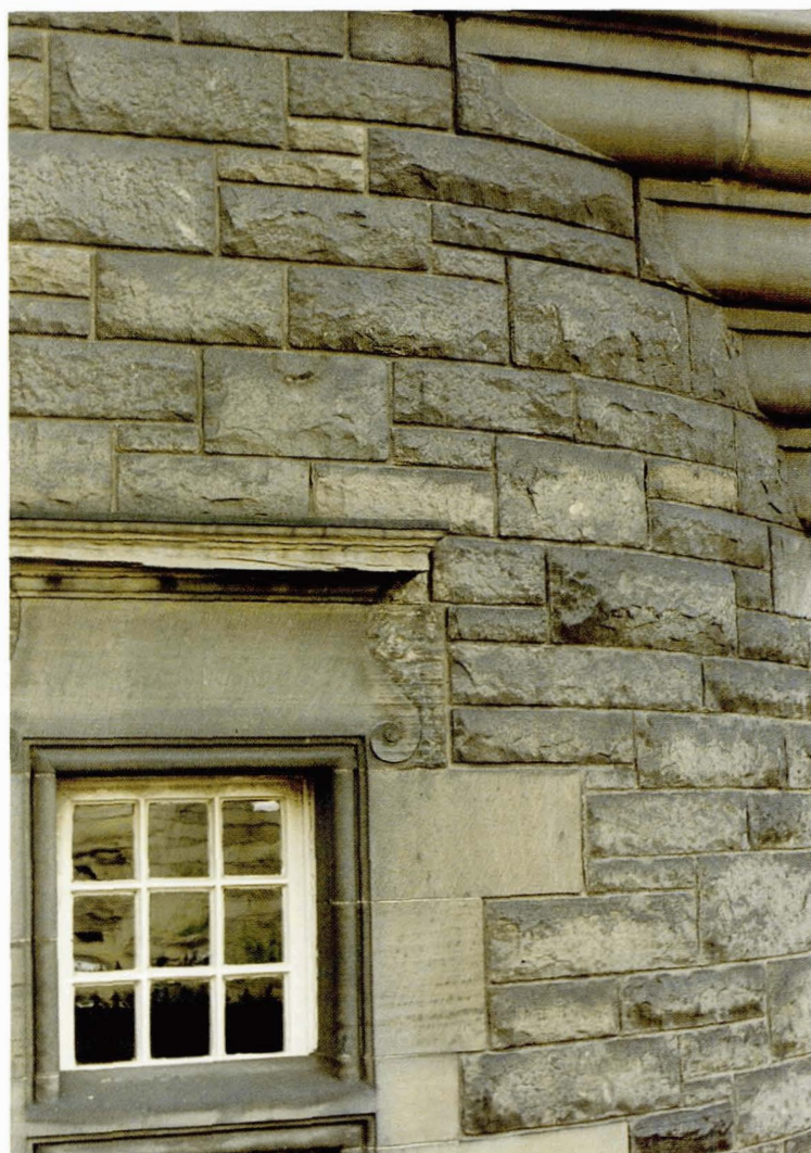
Plate 3.24 Soiling on rock faced stone. A low level of soiling can add to the visual complexity of a building and is not necessarily aesthetically detrimental.
