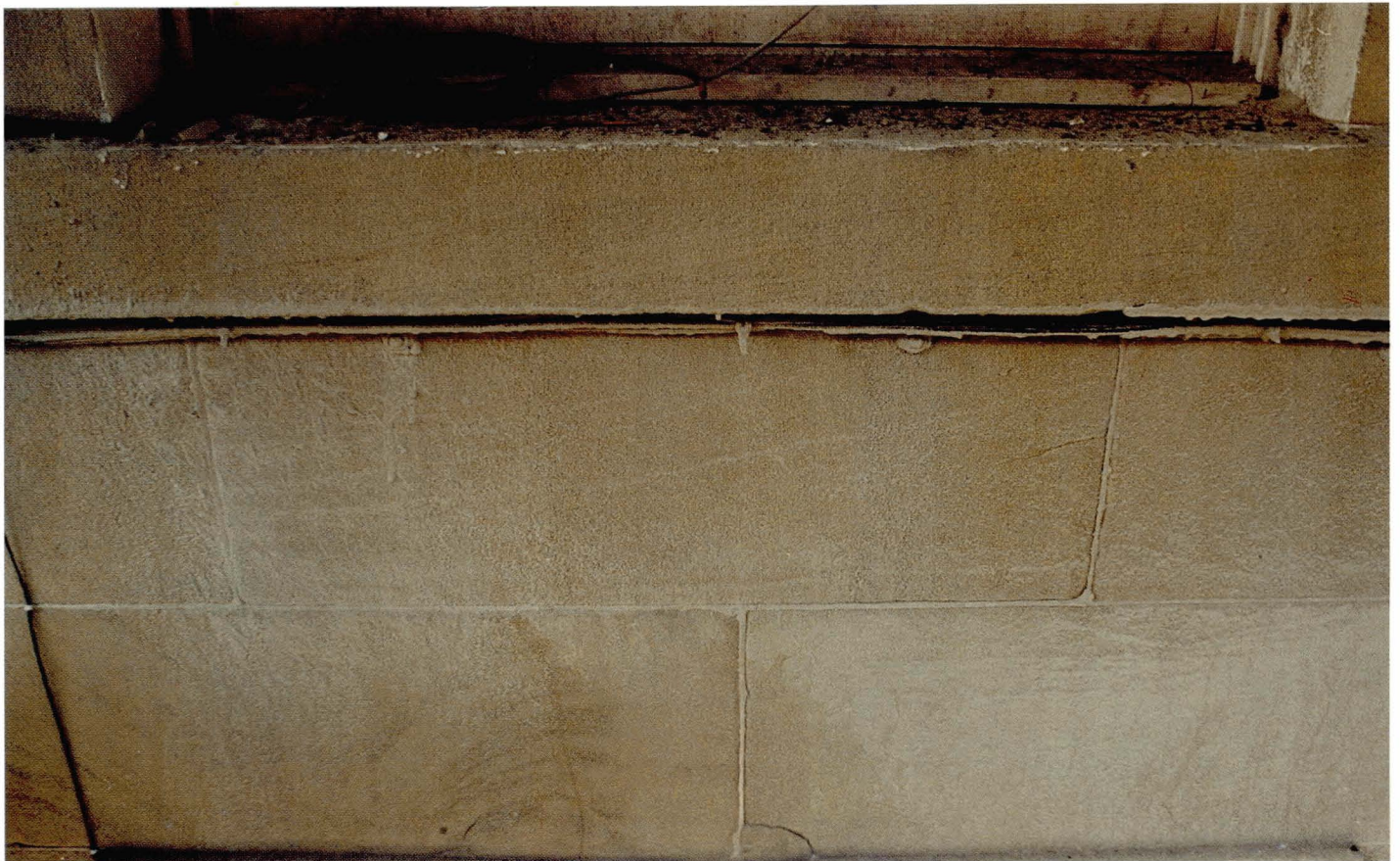
Plate 4.26 After wet grit blast cleaning (same area as above). Algal growth completely removed.
