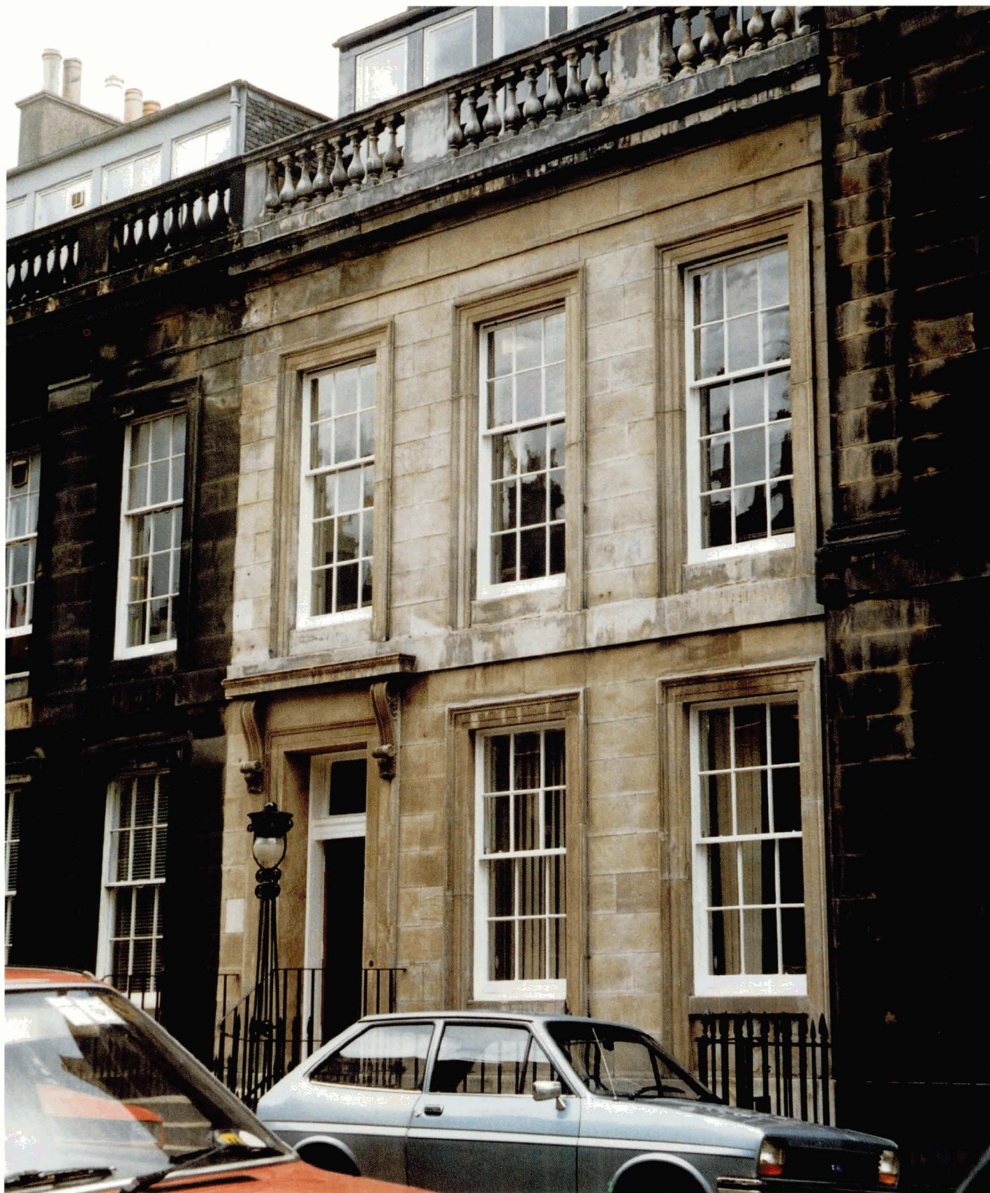
Plate 3.11 Part of a partially cleaned sandstone terrace.
