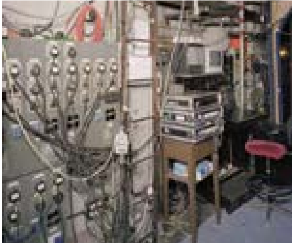
Illus 62 Theatres often have high intensity lighting, upholstered seating, large open-plan auditoriums, combustible props, stage production areas and special effects, all of which can create a high fire risk © Crown Copyright: RCAHMS. Licensor www.rcahms.gov.uk
