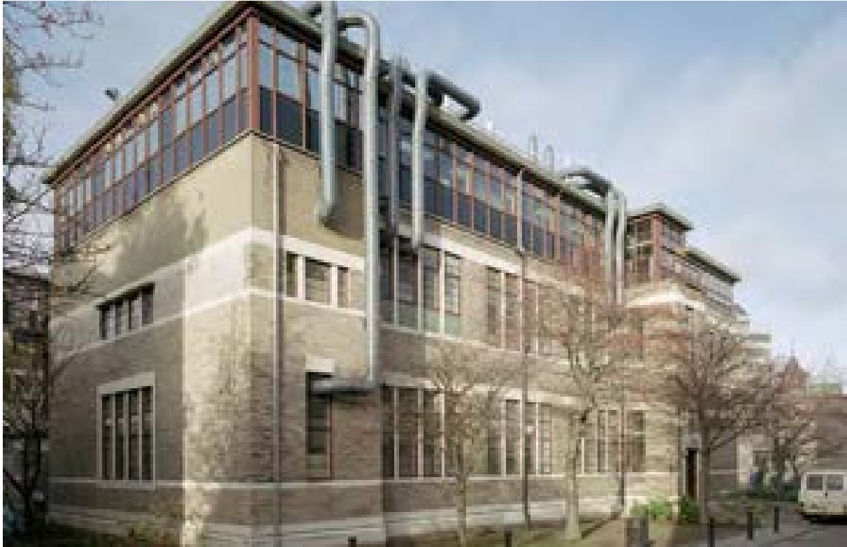
Illus 63 A category A listed University chemistry building is an obvious high fire risk © Crown Copyright: RCAHMS. Licensor www.rcahms.gov.uk
