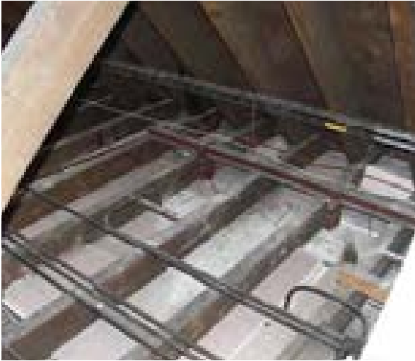
Illus 55 The wires have been fixed using cable clips rather than notching the timbers
