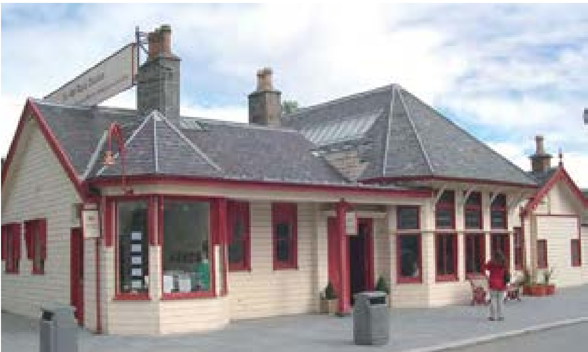
Illus 10 Successful conversion of the redundant Old Royal Station at Ballater into a museum, restaurant, shops and tourist centre © Denis Urquhart
