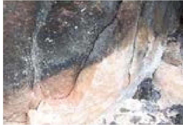
Illus 30 A localised fire that has caused discoloration of the sandstone in the area affected by flames and the stone above has been covered by soot. The heat also caused fracturing of the stone and loss of material © Dr Stephen McCabe
