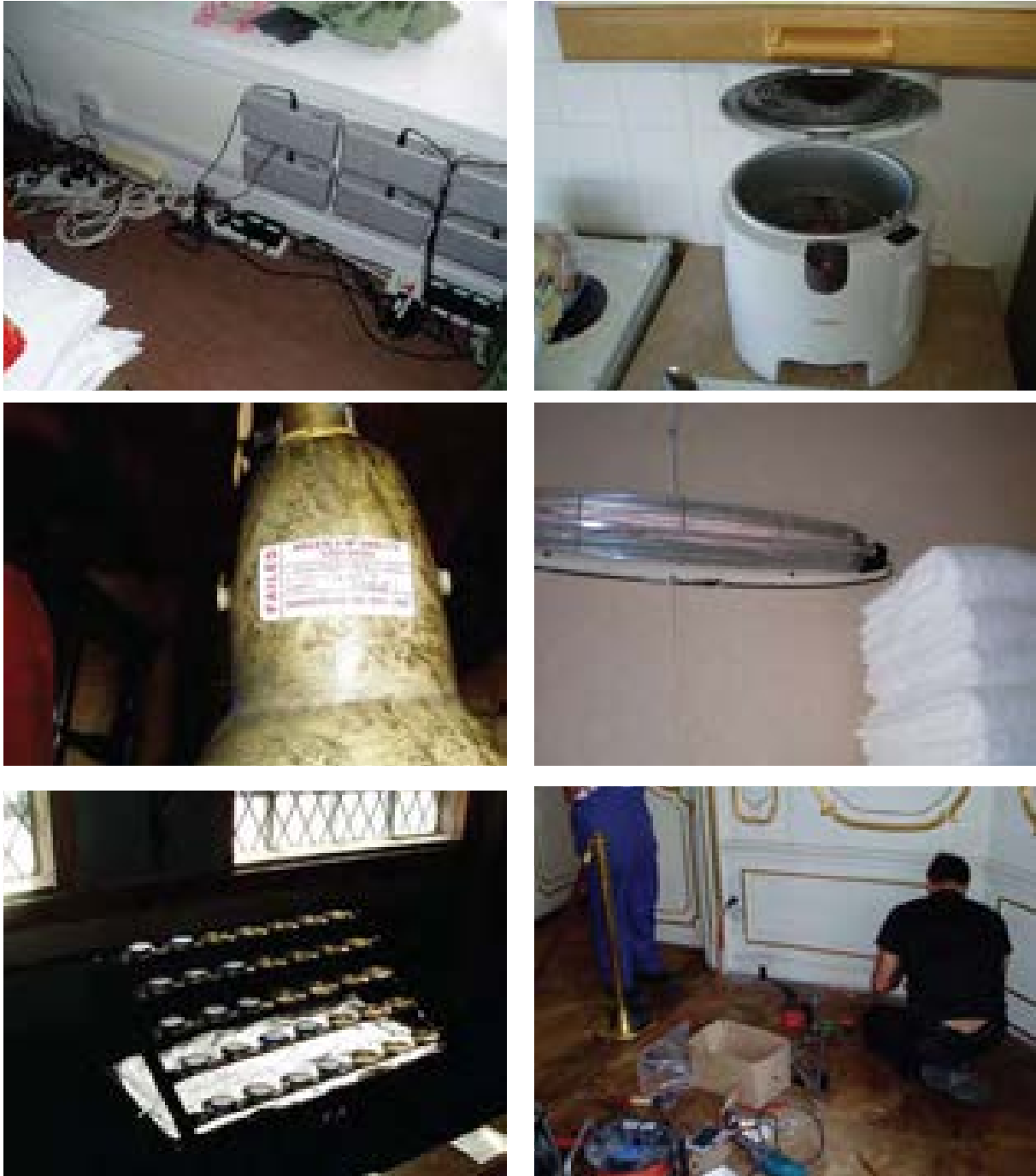
Illus 43 Some major contributory causes of fire include; overloading of circuits, neglecting to undertake routine electrical equipment checks, church candles, deep fat fryers, combustible material in close proximity to heaters and blow torches © Stewart Kidd
