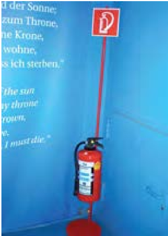
Illus 52 Where fire extinguishers are required to comply with legislation, subject to agreement with the fire authority there is no reason why they can't be allowed to be free standing as opposed to being physically attached to the wall © Stewart Kidd
