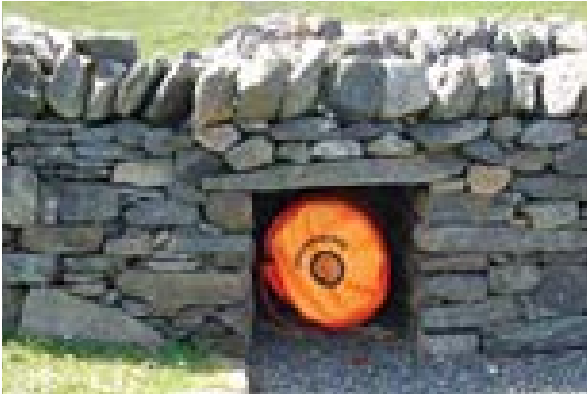
Illus 40 Fire represents a serious risk for thatched properties. Here the design for a contemporary enclosure for a fire hose has employed random rubble stonework like that used in the adjacent blackhouses, a visually sensitive approach
