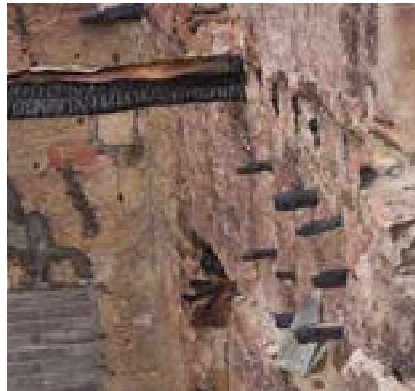
Illus 19 It is common practice in traditional buildings for floor and ceiling timbers to be built into supporting walls
