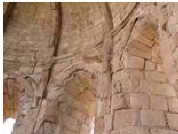
Illus 31 Fires have always been a threat - here the effect of a historical fire is evident by the severe spalling of the granite, especially around the windows © Dr Miguel Gomez-Heras
