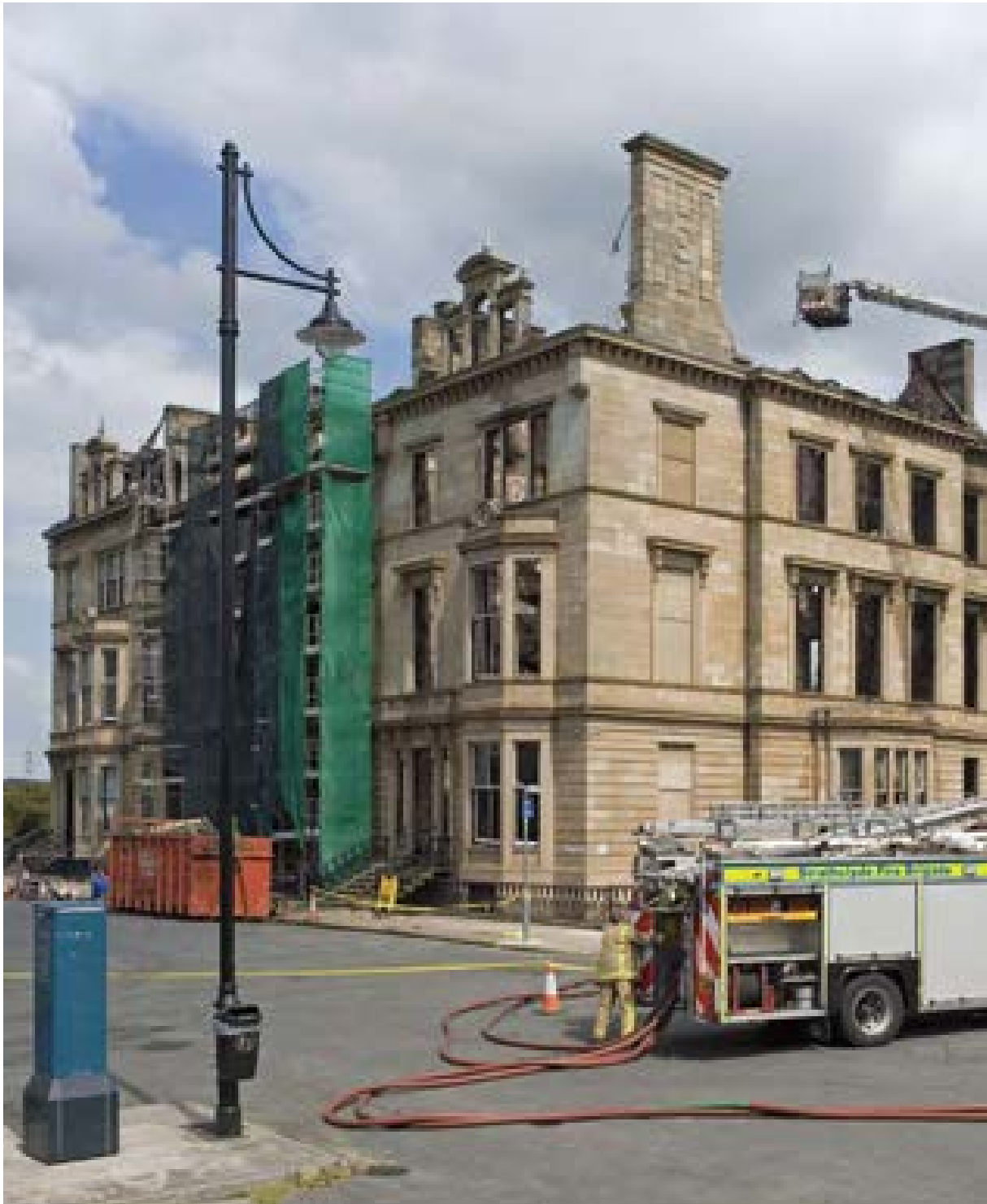
Illus 1 The aftermath of a serious fire in this category A listed terrace undergoing refurbishment © Crown Copyright: RCAHMS. Licensor www.rchms.gov.uk
