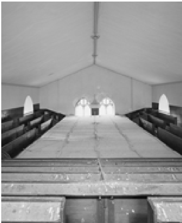
Illus 48 Suspended ceiling in this church, a consequence of a decreasing congregation size, has created a large cavity above © Crown Copyright: RCAHMS. Licensor www.rcahms.gov.uk
