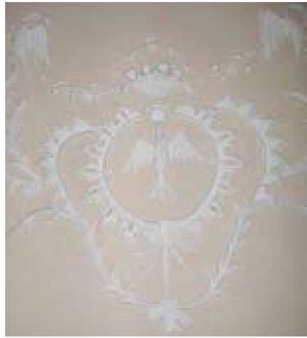
Illus 53 A concealed sprinkler head has been installed immediately in front of the bird's beak, almost invisible to the untrained eye © Stewart Kidd
