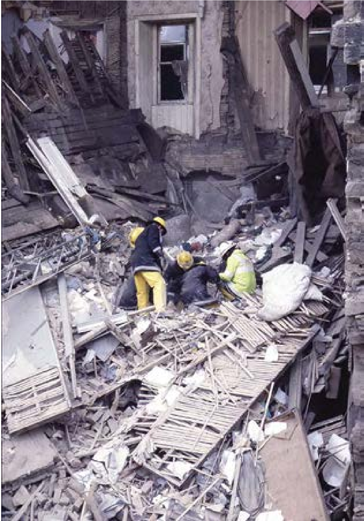
Illus 50 Fire Service personnel amidst the rubble following a gas explosion at Guthrie Street, Edinburgh © Lothian and Borders Fire and Rescue Service.
