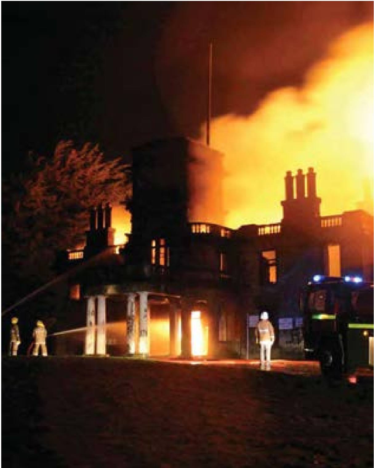
Illus 2 A fully developed fire in a country house © Central Fire and Rescue Service
