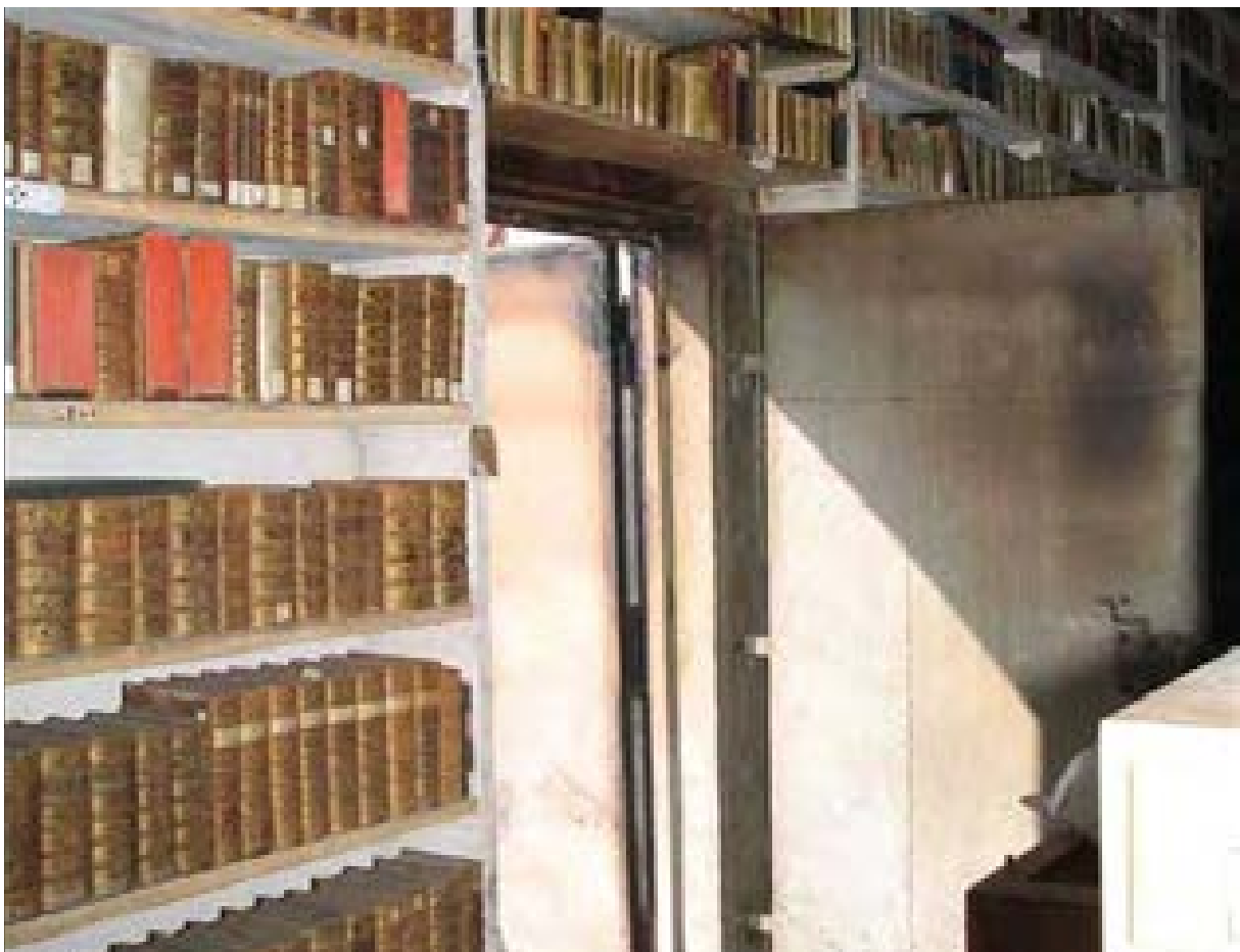
Illus 46 The benefits of compartmentation: complete loss on one side of the compartment wall and fire door and on the other side only superficial fabric damage and minor smoke damage to an archive of rare books, Anna Amalia Library, Weimar © Per Rohlén
