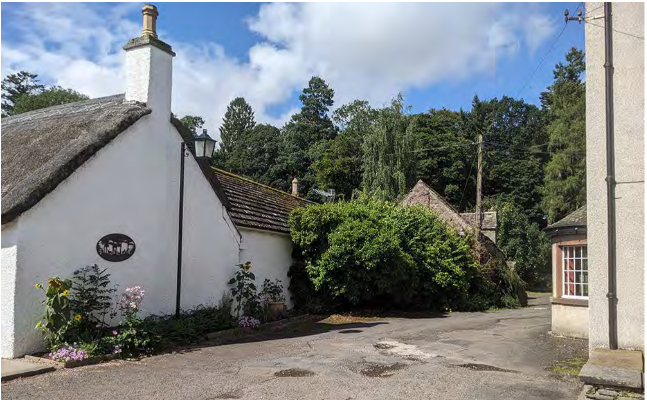
Figure 041: 1 Main Street, Glamis, Angus. The main roof is thatched, and the rear wing is roofed in flagstone. © Sara Carruthers.
