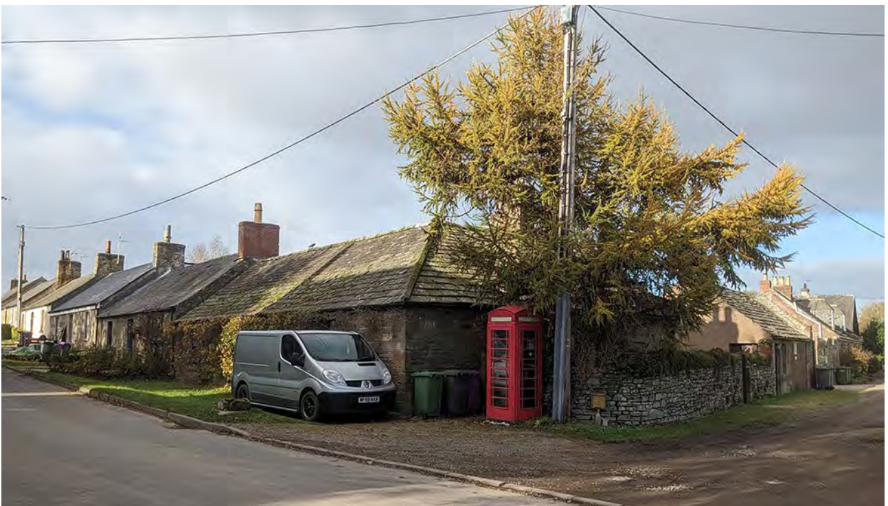
Figure 036: One of a row of quarrymen's cottages near to Leysmill Quarry, as well as an outbuilding. Near Arbroath, Angus. © Sara Carruthers.
