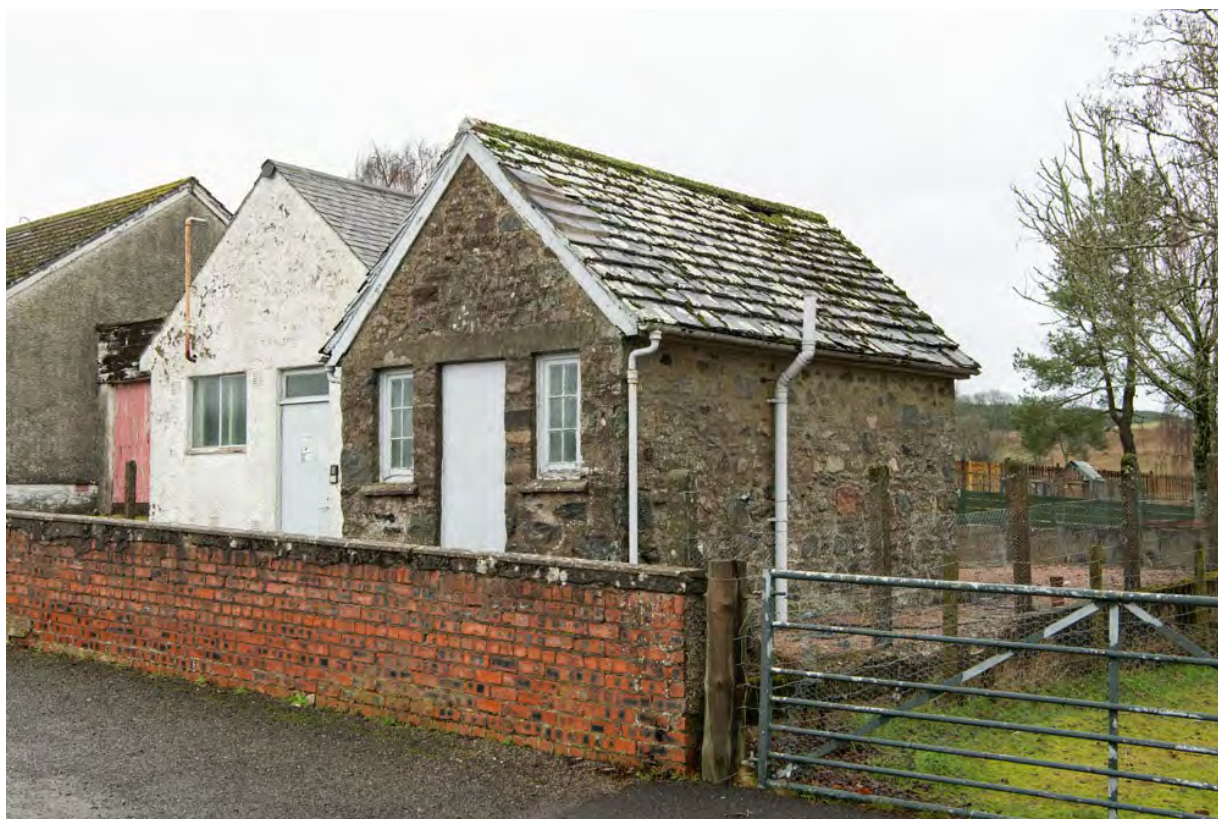
Figure 177: Telephone exchange, Dykehead, Angus.
