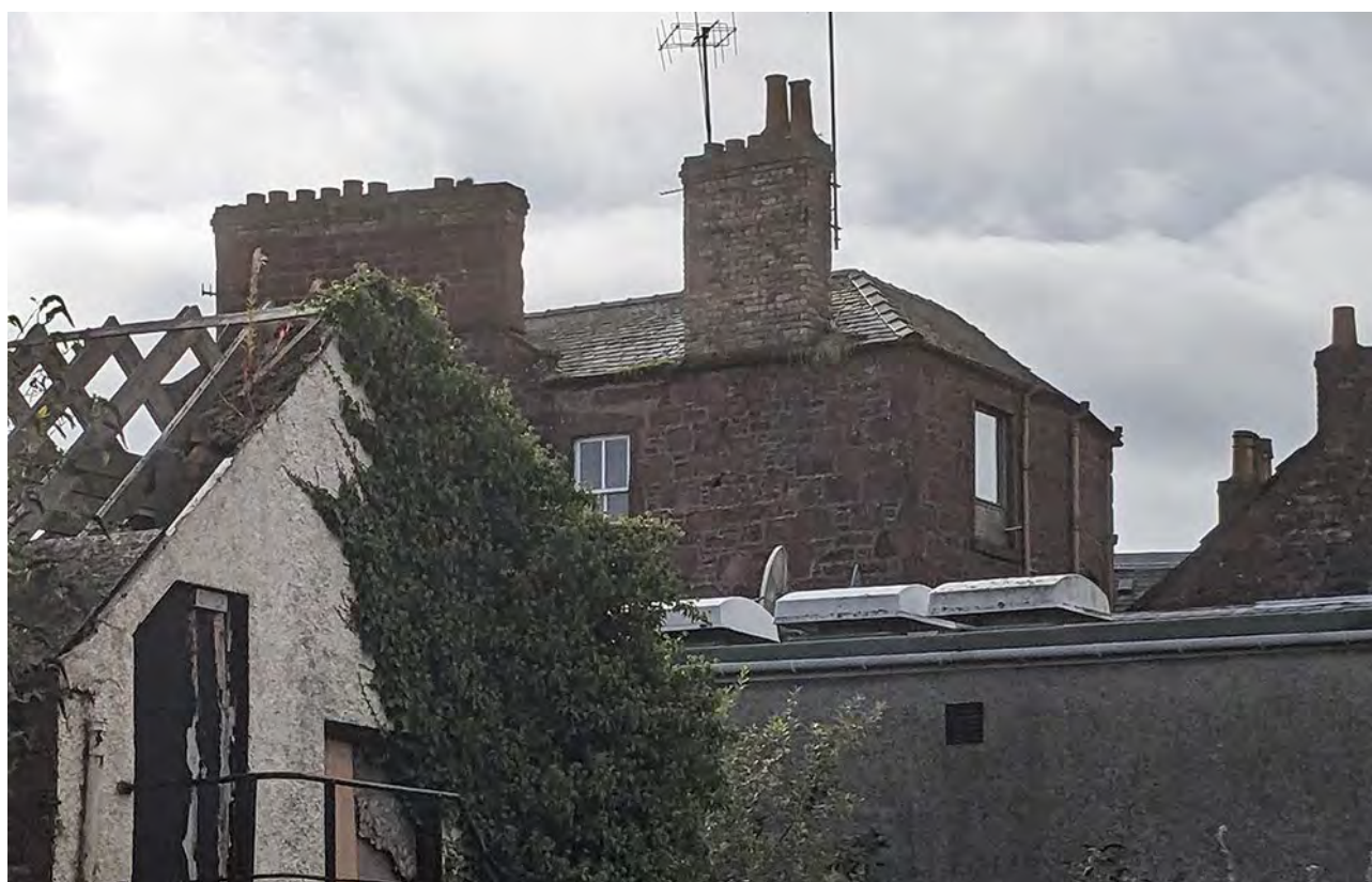
Figure 194: Originally called the Union Hotel, Kirriemuir, Angus. Piles of flagstone slates in the rear garden show previous use on the main building or an outbuilding. © Sara Carruthers.
