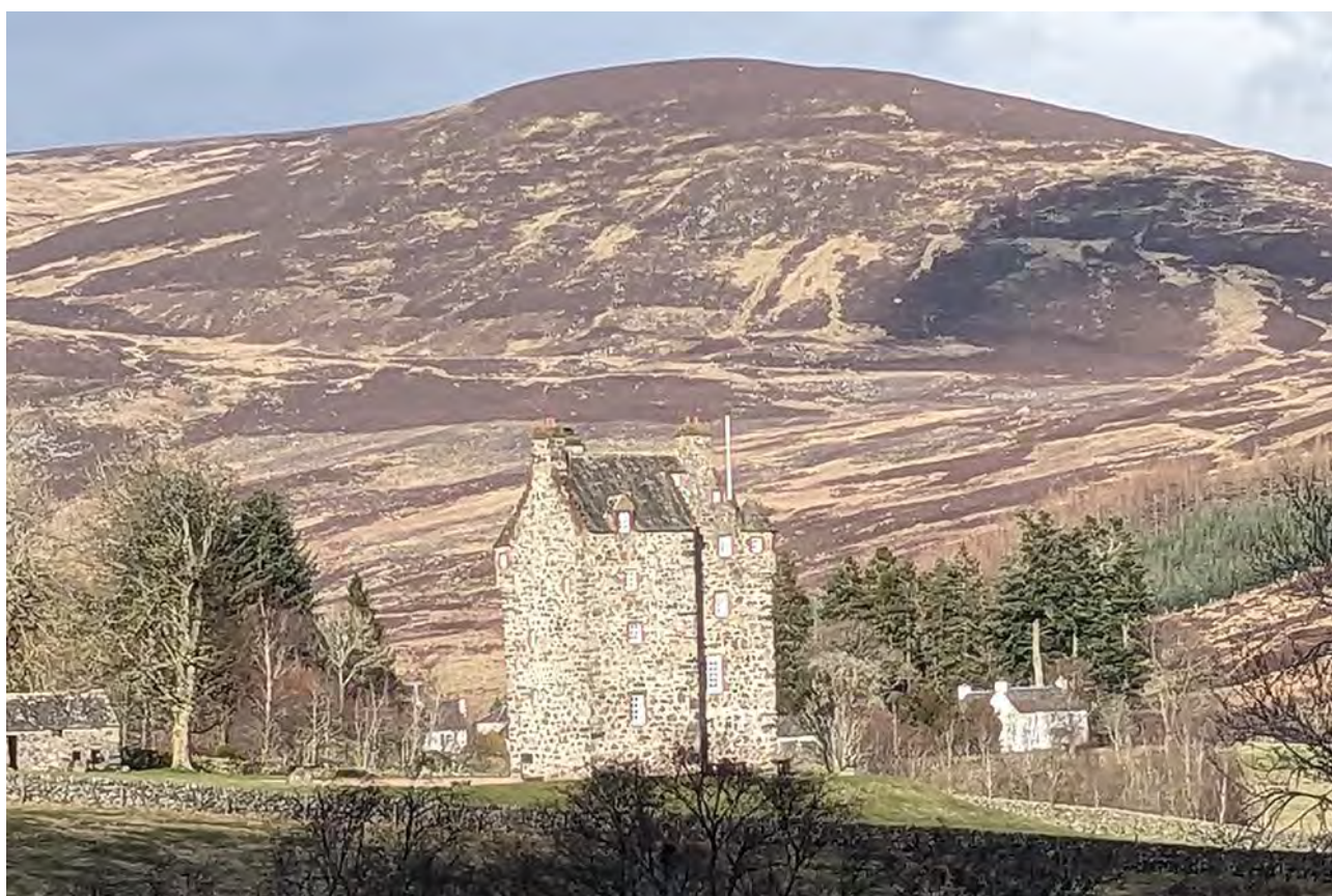
Figure 131: Forter Castle, Kirkton of Glenisla, Angus. The property was re-roofed in flagstone in 2000. © Sara Carruthers.
