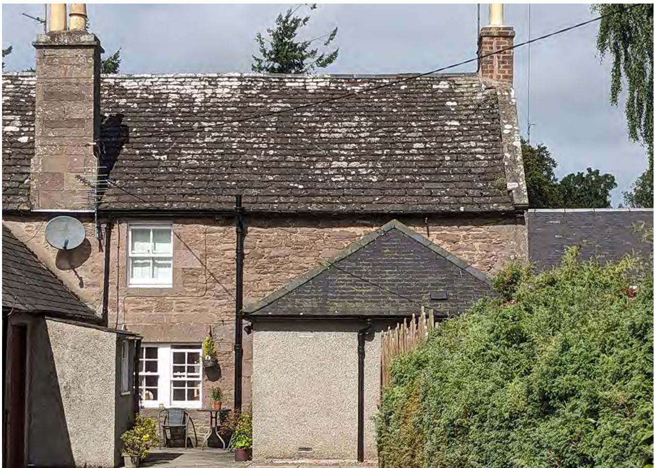
Figure 038: 6-7 The Square, Glamis. Angus flagstone is found only on the rear elevation. © Sara Carruthers.
