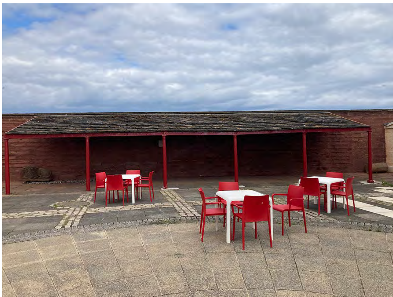
Figure 008: Outbuilding at Bell Rock Signal Tower, Arbroath, Angus. © Sara Carruthers.
