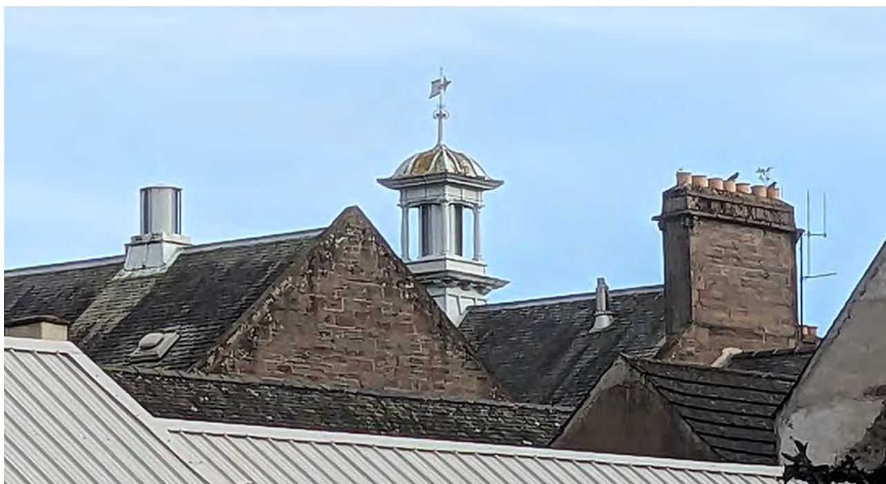
Figure 101: The rear wing of 24 West High Street, Forfar, Angus. It has a flagstone roof, seen here in the middle distance. © Sara Carruthers.
