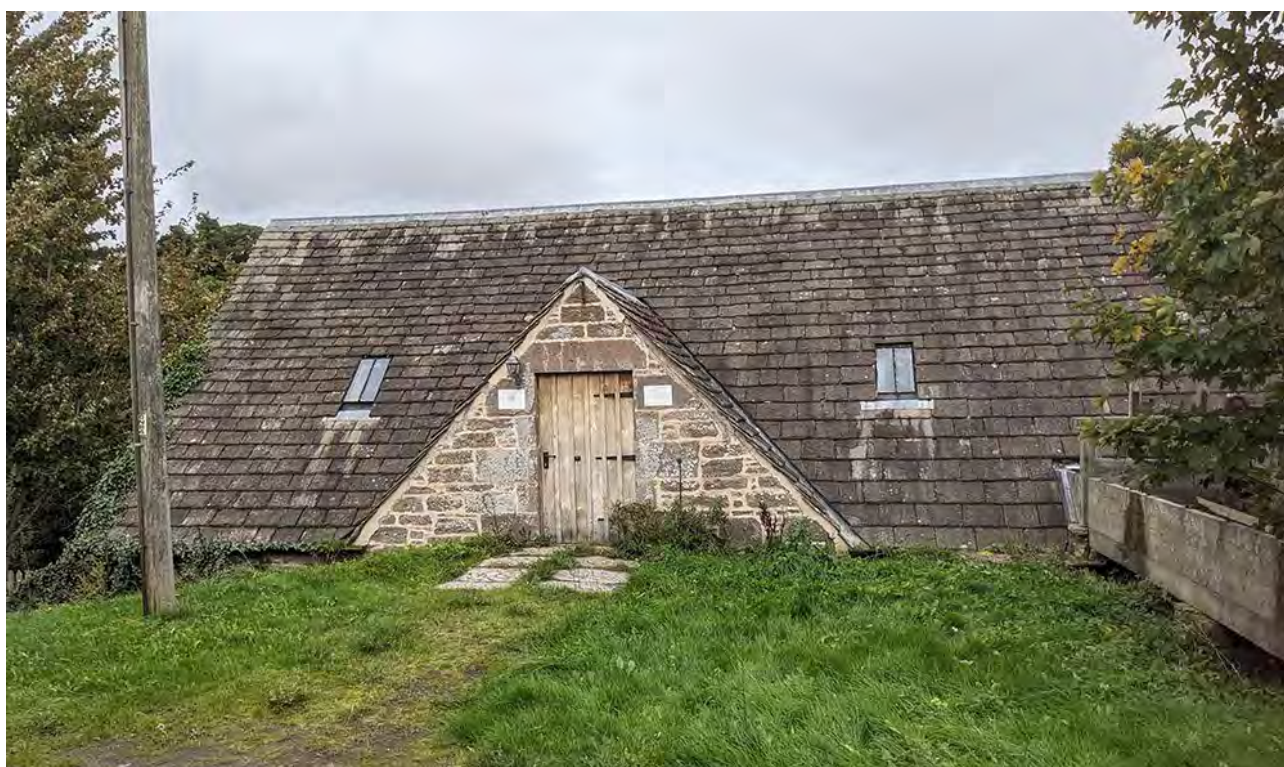
Figure 115: The flagstone roof of Lera Mill, Glamis, Angus. The building contains a working waterwheel. © Sara Carruthers.
