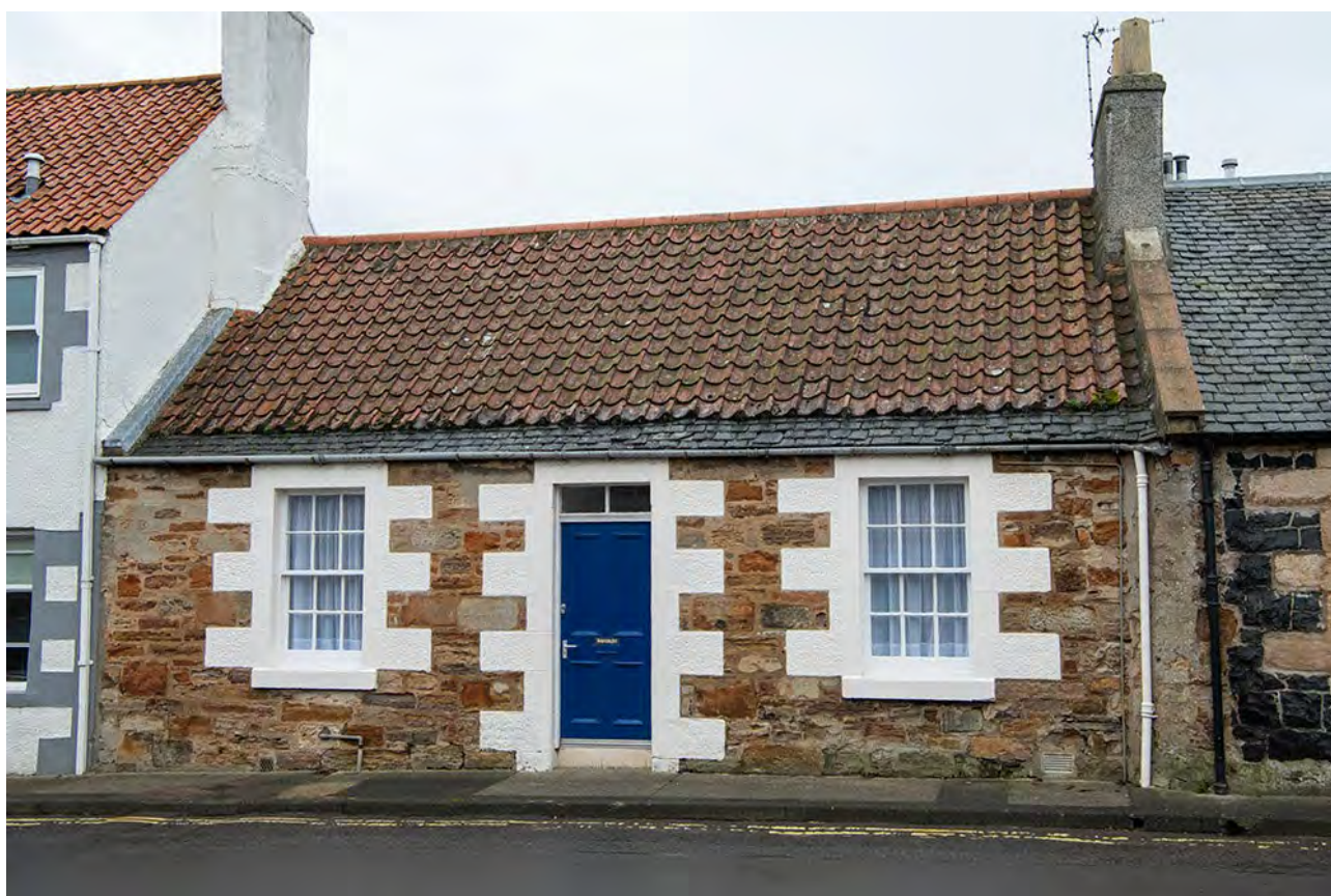
Figure 214: High Street, Earlsferry, Fife. Most of the roof is pantile, with the lower section flagstone.
