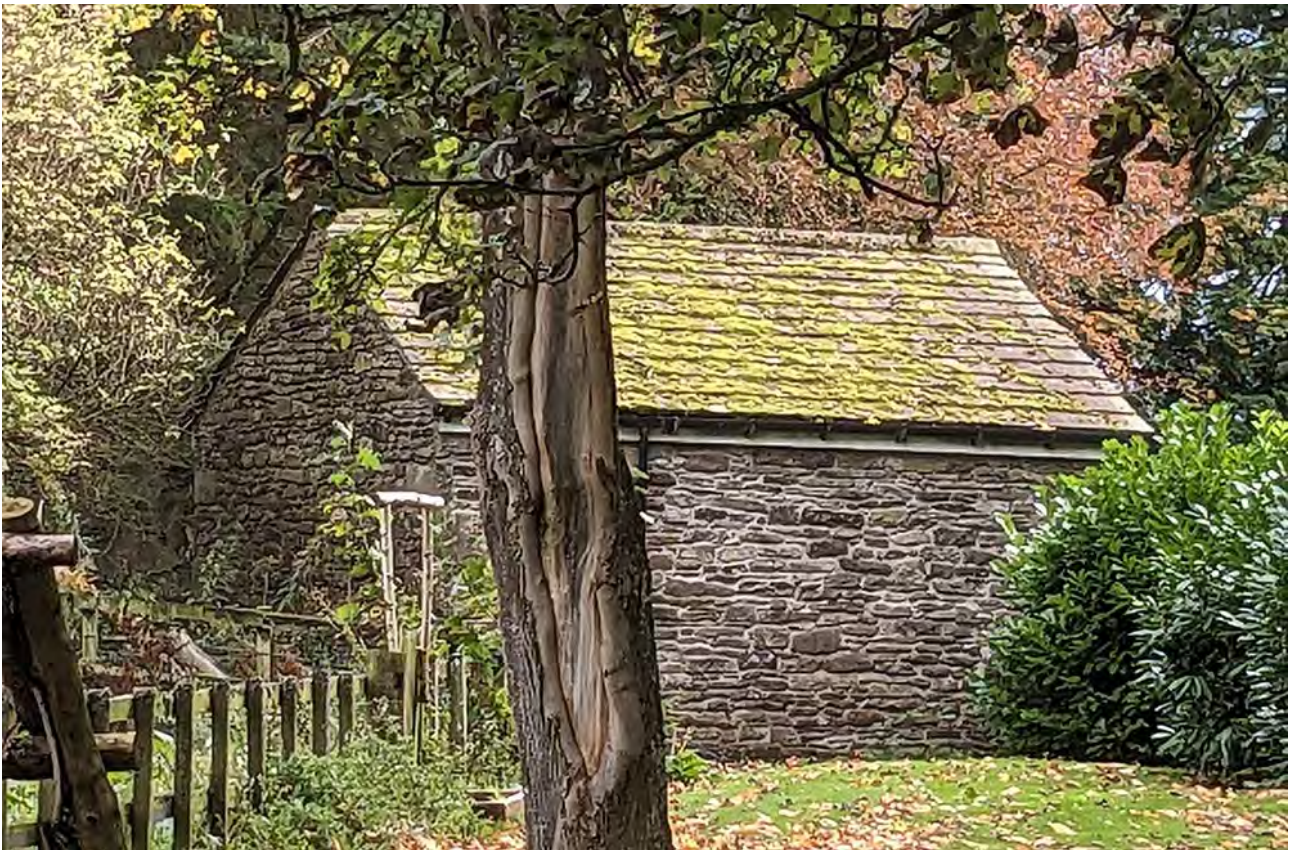
Figure 089: Outbuilding at Ballindarg House walled garden, Angus. © Sara Carruthers.
