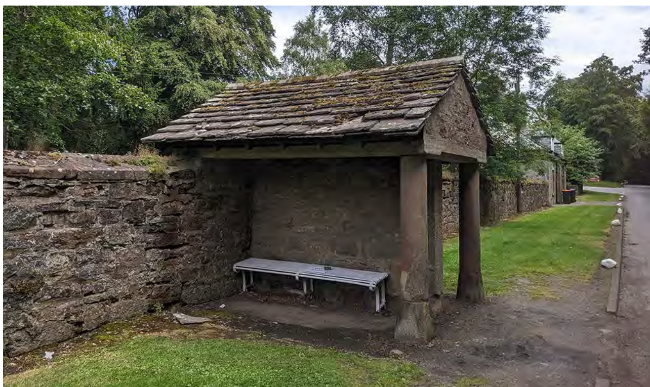
Figure 228: Public shelter on the B966 outside Edzell, Aberdeenshire. © Sara Carruthers.
