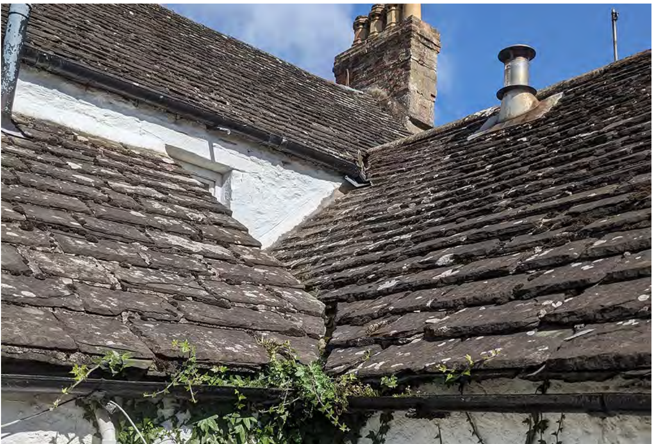
Figure 023: Roof detail, 8 & 9 The Square, Glamis, Angus. © Sara Carruthers.
