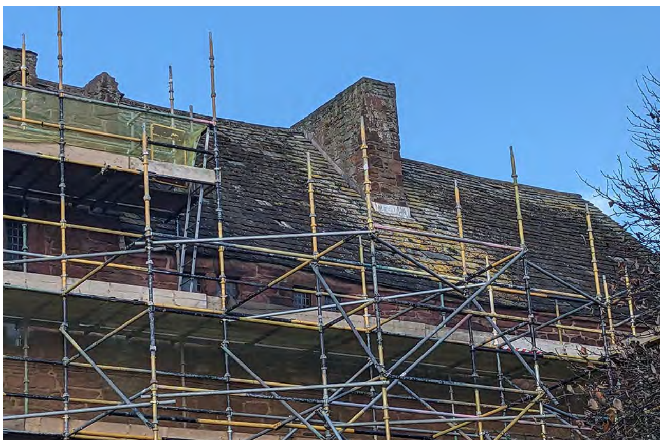
Figure 125: Part of Arbroath Abbey's structures, Angus. The Abbot's House (above) and a square tower both have flagstone roofing. © Sara Carruthers.
