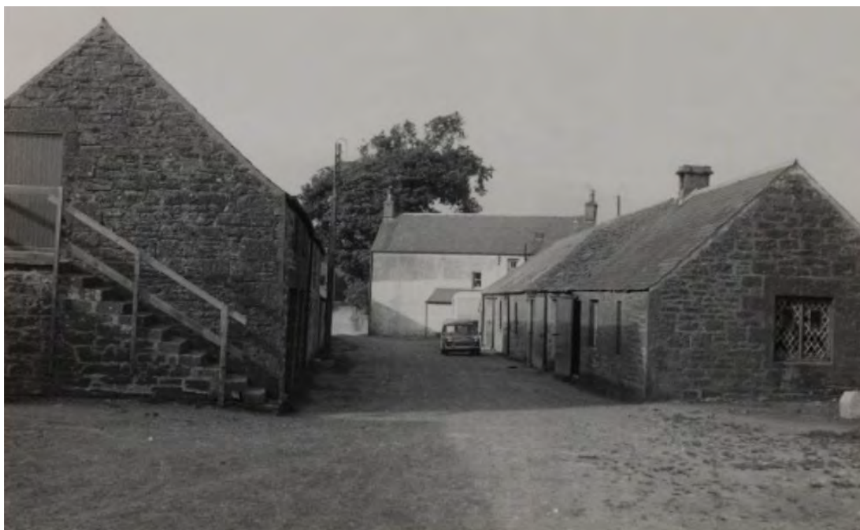
Figure 139: Steading building, Dryburn Farm, Forfar, Angus.
