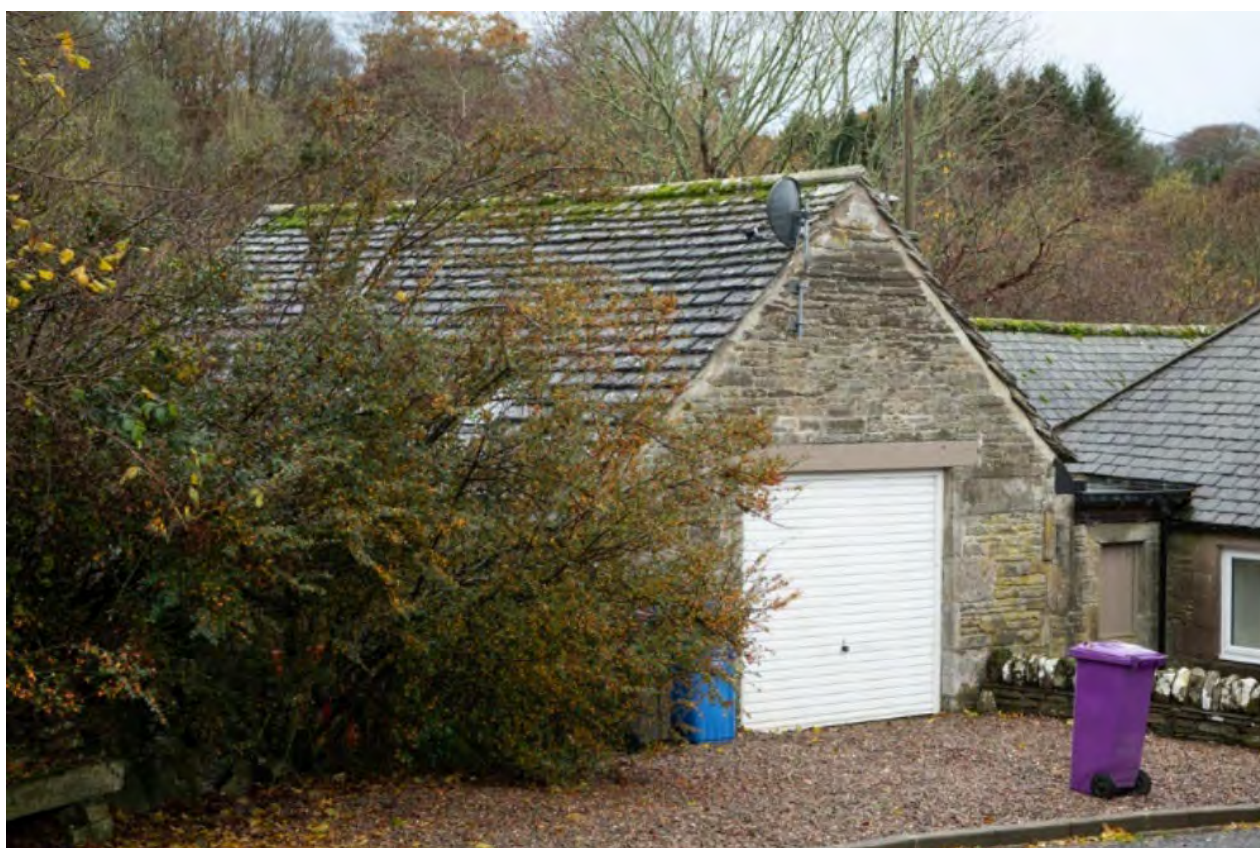
Figure 158: Garage building, West Milldens, Milldens, Angus.
