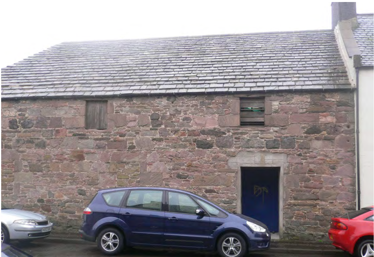
Figure 057: Flagstone-roofed barn is an ancillary structure to the later Links House Hotel, Montrose, Angus. © Mark Watson.
