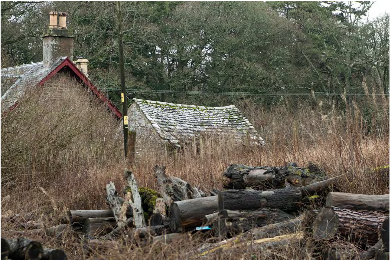
Figure 053: Cottage, Braehead Road, Glamis, Angus.
