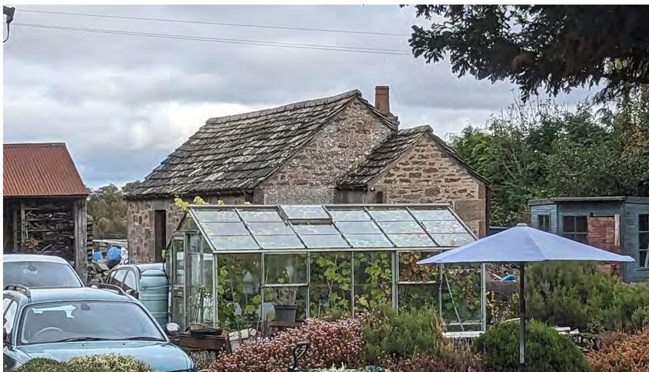
Figure 099: Outbuilding at Couttston Cottage, Newbarns, Angus. © Sara Carruthers.
