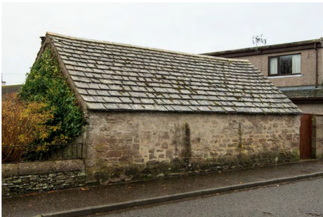
Figure 150: Outbuilding, Watson Street/East Hemming Street, Letham, Angus.
