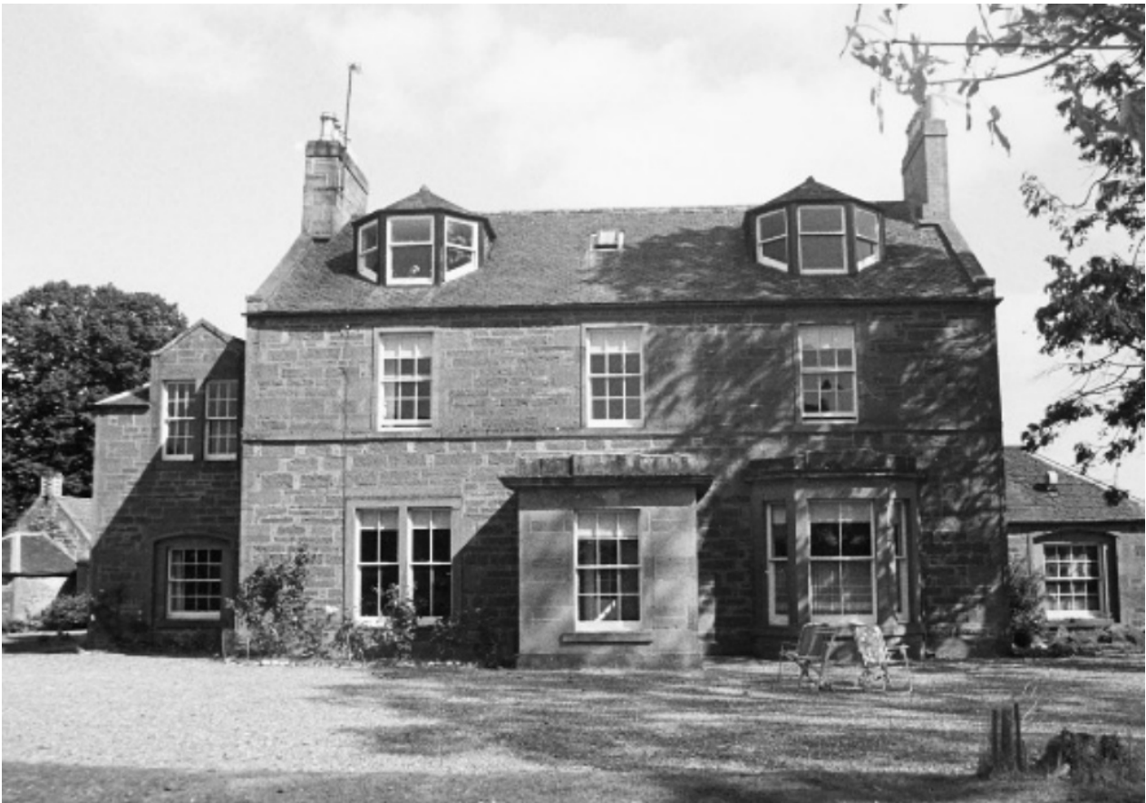
Figure 065: Waterside House and Manse of Stracathro, Angus.
