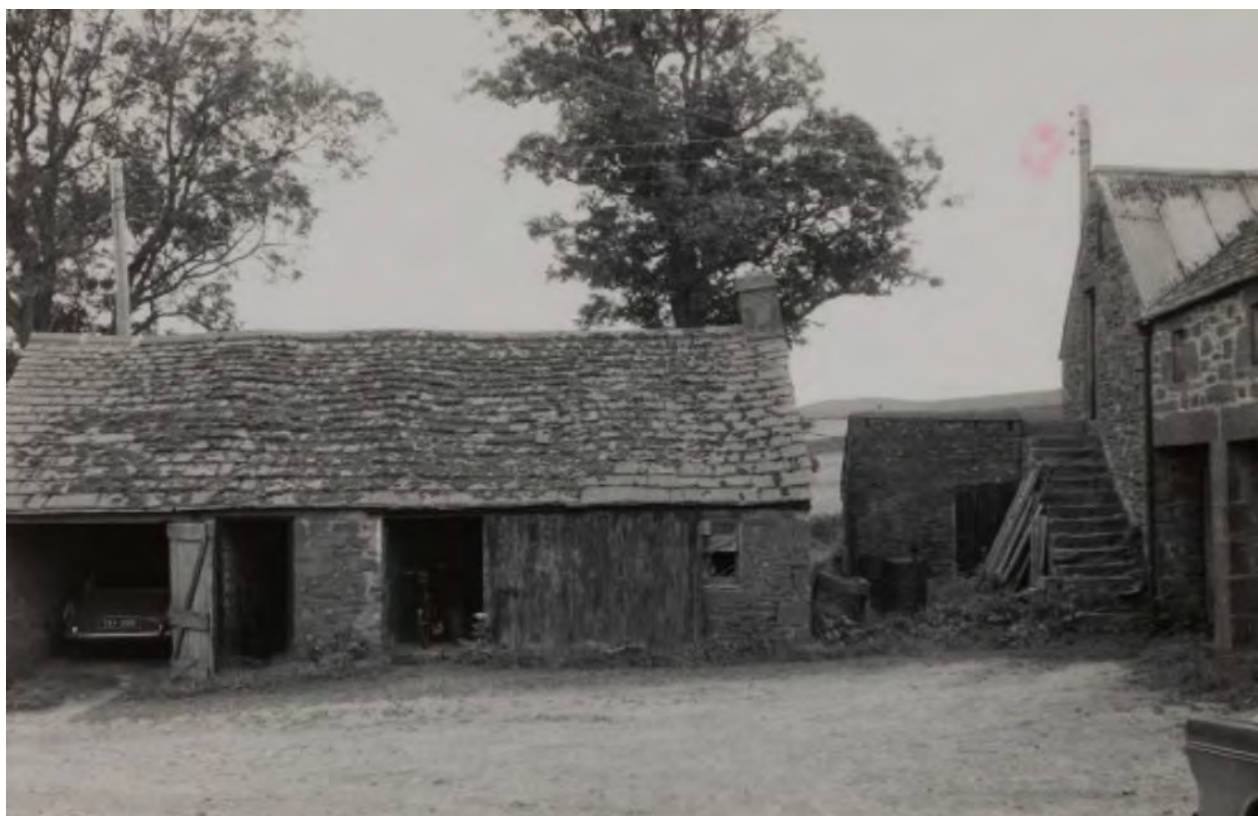
Figure 141: Nether Middleton Farm, Glenogilvie, Angus. This roof is believed to have been lost.
