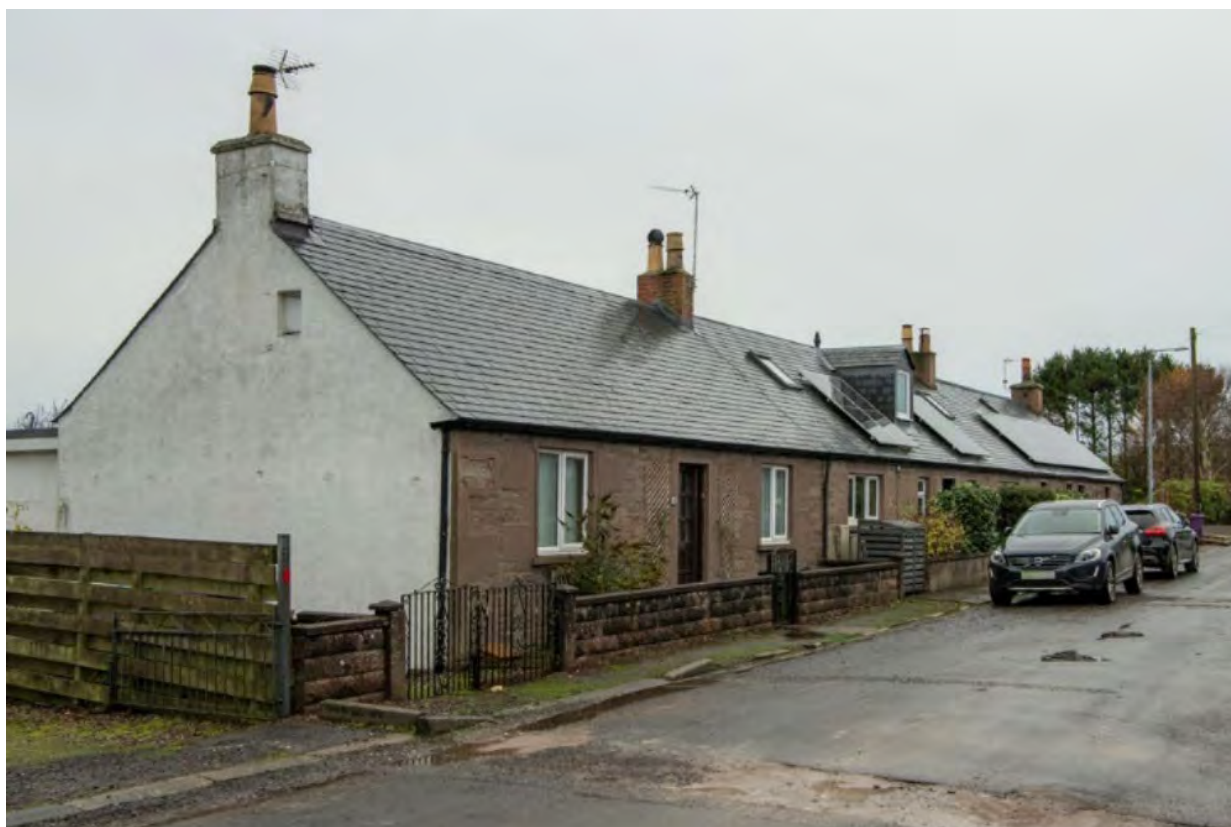
Figure 151: Terraced cottages, Watson Street, Letham, Angus. The flagstone roof has been lost.
