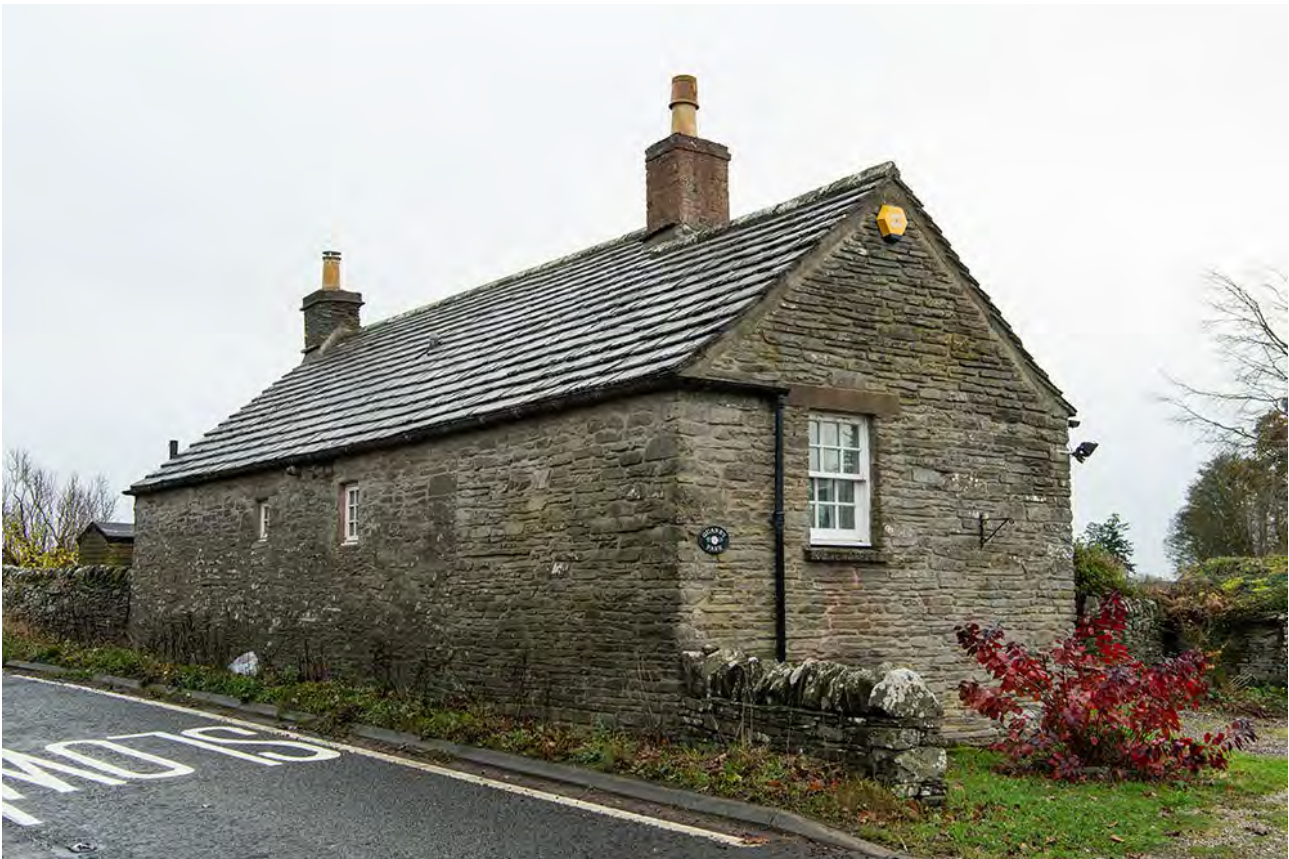
Figure 061: Quarry Park Cottage, Balgavies, Angus.
