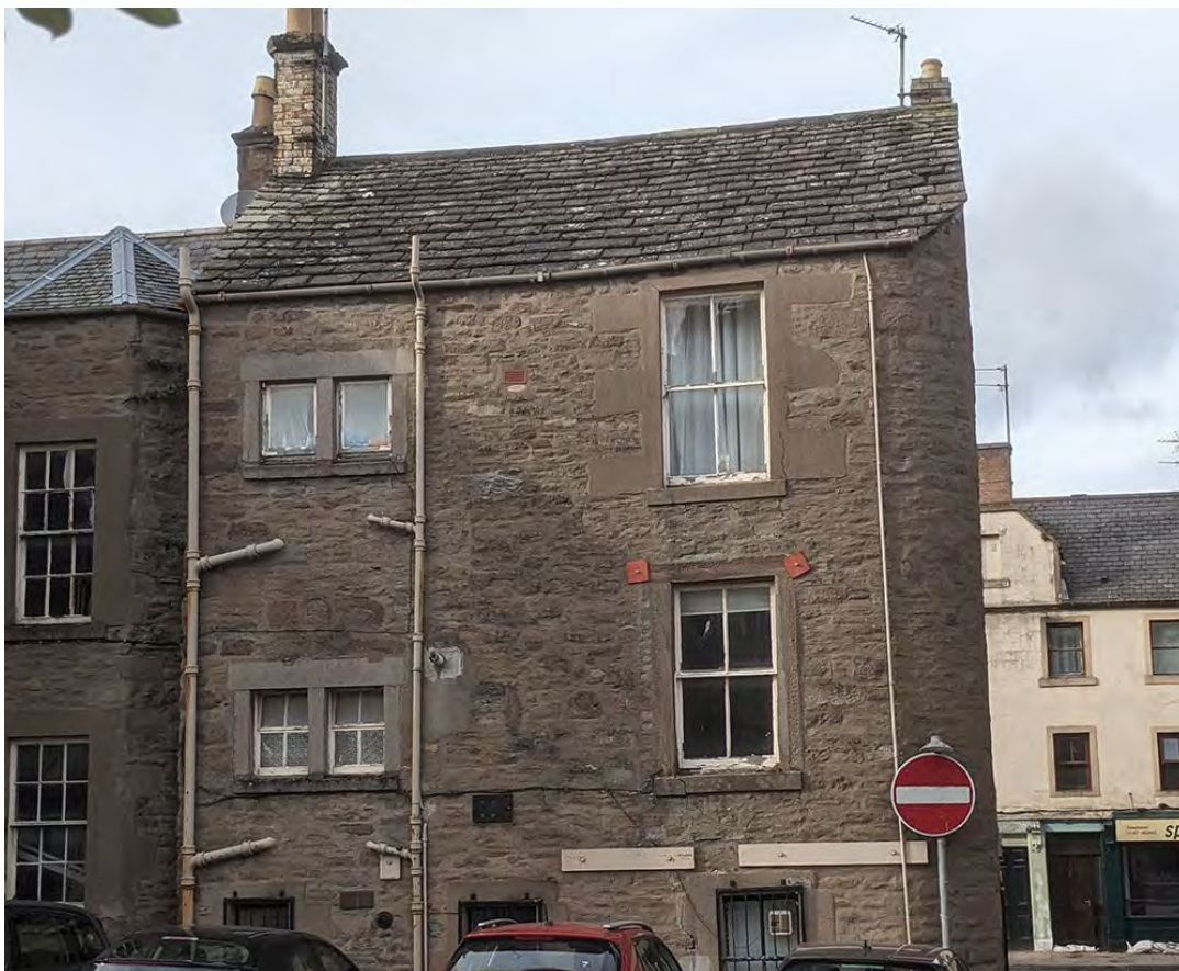
Figure 109: This is a double depth tenement between West High Street and Little Causeway, Forfar, Angus. The rear tenement is roofed in flagstone. © Sara Carruthers.
