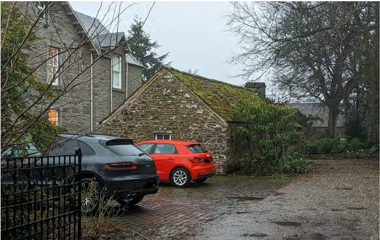
Figure 056: Flagstone-roofed outbuilding adjacent to Old Manse, Kirkton of Auchterhouse, Angus. © Sara Carruthers.
