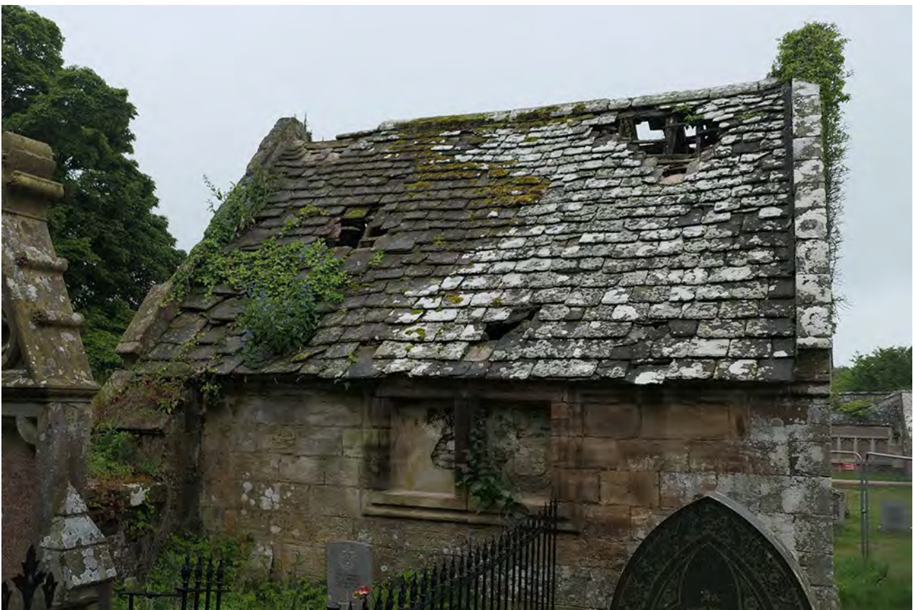
Figure 215: Monimail morthouse, also known as Melville Aisle, Fife. © Arc Architects.
