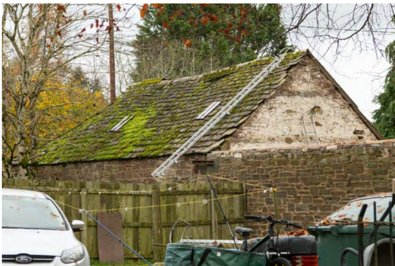
Figure 127: Outbuilding or steading, Lochhead Farm, Forfar, Angus.
