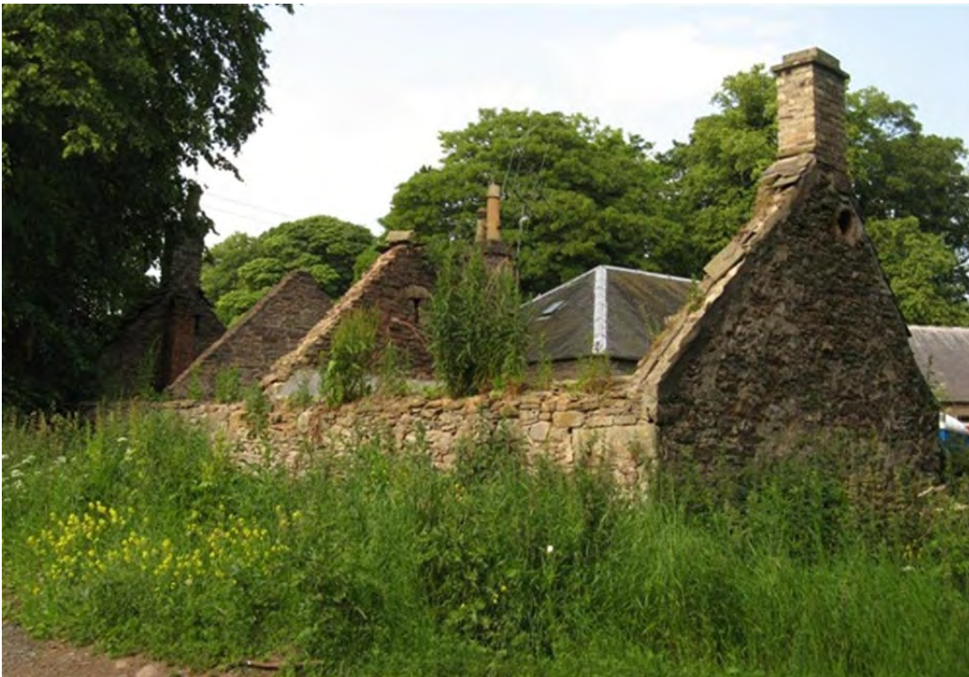
Figure 193: West Cottage, Ballumbie Gardens, Angus.
