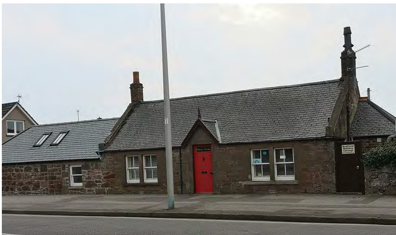
Figure 190: North Esk Road, Montrose, Angus, no longer with a flagstone roof.
