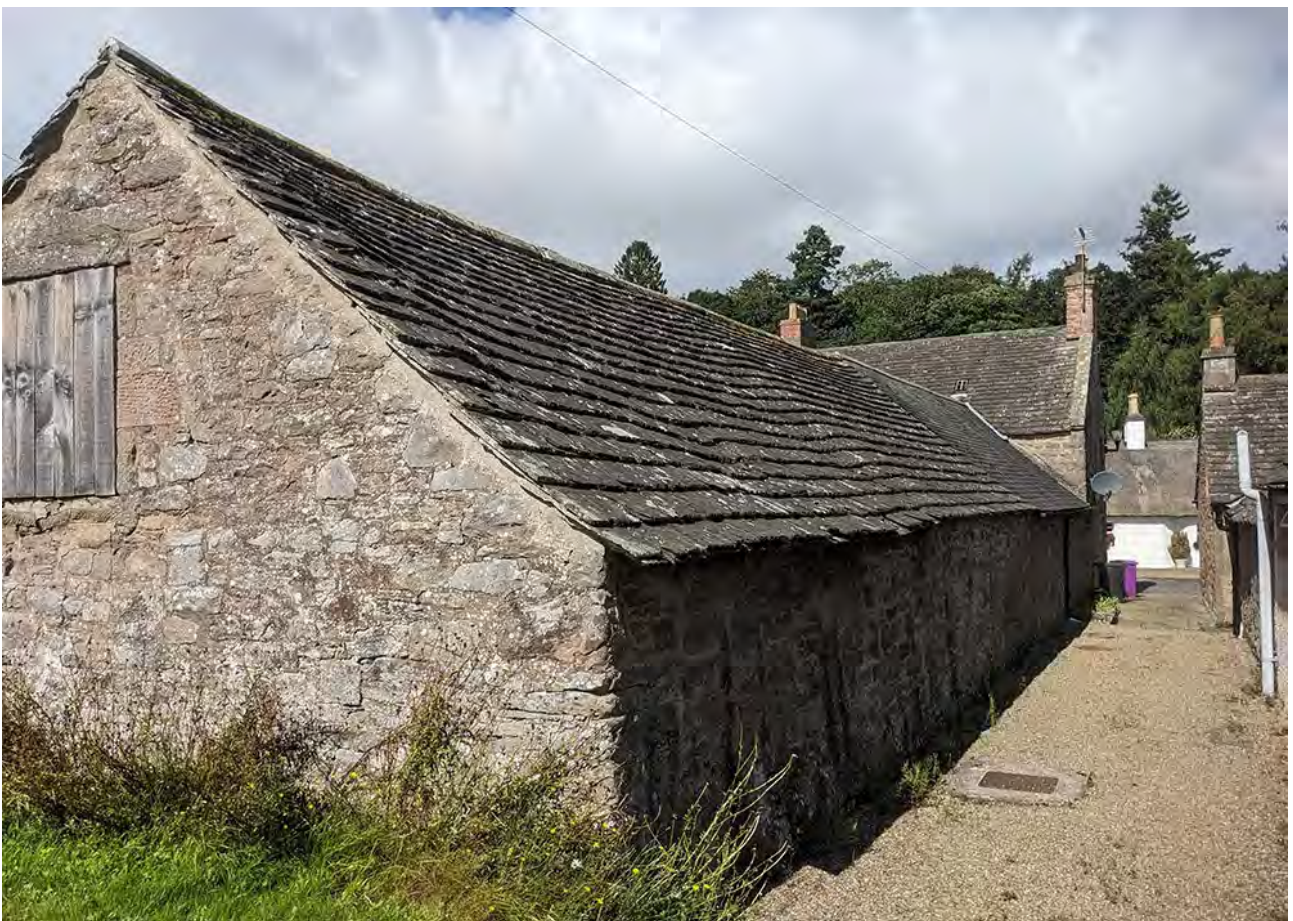
Figure 025: Outbuilding behind Main Street, Glamis, Angus. © Sara Carruthers.
