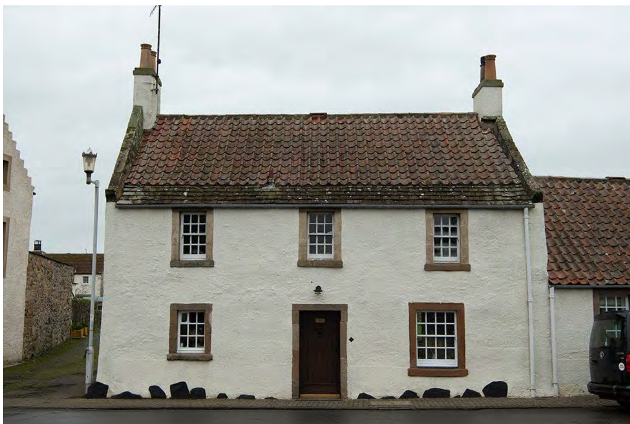
Figure 213: Main Street, Kilconquhar, Fife. The lower part of the roof is flagstone and the remainder is pantiles.
