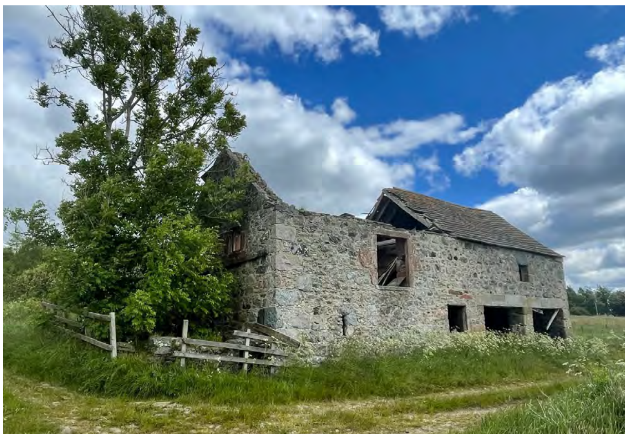
Figure 176: Bogside Steading, Glenmoy, Cortachy, Angus. Shown with half of the flagstone roof remaining. © Douglas Binnie.
