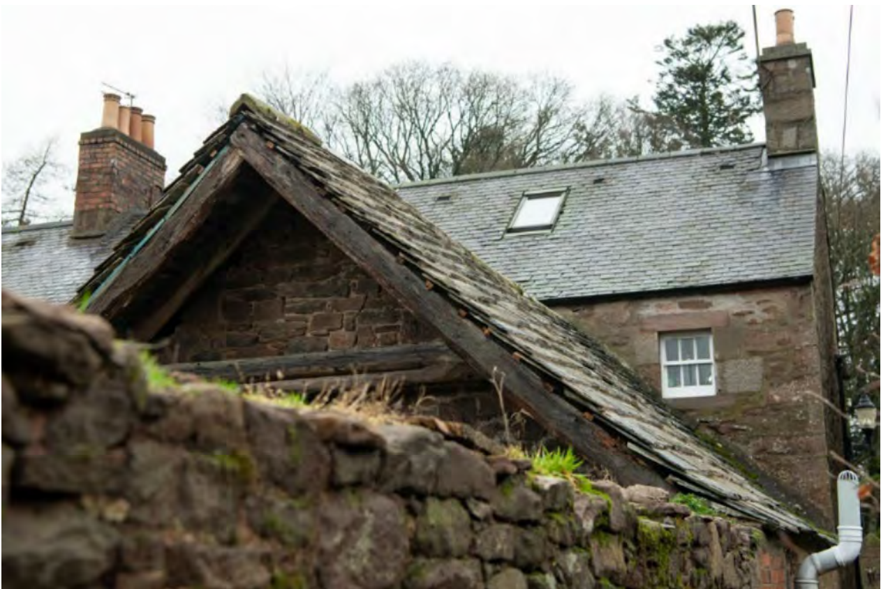
Figure 028: Outbuilding behind Main Street, Glamis, Angus.
