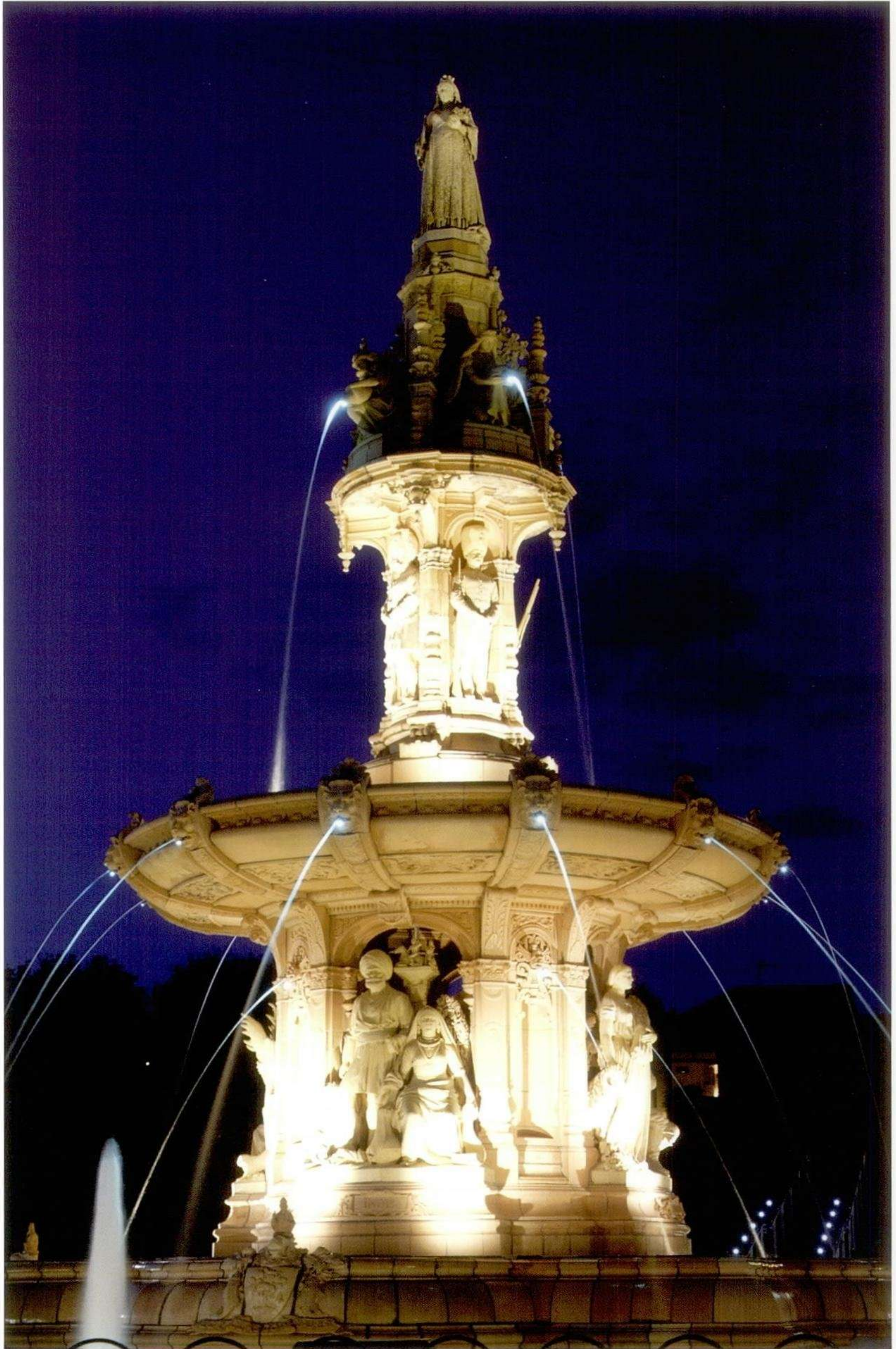
New lighting highlights the details of the ornate terracotta and the water jets, providing a spectacular display.
