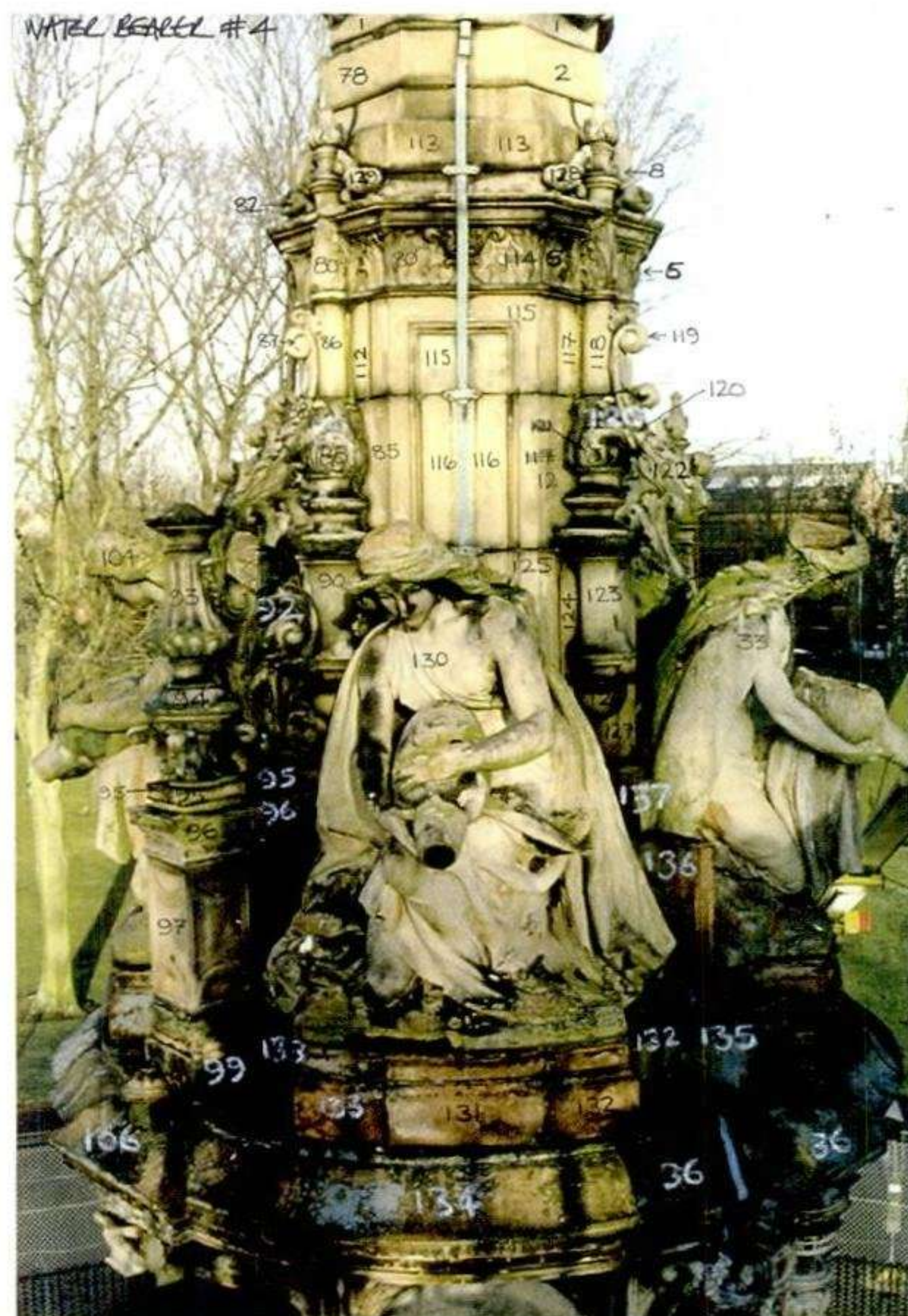
Examples of the individual block numbering system developed by GUARD.
