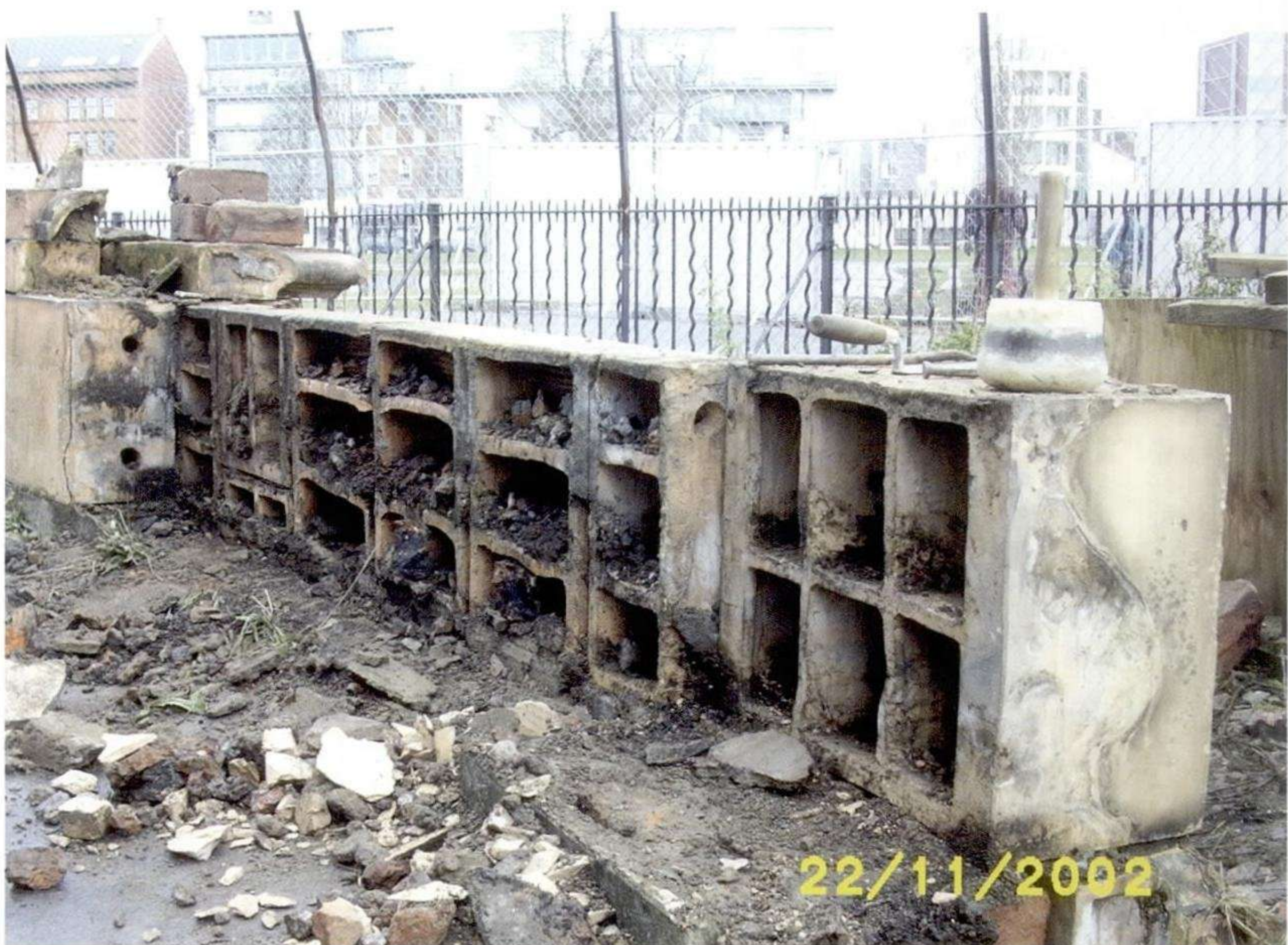
Construction of the outer basin wall.
