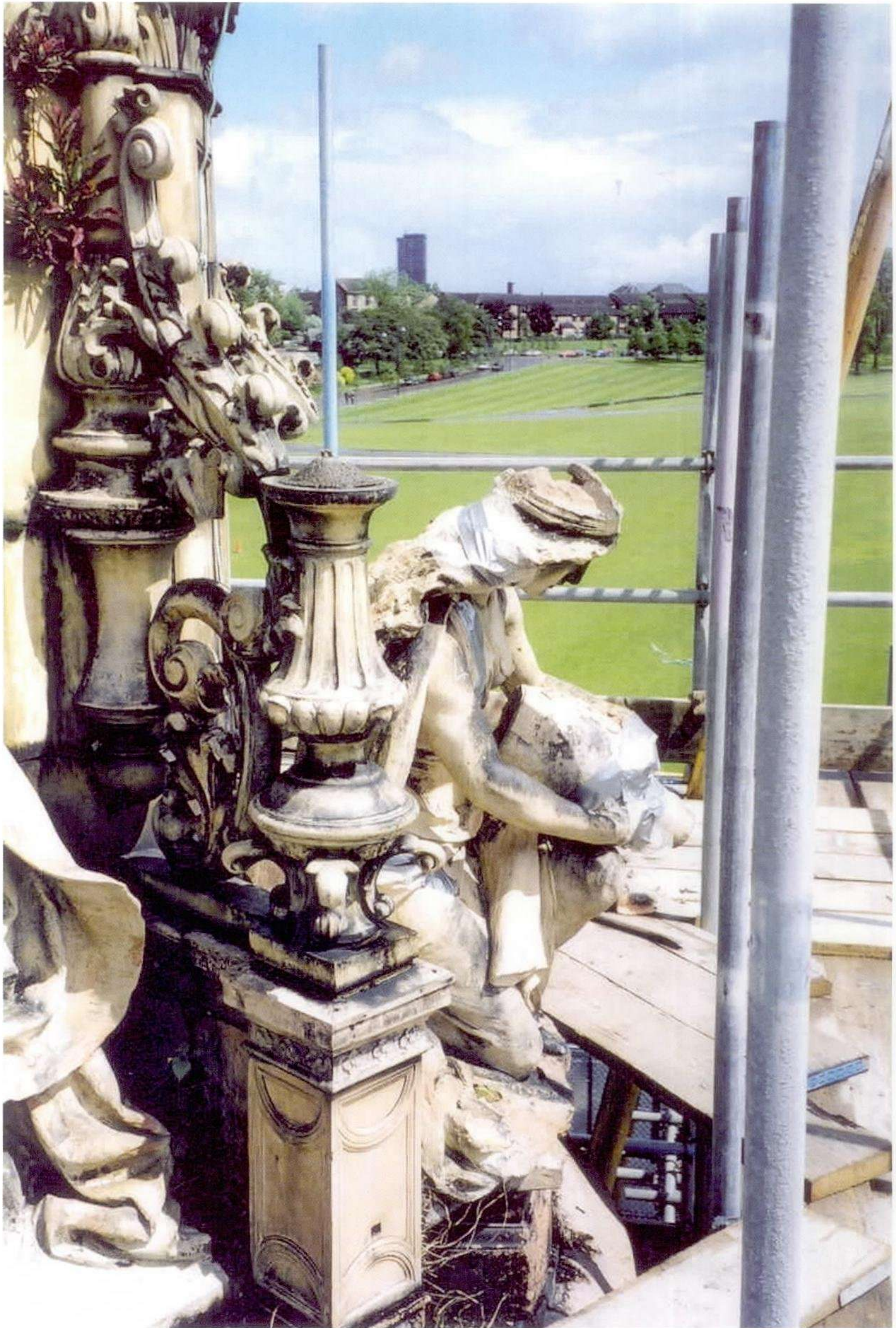
The delicate process of removing the water bearers sculptures began with stabilisation of delicate surfaces.
