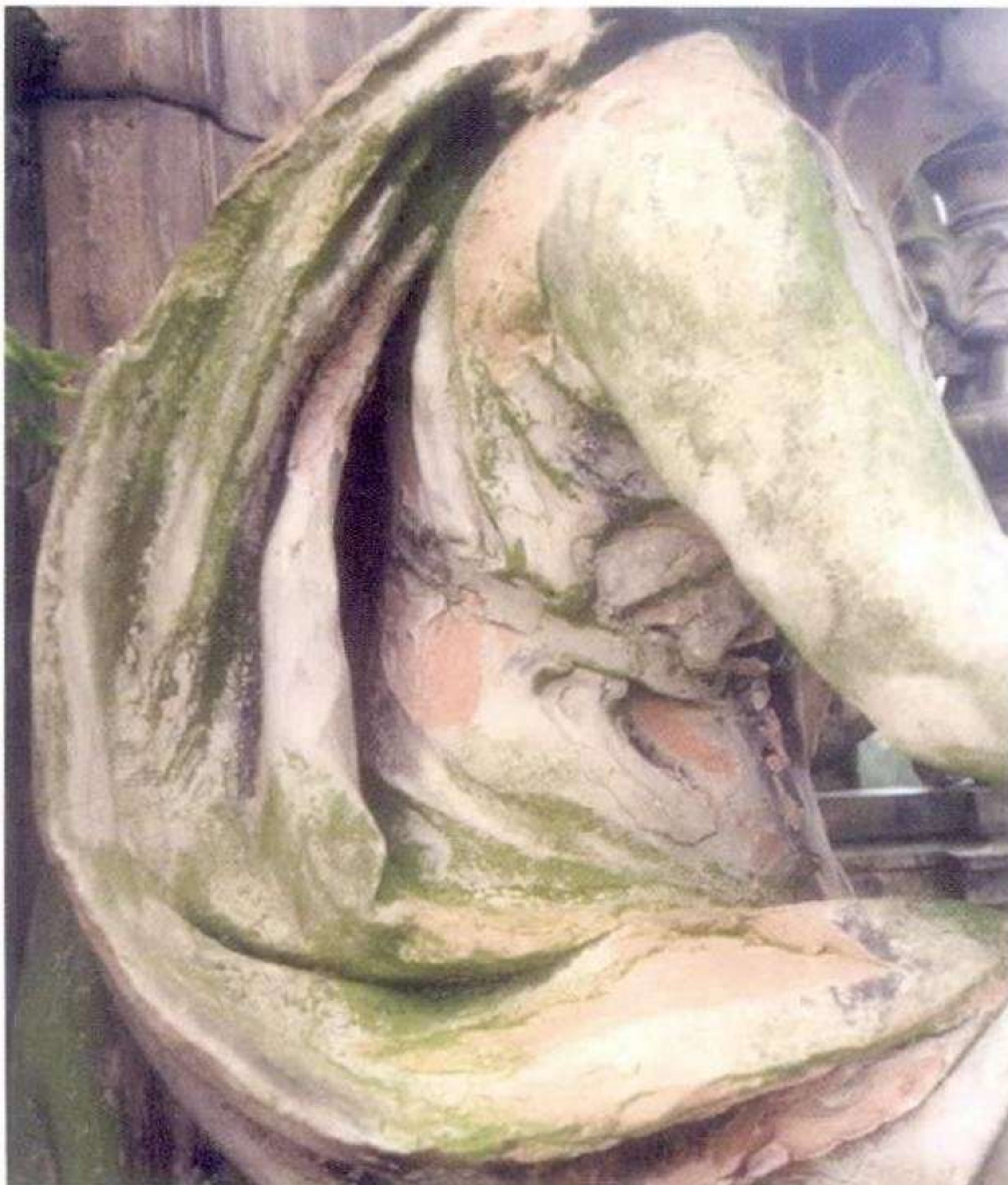
Details of the deteriorated condition of the four Water Bearers. Fracturing, delamination, frost damage and surface granulation were widespread. (All: Nicola Ashurst)
