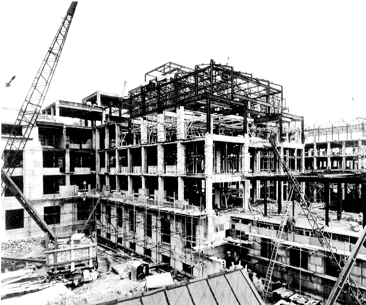
Figure 4. The construction of St Andrews House, Edinburgh. The steel frame, concrete encasement of the steelwork and the addition of stonework can be identified as construction progresses.
