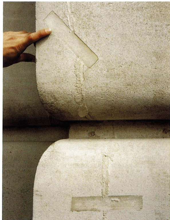
Figure 73. 'Dog cramps' on a Portland stone building.
