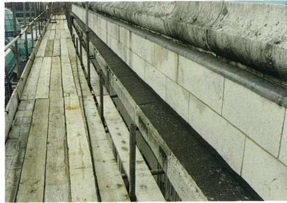
Figure 32. Bituminous waterproofing paint added to a cornice detail.
