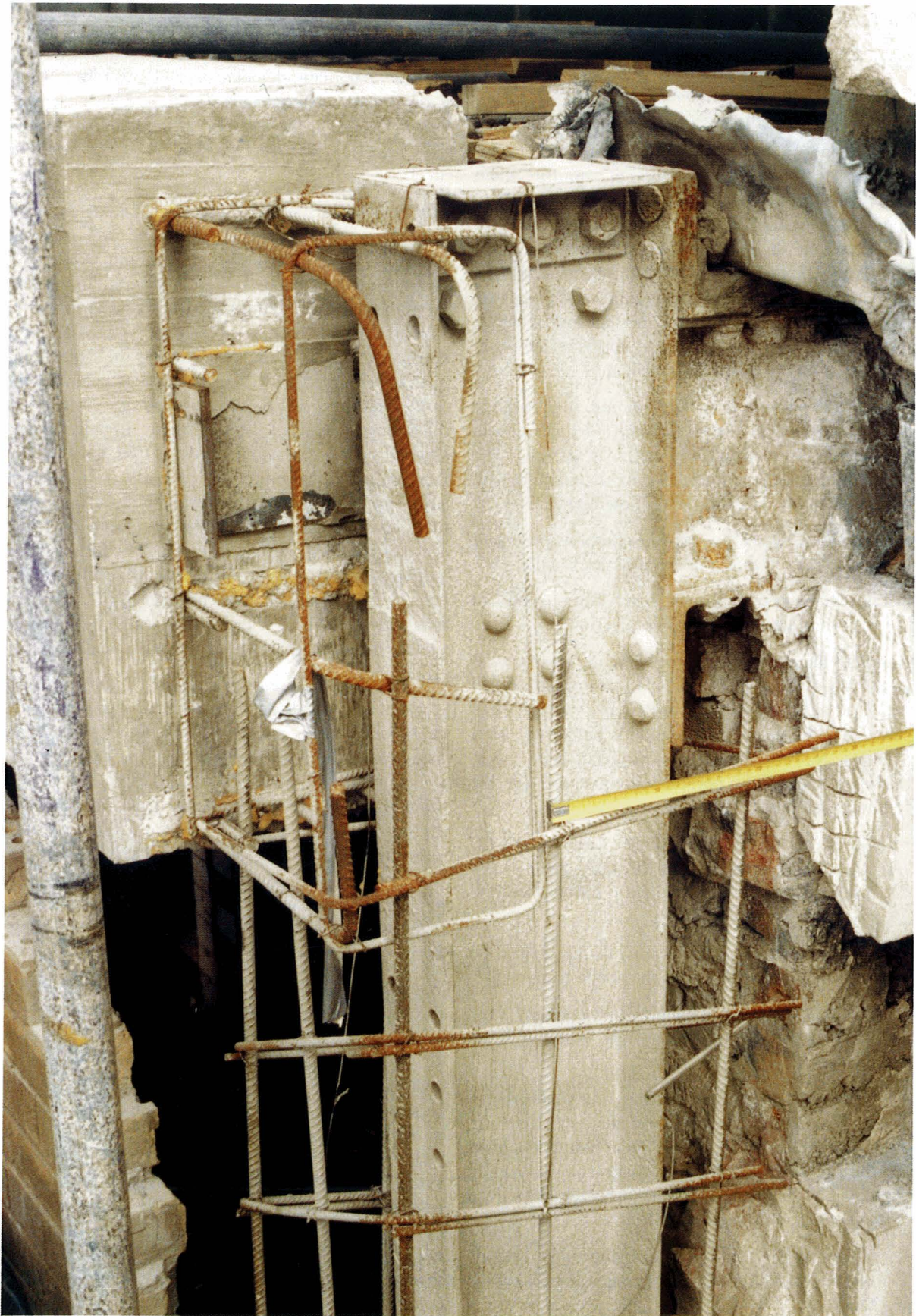
Figure 74. Preparation for the concrete encasement of a steel 'T' section.
