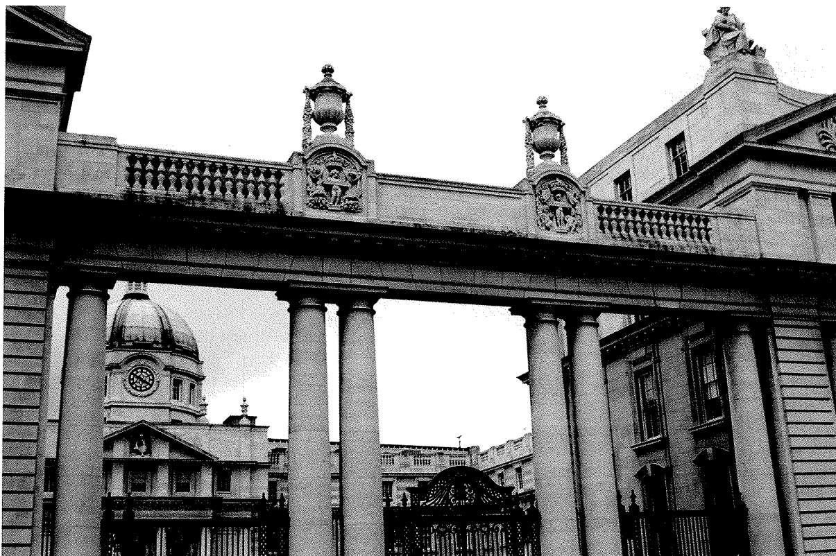
Figure 68. The entrance colonnade to the Royal College of Science, Dublin (1991), the first full scale cathodic protection system for the protection of corroding steel 'I' sections.
