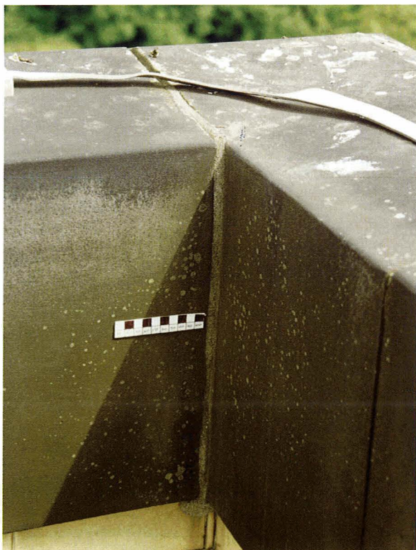
Figure 71. The installation of a precompressed tape sealant to a parapet joint.
