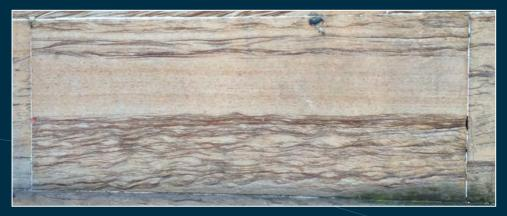
Fig. 1: Visible bedding planes in this sandstone ashlar.
