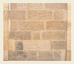
Fig. 6: Ashlar indents cut to fit and tooled to match existing masonry.
