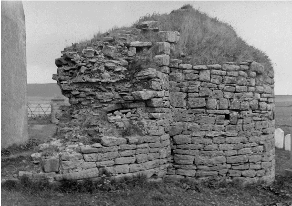
Figure 12: Early photograph showing proximity of the parish church ([left of image] constructed in 1829) to ruins of St Nicholas Church. The building and subsequent demolition of the parish church removed the full arc of the circular nave. © Courtesy of HES.
