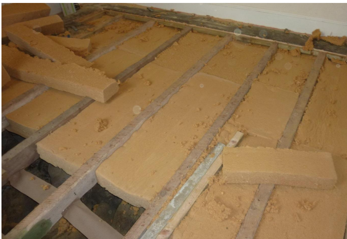
Figure 15: Floor opened up, showing the wood fibre board insulation in place
