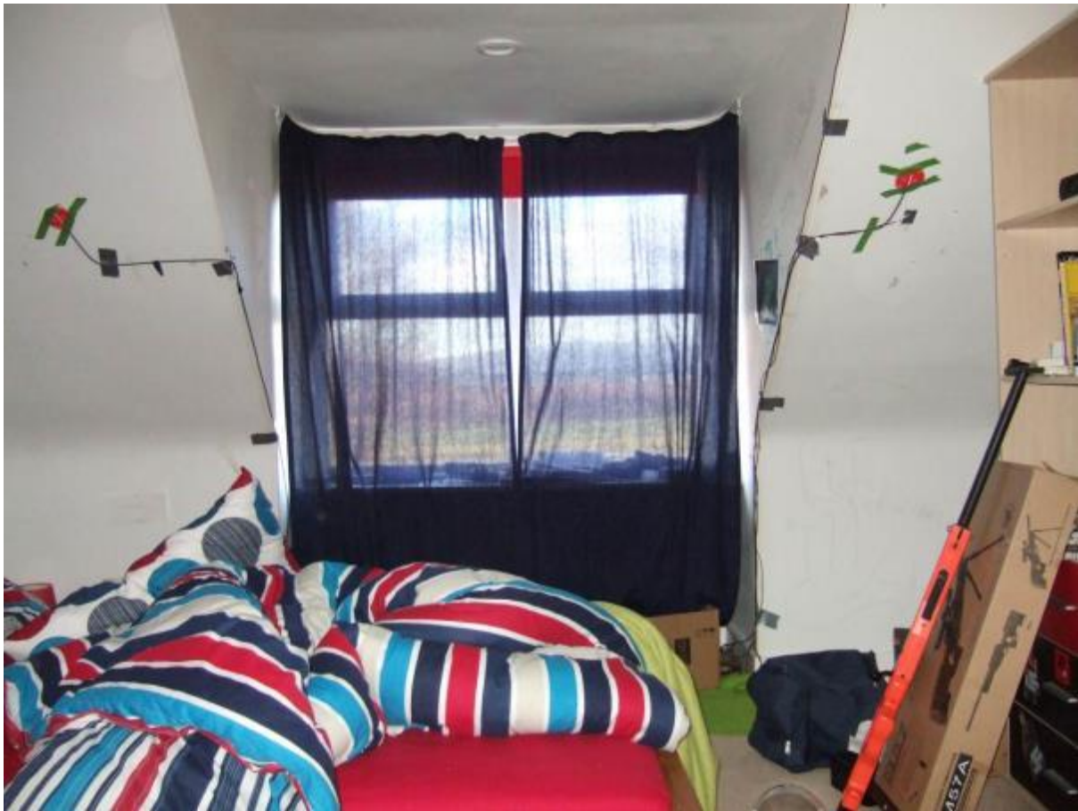
Figure 4: Heatflux plates sited either side of the dormer used to assess heat flow for in situ U-value measurement
