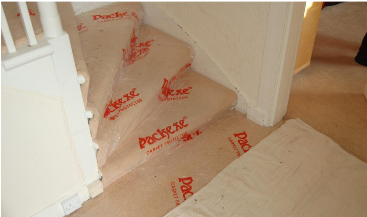
Figure 6: Protection of carpets during the works
