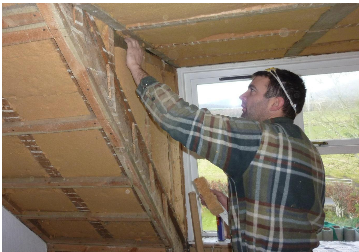
Figure 9: Fitting wood fibre insulation to the dormers
