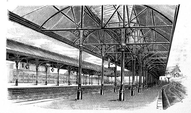
No. 2401.—The above illustration, which is from a photograph, shows part of a large extent of Iron Roofing over Passenger Platforms recently erected by us at New Bridge Street Station, Newcastle-on-Tyne. The different Spans are of the Curved type, with large Ventilator of strong glass along top of each, to afford the necessary lighting and ventilation.
