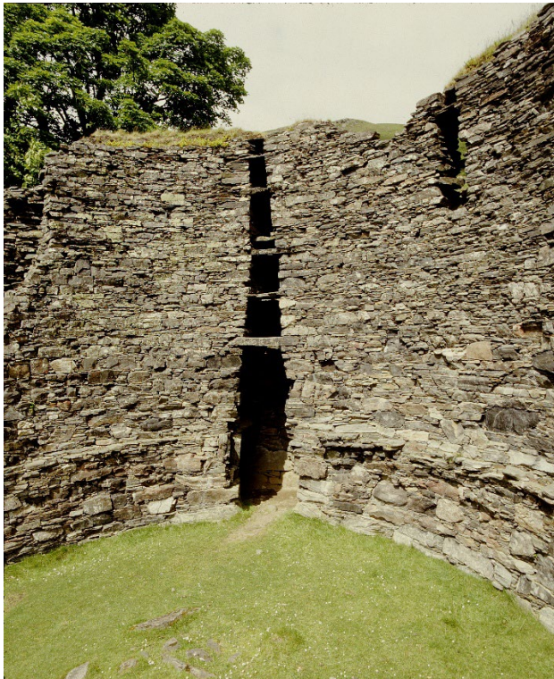
Figure 12: Interior, showing scarcement. 008-001-000-083-R © Crown Copyright: HES
