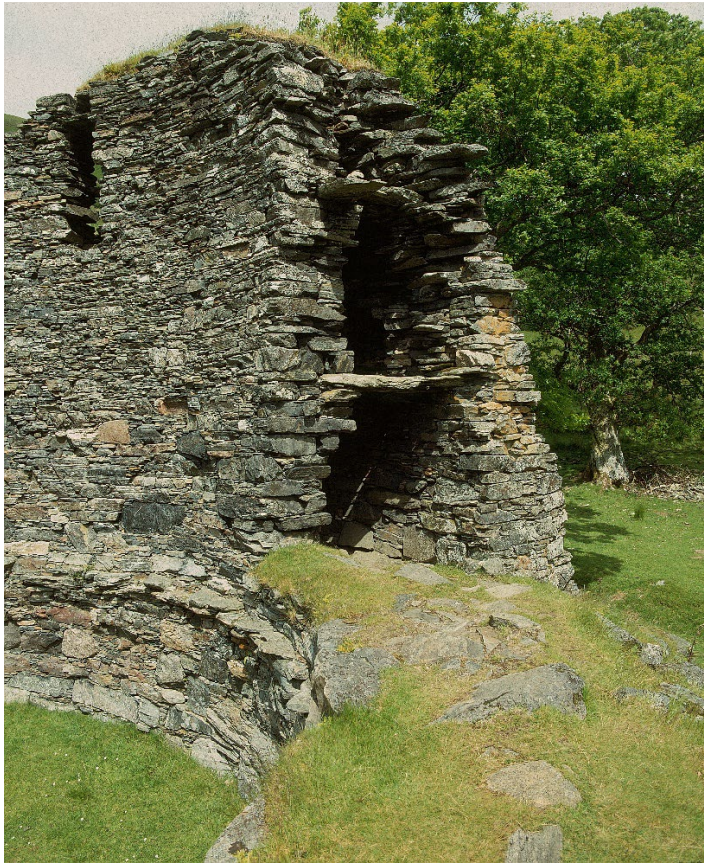
Figure 13: Eastern end of high-surviving wall, showing gallery levels. 008-001-000-081-R © Crown Copyright: HES
