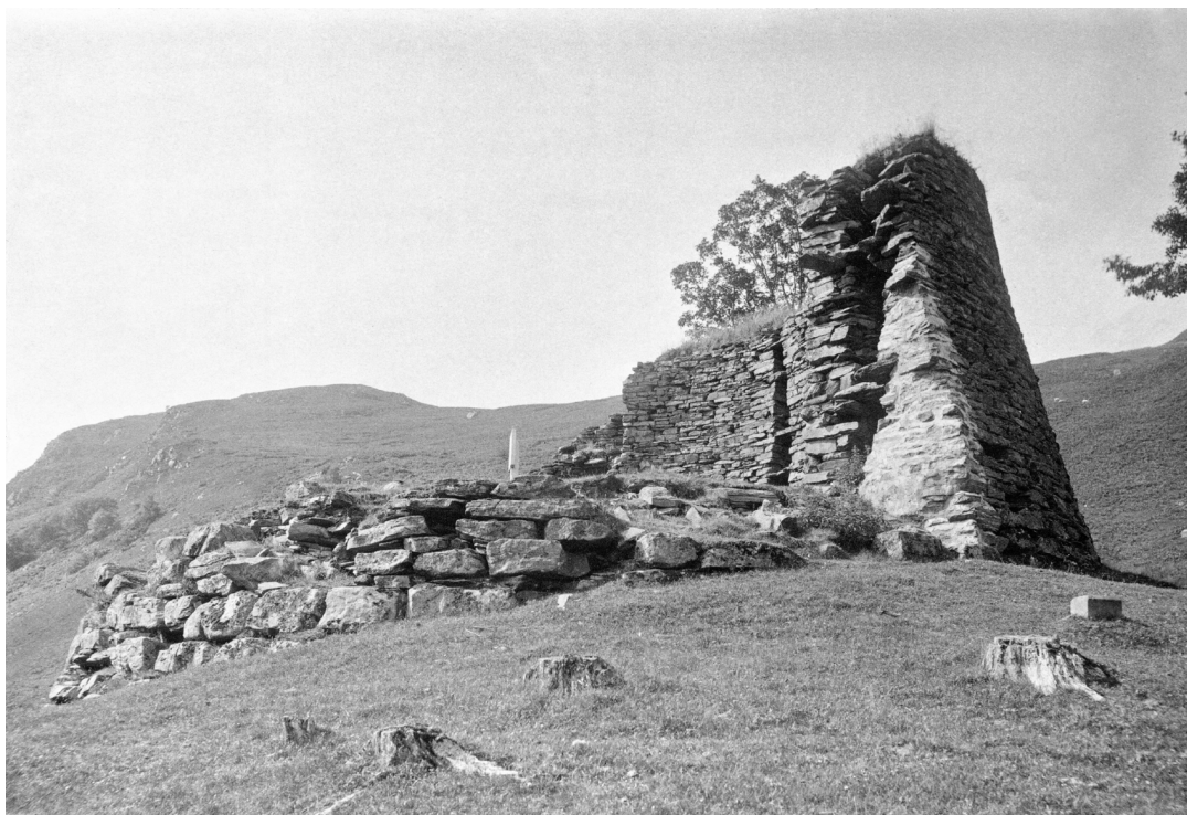
Figure 6: 1897 photograph by Erskine Beveridge – with early cement repairs clearly visible on right. SC 1142521 © Crown Copyright: HES
