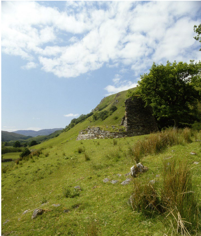
Figure 10: Distant view showing position on hillside ledge. 008-001-000-085-R
