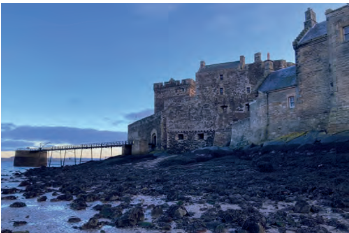
Figure 2.2.14 Blackness Castle from Blackness Bay showing the nineteenth-century pier and Officers Quarters.
