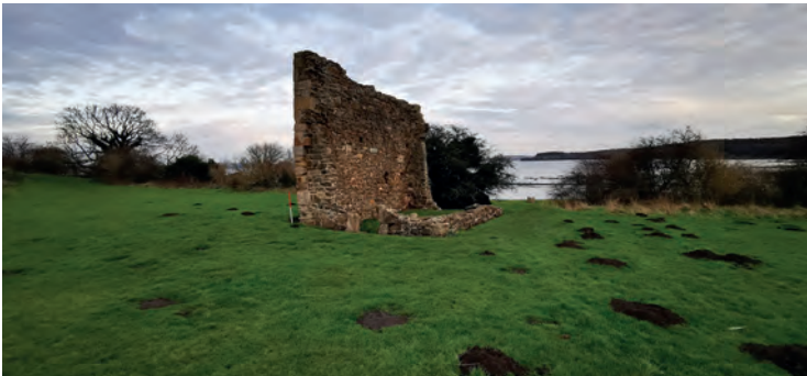
Figure 2.2.10 The ruinous dovecote (OA21) facing east.
