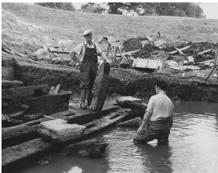
Centuries of immersion in water have preserved the footings of a timber bridge.
