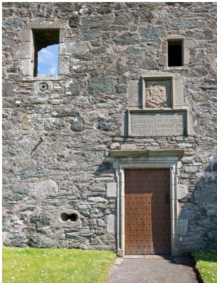
Figure 4: View of lugged architrave doorway, with carved panels above. © Crown Copyright HES.
