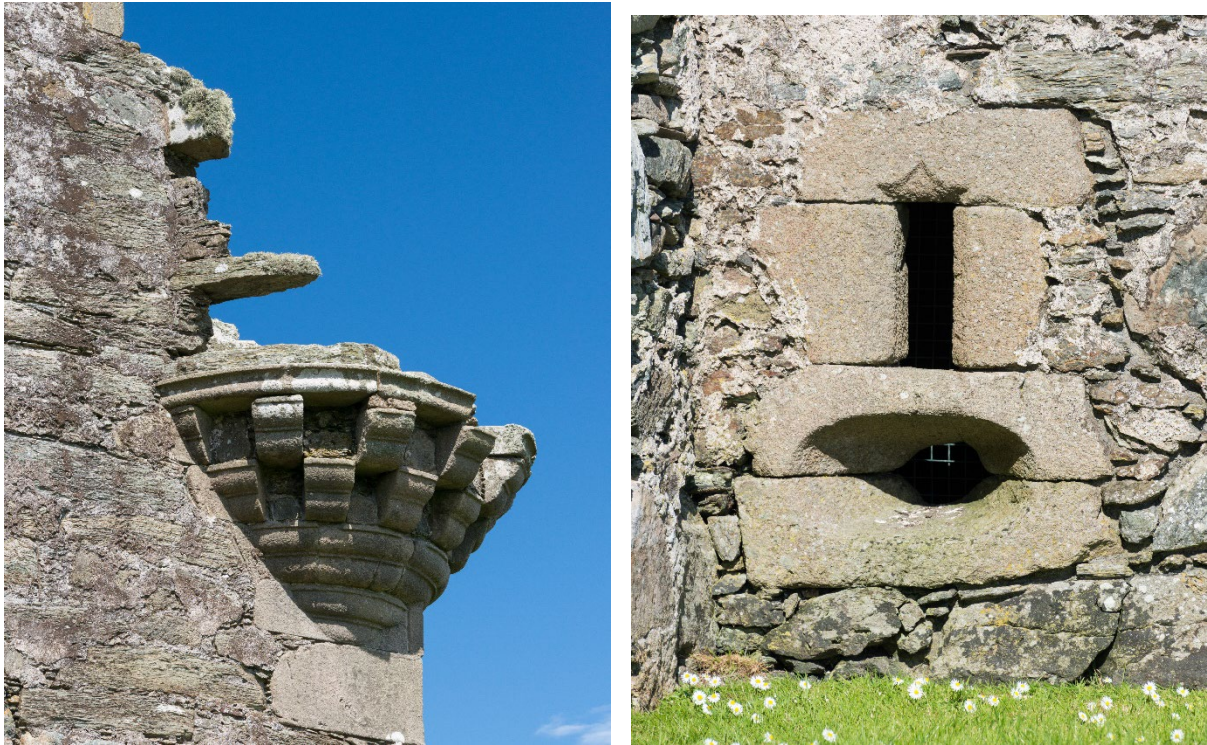
Figure 5 (left): Detail of corbelled turret. Figure 6 (right): Detail of narrow window with incised arc detail on its lintel, and gunloop below. Both images © Crown Copyright HES.
