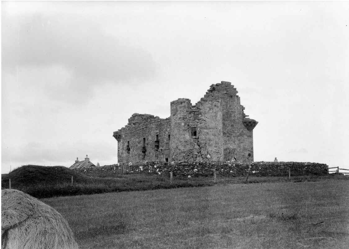
Figure 12: Muness Castle in c.1930, prior to the consolidation works which followed the site entering State care in 1956. The mound to the south of the castle is visible behind the haystack, in the bottom left-hand corner of the image © Crown copyright: HES.
