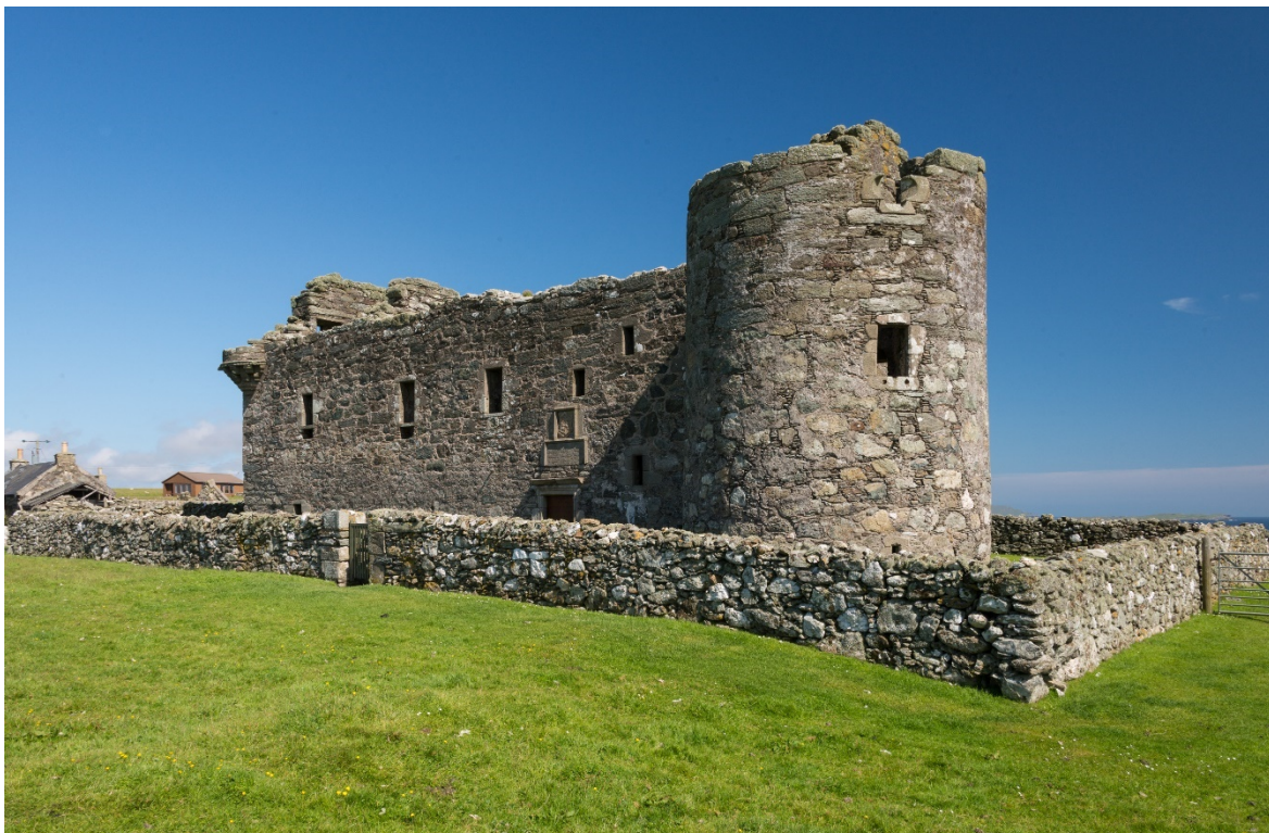
Figure 2: View of Munness Castle from the south. © Crown Copyright HES.
