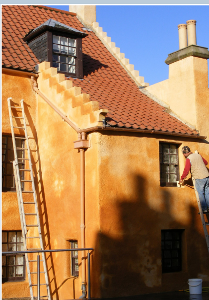
Harling being carried out at Dymock's, Bo'ness. © N. Haynes.
