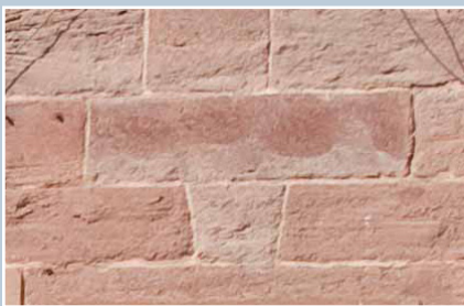
High Street, Arbroath. Rich pink-red sandstone, typical of parts of Angus. Here the stone is laid in regular courses. © N. Haynes.
