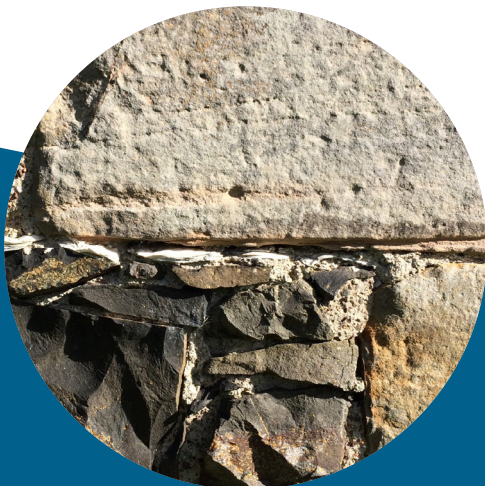
Oyster shell pinnings in mortar joints - Elcho Castle, Perthshire.
