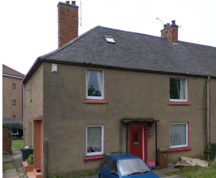
Figure 2.3. CS3 from the South East. (Image: Google Streetview.)
