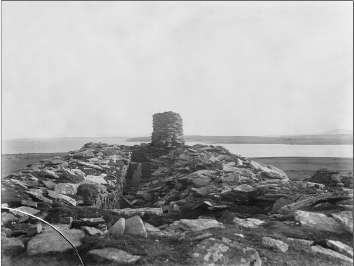
Fig. 03: The exterior of the tomb in 1929. Original image © Historic Environment Scotland (reference SC01219141) and reproduced with kind permission. The drystone rubble stack is a naval navigation marker cairn which was built in the 19 th or early 20 th century.
