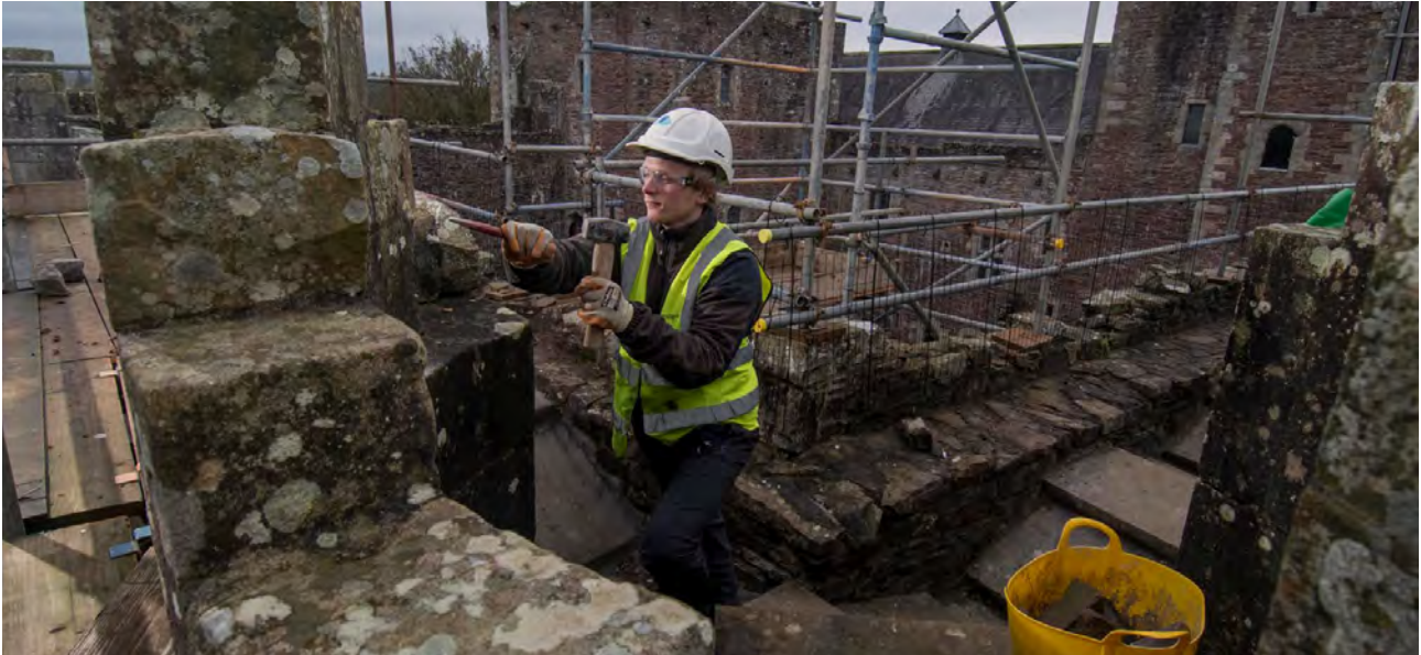
Figure 10: A stonemason working at Doune Castle. © Donald MacLeod
