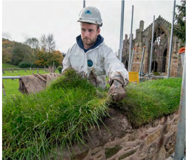
Figure 14: Installing a soft capping at Melrose Abbey. Soft capping can have biodiversity benefits. © Donald MacLeod
