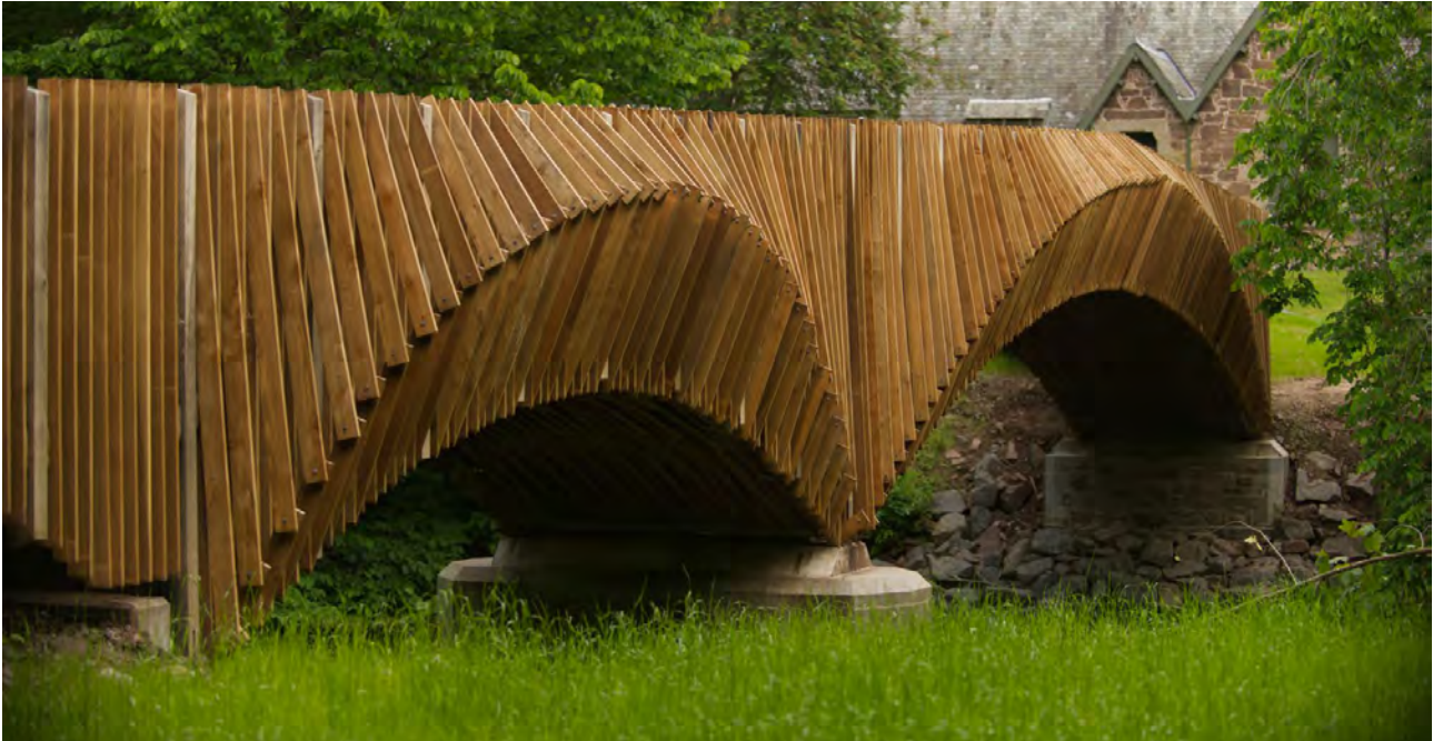
Figure 66: At Doune, larch was used to create a new bridge connection between the castle and town. Laminating the timber meant that smaller, lower-grade pieces could be used, providing more flexibility and opportunity to source the timber locally. © Rob McDougall
