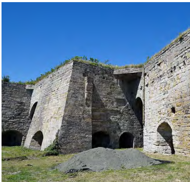
Figure 33: Lime kilns like these examples at Charlestown, Fife, used to operate across Scotland. However, lime has not been commercially manufactured in Scotland since the early 1960s. © Greg MacVean
