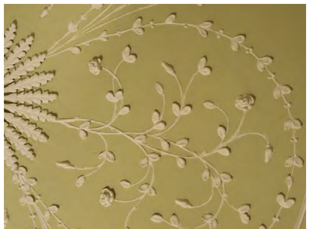
Figure 29: Plasterwork ceiling of the Drawing Room at Bute House, Edinburgh. Lime is used internally and externally in a variety of contexts, from fine plasterwork to mortar, harl and limewash.
