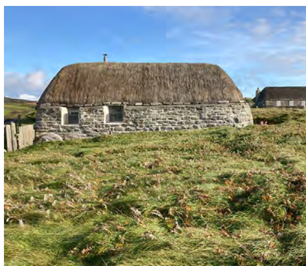
Figure 54: Distinct regional styles of thatching use local materials to suit climatic and geographic conditions. In the Western Isles, marram-thatched roofs with a distinctive rounded shape developed to cope with strong winds. © Sanne Roberts
