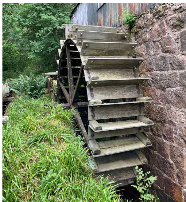
Figure 64: Durable hardwood timbers like oak and elm were used to construct waterwheels, such as this example at Birse Mill. © Graham Briggs
