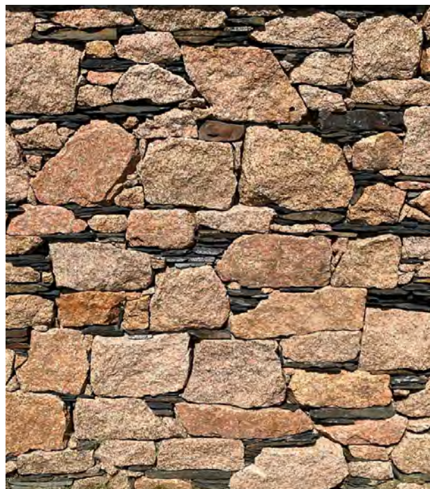
Figure 51: A small historic quarry was able to supply local Ross of Mull Granite for the construction of Iona Village Hall. Opportunities like this, where smaller, historic ‘snatch’ quarries can provide locally distinctive materials, are often overlooked, yet they offer significant cultural and sustainability benefits. © Graham Briggs
