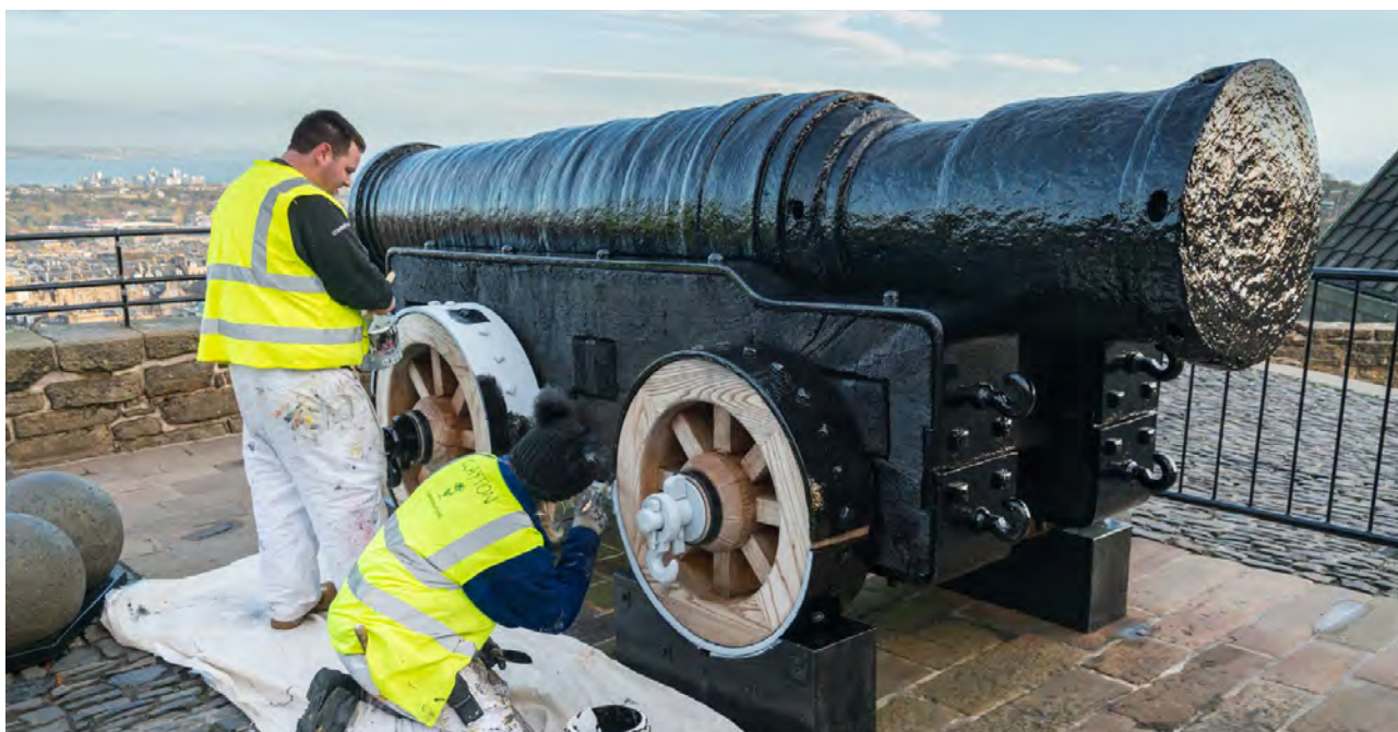
Figure 43: Mons Meg being painted at Edinburgh Castle. Selecting and specifying appropriate paint coatings is an important part of repainting programmes.
