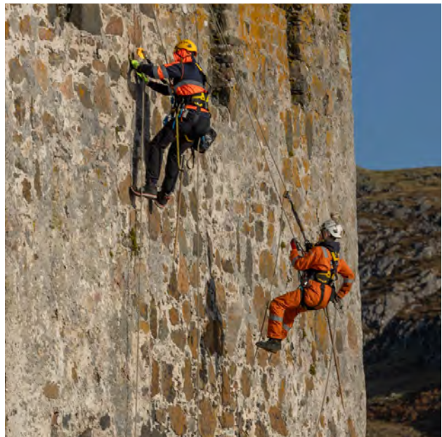
Figure 7: Robust survey and data analysis lie at the heart of informed decision-making. This rope survey team is working on Kisimul Castle, Isle of Barra. © Sandie Photos
