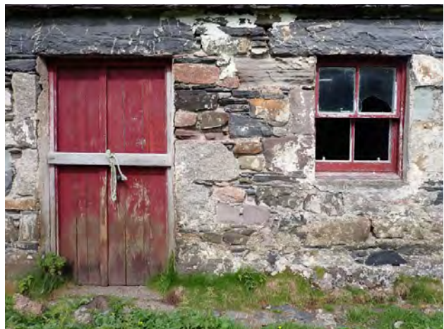
Figure 30: A house on Lismore, Inner Hebrides. Evidence often survives of historic lime surface finishes. © Sanne Roberts
