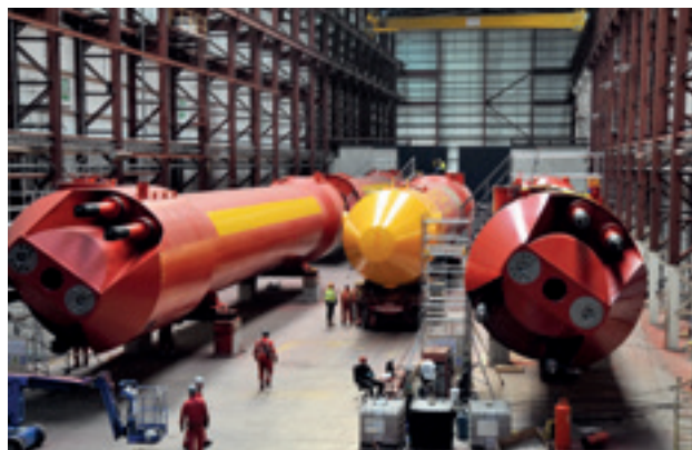
A Pelamis wave device under construction in Scotland, indicating the scale of engineering involved. Image © Pelamis Wave Power.
