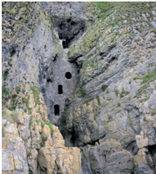
Culver Hole is a remarkable example of the use of coastal resources in the past: the medieval dovecot is built into the entrance of a coastal cave in Wales, and is a Scheduled Monument. Image © Copyright GGAT.
