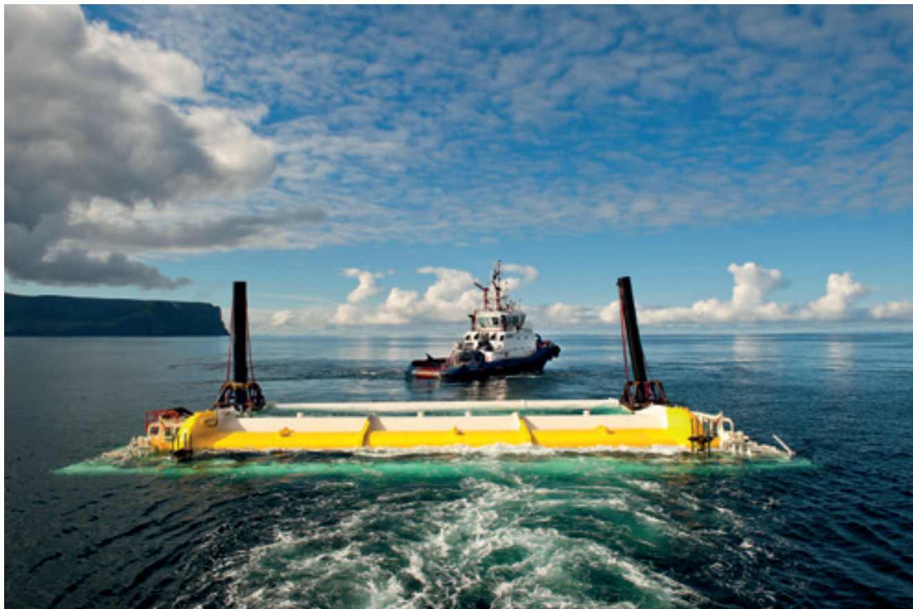
Oyster 800 being towed into position: a wave device built onto the seabed but with major elements that operate at the surface. Image © Aquamarine Power.
