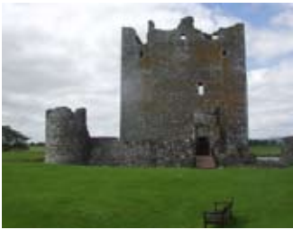
The tower house and artillery tower
