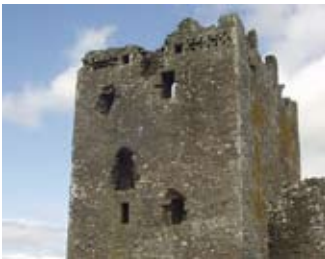
Top of tower showing holes for timber platform
