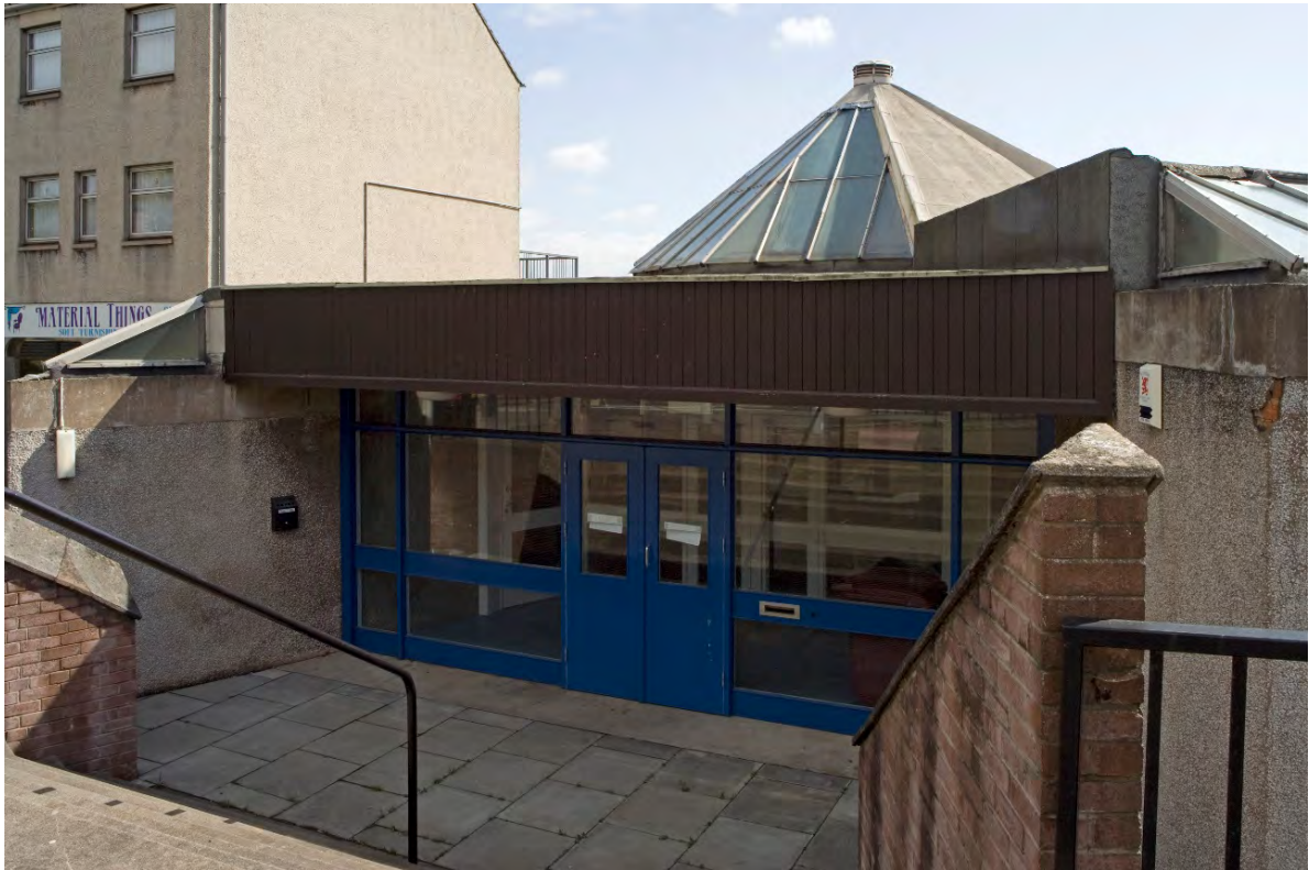
Figure 21: Inverkeithing Library (1969-1971), designed by Frank Mears and Partners © HES
