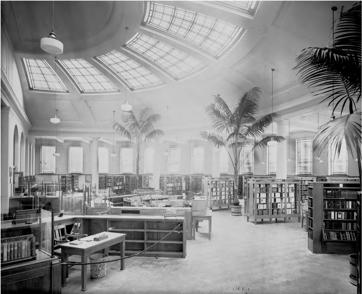
Figure 58: Open-access lending in former reading room at Leith Public Library © HES
