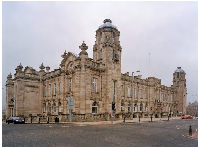
Figure 30: Hamilton Library, Cadzow Street, Hamilton, Glasgow (construction began 1906-07), designed by Alexander Cullen of Cullen, Lochhead & Brown © HES
