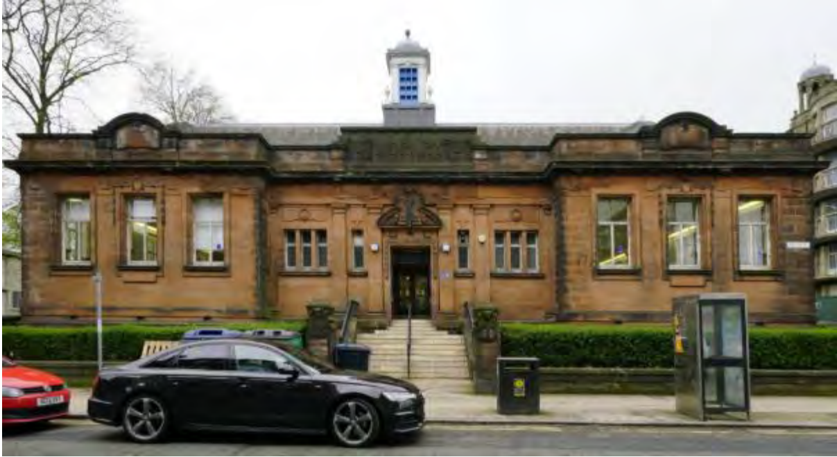
Figure 57: Langside Library, Glasgow (1913-15), designed by George Simpson © Oriel Prizeman
