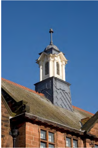
Figure 43: Detail of turret on Montrose Library © HES
