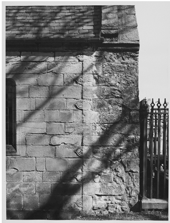
Figure 5: Detail of buckle quoins © Crown Copyright: HES.
