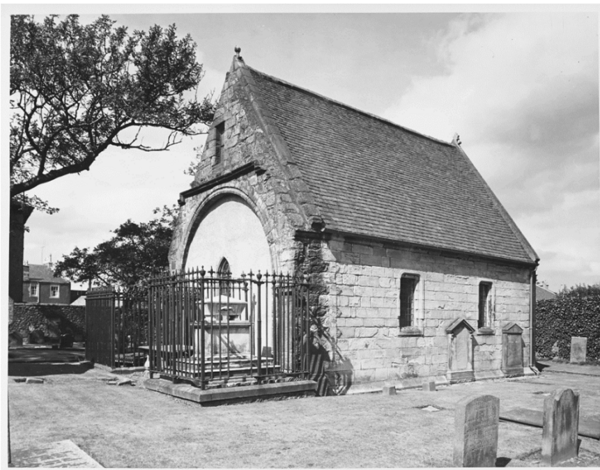
Figure 8: Arch on south side of Aisle, which previously opened to the former parish church, prior to its demolition in 1812 © Crown Copyright: HES.
