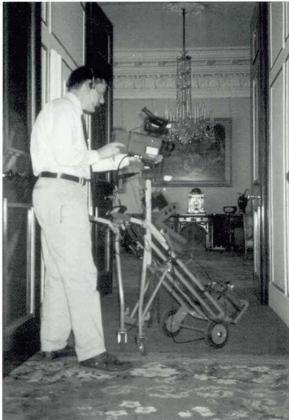
Plate 5 Thermographic inspection in progress. Hand held camera is panned across the wall and the results viewed as an image on the trolley mounted processor. Power is supplied as an unspillable (gel type) 12V car battery.
