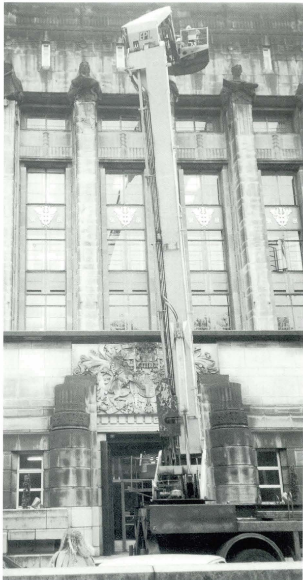
Plate 11 Photograph of survey being carried out from hydraulic hoist
