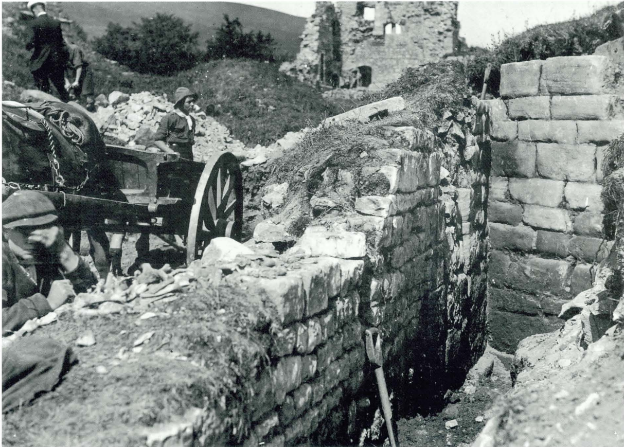
Plate 13 Repair works at Kildrummy Castle in the early twentieth century.
