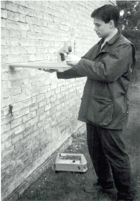
Plate 7 FEMR methods being used to trace an iron drain pipe behind a wall
