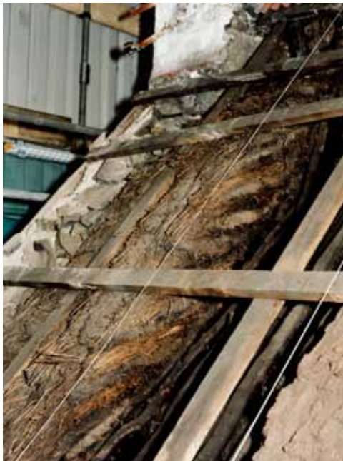
Illus. 31 An excavated section through the thatch (Historic Scotland)
