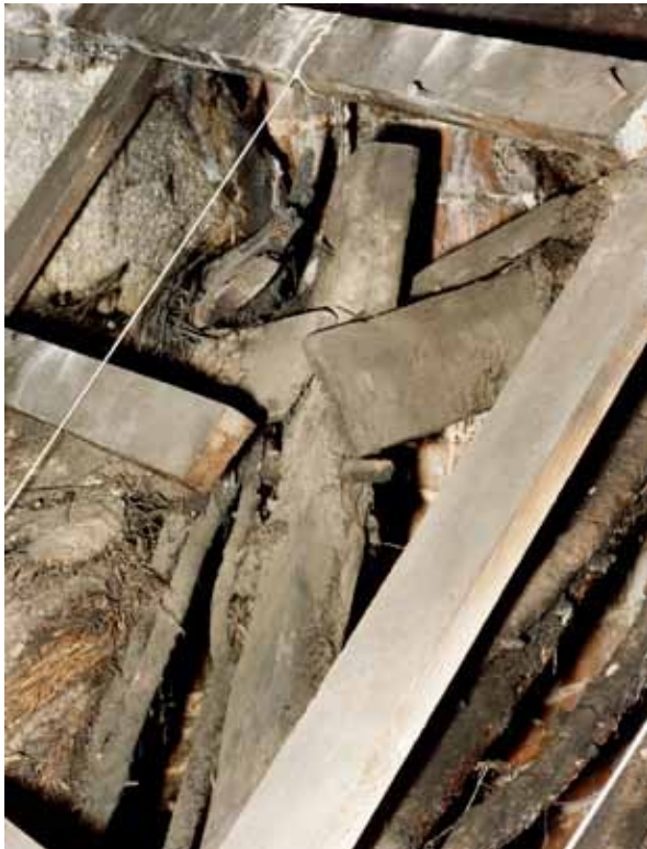
Illus. 60 Timbers of the canopy chimney taken through the excavated section of the thatched roof (Historic Scotland)
