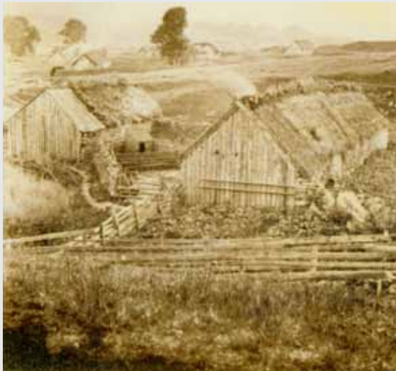
Illus. 54 Timber extension (Atholl estate archives)
