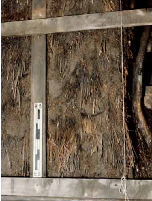
Illus. 31 An excavated section through the thatch (Historic Scotland)
