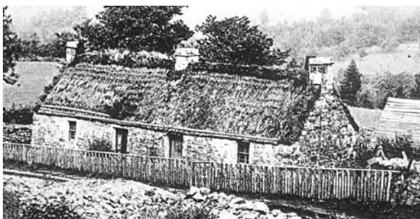
Illus. 62 A cottage in Moulin with a canopy chimney supported against a false masonry stack – this is very similar in form to Sunnybrae Cottage (BW from a GWW postcard)
