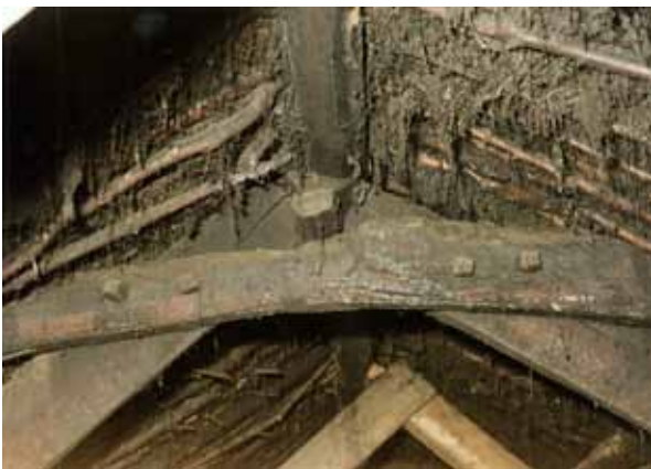
Illus. 16 The apex of the W face of the W cuppill showing the pegging (Historic Scotland)
