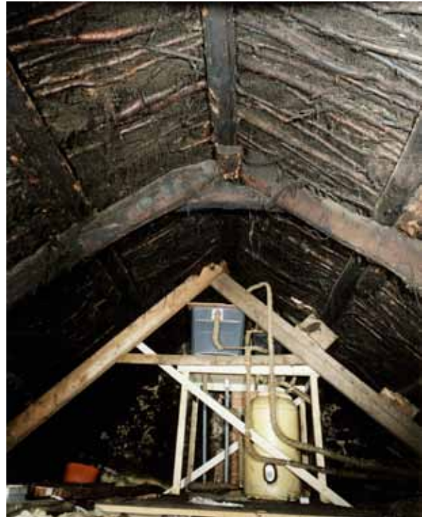
Illus. 5 The roof space 1998 (Historic Scotland)
