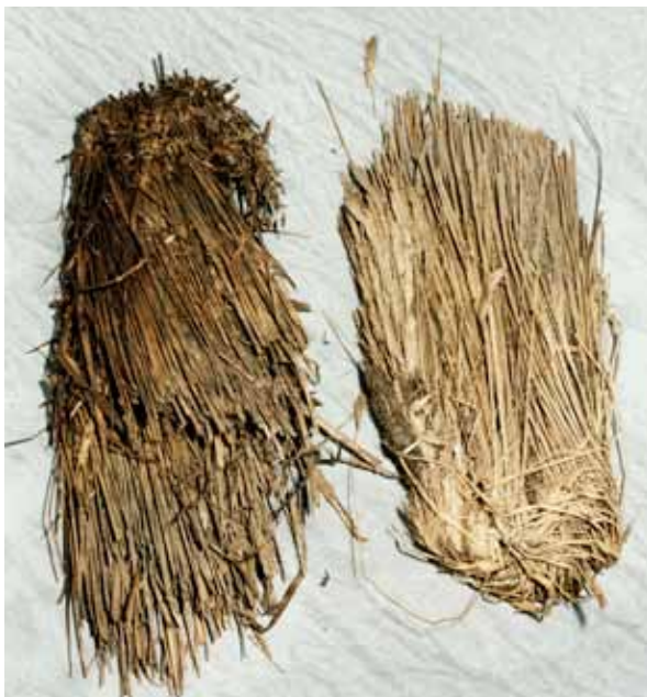
Illus. 33 Tippets or grips from the body of the roof (Historic Scotland)
