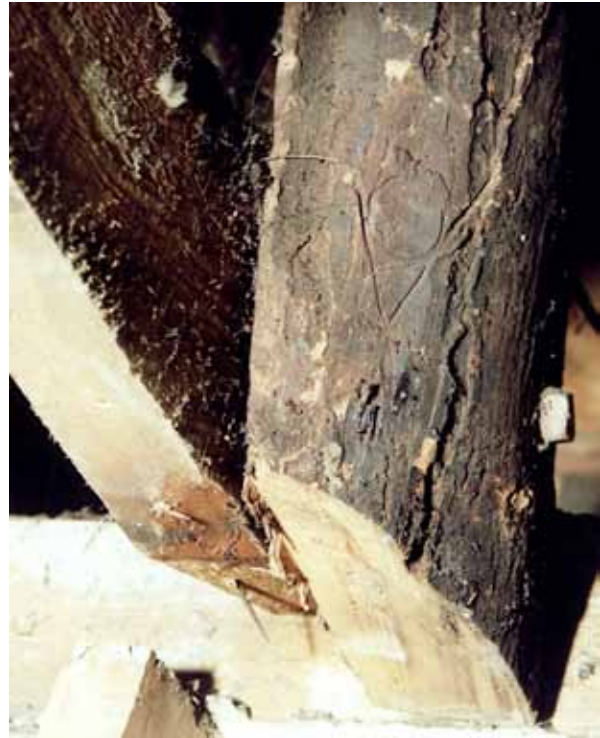
Illus. 22 Detail of timber marks – W Cuppill, N sile (Historic Scotland)
