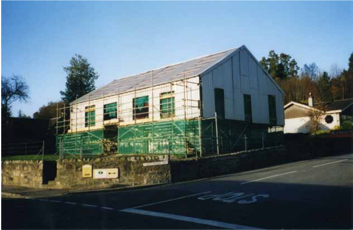
Illus. 8 The scaffolding shell
