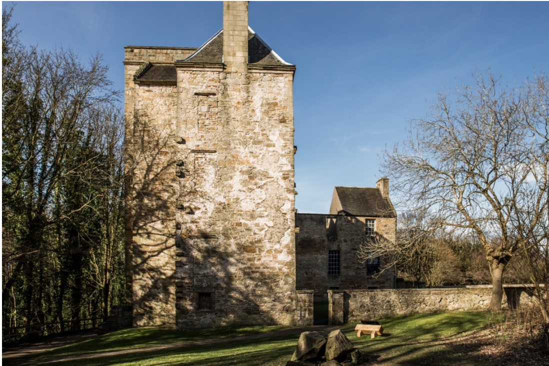
Figure 2: Kinneil House south elevation © Marcin Klimek
