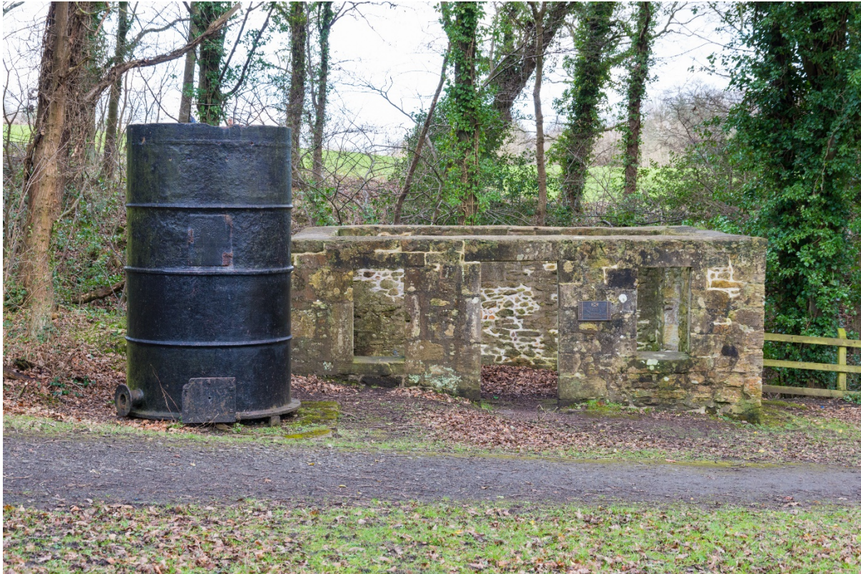
Figure 7: Kinneil Watt 'cottage' and boiler. © Historic Environment Scotland.
