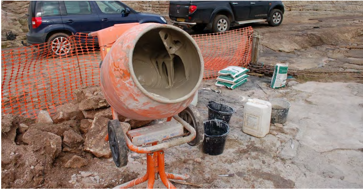
Figure 10. Mixing the grout in a small standard Belle type mixer.
