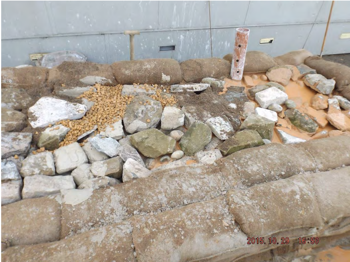
Figure 6. The trial grouting rig at the yard in Fife, prior to the pouring tests.
