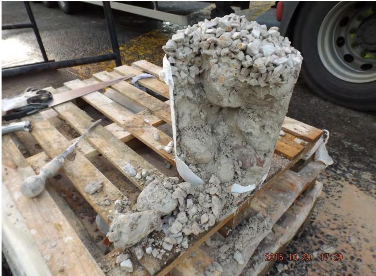
Figure 5. One of the early off-site trials to establish if larger aggregate could be transported by the grout – a wall core mock up in a large plastic bucket.
