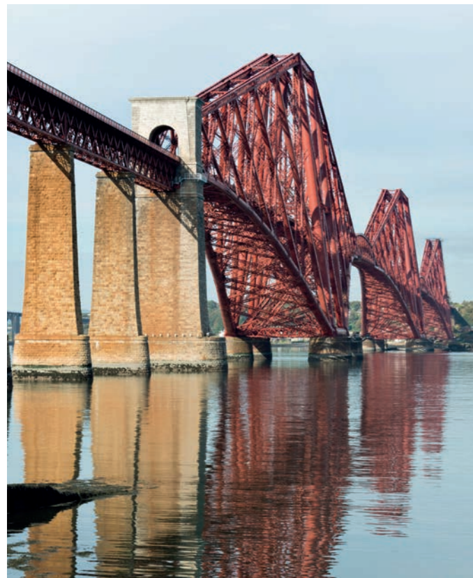
The Bridge seen from North Queensferry.
