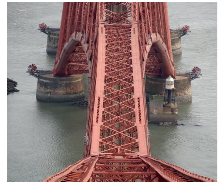
View showing the construction of the Bridge.
