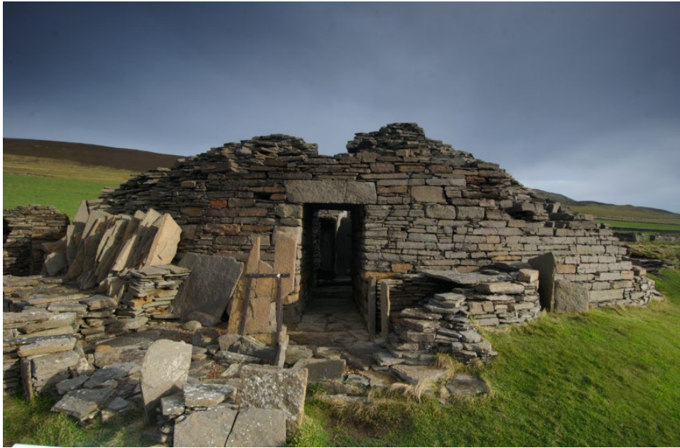
Midhowe Broch, entrance with stacked slabs to left – once thought to be evidence of buttressing, these are now interpreted as material being removed as the broch was reduced in height, and set aside for use in later building work
