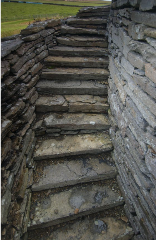
Midhowe Broch, stair
