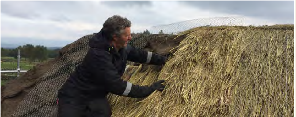
Fig. 6 Thatching a Hebridean blackhouse roof with turfes under marram.
