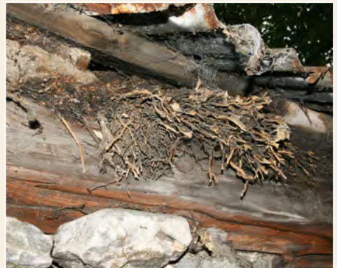
Fig. 5 Bracken and heather thatch surviving under corrugated iron, Kingussie.
