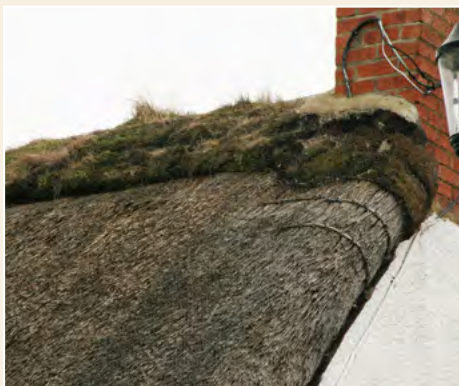
Fig. 8 Rolled skew detail, Scottish Borders.
