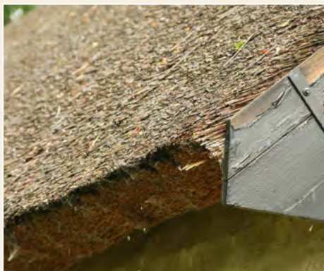
Fig. 9 Bargeboard detail, Perth and Kinross.
