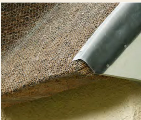
Fig. 13 Timber and lead verge detail, Perth and Kinross.
