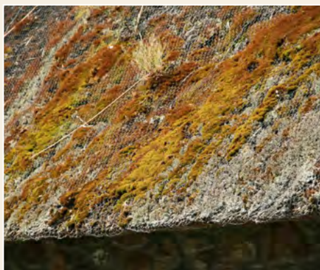
Fig 16. Moss and vegetation will eventually degrade the thatch if it is allowed to accumulate.
