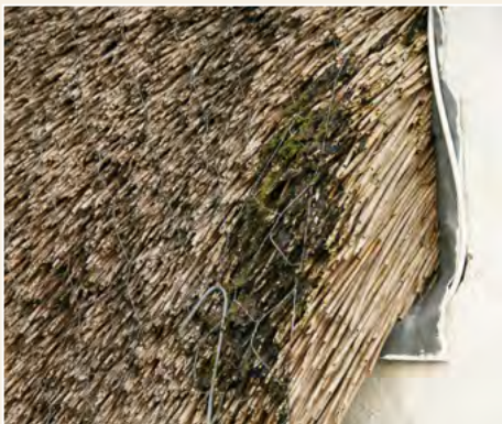
Fig. 11 Discreet lead flashing detail at chimney abutment, Western Isles.
