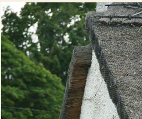
Fig. 12 Overhanging verge detail, Angus.
