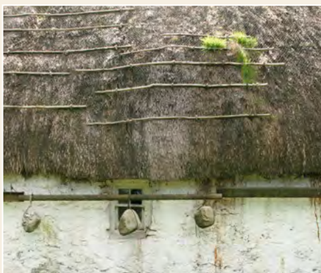
Fig. 14 Thatched cottage fixed with metal and timber poles, and weighted with field stones, Kyle, Highlands.
