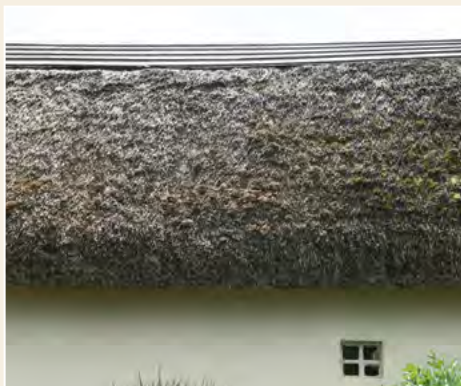
Fig. 7 Timber ridge detail, characteristic of Ayrshire.
