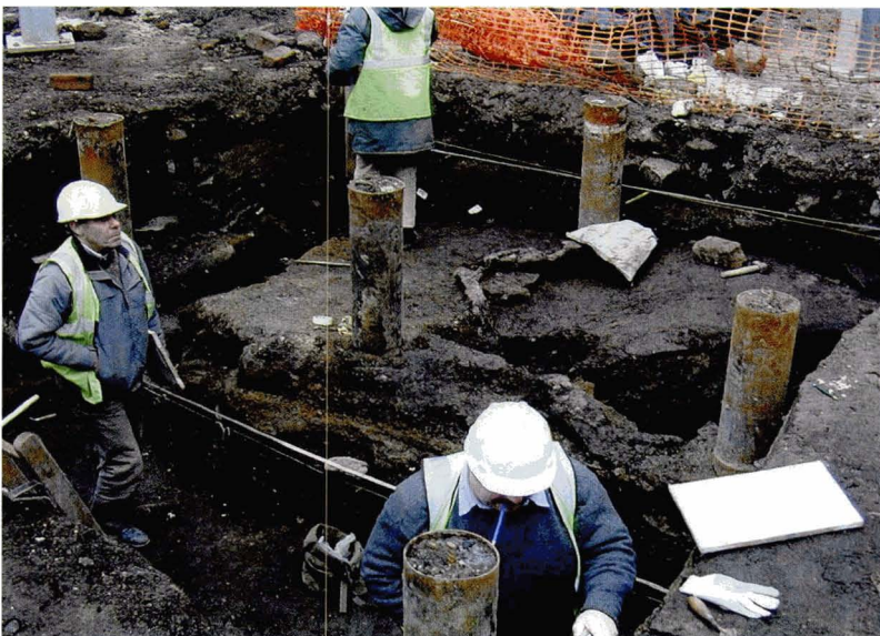
8 Skinnergate, Perth: hand excavation of new lift shaft to formation level.
