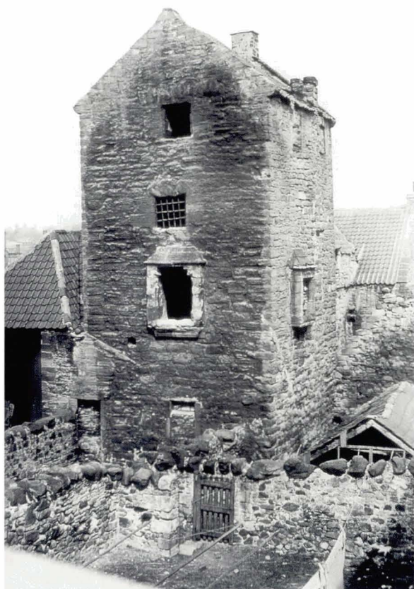
14 Town house of the Knights Hospitallers, Linlithgow. Demolished in 1885.
