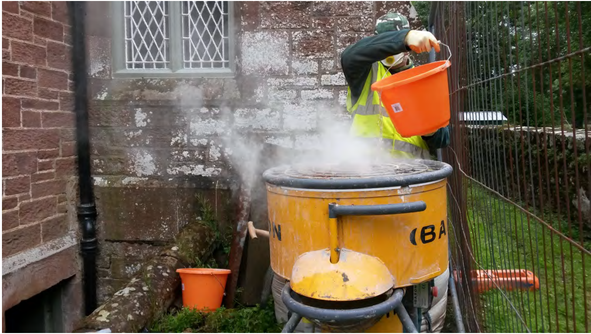
Figure 4. Addition of water during the batching of the pointing mortar.
