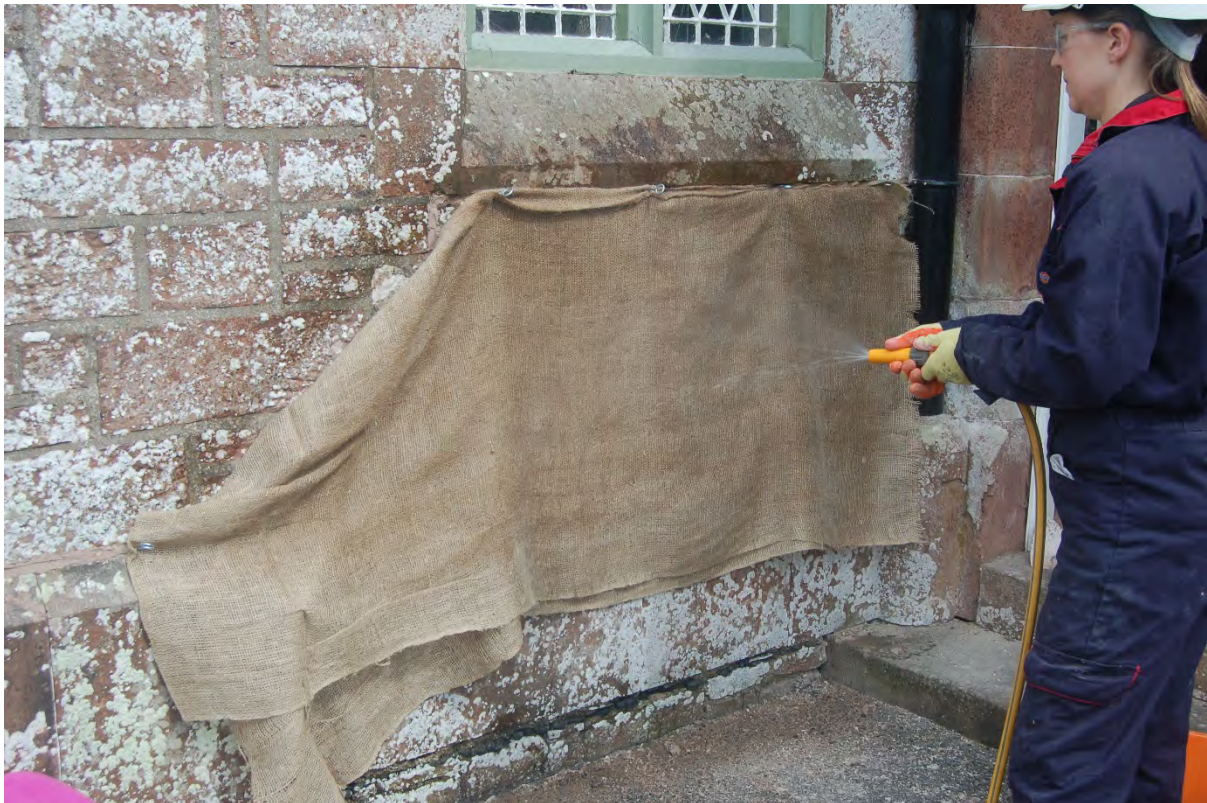
Figure 7. Finished pointing protected behind hessian. This needed wetting down for the first 24 hours while the initial set took place.
