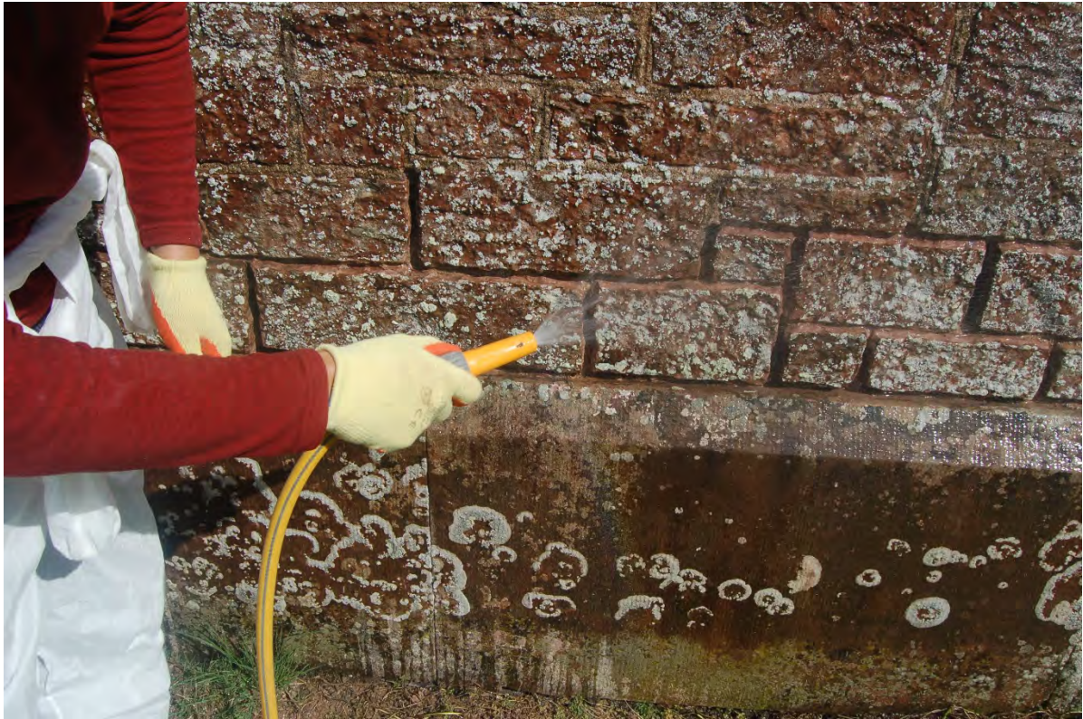
Figure 5. Cleaning the raked out joints prior to re-pointing.
