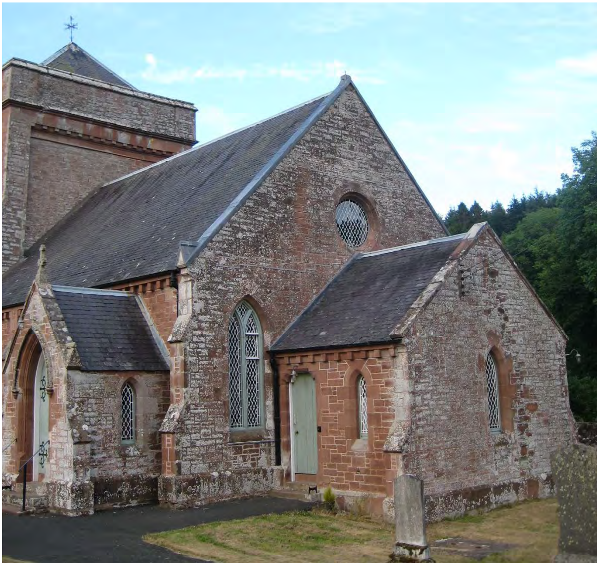
Figure 14. Hobkirk Church in 2018, demonstrating that the lime pointing work undertaken in 2013 and 2014 has held up well. Subsequent high level repairs and adaptations have also been carried out to help the building cope with increased rainfall due to a changing climate.
