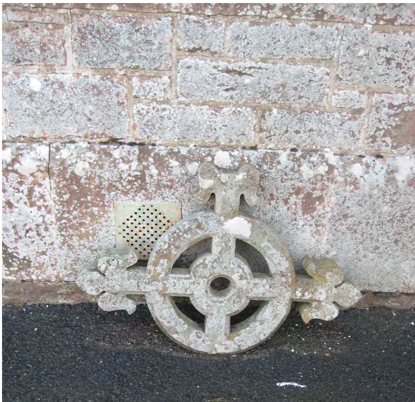
Figure 11. The finial after its repair.
