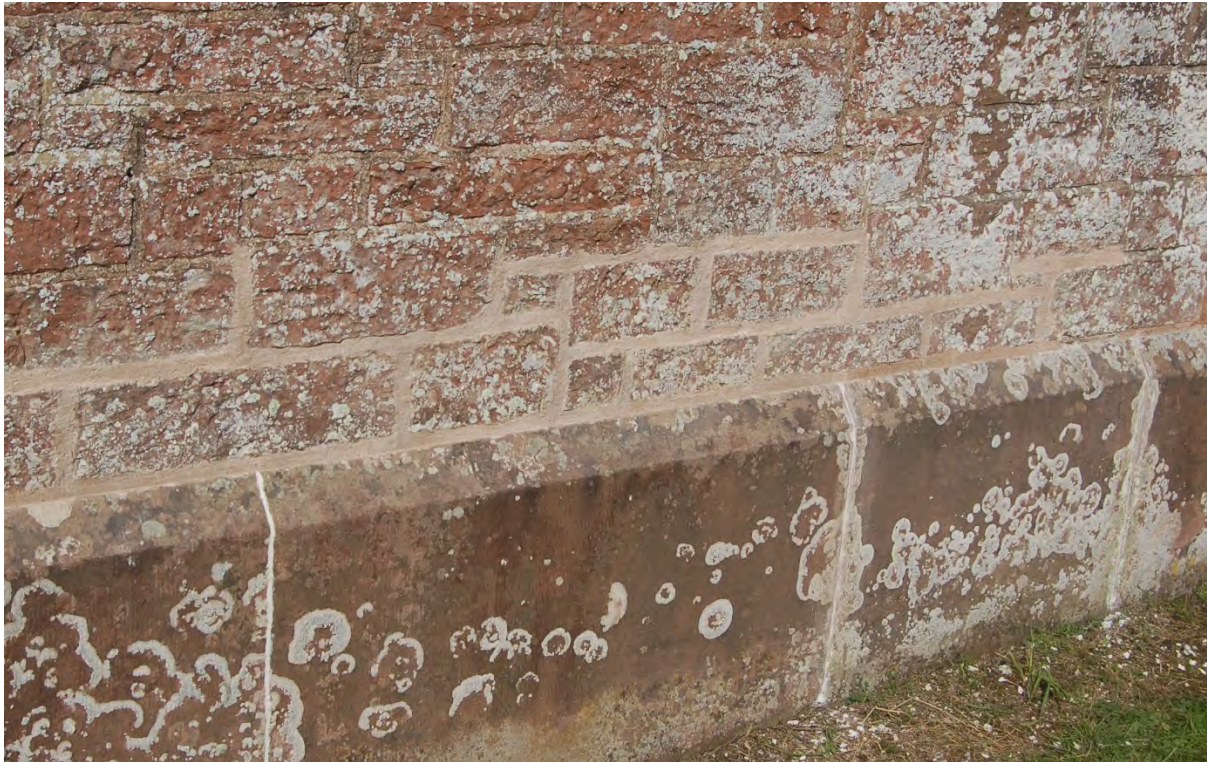
Figure 8. The finished rubble joints from the 2014 working party.
