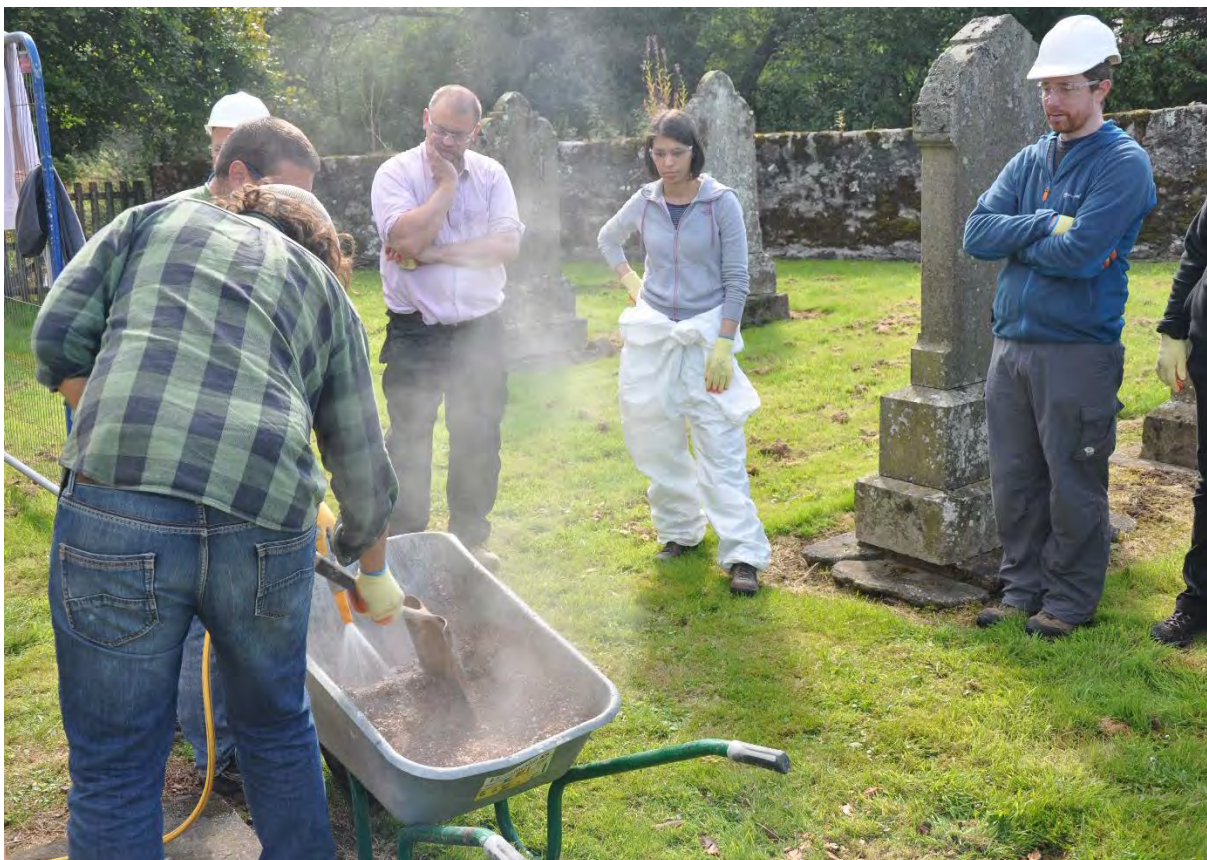
Figure 3. Demonstration of lime mortar mixing given to the volunteers prior to works commencing.
