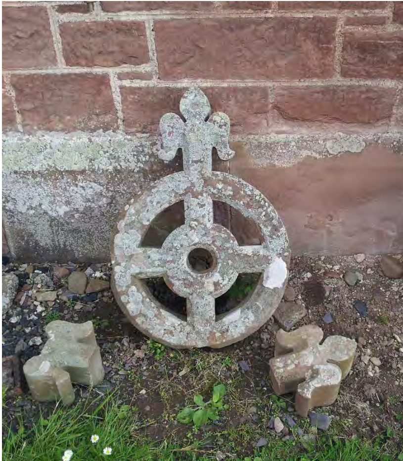
Figure 10. This decorative stone finial was carefully repaired by a stone conservator.
