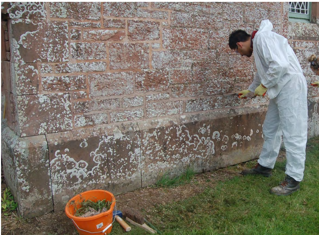
Figure 6. A volunteer re-pointing the vestry wall.
