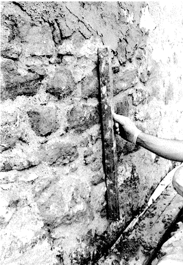
Fig. 73 Final stages of building-out.
