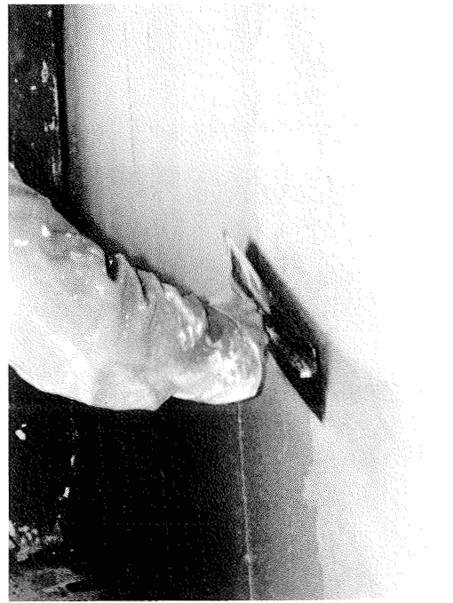
Fig. 91 Applying the finishing coat.
