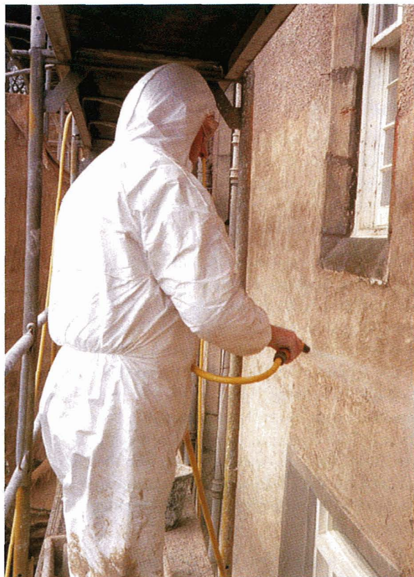
Fig. 32 Dampening-down after harling to control drying out.
