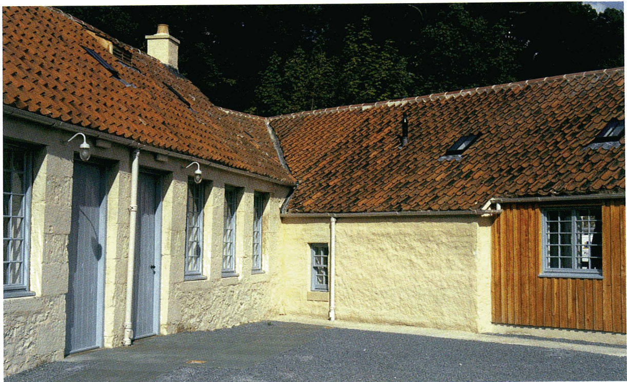
Fig. 3 Charlestown Workshop at the Scottish Lime Centre. Limewash on sandstone and new lime harling. These materials were produced by burning and slaking local limestone.
