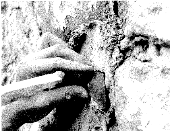
Fig. 66 Pushing pinnings into wide and eroded joints.
