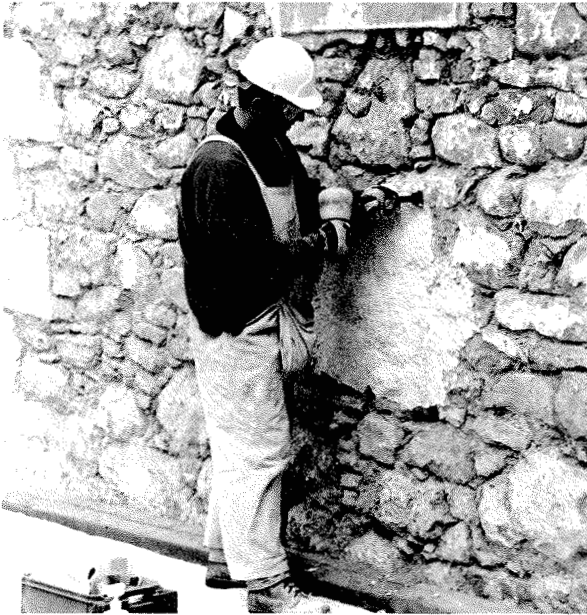
Fig. 60 Removing defective harling.
