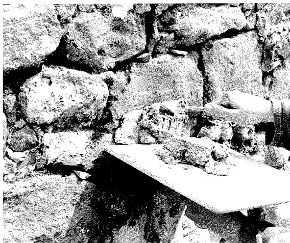
Fig. 68 Placing mortar in joints.
