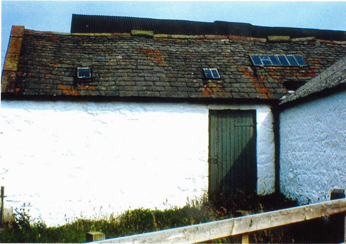
Fig. 9 Limewash on stonework.
