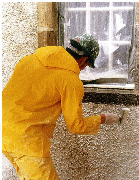
Fig. 48 Working limewash into the surface as it starts to gel.
