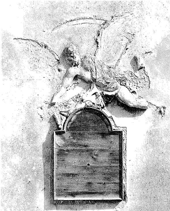
Fig. 7 Hedderwick House, 'Time' A significant example of external decorative plasterwork is recorded in photographs of the Old House of Hedderwick, near Montrose (held in the National Monuments Records in Edinburgh). Now demolished, this house of c.1700 had a lined-out smooth lime render; mimicking fine ashlar; with plaster egg-and-dart moulded window architraves, and a high relief plaster sculpture.
