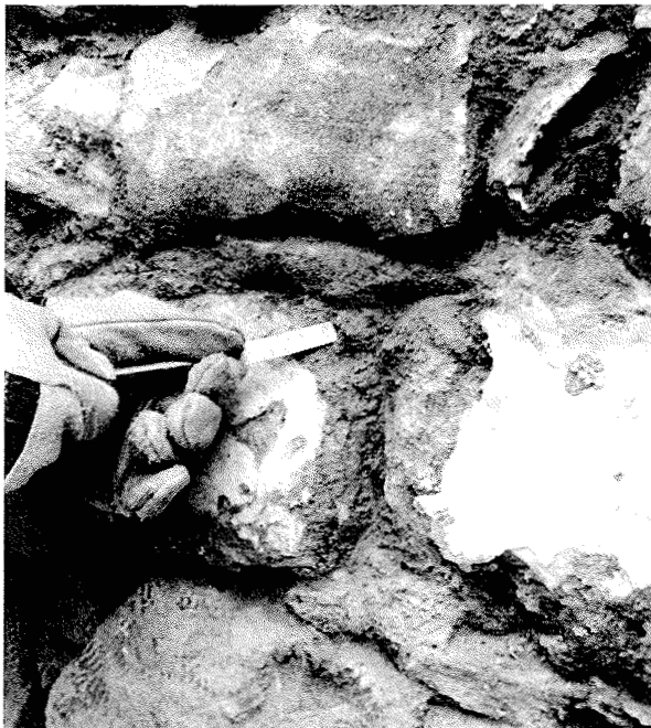
Fig. 63 Removing loose mortar from joints.
