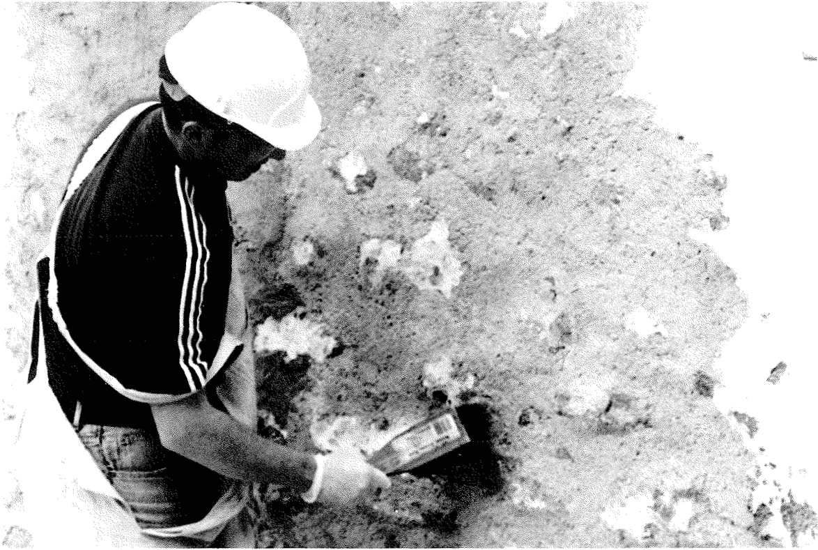
Fig. 75 Going over surface with brush after building-out.
