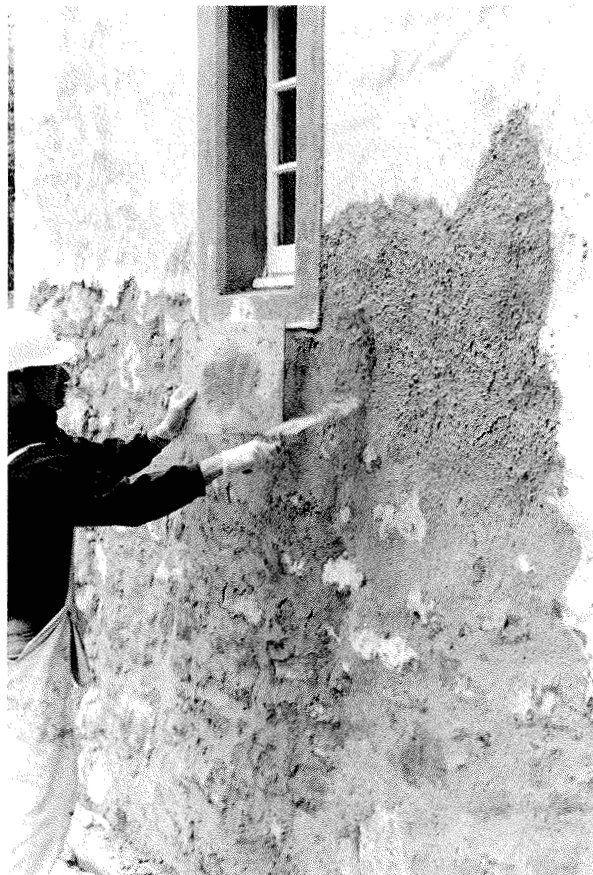
Fig. 77 Working up to a window margin.
