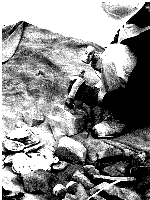
Fig. 18 Preparing a range of suitable materials from which to make pinnings.
