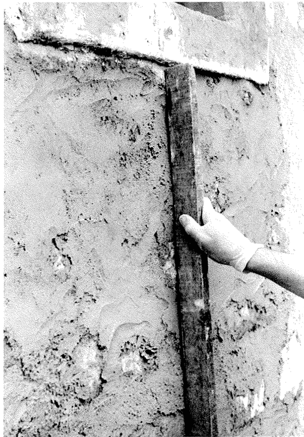
Fig. 74 Checking level of surface.
