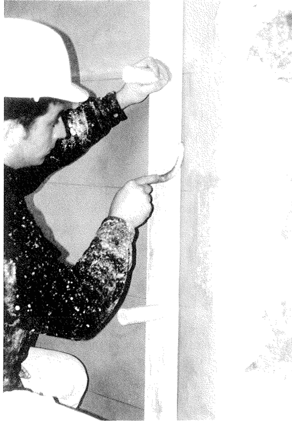
Fig. 93 Ruling in vertical joint lines. The horizontals were lined first.
