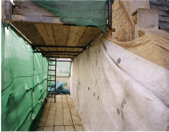
Fig. 31 Protection placed in front of new harling during cold weather.
