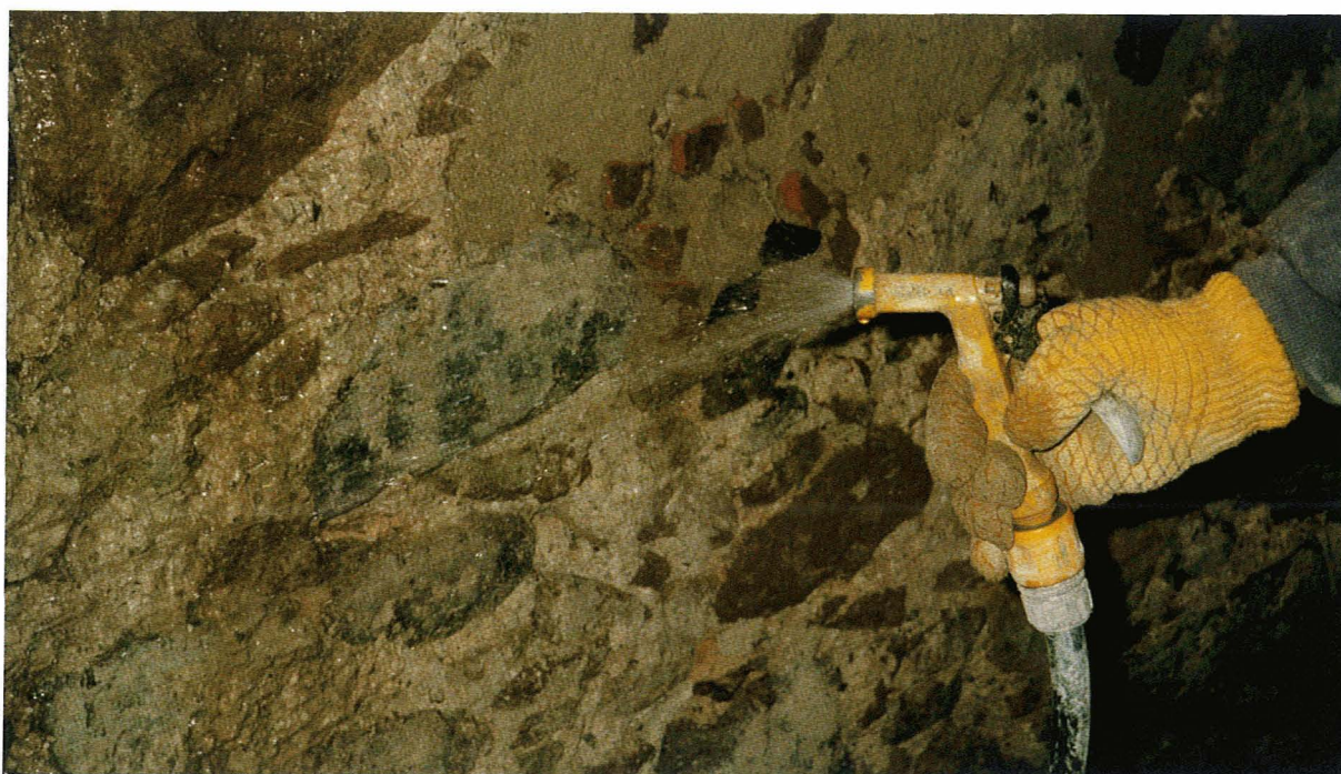
Fig. 24 Dampening down before applying coatings.
