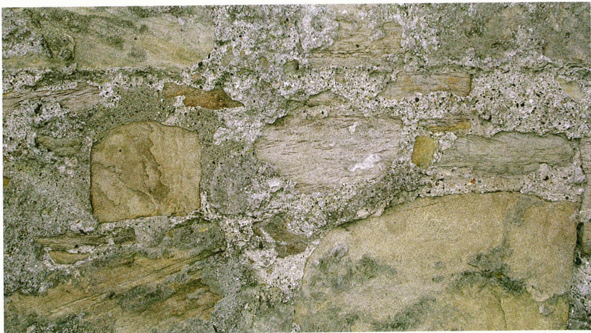
Fig. 22 Remnants of original lime harl.
