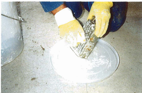
Fig. 44 Small quantities of tallow are usually added at the slaking stage to ensure good dispersion throughout the limewash.
