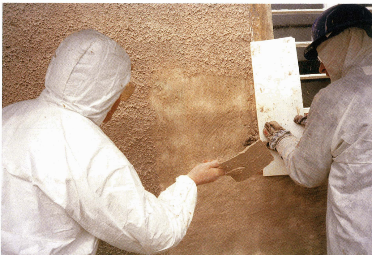
Fig. 27 Working up to dressed stone. Note safety protection worn by operatives.
