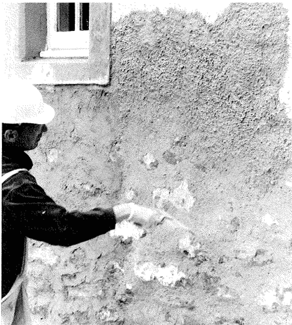
Fig. 76 Forehand casting action.
