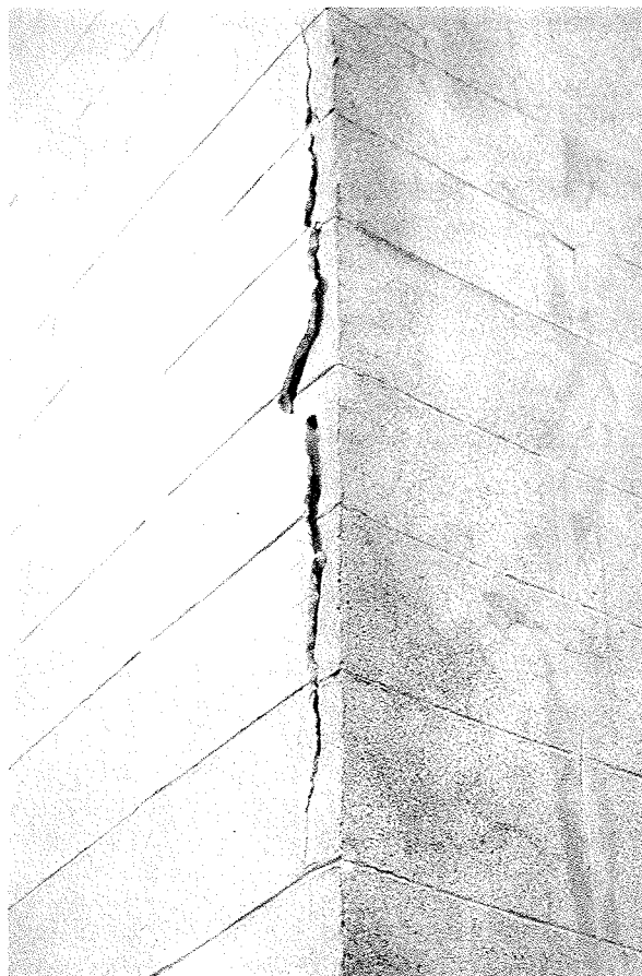
Fig. 14 Cracked modern portland cement render.
