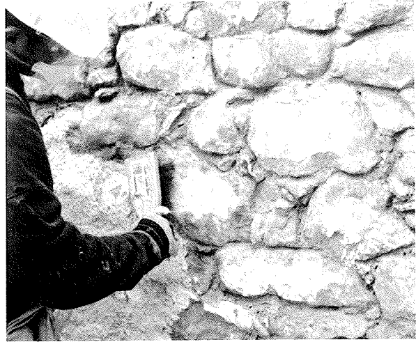
Fig. 65 Brushing down to remove any dust.
