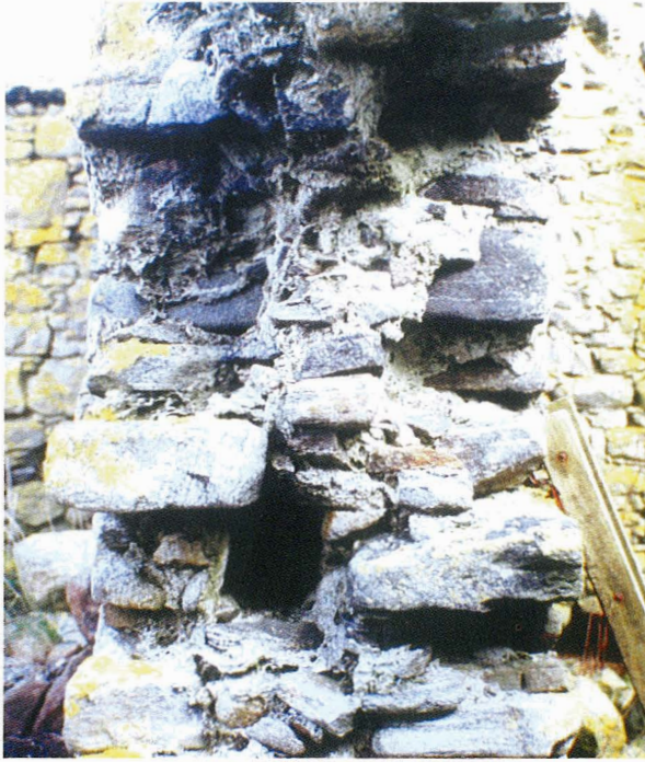
Fig. 10 Traditional masonry wall construction.
