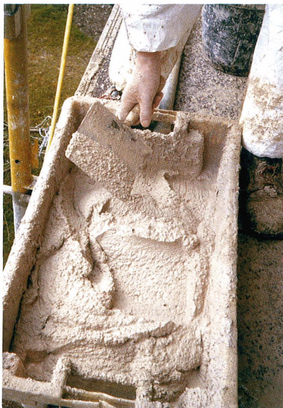
Fig. 25 The consistency of mortar suitable for harling.
