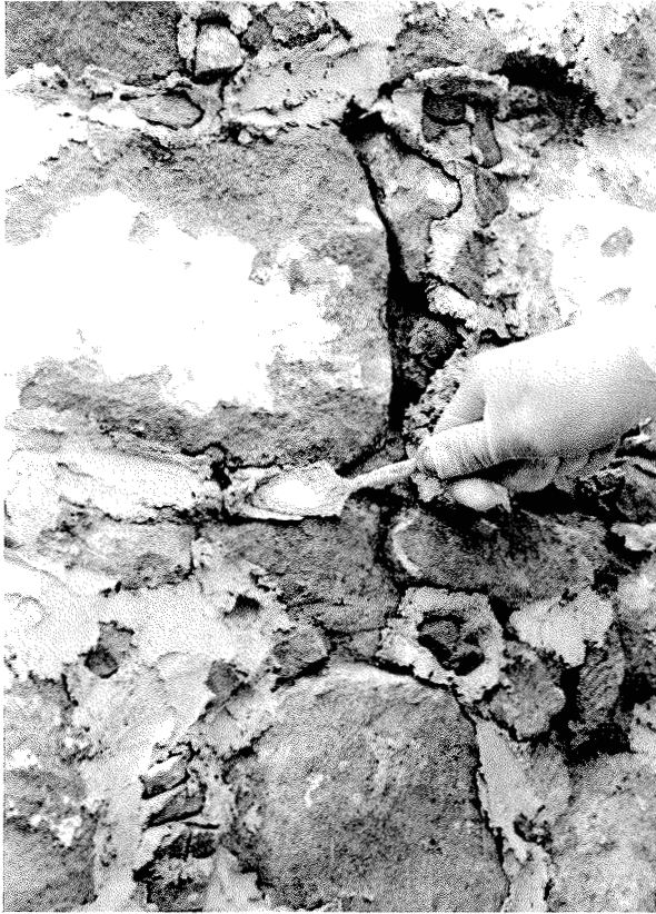
Fig. 71 Working over pinnings.
