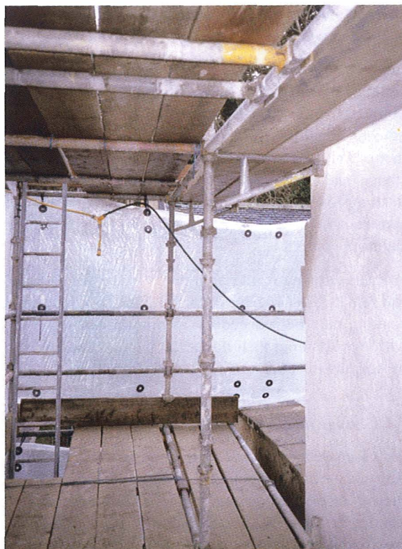
Fig. 56 Outer protection to the scaffold. Note also the water distribution pipework.
