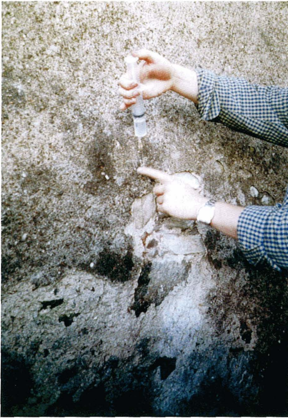
Fig. 30 Specialist technique of grouting voids behind loose coatings.
