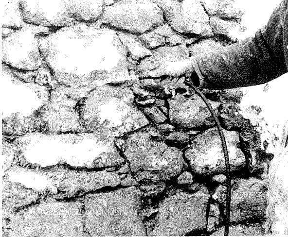
Fig. 64 Washing down the surface to remove any loose material.
