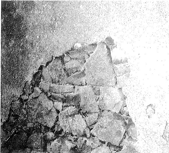
Fig. 5 'On the outside they fill up the interstices by driving in flat stones of a small size, and in the end, face the work all over with mortar thrown against it with a trowel, which they call harling'. (North of Scotland 1754: Dictionary of the Scottish Language Vol. II p.536)
