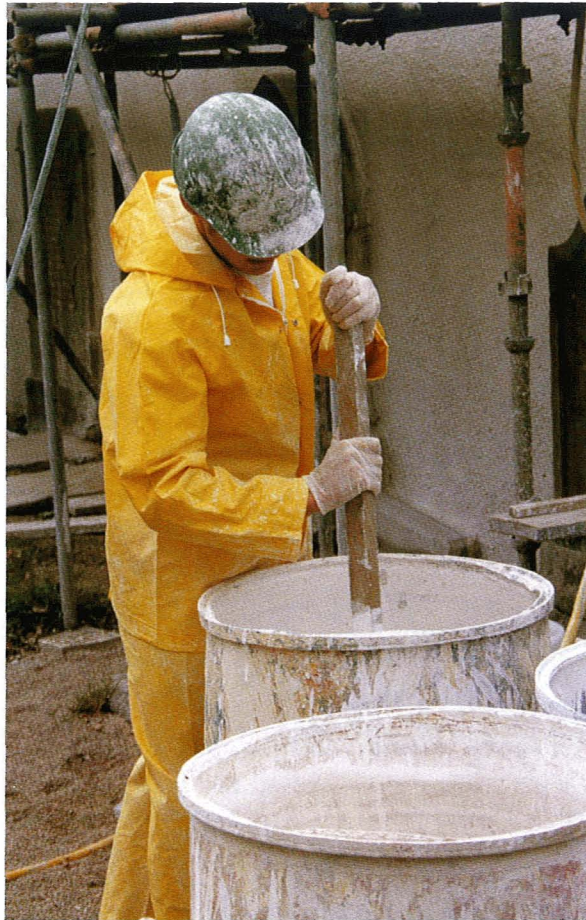
Fig. 46 Mixing a limewash to ensure an even consistency.
