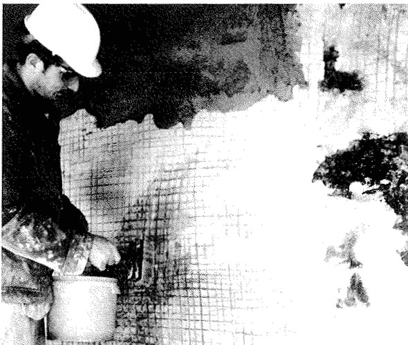
Fig. 87 Damping down to test suction.
