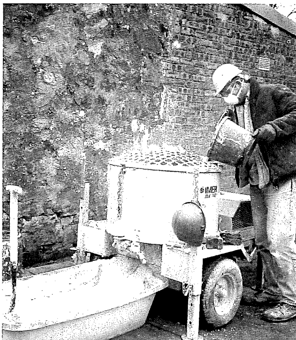
Fig. 20 Quicklime being slaked with aggregates in a paddle mixer. The 'hot lime' mortar was for immediate use.
