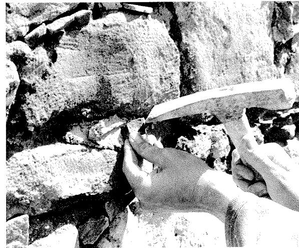
Fig. 69 Placing pinnings into joints.
