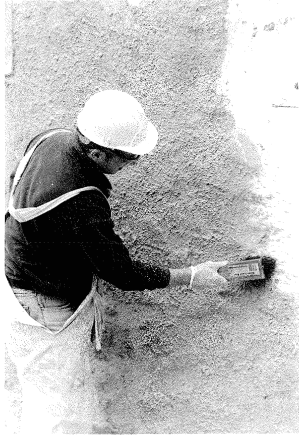
Fig. 79 Working up to existing sound work.
