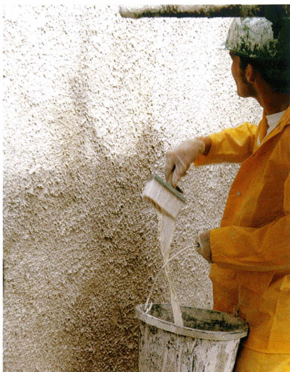
Fig. 47 Limewash should normally have a thin consistency and be liberally applied. The use of goggles is recommended.
