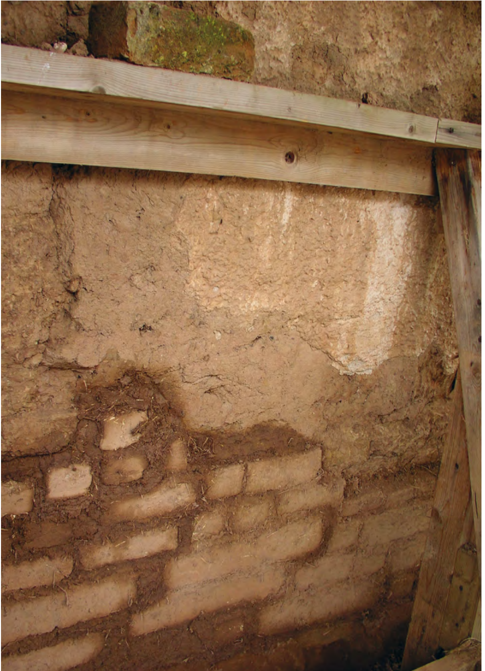
Fig. 9 Earth block repairs can be an appropriate solution where it is not possible to replicate original methods of construction.
