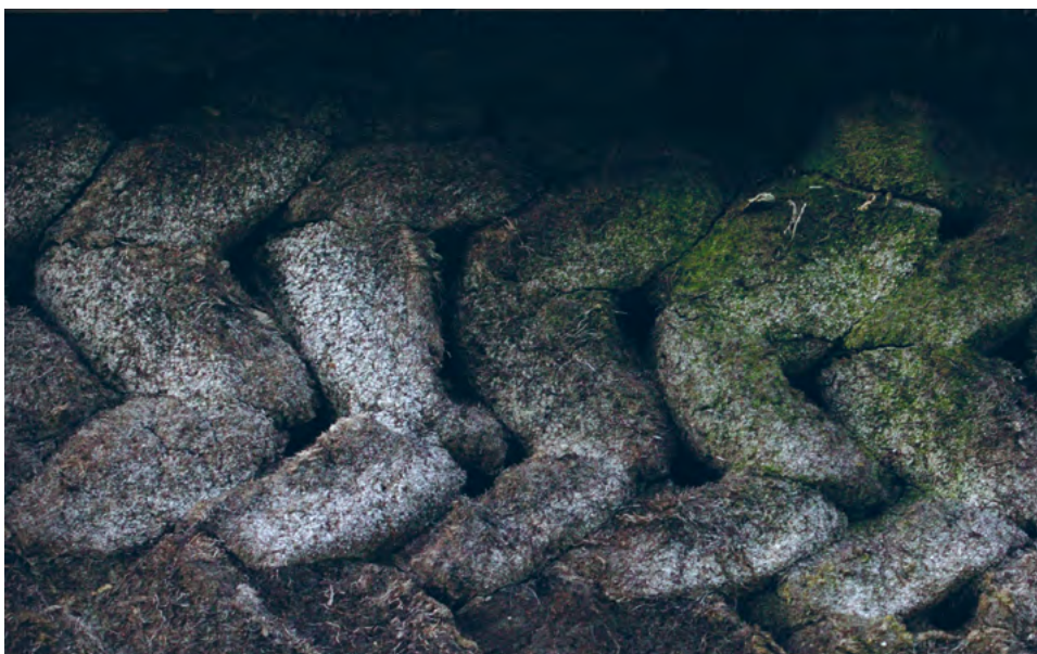
Fig. 3 Turf was commonly laid in a herringbone pattern for added strength.
