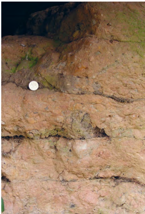
Fig. 1 Mudwall built up in short lifts, Dumfriesshire.
