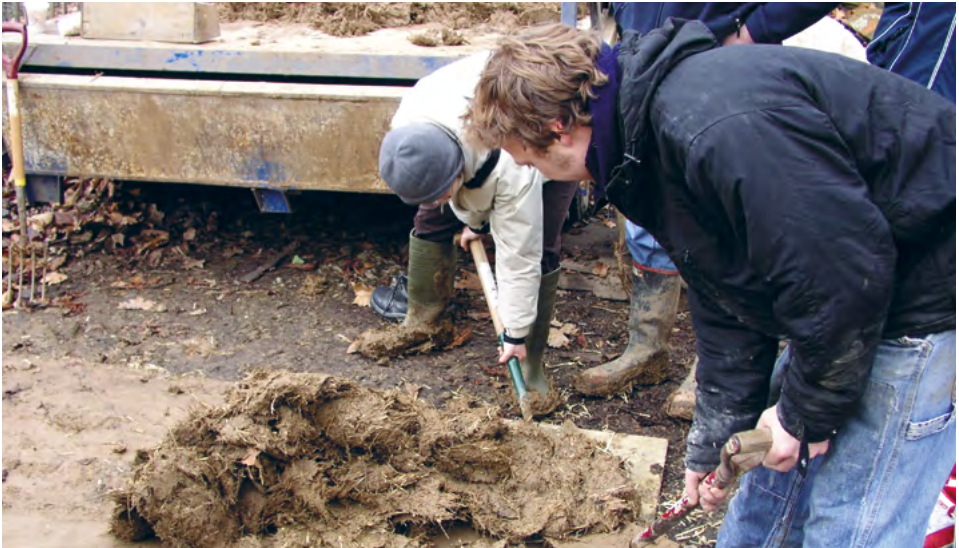
Fig. 5 Hand mixing of earth building material containing plant fibres.
