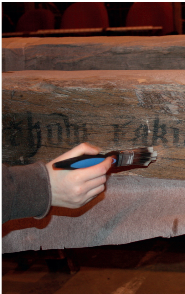
Figure 4 Size glue being applied through Japanese tissue paper to one of the Carnock House beams.
