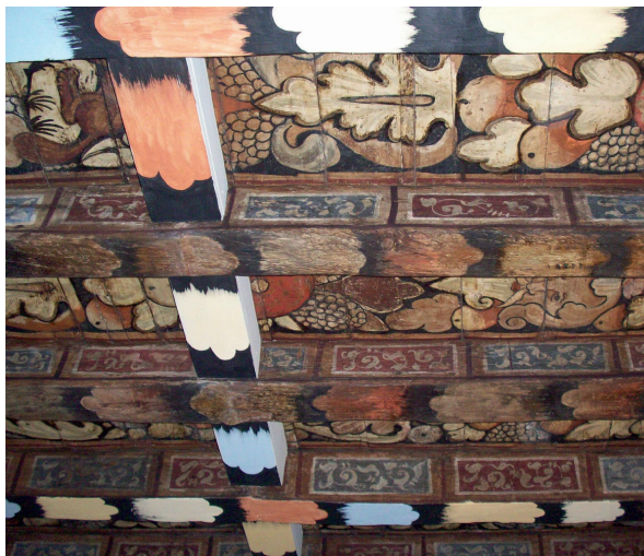
Figure 23 Floor 3, Lawnmarket: boards space-filling floral, beams with framed arabesques and trailing tassels, restored (SWPG)
