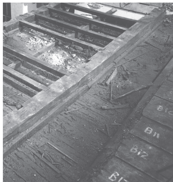
Figure 3 Abbey Strand: the small painted beams jointed between the larger painted beams. Some of the boards examined in this study can be seen in the right-hand corner.
