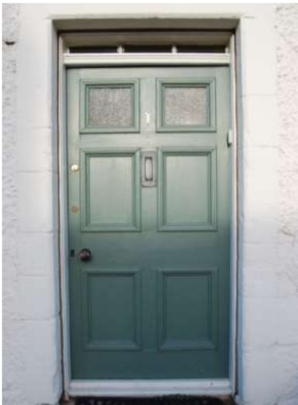
Fig. 16: External front door with wooden threshold to prevent driving wind and rain ingress at the periphery.
