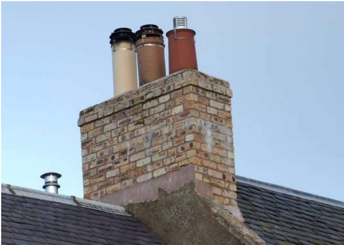
Fig. 10: New chimney stack built used reclaimed colliery brick.
