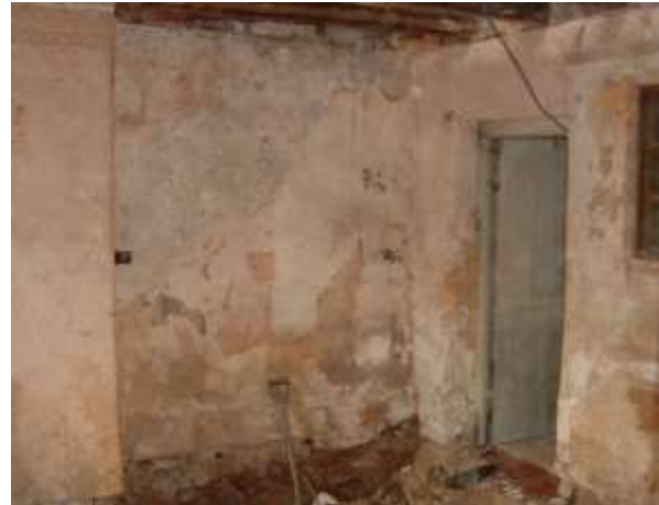
Fig. 26: Master bedroom works to re-plaster on the hard.
