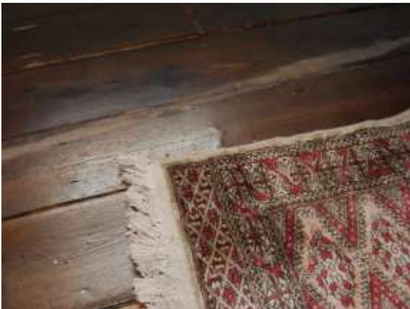
Fig. 19: Existing timber floor boards were re-laid.
