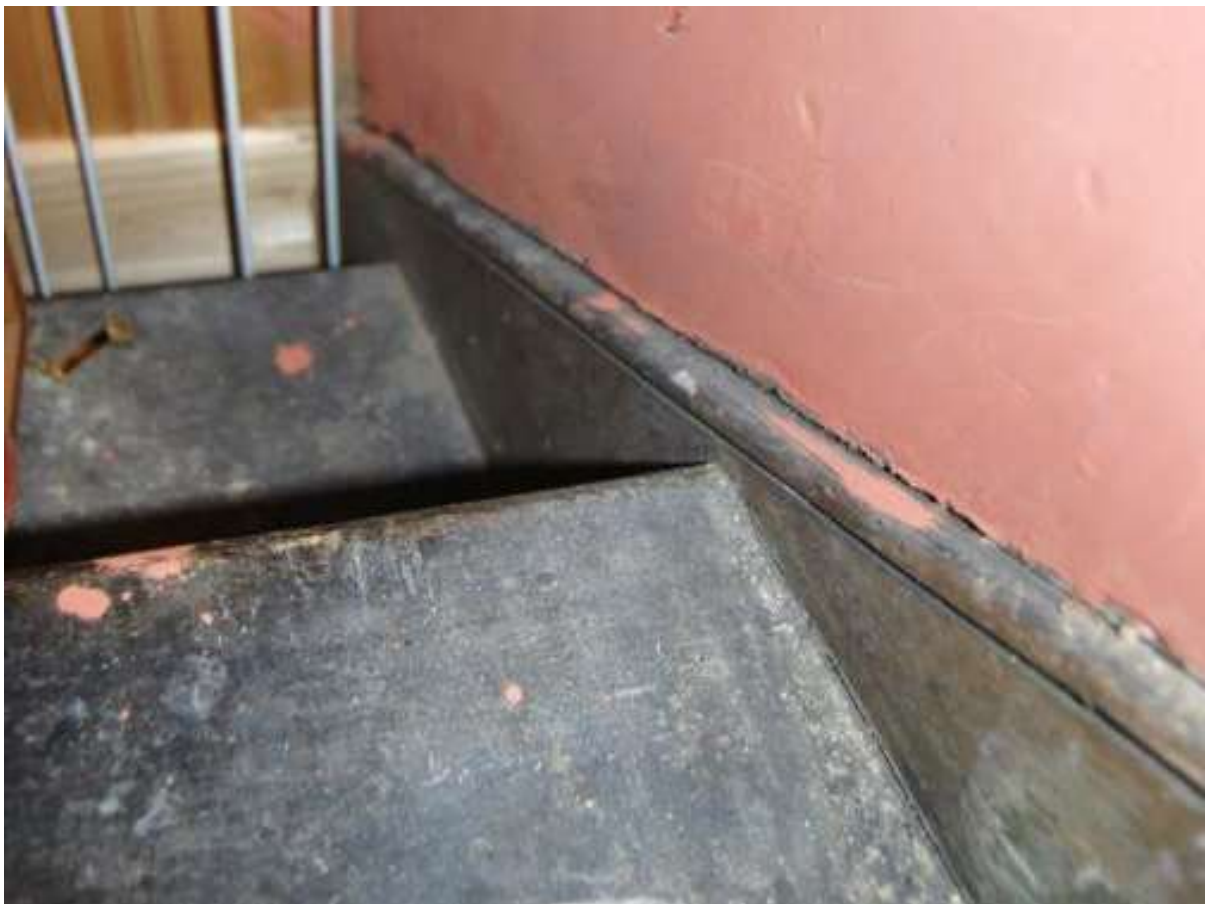
Fig. 3: Former stairs adjoining terrace to neighbouring property.
