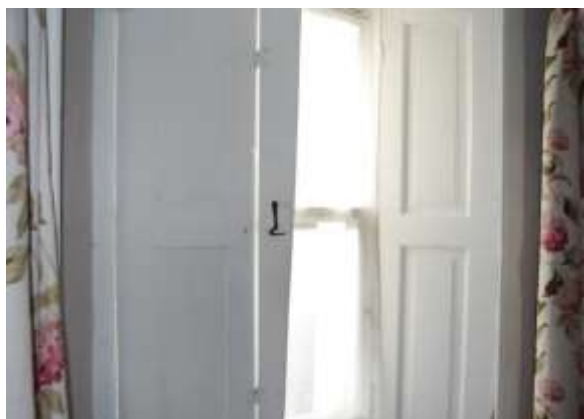
Fig. 27: Existing timber window shutters restored.
