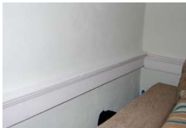
Fig. 28: Existing timber dado rails restored.
