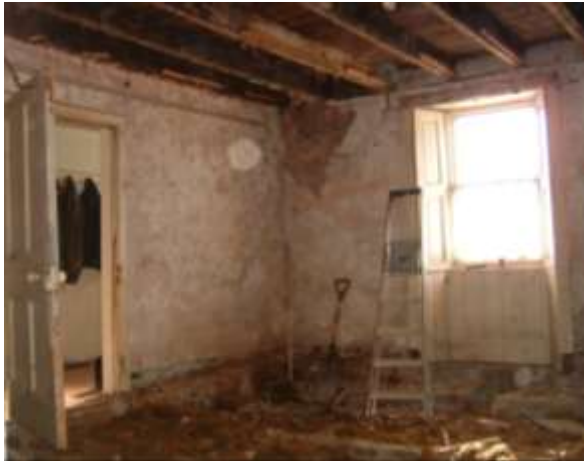
Fig. 25: Master bedroom works to re-plaster on the hard.
