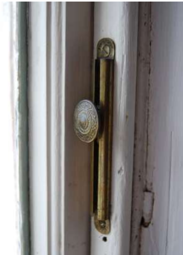
Fig. 31: Existing ironmongery cleaned and reused.
