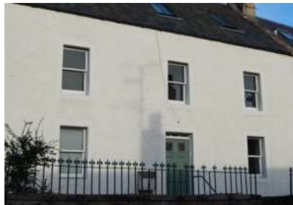
Fig. 13: Traditional mineral paint used on the principal façade.
