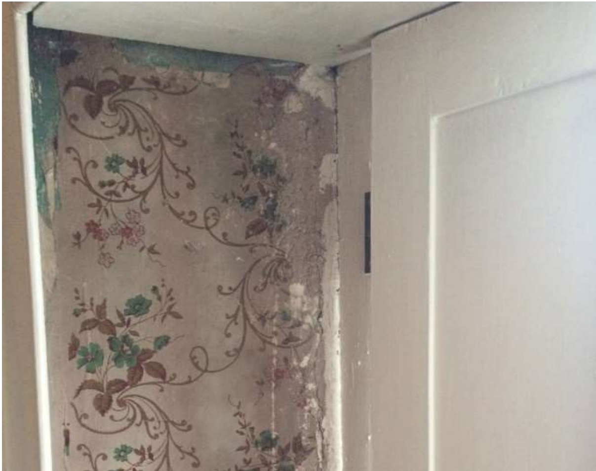
Fig. 33: Existing wallpaper retained behind sitting room timber window shutter.
