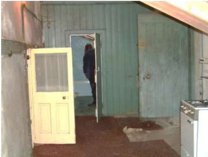
Fig. 1: Existing kitchen space located in later lean-to extension.
