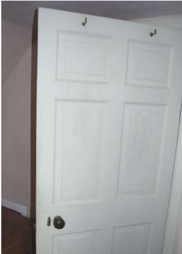
Fig. 29: Existing panelled doors restored.
