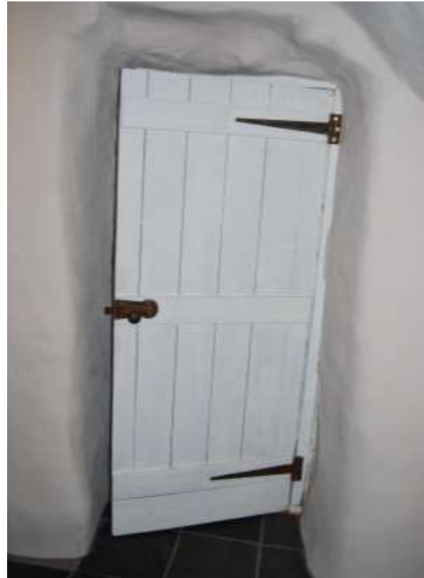
Fig. 30: Existing plain boarded doors restored.
