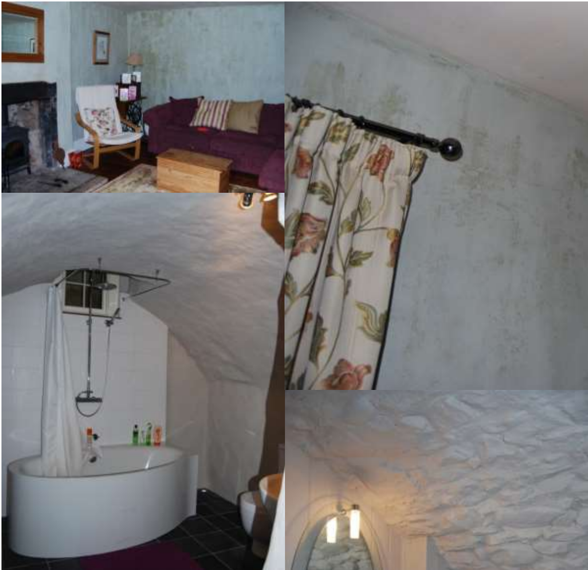
Fig. 32: Decoration works including: lime paint in the sitting room and clay paint in the cellar bathrooms.
