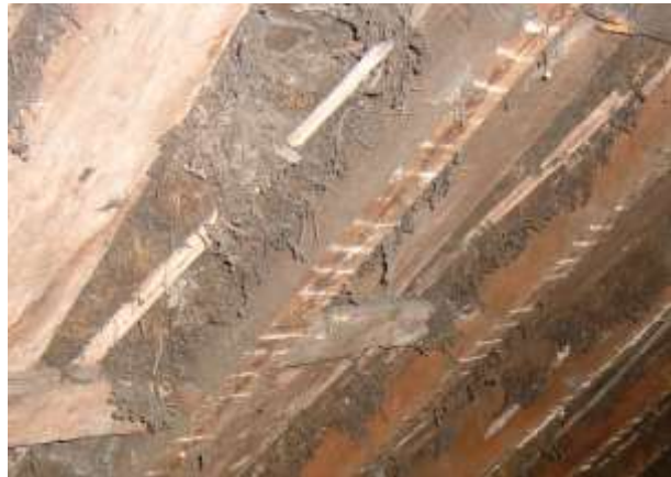
Fig. 18: Dried packed heather (grey colour) revealed in the floor zone.
