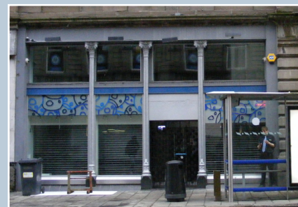
One of the cast-iron shopfronts that came to light during recent refurbishment of Dundee's Improvement Act streets.
