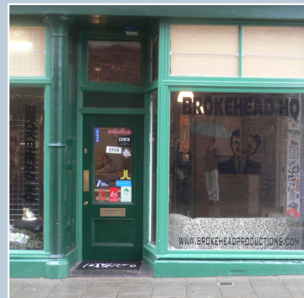
A shopfront restored through the Arbroath Townscape Heritage Initiative.
