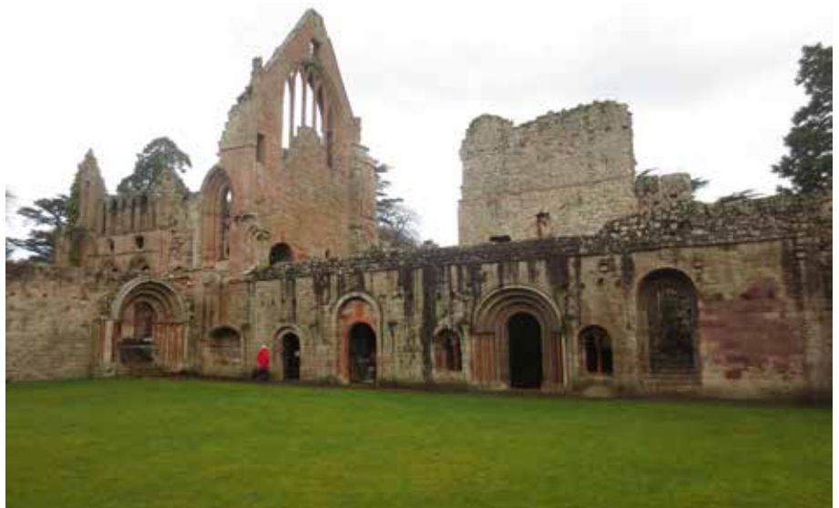
P01d Cloister looking towards south transept and east range
