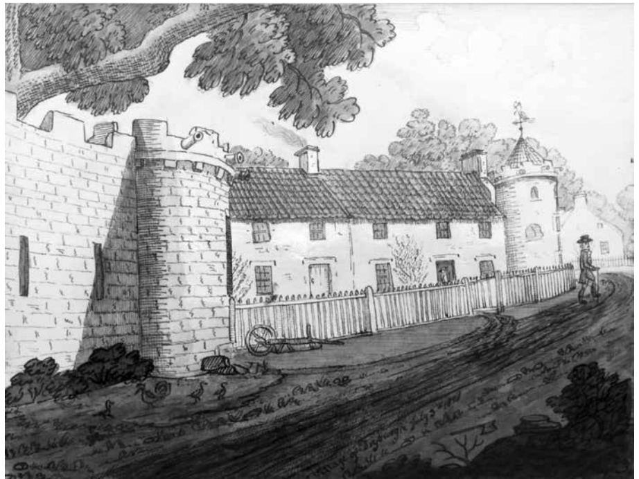
DSE sketch 11 of Stirling cottages and tower, with corner tower of Orchard field wall on the left
