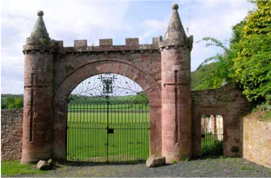
B16, B16a Orchard gate with part of Orchard Field walls
