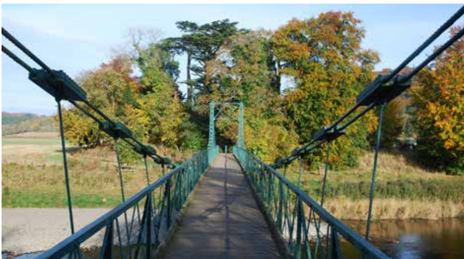
B23 Dryburgh suspension bridge and Bass hill
