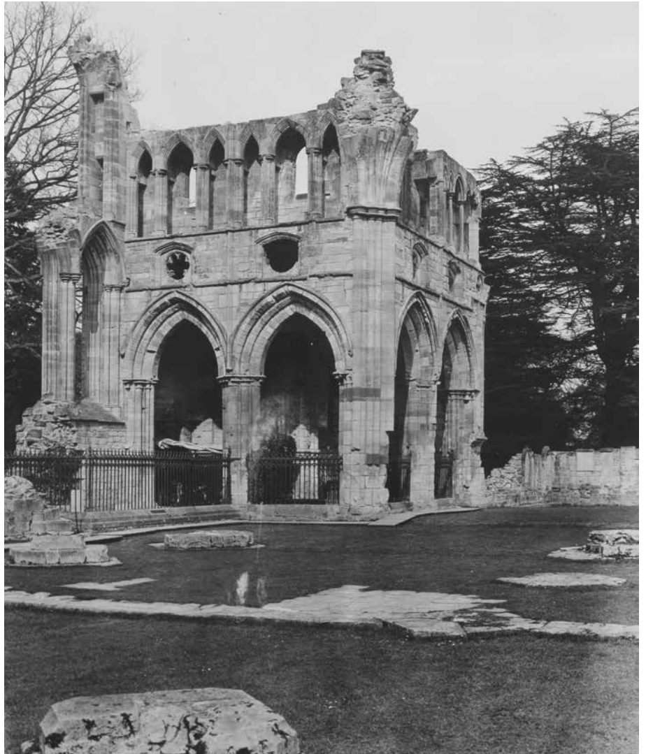
Apx 4.23 Early 20thC North transept from south-west of nave
