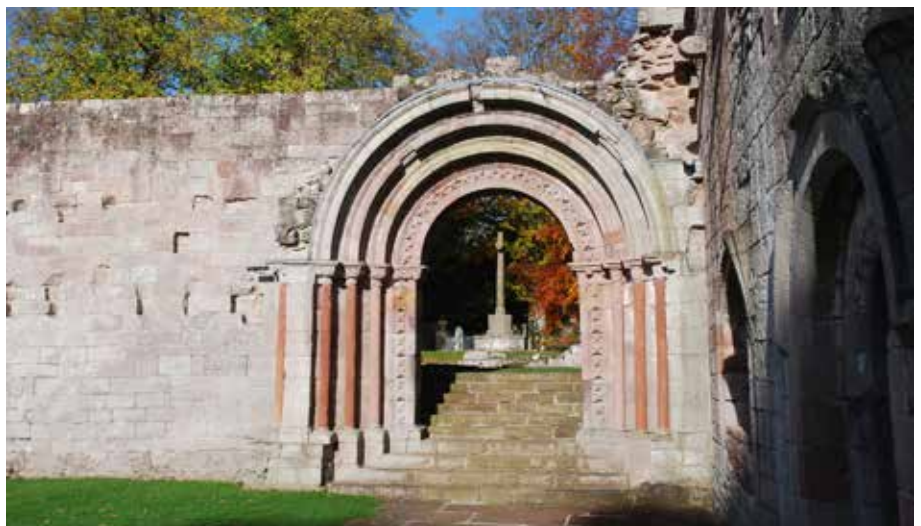
B01 Dryburgh Abbey, processional door between cloister and nave
