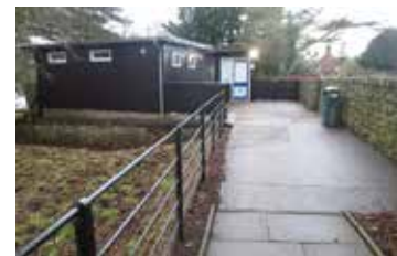
B01d Custodian's office and shop
