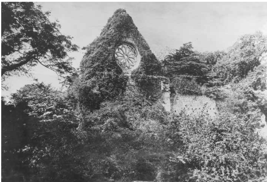
Apdx 4.13 Mid 19thC St Catherine's window, overgrown state
