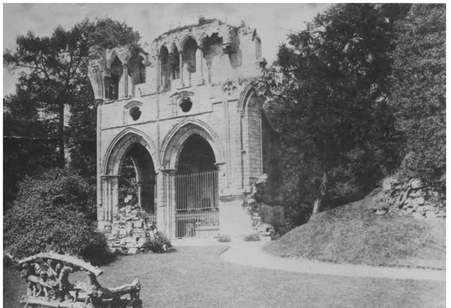
Apdx 4.18 Late 19thC North transept from south-east
