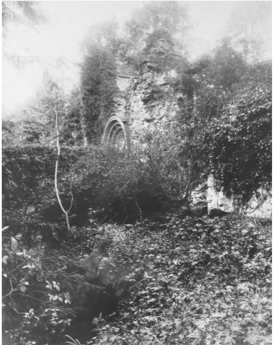
Apdx 4.14 Mid 19thC West door, overgrown state
